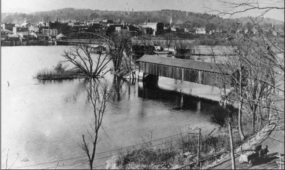
FIGURE 2: Hinsdale "Little River" Covered Bridge over east channel during high water event sometime between 1903 and 1920. Note truss over main channel, built 1903, in background (Cheshire County Historical Society).
