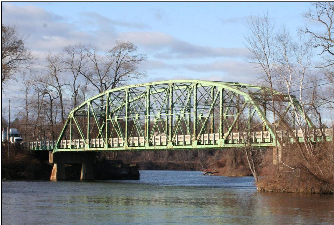
FIGURE 1: Hinsdale Bridge, built 1926. Downstream side from New Hampshire shore (Historic Documentation Co. Inc. 2012).
