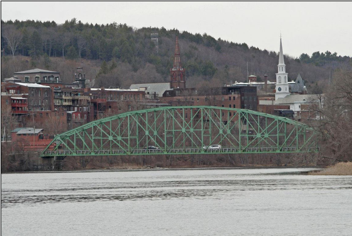
FIGURE 1: Hinsdale-Brattleboro Bridge, built 1920. Downstream side, from New Hampshire shore, with city of Brattleboro, Vermont in background (Historic Documentation Co. Inc. 2012).
