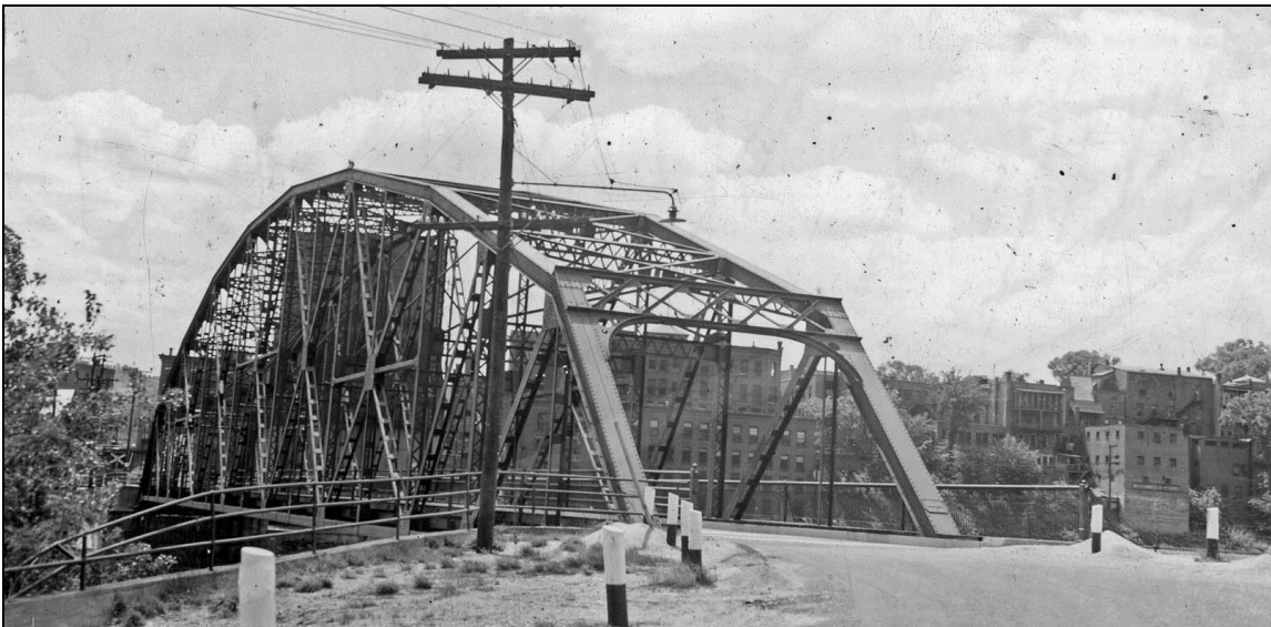
FIGURE 7: Hinsdale-Brattleboro Bridge, built 1920, looking toward Brattleboro (NHDOT 1941).
