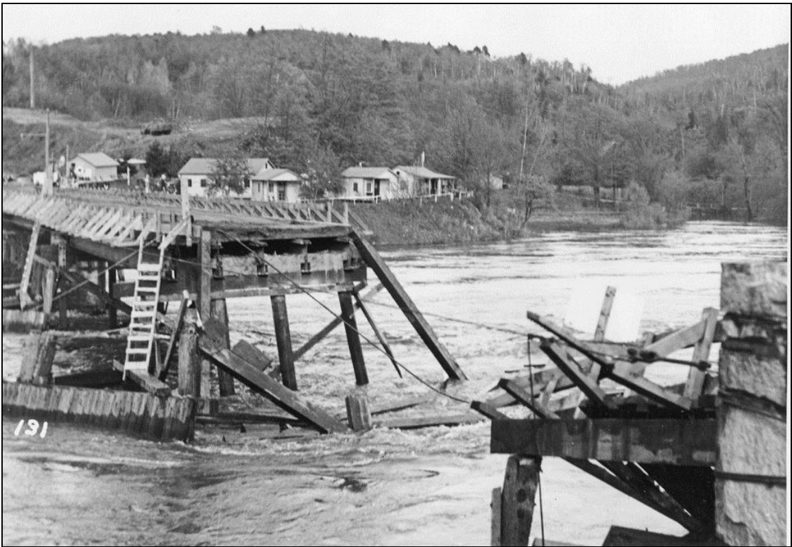
FIGURE 11: Photo, 1937, showing section of temporary wood trestle bridge washed out (NHDOT 1941).
