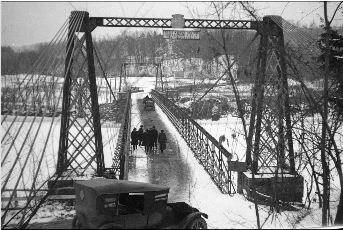
FIGURE 6: Chesterfield-Brattleboro Suspension Bridge in 1922 (Storrs 1922).
