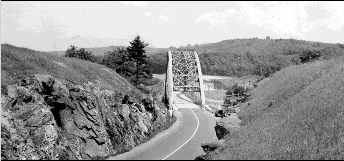
FIGURE 14: Chesterfield-Brattleboro Arch Bridge, completed 1937, Vermont end shown in 1941 (NHDOT 1941).
