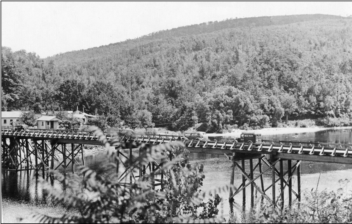
FIGURE 10: Photo, 1937, showing traffic passing over temporary wood trestle bridge erected after 1936 flood (NHDOT 1941).
