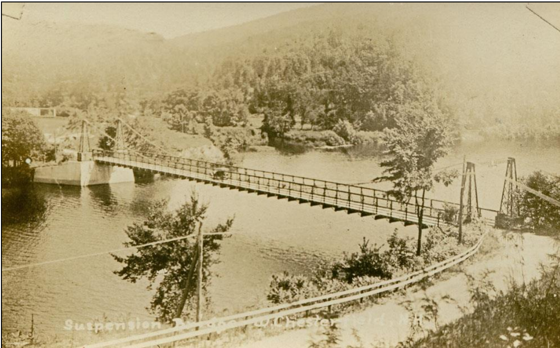
FIGURE 4: Chesterfield-Brattleboro Suspension Bridge (Chesterfield Historical Society).
