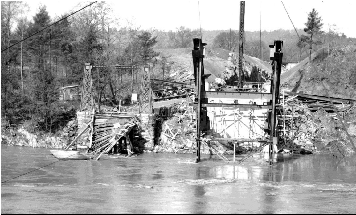
FIGURE 8: Photo, 1937, showing at left, remains of 1888 suspension bridge destroyed by 1936 flood, and at right, the initial construction of steel arches for Chesterfield-Brattleboro Arch Bridge (NHDOT 1941).
