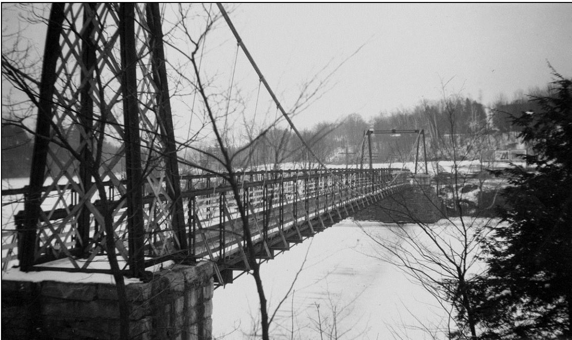
FIGURE 7: Chesterfield-Brattleboro Suspension Bridge in 1922 (Storrs 1922).
