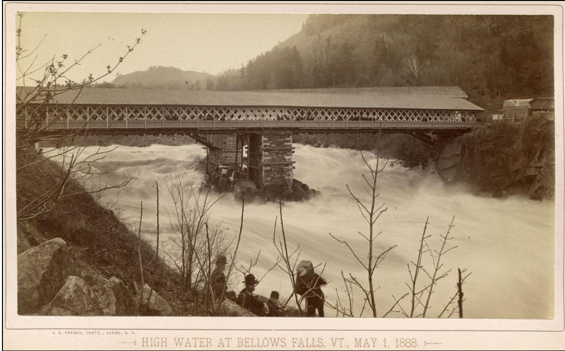
FIGURE 5: Tucker Bridge photographed in 1888 by J. A. French of Keene, NH. Note photographer at center foreground (Cheshire County Historical Society).
