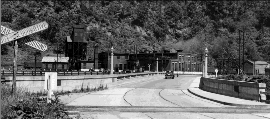
FIGURE 9: Vilas Bridge in 1941 from Vermont side (NHDOT 1941).
