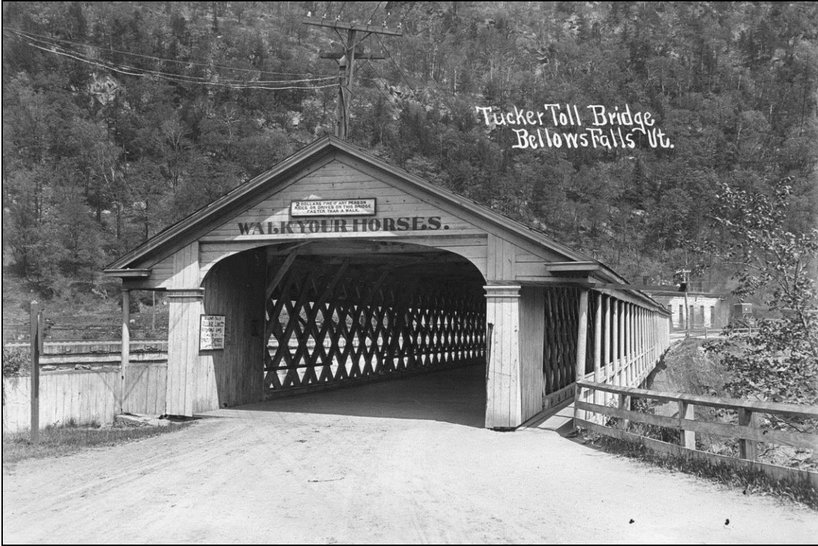
FIGURE 7: Tucher Bridge, Bellows Falls end, shown sometime after 1902. Sign above portal reads: "2 dollars fine if any person rides or drives on this bridge faster than a walk." Sign on wall reads "Bellows Falls Village Limits Automobile Laws will be Strictly Enforced (Cheshire County Historical Society).
