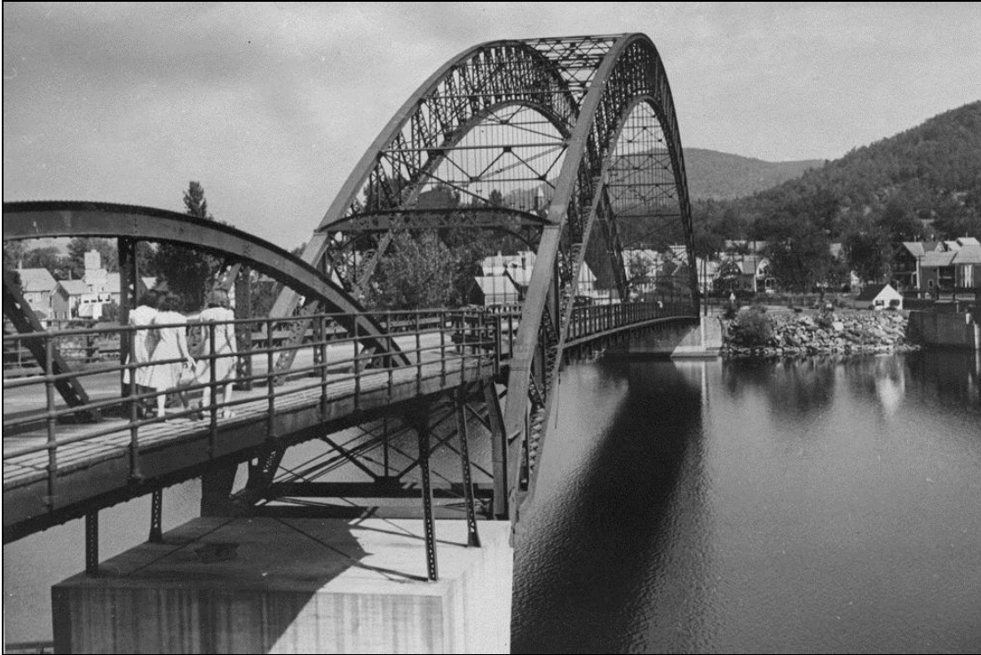
FIGURE 7: Arch Bridge, downstream side, from Vermont, c.1945, showing bowstring truss approach span (at left), replaced in 1961 with steel stringer span (Cheshire County Historical Society).
