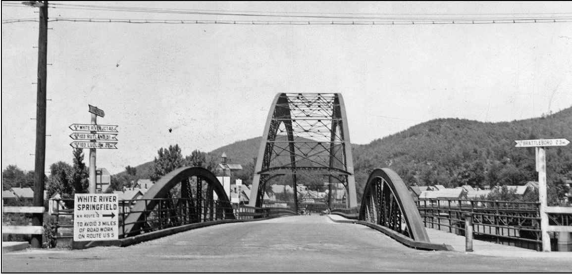
FIGURE 4: Arch Bridge, Bellows Falls end, showing bowstring truss span over the tracks of the former Rutland Railroad (NHDOT 1941).
