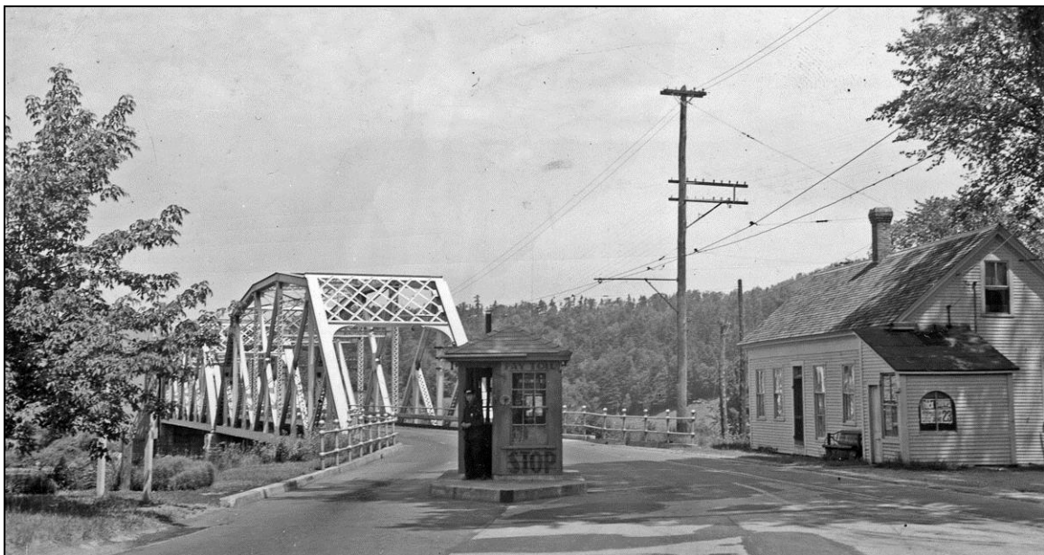
FIGURE 7: Cheshire Toll Bridge, built 1930 and presently in service. New Hampshire end shown in 1941. Compare to photos in Figures 5 and 6 and note widened approach, removal of store, alterations to toll house and new toll booth (NHDOT 1941).
