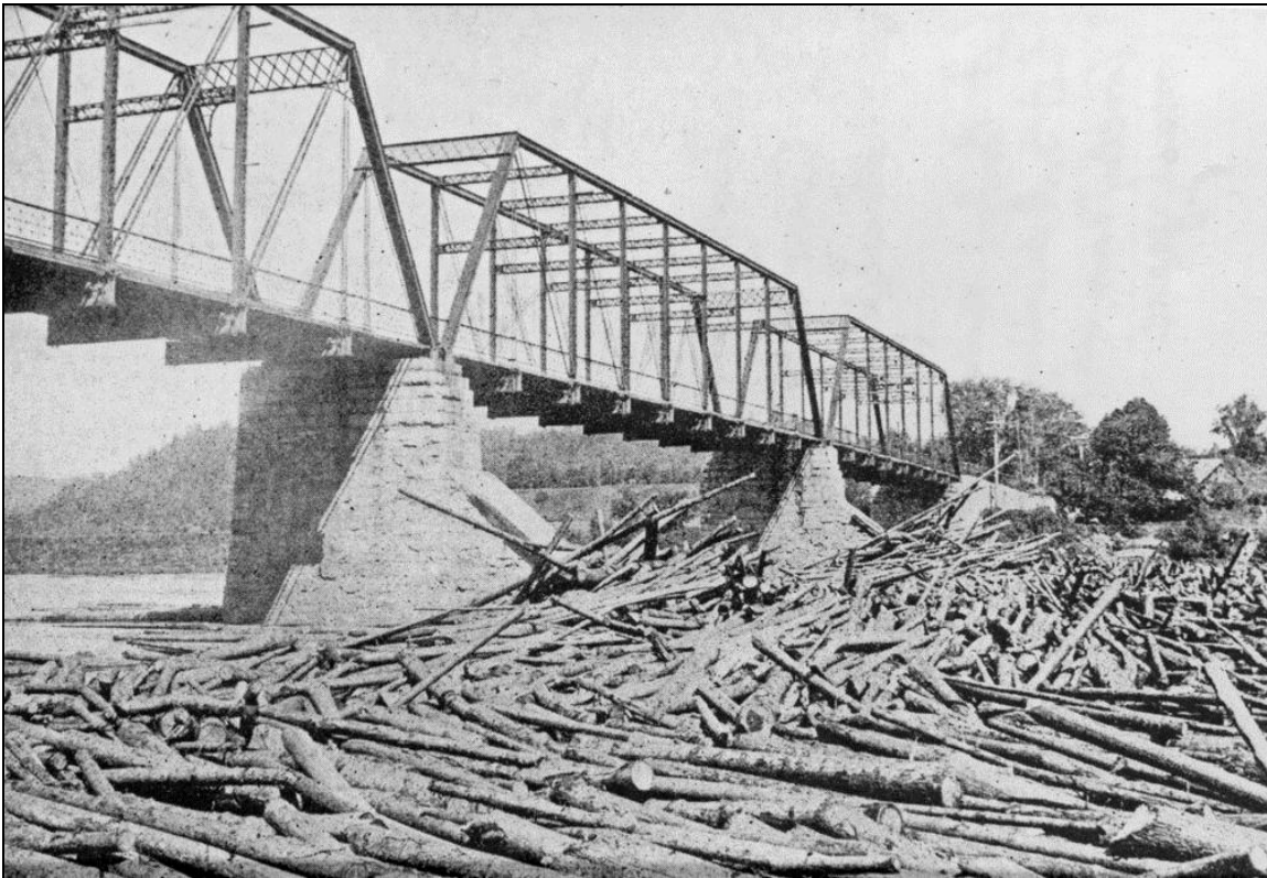
FIGURE 4: Cheshire Toll Bridge, log jam against piers of 1896 bridge. Photo credited to O. E. Noyes, a Springfield tailor, probably taken c.1900 (Charlestown Historical Society).
