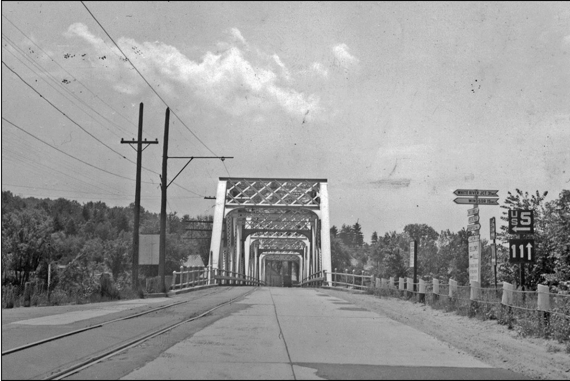
FIGURE 8: Cheshire Toll Bridge built 1930, and presently in service. Vermont end shown in 1941 (NH DOT 1941).
