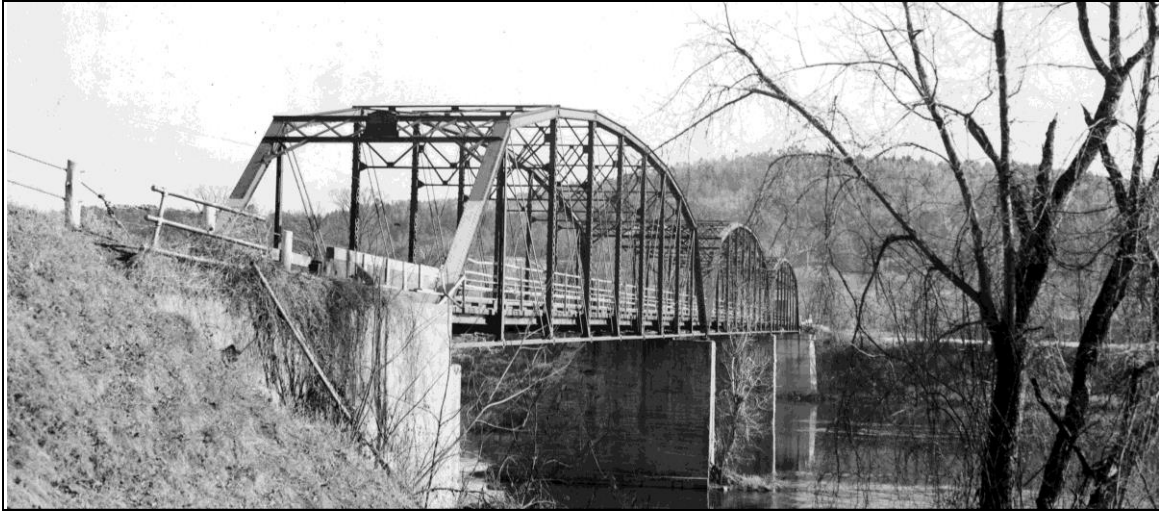
FIGURE 3: Ascutney Bridge, built 1908. Photo of downstream side in 1940. Parker Truss designed by Storrs & Storrs. Demolished 1969 (NHDOT 1940).
