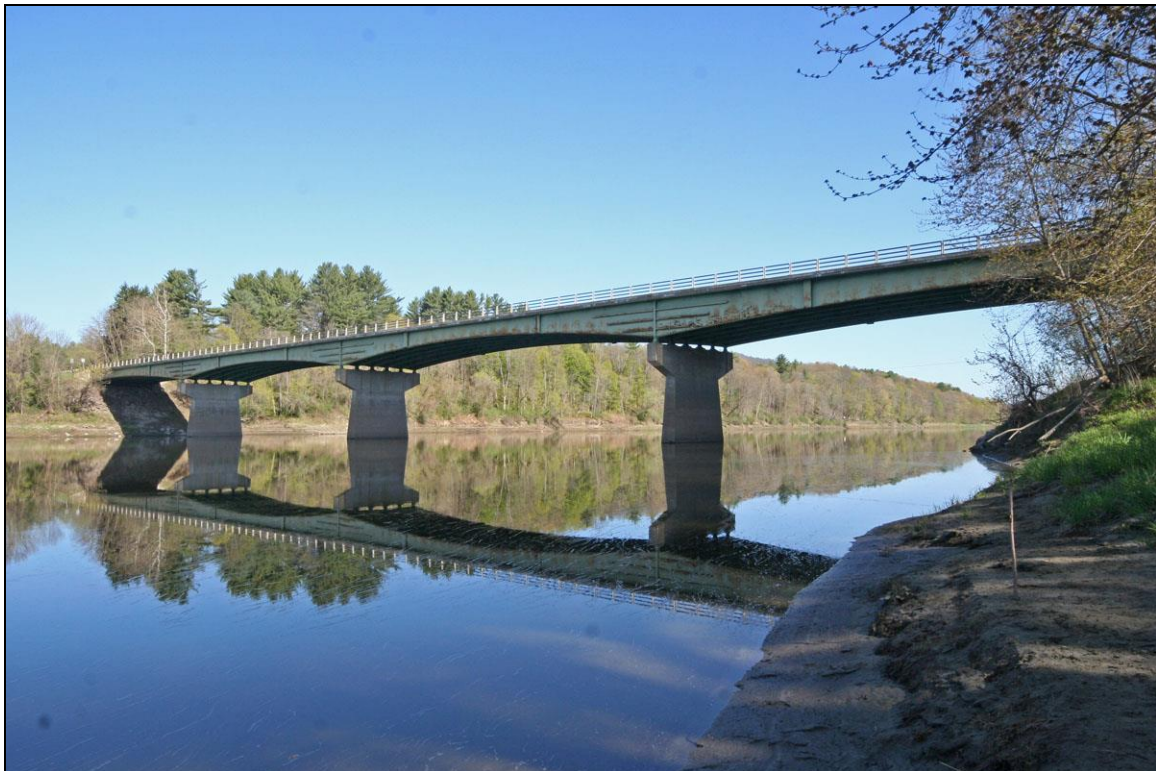
FIGURE 1: Present Ascutney Bridge, four span continuous welded plate girder built 1969 (Historic Documentation Company Inc. 2013).
