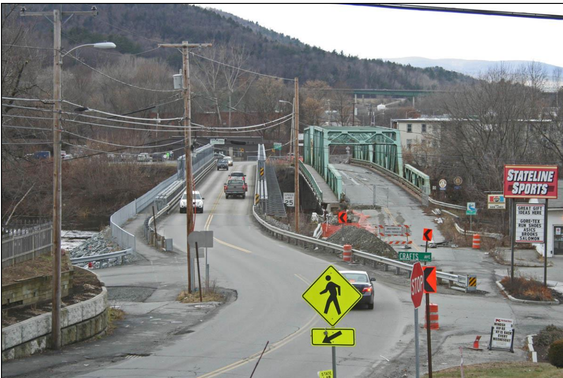
FIGURE 9: Lebanon-Hartford Bridge, 1936, shown closed with temporary bridge open on downstream side (Historic Documentation Company Inc. 2012).
