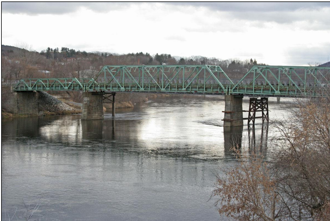
FIGURE 1: Lebanon-Hartford Bridge, built 1936. Upstream side. Note steel piers supporting temporary bridge on downstream side, erected to maintain traffic following closure of the bridge and during demolition and construction of new bridge 2013-2015 (Historic Documentation Company Inc. 2012).
