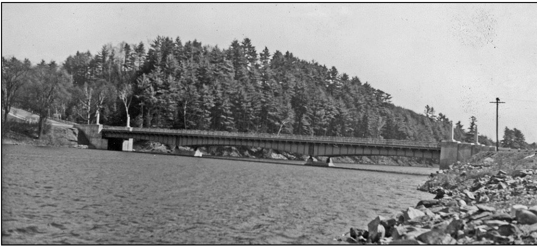
FIGURE 5: Ledyard Bridge, built 1935. Upstream side from Vermont in 1942 (NHDOT 1942).
