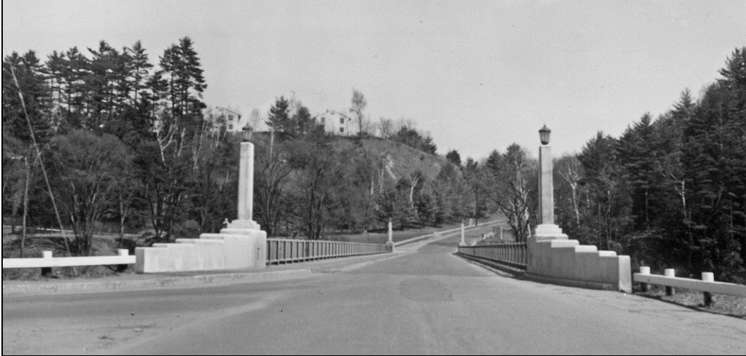
FIGURE 4: Ledyard Bridge, built 1935. Vermont approach in 1942 (NHDOT 1942).
