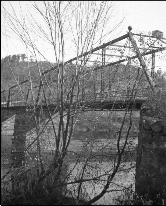
FIGURE 3: East Thetford Bridge, 3-span, pin-connected Pratt truss built 1896. View of upstream side from Vermont in 1922 (Storrs 1922).
