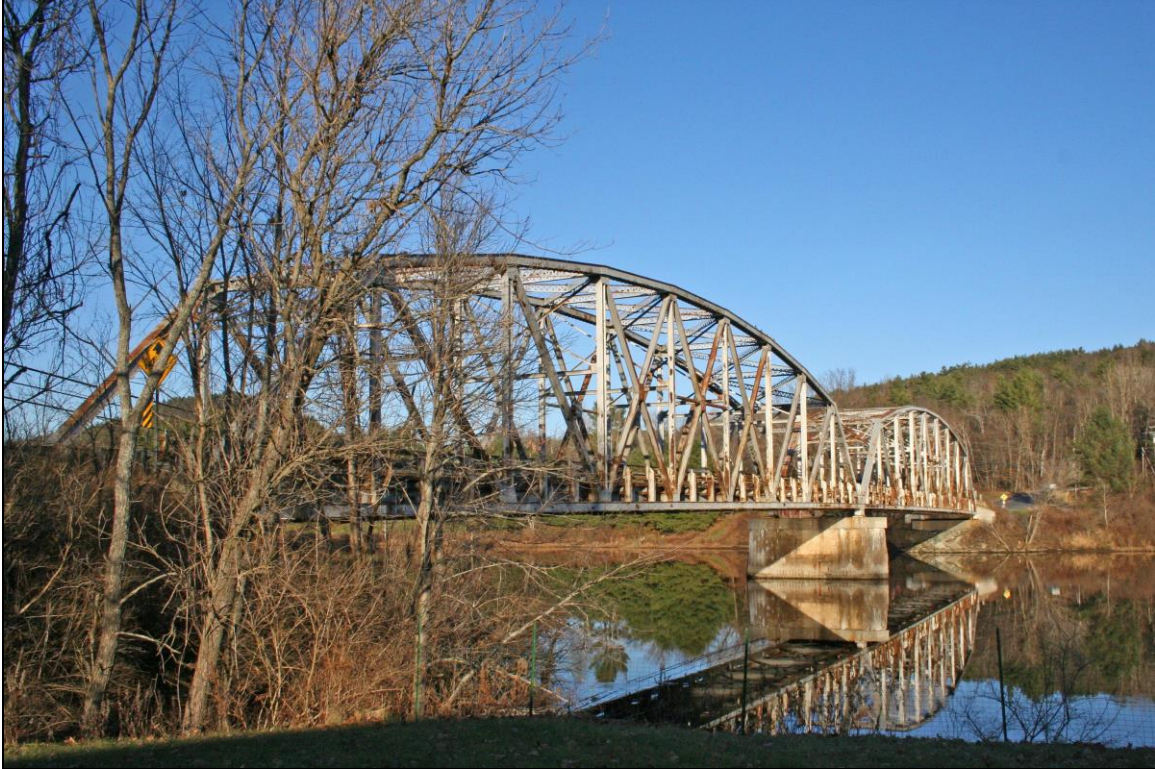
FIGURE 6: East Thetford Bridge, downstream side from Vermont (Historic Documentation Co., Inc. 2012).
