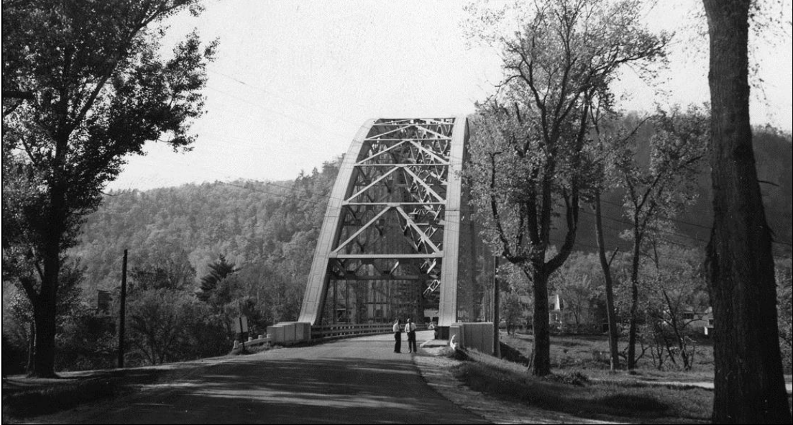
FIGURE 7: Orford-Fairlee Arch Bridge, New Hampshire approach, New Hampshire Highway Department inspection in 1941 (NHDOT 1941).
