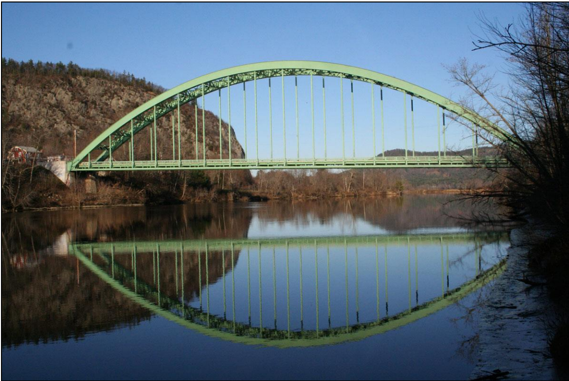
FIGURE 8: Orford-Fairlee Arch Bridge, downstream elevation (Historic Documentation Co. Inc. 2012).
