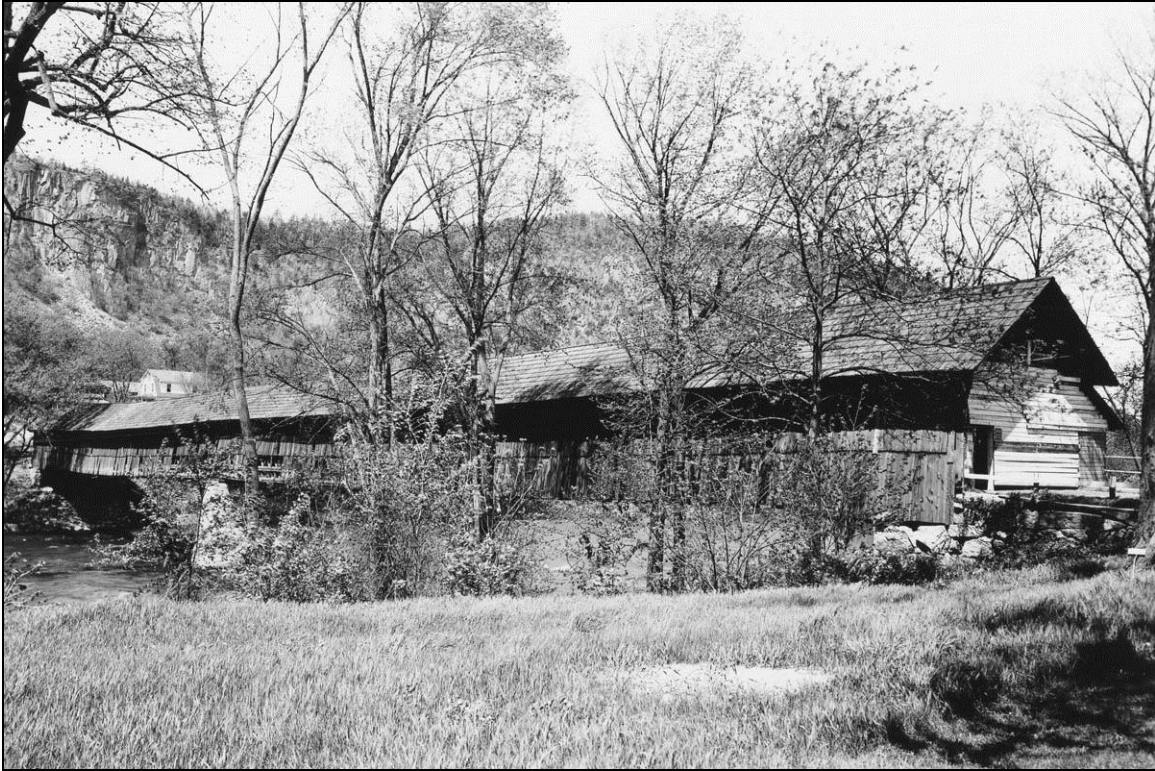
FIGURE 3: Orford Bridge, built 1856. Downstream side from Orford shore, May 14, 1936 (HABS 1936).
