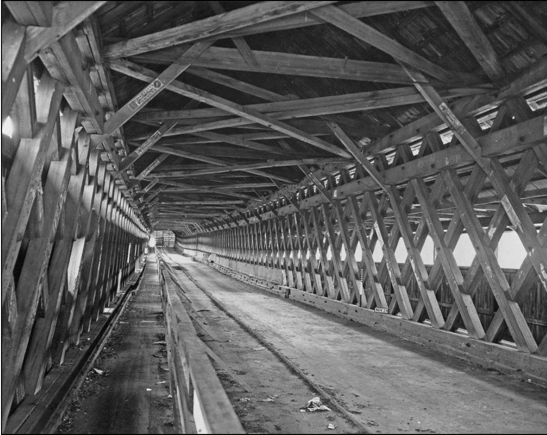
FIGURE 5: Orford Bridge, built 1856. Interior view toward Fairlee, May 14, 1936 (HABS 1936).
