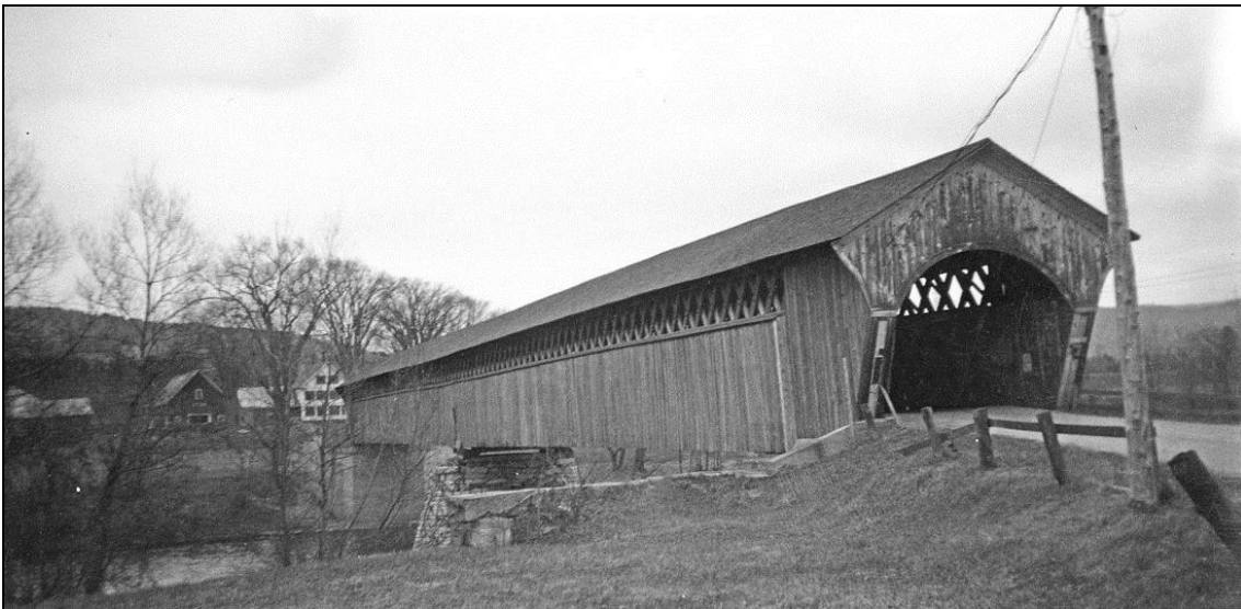
FIGURE 2: Covered bridge, Town lattice built 1850, reconstructed 1877 and destroyed by 1927 Flood. Vermont end shown in November 1922 (Storrs).
