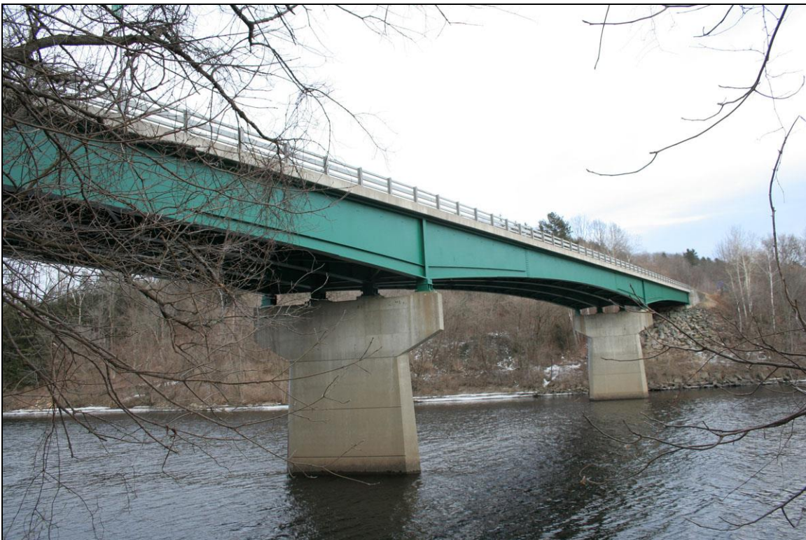
FIGURE 1: Newbury Bridge, built 1971 (Photo by Jerry Zoller, NHDOT).
