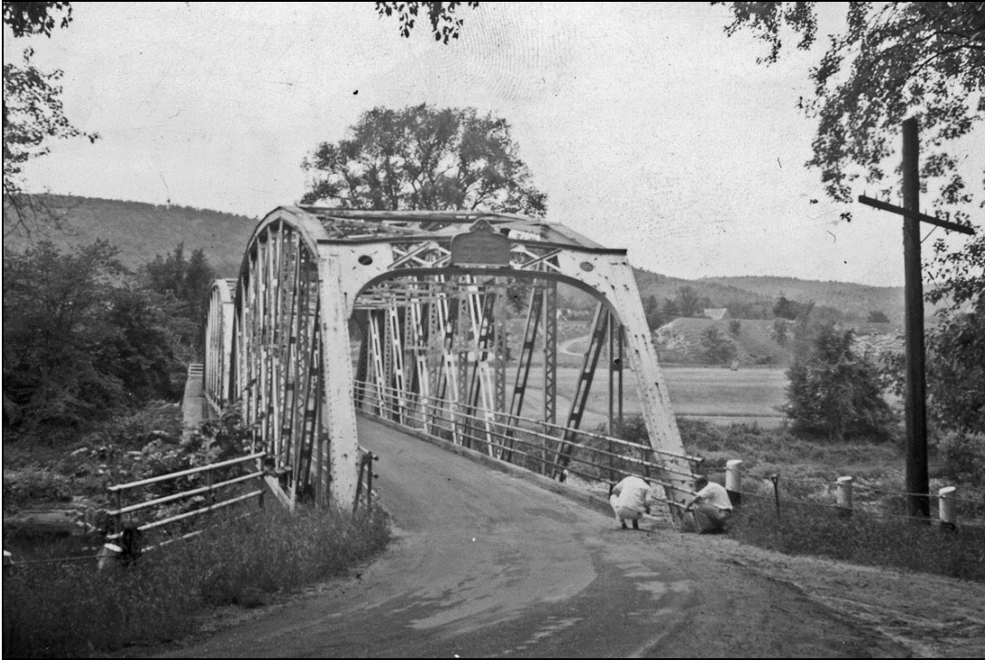
FIGURE 3: New Hampshire approach to 1913 truss bridge in 1942 (NHDOT 1942).
