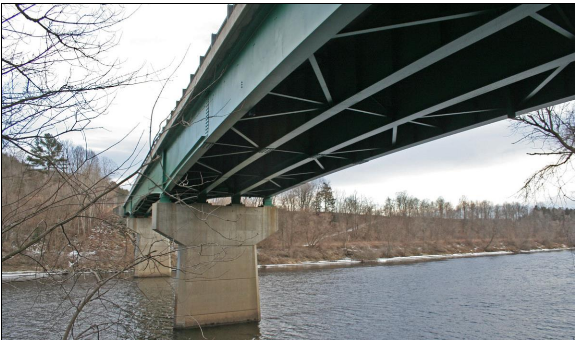
FIGURE 2: Newbury Bridge (1971) showing variable depth girders (Photo by Jerry Zoller, NHDOT).
