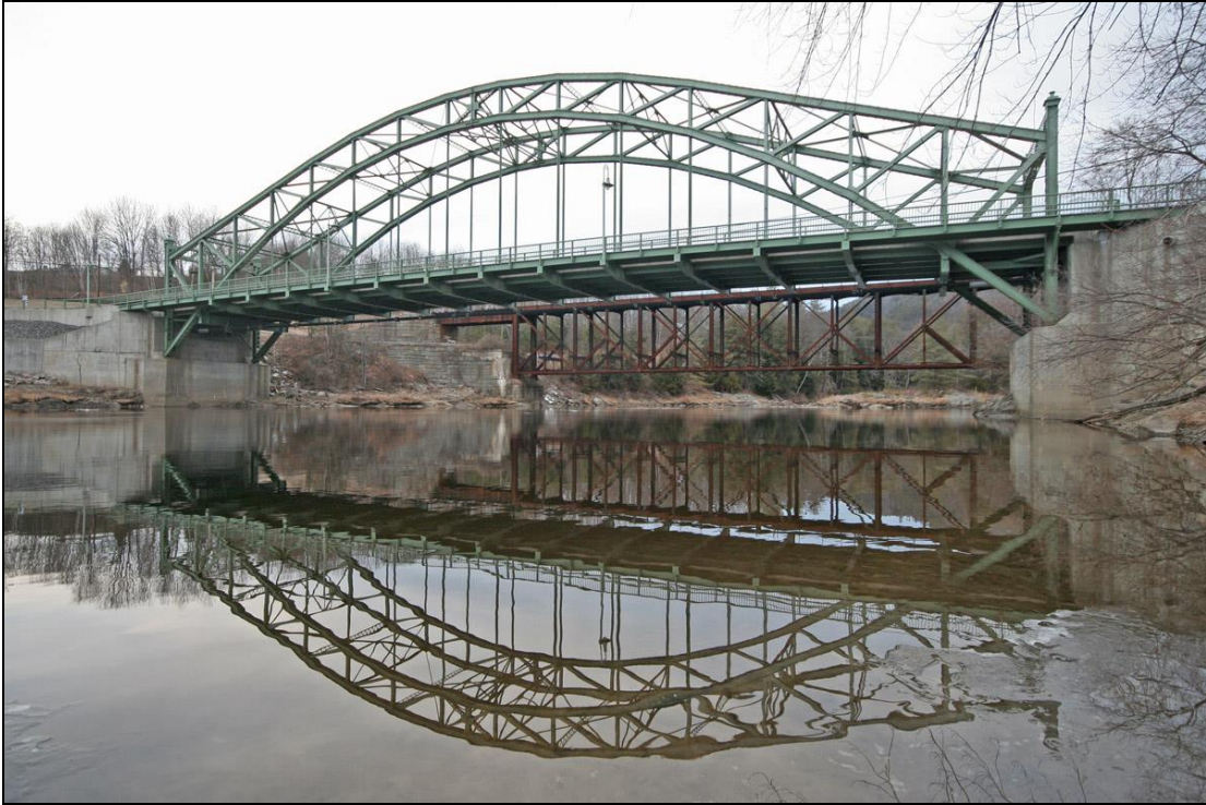
FIGURE 2: Woodville-Wells River Bridge, built 1923, showing Boston & Maine Railroad deck truss bridge in background (Historic Documentation Company, Inc. 2012).
