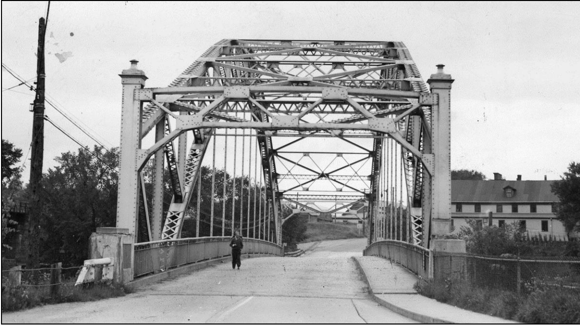
FIGURE 5: Woodville-Wells River Bridge, built 1923. Vermont end in 1940 (NHDOT 1940).
