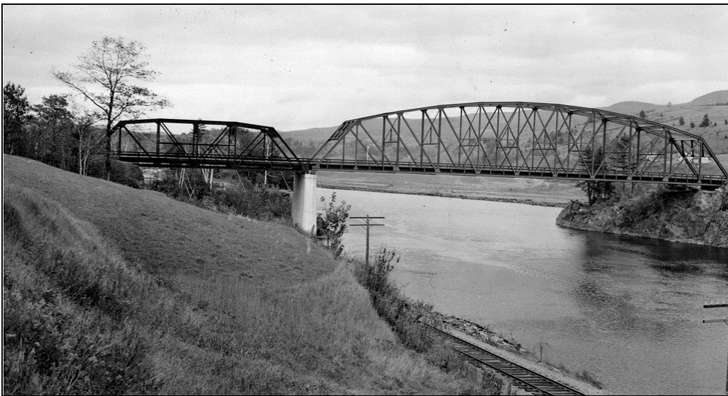
FIGURE 7: Barnet Road Bridge. Downstream side from Vermont in 1941 (NHDOT 1941).
