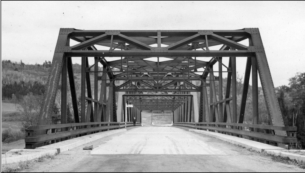
FIGURE 6: Barnet Road Bridge, built 1938. Vermont end in 1941 (NHDOT 1941).
