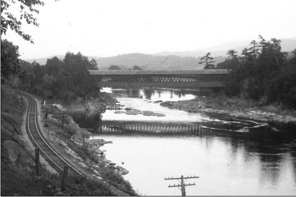
FIGURE 3: Stevens Village Bridge, built 1875, replaced 1937. Downstream side from Vermont, June 23, 1921 (Storrs).
