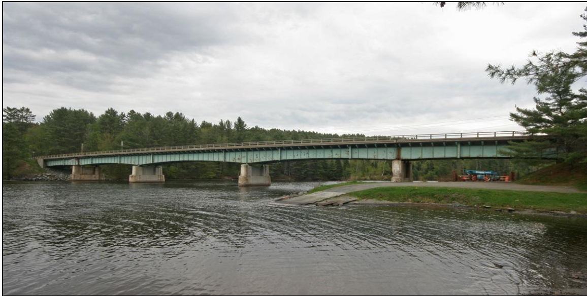
FIGURE 1: Route 18 Bridge, built 1934. Downstream side from New Hampshire (Historic Documentation Co. Inc. 2012)
