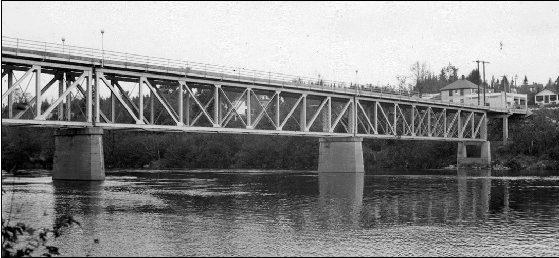
FIGURE 3: Whitcomb Bridge, built 1928. Upstream side, view to Vermont in 1941 (NHDOT 1941).
