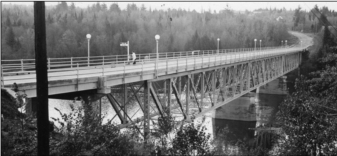
FIGURE 4: Whitcomb Bridge. Downstream side, view to New Hampshire in 1941 (NHDOT 1941).
