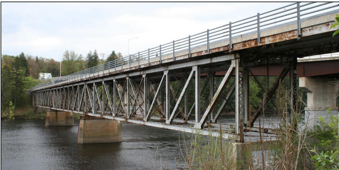
FIGURE 5: Whitcomb Bridge. Downstream side, view to Vermont (Historic Documentation Co. Inc. 2012).
