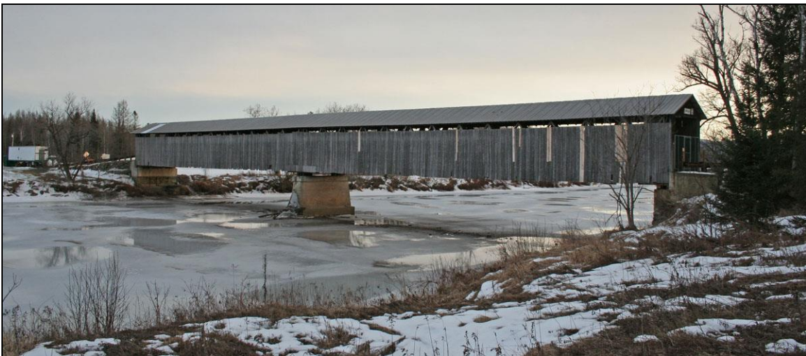
FIGURE 3: Mt. Orne Covered Bridge, built 1911. Upstream side, from Vermont (Historic Documentation Co. Inc. 2012).
