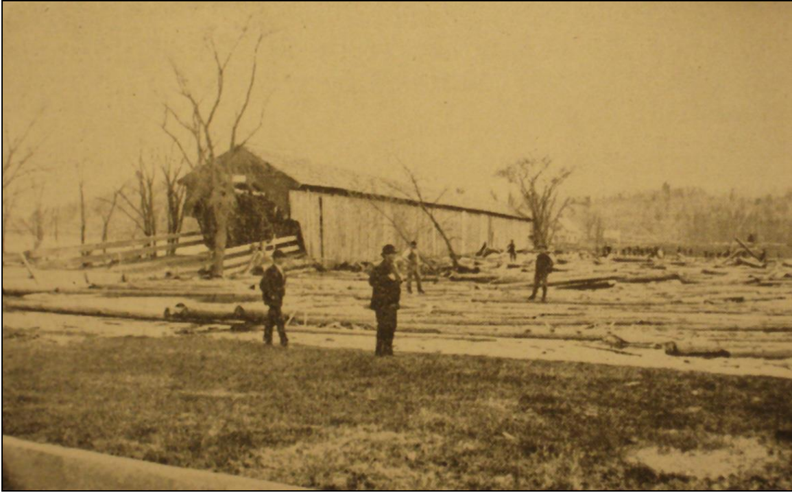
FIGURE 2: Covered bridge, built before 1844, replaced in 1901-1902 (photo circa 1890-1900). Caption reads "The combination of high water and log drives in the spring was hard on the Connecticut River bridges. Jams like this one damaged this bridge so badly in the 1890's that it was replaced in 1901 by another" (Lancaster Historical Society).
