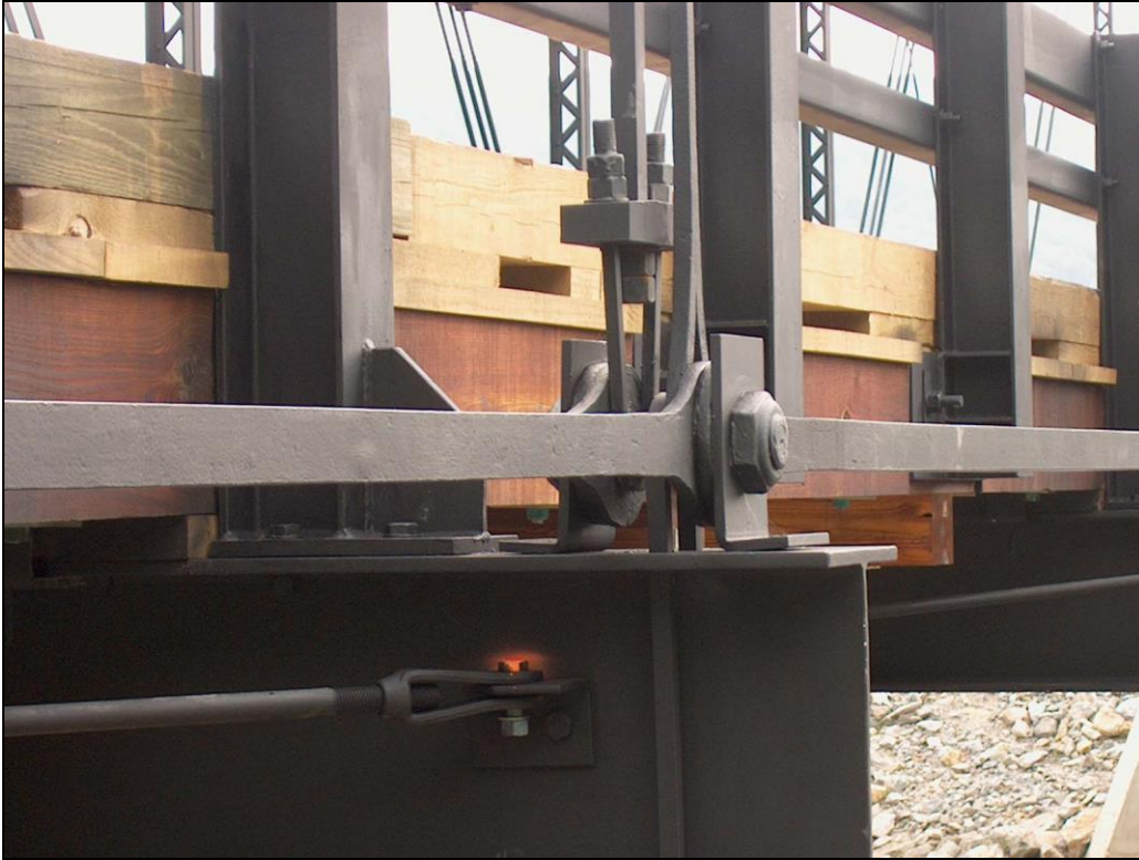
FIGURE 5: Floor beam, post and lower chord reconstruction, 2005 (Historic Documentation Co. Inc. 2012).
