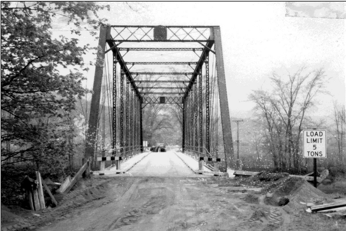
FIGURE 2: Stratford Hollow Bridge during repairs in 1958 (NHDOT 1948).
