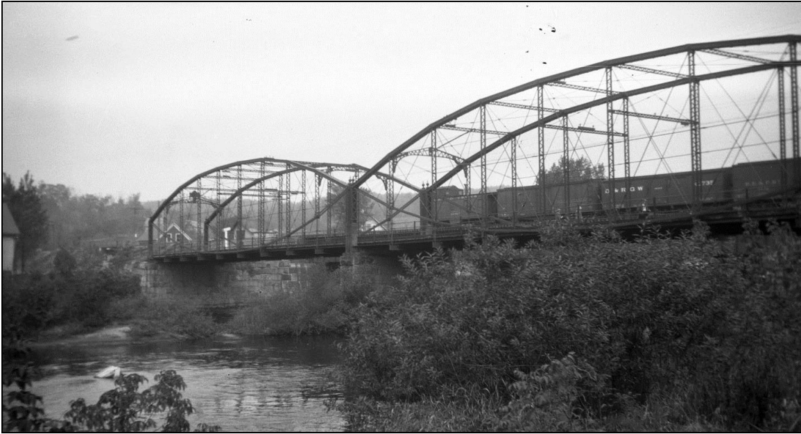
FIGURE 2: North Stratford Lenticular Truss Bridge, built 1893. Photo dated October 3, 1922, showing upstream side from Vermont shore (Storrs).
