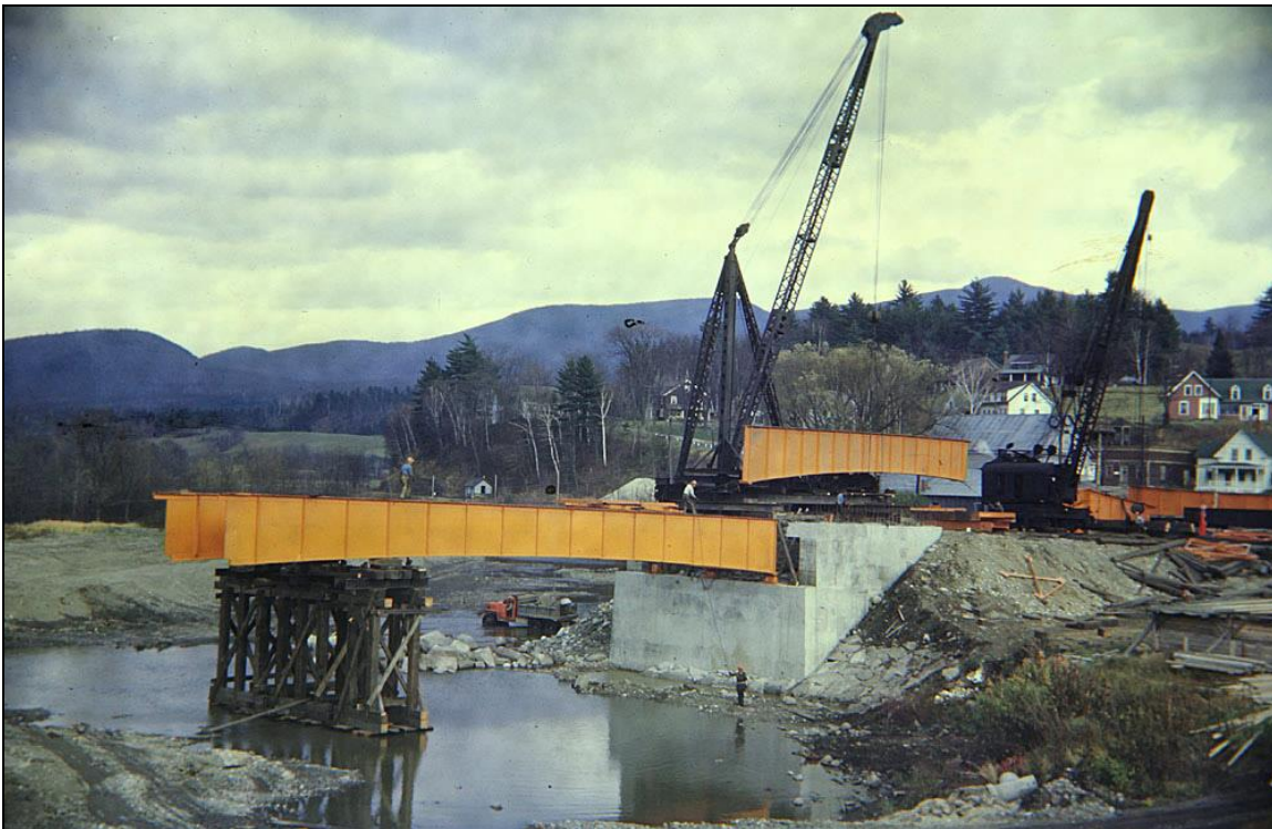
FIGURE 5: North Stratford-Bloomfield Bridge, showing construction of continuous steel girders in 1947 (NHDOT 1948).
