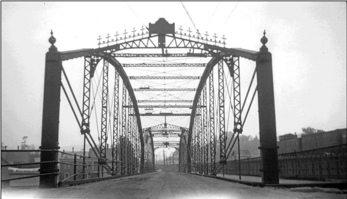
FIGURE 3: North Stratford Lenticular Truss Bridge, built 1893. Photo dated October 3, 1922, Vermont end, looking to New Hampshire (Storrs).
