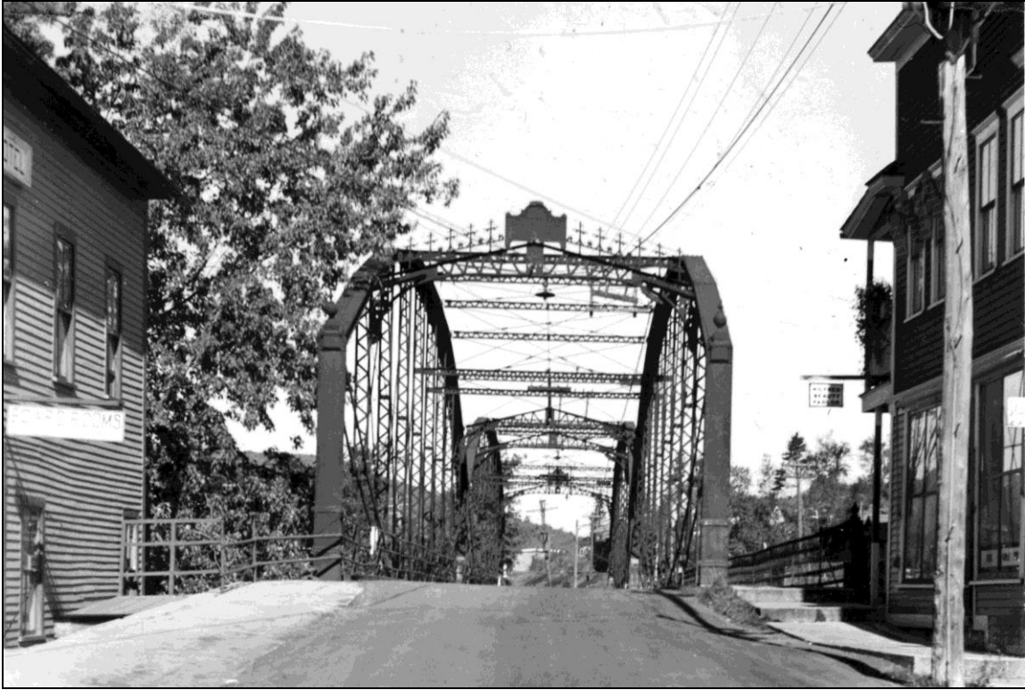
FIGURE 4: North Stratford Lenticular Truss Bridge, built 1893. Photo dated September 13, 1941, showing New Hampshire end, looking to Vermont (NHDOT 1941).
