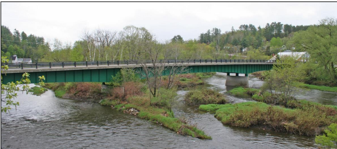
FIGURE 1: North Stratford – Bloomfield Bridge, built 1947. Downstream side from Vermont shore (Historic Documentation Company Inc. 2012).
