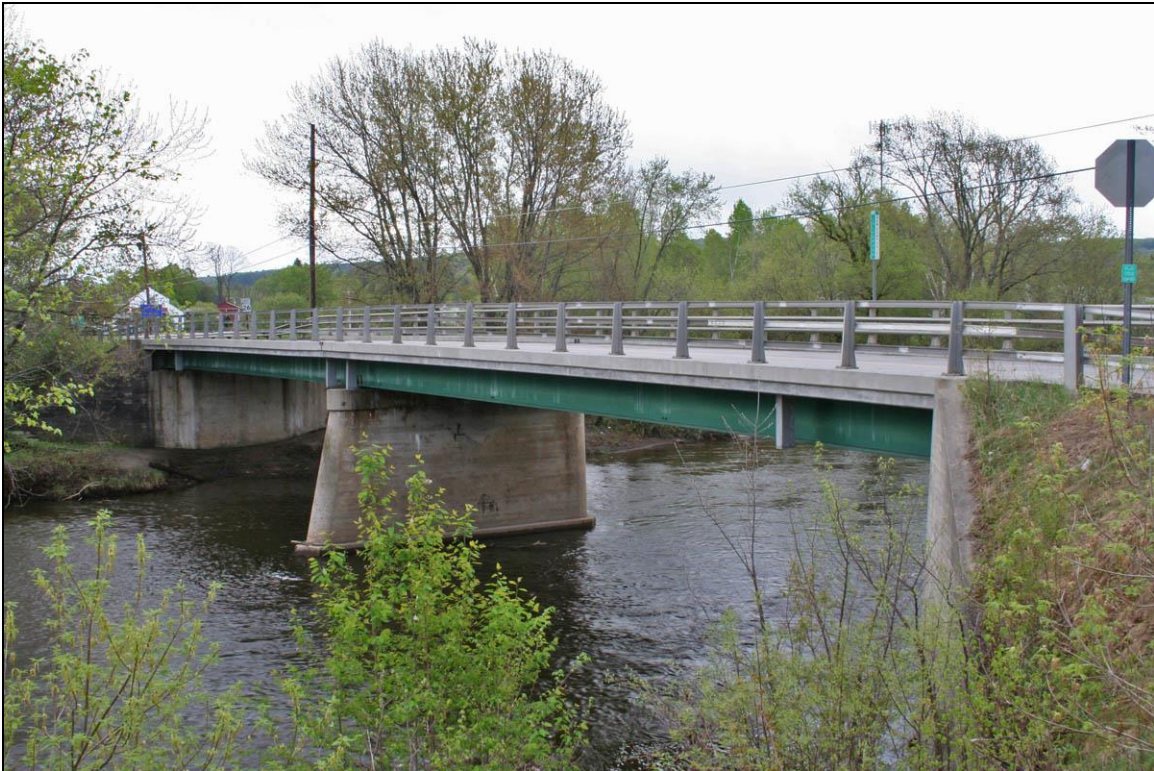
FIGURE 1: Colebrook – Lemington Bridge, upstream side from Vermont (Historic Documentation Co. Inc. 2013).
