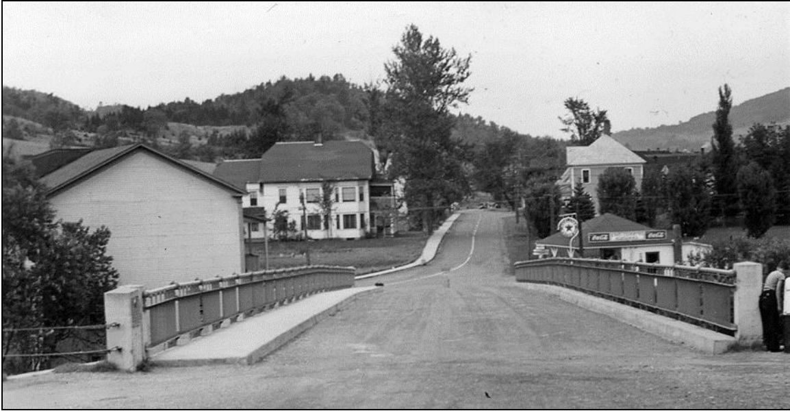
FIGURE 4: Beechers Falls Bridge, built 1930. New Hampshire approach shown September 9, 1941 (NHDOT 1941).
