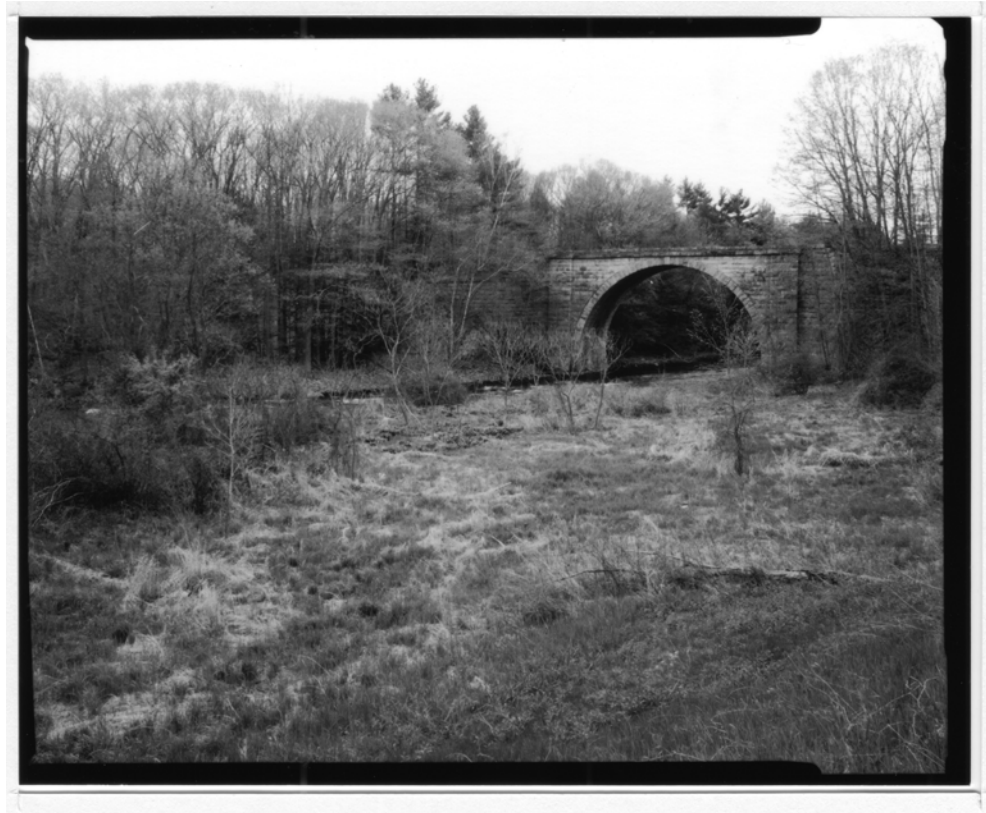
NH-630-2 View of bridge in context with floodplain. Looking southwest.
