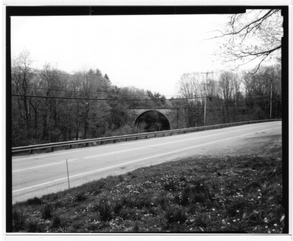
NH-630-1 View of bridge in context with Route 101. Looking southwest.
