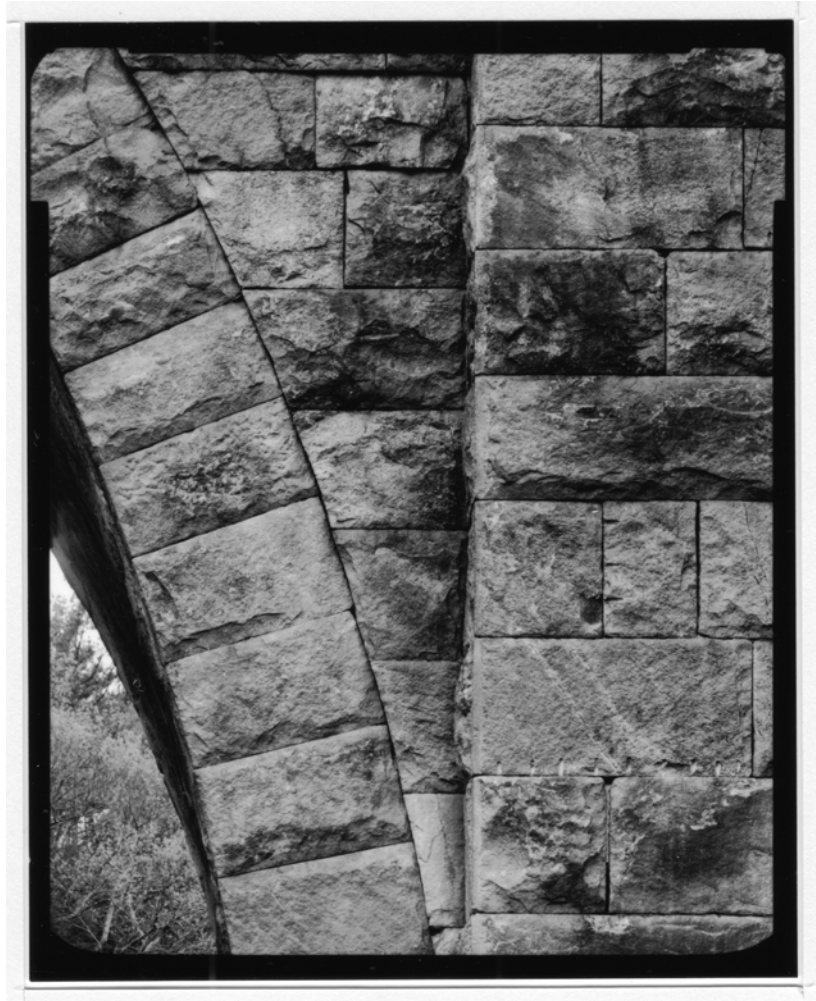
NH-630-13 Detail of arch and buttress stonework. Looking southwest.
