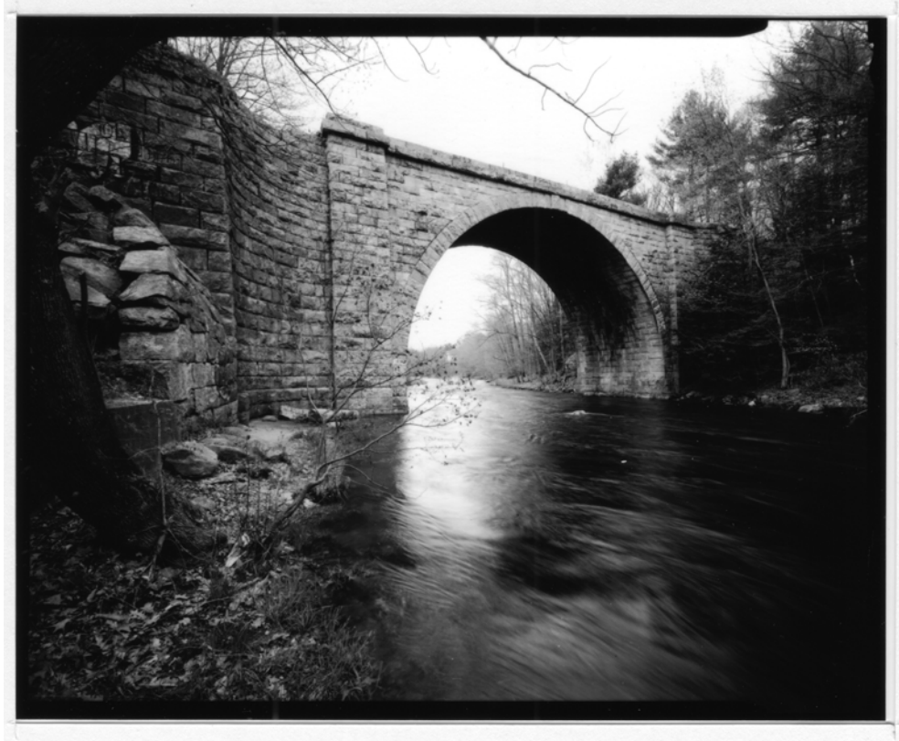
NH-630-5 Downstream elevation, south half. Looking east.
