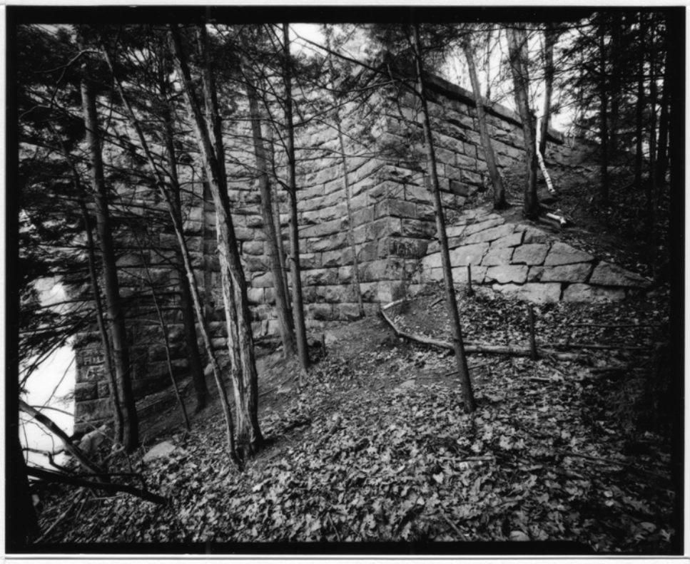
NH-630-8 Southwest wingwall. Looking east.
