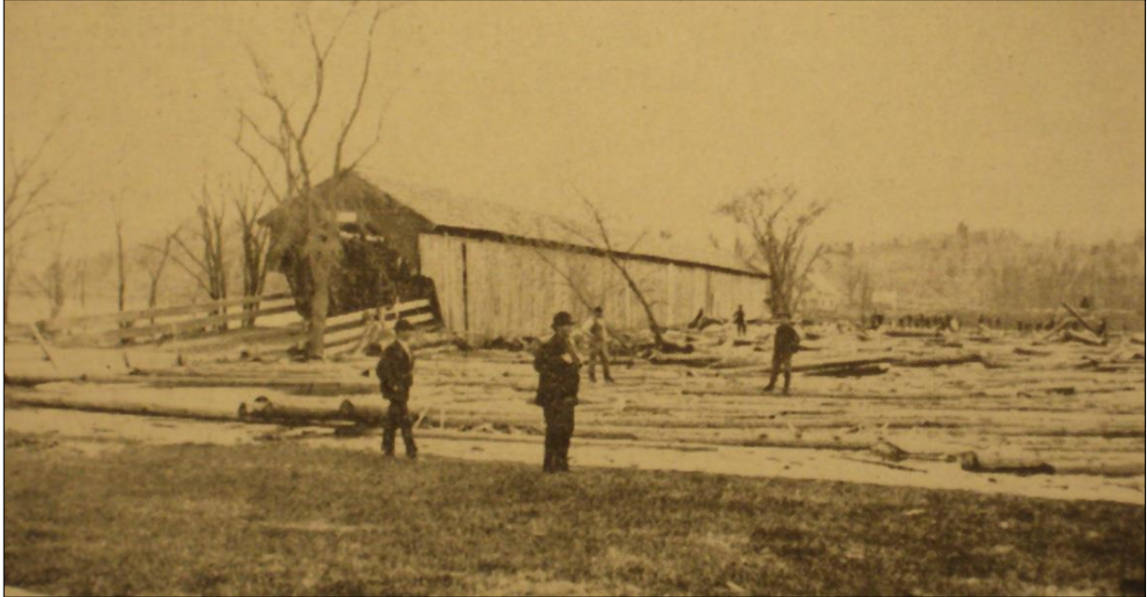
FIGURE 2: Covered bridge, built before 1844, replaced in 1901-1902 (photo circa 1890-1900). Caption reads "The combination of high water and log drives in the spring was hard on the Connecticut River bridges. Jams like this one damaged this bridge so badly in the 1890s that it was replaced in 1901 by another." Source: Lancaster Bicentennial Committee, 1964.
