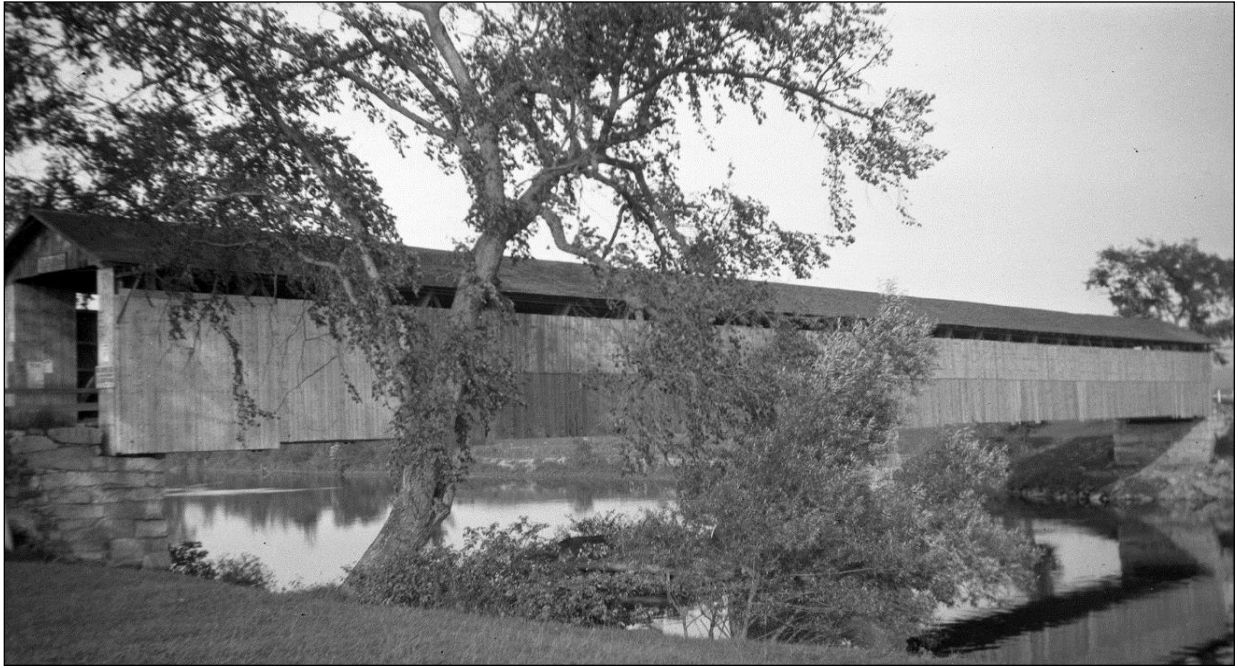
FIGURE 3: Photograph dated October 2, 1922, of covered bridge, built 1901-1902, demolished and replaced in 1950 with Rogers Rangers Bridge. Source: Storrs Photograph Collection, New Hampshire Division of Historical Resources.
