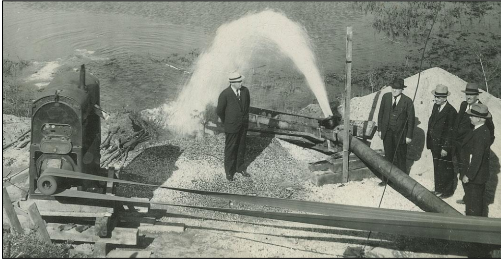
FIGURE 22: Testing Smith Well, August 15, 1940 (close up of Figure 21). The men inspecting the well are believed to include Mayor Samuel Blair, well-driller David Smith and some members of the Board of Water Commissioners. In 1940 the Board members were Samuel B. Blair, Philip C. Brown, John D. Grady, Cesaire Houde, and Frederick C. Smalley.
