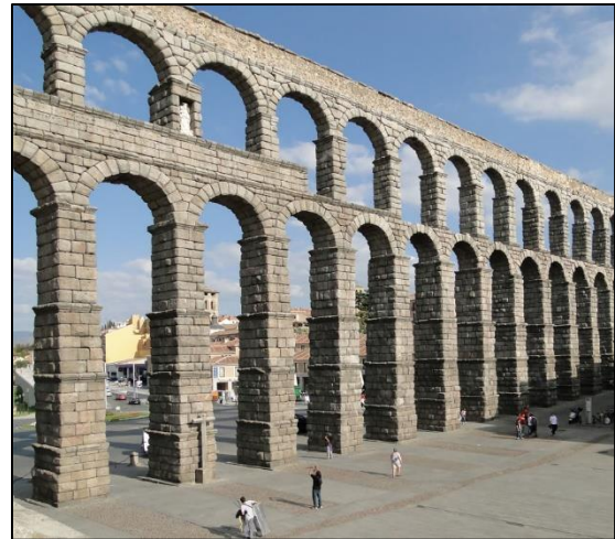
FIGURE 1: Roman aqueduct, Segovia, Spain, 11 miles long overall, 94 feet high through the city, resting on foundations 20 feet deep (Aqueduct of Segovia).
