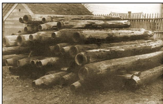
FIGURE 3: Logs were bored out with a long drill bit and then tapered externally and internally at opposite ends to jam tightly together end-to-end. Iron ties or clamps often secured the joints. These redwood pipes in the photo above were unearthed from the early system installed at Fort Bragg, North Carolina in the 19 th century. In New Hampshire similar log pipes but of white pine, elm or hemlock were typically used (Mendocino Coast).
