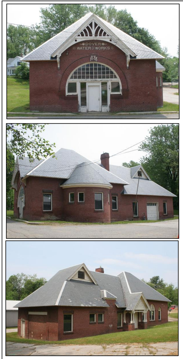
FIGURE 10: Dover Water Works Pumping Station, in 2011. From top down: north side with main entrance set in arched opening; west side with round bay with conical roof; south side with entrance portico on paired columns (Historic Documentation Company, Inc.).
