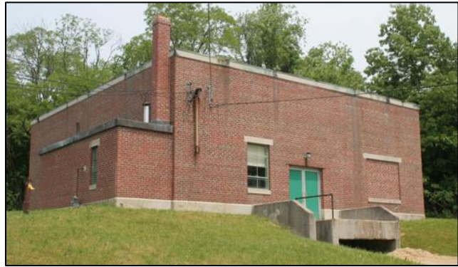
FIGURE 26: Water Treatment Plant building built in 1955 at Lowell Avenue water works facility (Historic Documentation Co., 2011).
