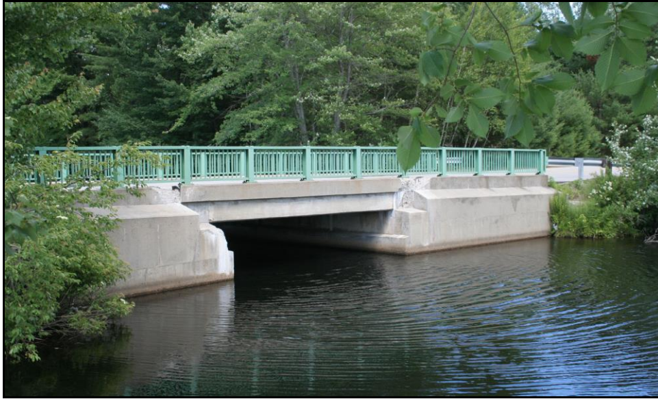
Figure 4.2: New Durham 199/054 [1926]. New steel balustrade-type bridge railing. Survey photo, 2010, south elevation.
