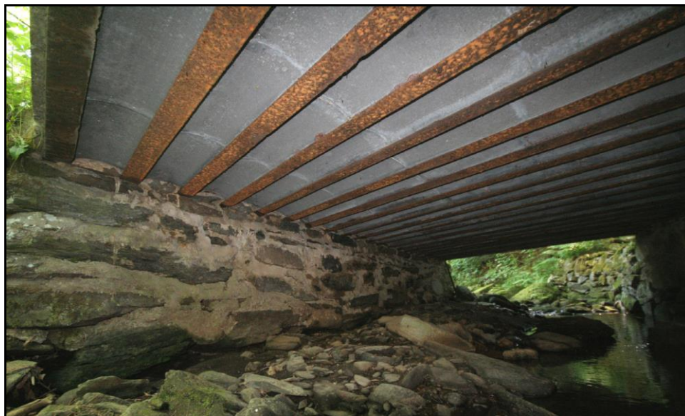
Figure 3.17: Charlestown 142/101. Non-corrugated galvanized forms. Survey Photo July 2010.
