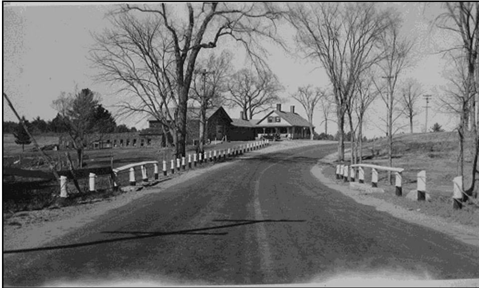
Figure 4.5: Chichester 130/100 [1931]. Photo from Bridge Card, 1941. Compare setting to today in photo below. Note steel cable guardrail.
