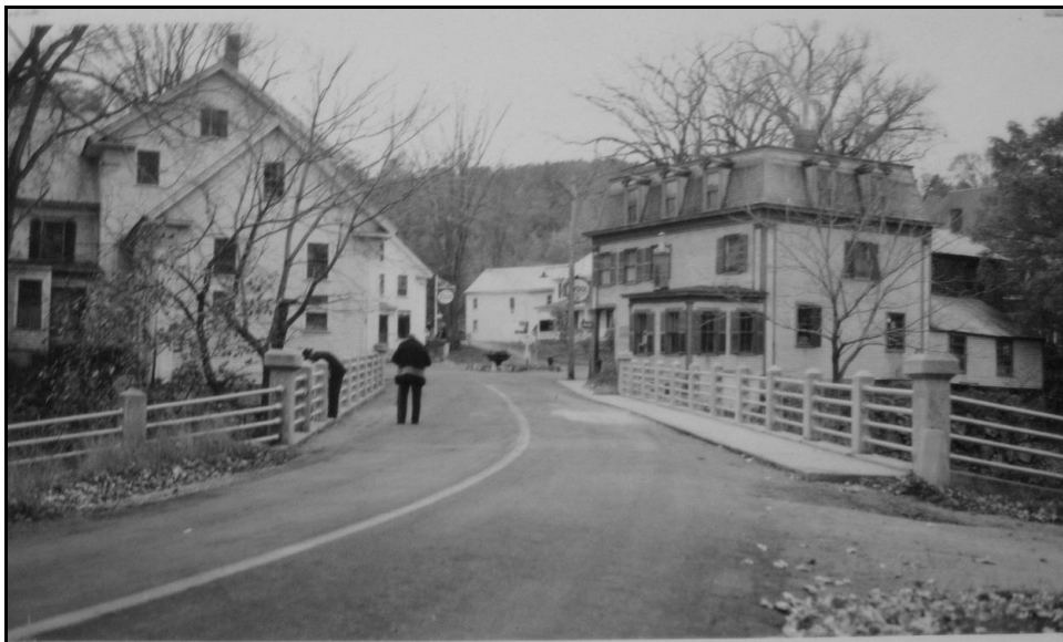
Figure 3.29: Freedom Bridge 185/067 [1922]. Steel pipe railing on concrete posts. Photo from Bridge Card, 1940. NHHD bridge inspectors shown at work.
