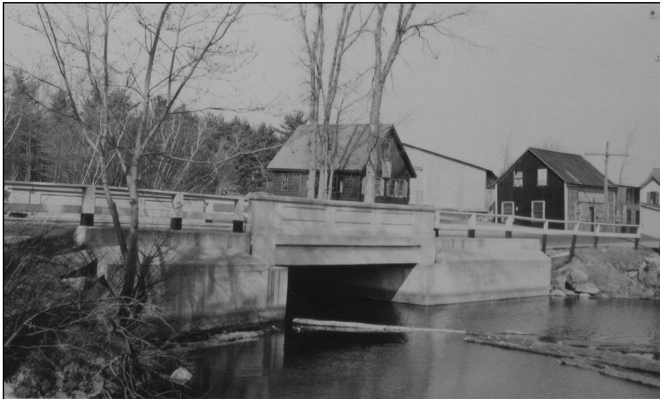
Figure 4.1: New Durham 199/054 [1926]. Original bridge railing. Photo from bridge card, 1941, south elevation.
