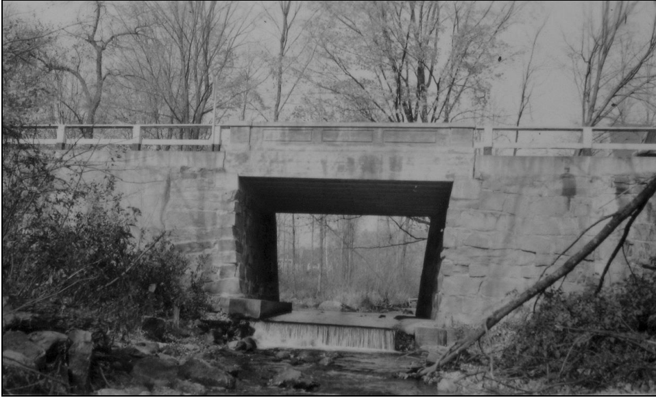
Figure 3.12: Tamworth 095/162 [1925]. Photo from bridge card, 1941
