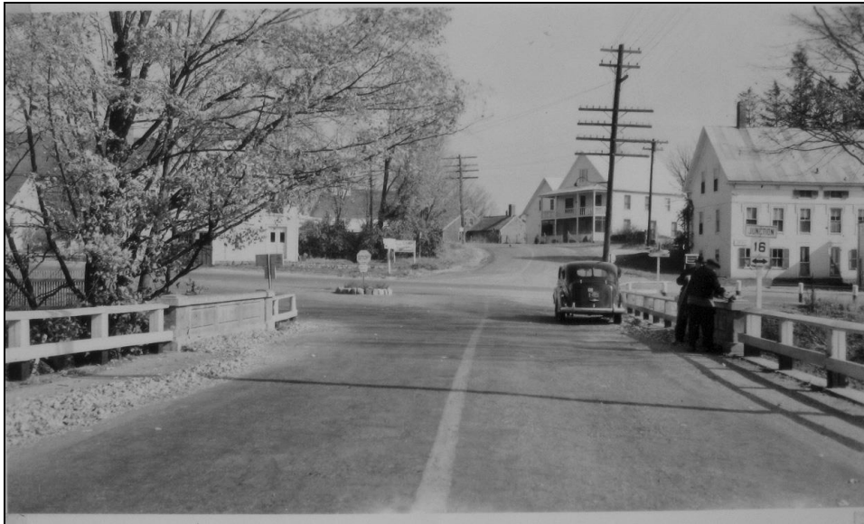
Figure 3.11: Tamworth 095/162 [1925]. Photo from bridge card, 1941
