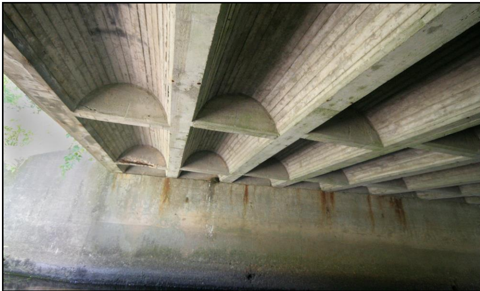
Figure 3.23: Goffstown 053/119 [1923]. Designed by Harold Langley. Survey Photo July 2010.
