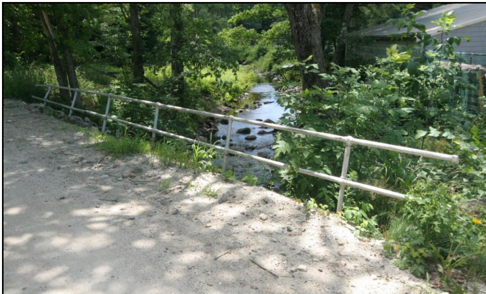
Figure 3.28: Peterborough 132/134 [1940?]. Surviving two-rail pipe railing. Survey Photo July 2010.
