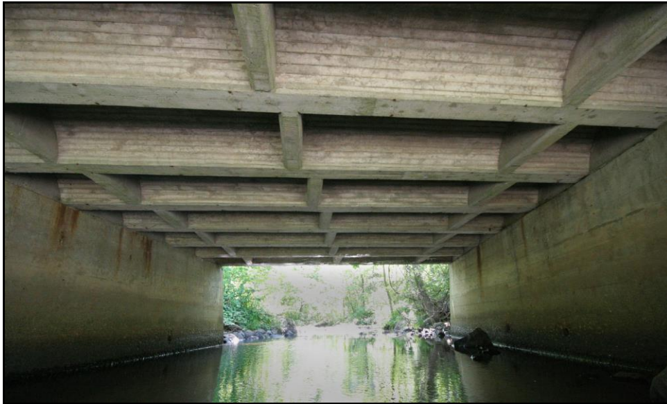
Figure 3.22: Goffstown 053/119 [1923]. Designed by Harold Langley. Survey Photo July 2010.
