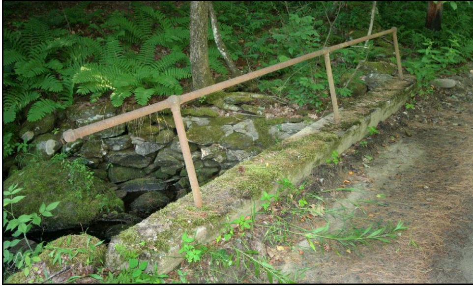
Figure 3.27:Charlestown 142/101 [1940]. Surviving one-rail pipe railing. Photo July 2010.
