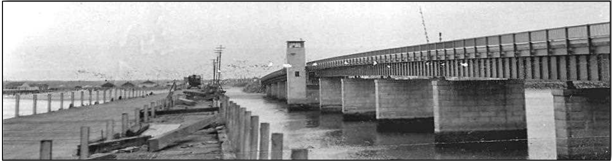
Underwood Bridge completed, 1950, with Mile Long Bridge awaiting demolition. Photo courtesy of Lane Memorial Library.
