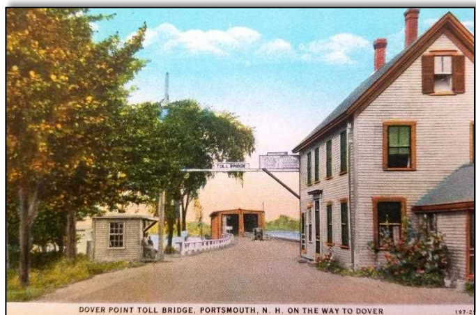
South end of bridge, showing the separated lanes of the covered truss span, with the railroad on the east side and highway on the west side (Dover Public Library).
