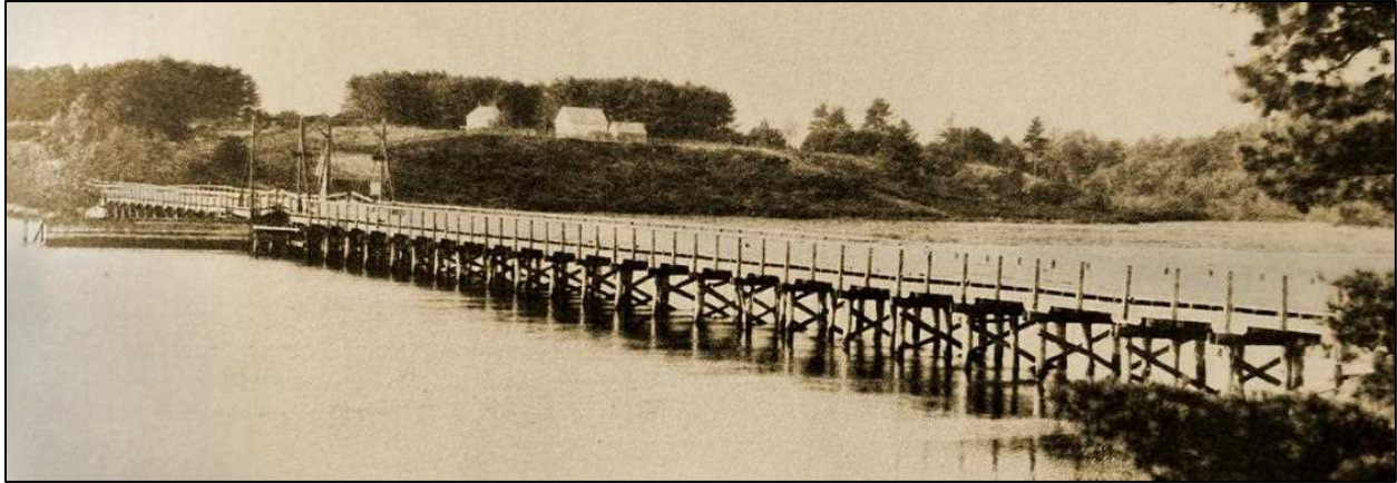
Eliot Bridge about 1898, looking toward the Dover shore, showing double-leaf bascule draw span. Courtesy Dover Public Library.
