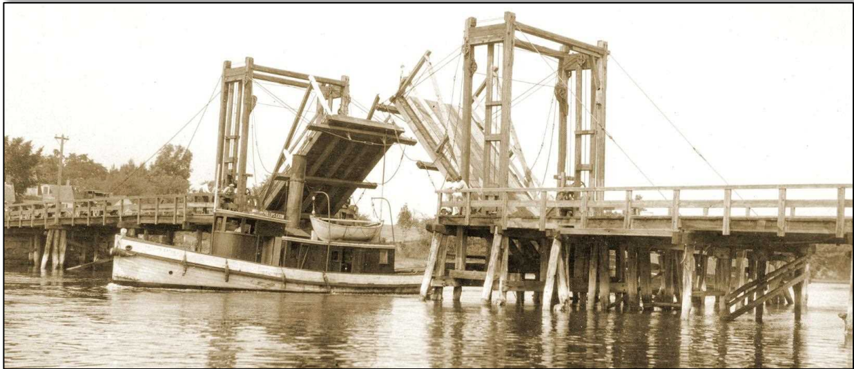
Stratham Bridge over Squamscott River, photo ca. 1920, showing the double-leaf, cable-lift bascule draw span built 1884. Courtesy Stratham Historical Society.
