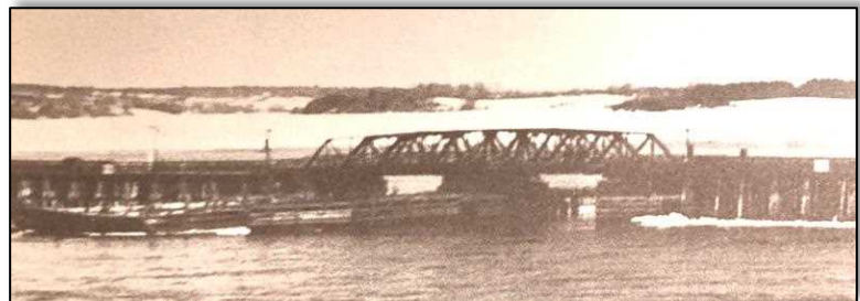
Dover Point Bridge, photo c. 1934, showing steel swing span installed 1915. Courtesy Dover Public Library.
