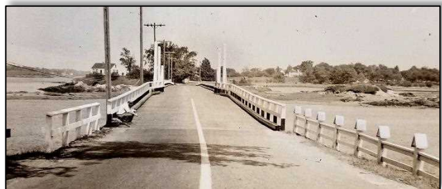
Below: West approach to middle trestle of the bridge taken July 3, 1940 by NHHD bridge inspector Wendell H. Piper.
