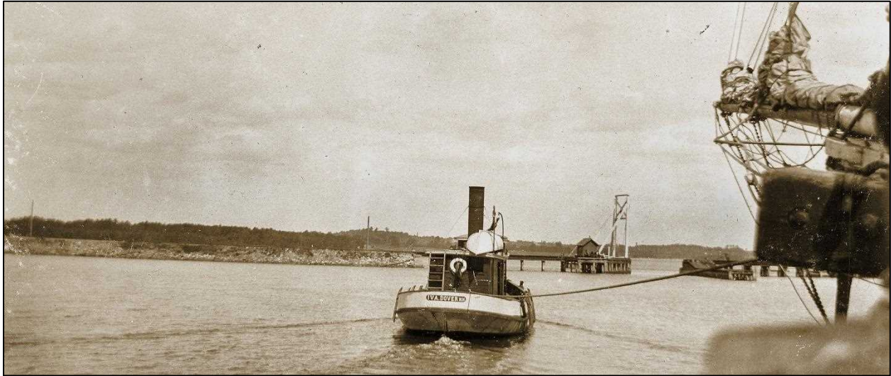
View of bridge ca. 1920, from schooner Ada J. Campbell being towed down the Squamscott River to Great Bay by tug Ida of Dover. The draw span, known as a shear pole or shear leg swing, has been swung open on the bay side, suspended by cables from the upright frame tower (Stratham Historical Society).
