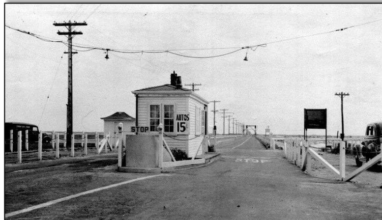
Toll booth at Seabrook end of bridge. The overhead timber frame supporting the lifting cables for the bascule draw span is visible in the distance. No plans or photos of the draw were located. This photo and one below taken July 1, 1940 by NHHD during inventory of the state's bridge conducted just prior to World War II (Bridge inventory card, Hampton 300/043).
