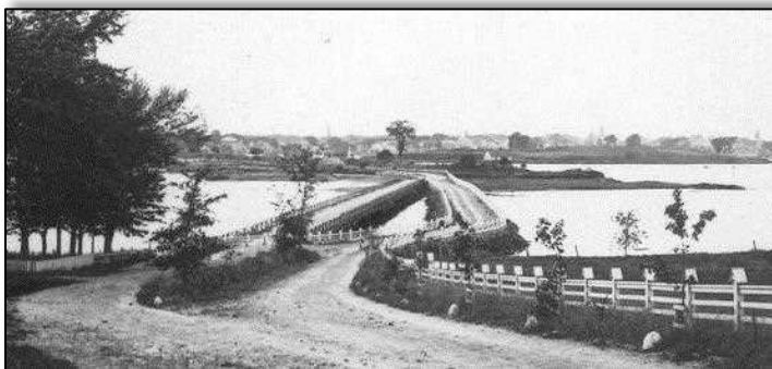
During World War II the old military forts on New Castle Island were reactivated to defend Portsmouth Harbor. Heavy trucks loaded with building materials and military supplies greatly exceeded the capacity of the wood trestle bridges to the island. The trestle between Goat Island and New Castle was bypassed with a gravel-filled causeway seen completed at left. Photo courtesy of NH Port Authority.
