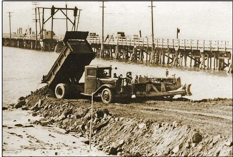
Construction of gravel filled approach causeways for the Underwood Bridge on the seaward side of the Mile Long Bridge, visible in background, in the fall of 1947 (Courtesy Lane Memorial Library).
