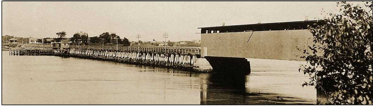
Portsmouth & Dover Railroad's "Dover Point Bridge" over Great Bay, a wood pile trestle 1600' long with a 180' covered "steel truss" span on granite piers for small boats and ice to pass and a swing span for fixed-mast vessels. Courtesy Dover Public Library.
