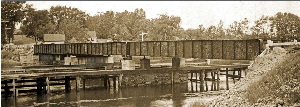
Newfields-Stratham Swing Bridge over Squamscott River. Photo 1941, New Hampshire Highway Department.
