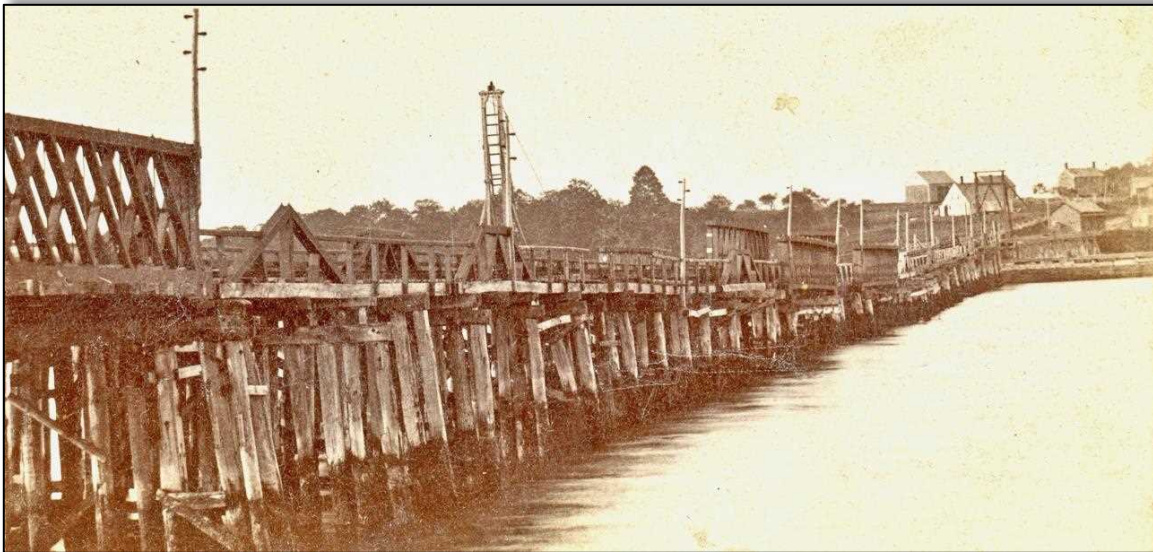
Portsmouth Bridge was a wood pile trestle highway bridge that stretched 1600 feet across the Piscataqua from Portsmouth to Kittery. Extreme currents, tidal range and depth of water made the bridge a monumental undertaking few thought feasible. This photo, ca. 1885, courtesy of Portsmouth Athenaeum, shows the downstream side of the Eastern Railroad trestle, built 1842, immediately alongside the Portsmouth Bridge.
