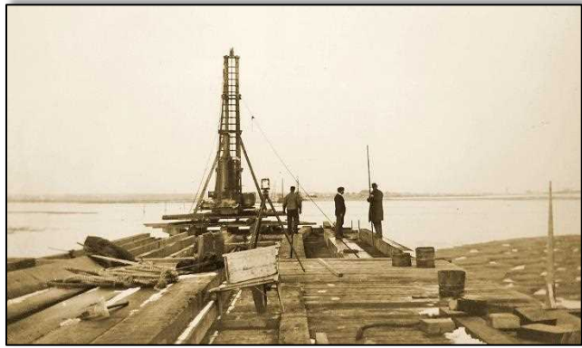
Cowles & Childs Construction Co. driving piles for the bridge in 1901. The 4,923-foot structure stood on 5,270 oak piles. It was completed in one year by three steam pile drivers. A 30-foot bascule draw spanned the river channel near the middle of the bridge. Photo courtesy of Lane Memorial Library.
