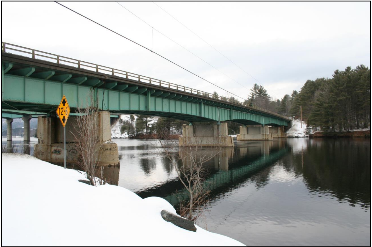
Littleton Bridge 109/134 carrying NH 18 over the Connecticut River, built 1934
