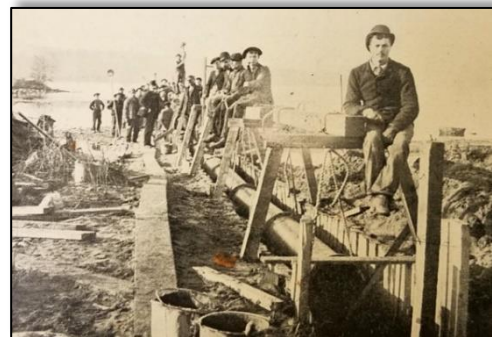
Laying Laconia's 15" main outlet pipe discharging into the Winnepesaukee River at Dixon's Point in 1891 (Waring 1892).
