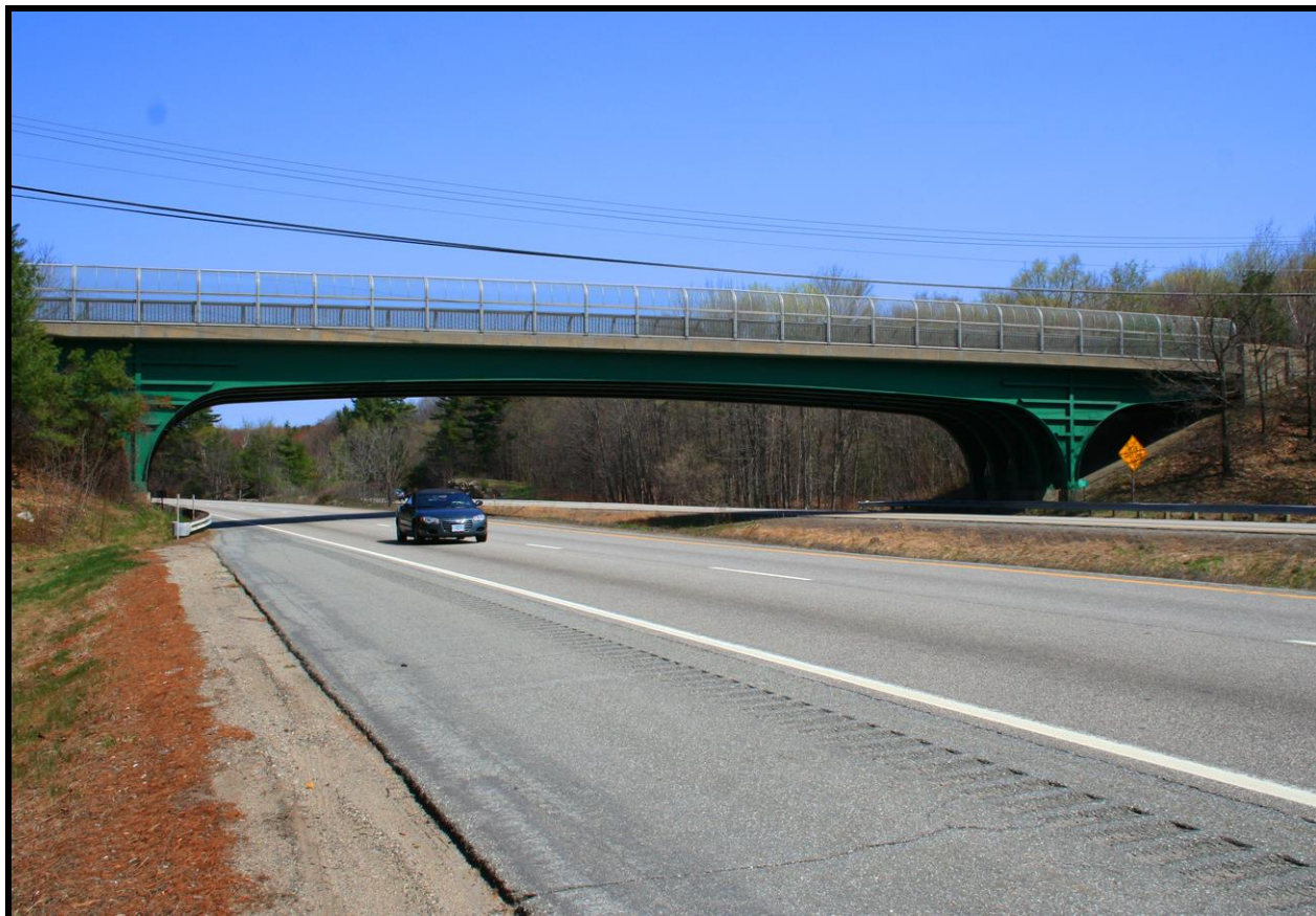
Prowse Memorial Bridge, Ash Street over I-93, Derry, NH, built 1962
