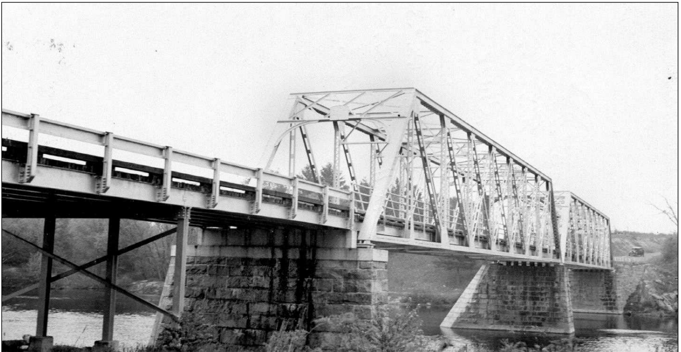
FIGURE 46: Concord 070/117, Sewall's Falls Bridge, downstream elevation. Field inspection photo made by NHHD engineer Wendell H. Piper, May 15, 1942 (NHHD Bridge Inventory Card).
