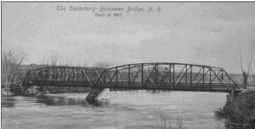
FIGURE 5: Boscawen-Canterbury 132/085, a 2-span riveted Parker truss designed by John Storrs, built by United Construction Company in 1907 to replace 1857 covered bridge. Demolished 2015. Postcard photo undated (Canterbury Historical Society).
