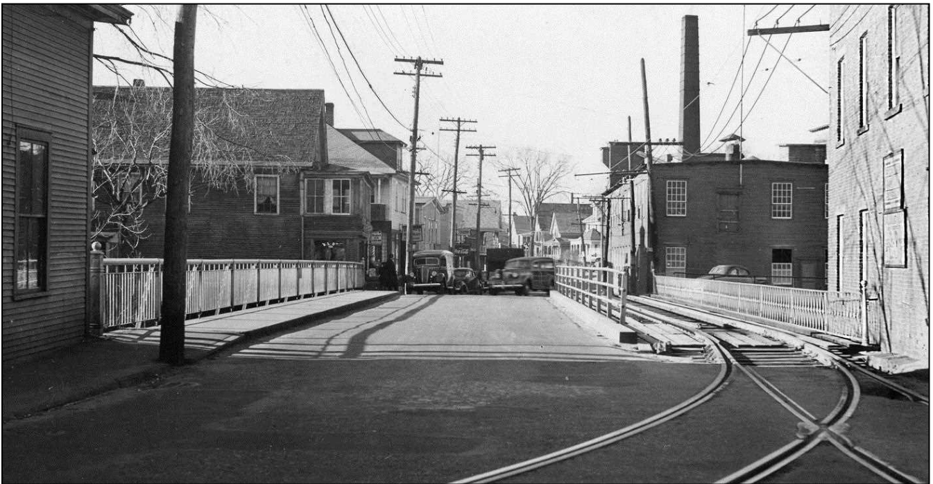
FIGURE 49: Claremont 122/098, "Lower Village Bridge" (1915). Note the Claremont Railway tracks carried on a separate Warren deck truss span erected in 1903 which limited the width of the highway bridge to 20 feet. Photo November 19, 1940 (NHHD Bridge Inventory Card).
