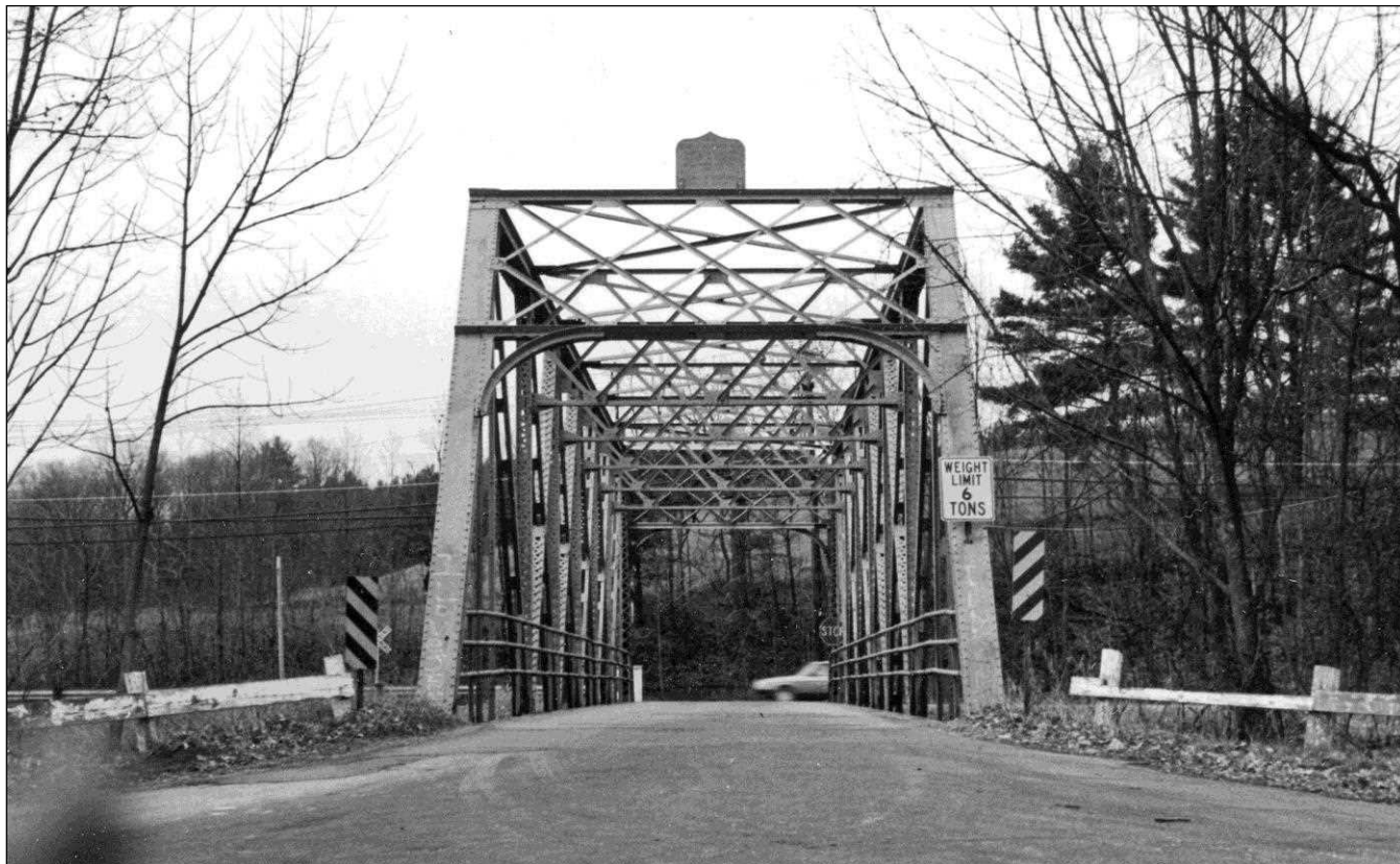
FIGURE 21: Milford 062/138. Jones Crossing Bridge over Souhegan River, a single span Pratt thru truss designed by Storrs in 1908, built by Canton Bridge Co., Canton, Ohio in 1910, demolished in 2015. Clear span between bearings of 150 feet. Photo November 20, 1989 (NHHD Bridge Inventory Card).
