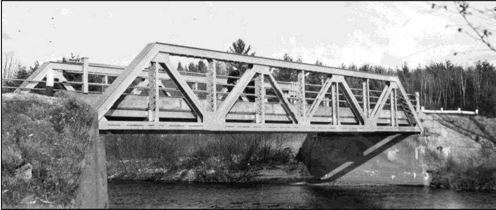
FIGURE 69: Canaan 103/049, US 4 over Mascoma River. Storrs designed this 73' Warren pony truss under the Federal Aid program for federally designated highways. Built by United Construction Co. in 1919, replaced in 1965. Storrs designed an identical span, also over Mascoma River in 1921, see below. Photo November 25, 1940 (NHHD Bridge Inventory Card).
