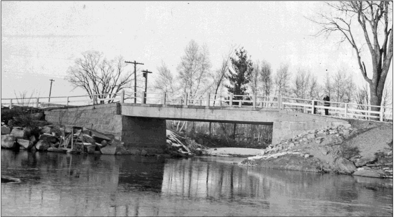
FIGURE 63: Conway 062/042, River Road over Lovejoy Brook. This concrete T-beam bridge was built 1917 with a clear span of 41'-6". Replaced in 1961. Contractor undetermined. Photo November 25, 1941 (NHHD Bridge Inventory Card).
