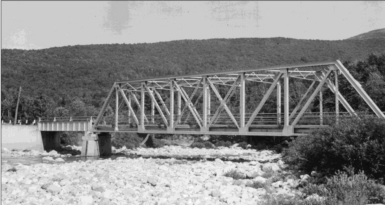
FIGURE 30: Gorham 092/058, NH 16 over Peabody River. Built 1912 by United Construction Co., Replaced in 1950. One high Pratt truss span and one thru-plate-girder span. The truss had eight panels, 16'-0" long, for a total length between the bearing pins of 128'-0". Photo August 29, 1940 (NHHD Bridge Inventory Card).
