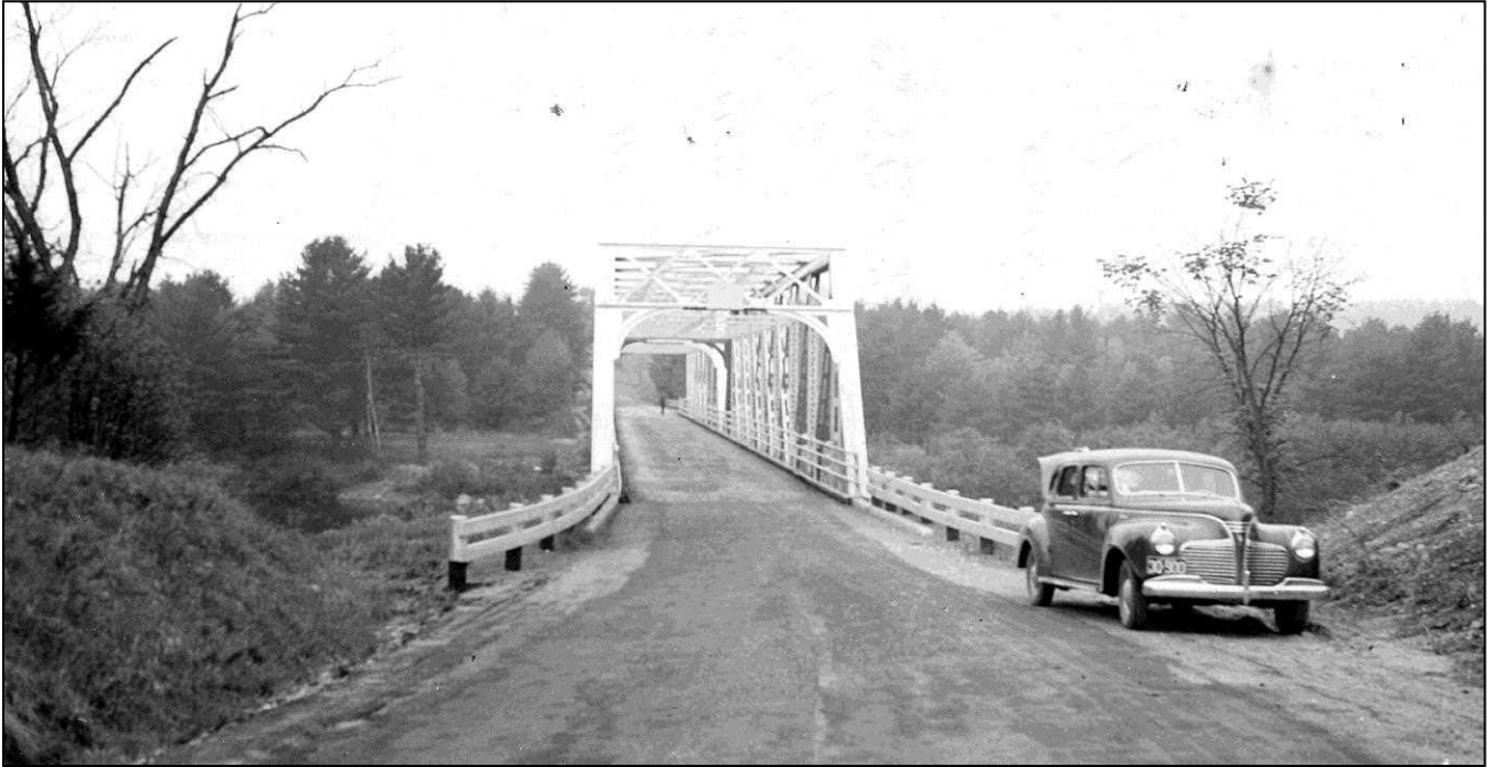
FIGURE 45: Concord 070/117, Sewall's Falls Bridge, north approach. Two 165' high Pratt truss spans carried Sewall's Falls Road over Merrimack River. Built 1915 by Berlin Construction Company, Berlin, CT. Replaced in 2016. Of the five bridges that Storrs designed for the City of Concord in 1915, this was the last to be completed; it opened on December 23, 1915. Field inspection photo made by NHHD engineer Wendell H. Piper, May 15, 1942 (NHHD Bridge Inventory Card). Also see Cover Photo.
