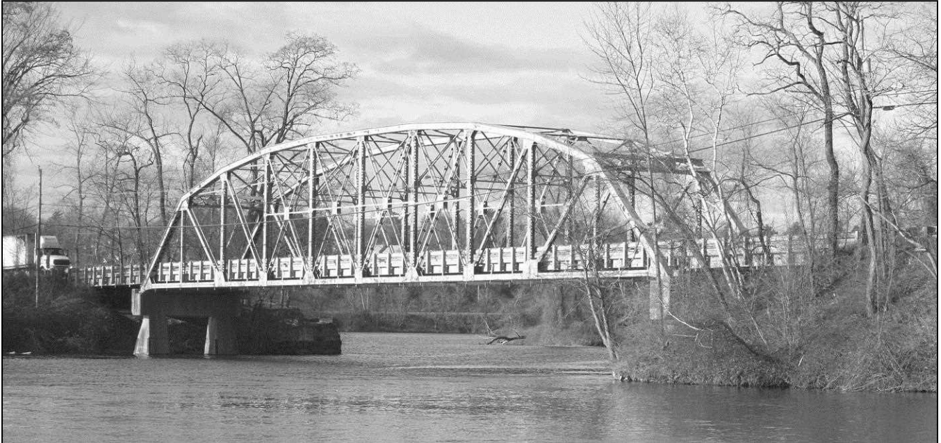
FIGURE 75: Hinsdale 042/044, "Hinsdale Bridge," carries NH 119 over the east channel of the Connecticut River between "the mainland" and a small island in the river. This single-span riveted Parker truss (a Pratt truss with a polygonal top chord) is 200 feet long. It was designed by Storrs for the Town of Hinsdale and erected by the Boston Bridge Works in 1926. It replaced a covered bridge, thought to be largely the same bridge built in 1862. Single plate girder approach spans are located at each end of the bridge. Photo by NHHD, June 11, 1941, shows downstream side taken from Hinsdale shore. (NHHD Bridge Inventory Card).
