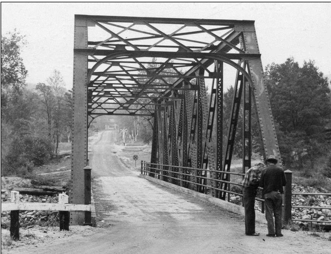
FIGURE 29: Shelburne 075/110, North Road over Androscoggin River. Built 1912, replaced in 1973. This single-span riveted high Pratt truss had eight panels, 17'-4" long, for a total length of 138'-0" between the bearing pins. Note NHHD engineers conducting inspection of bridge, September 23, 1941 (NHHD Bridge Inventory Card).
