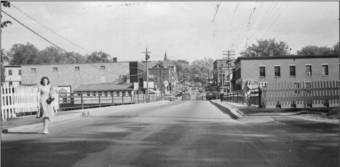
FIGURE 43: Concord 040/090, Main Street Bridge Penacook (1915). Photo, north approach, dated June 12, 1940 (NHHD Bridge Inventory Card).
