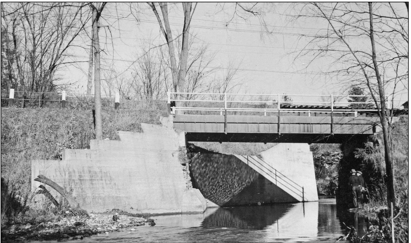
FIGURE 14: Claremont 106/120, NH 12/103 over Red River Brook. Designed by John Storrs and built by C. E. Walbridge, Plymouth NH in 1908. Replaced in 1997. This was a 30' span I-beam stringer bridge with a reinforced concrete slab deck. Photo November 19, 1940 (NHHD Bridge Inventory Card).
