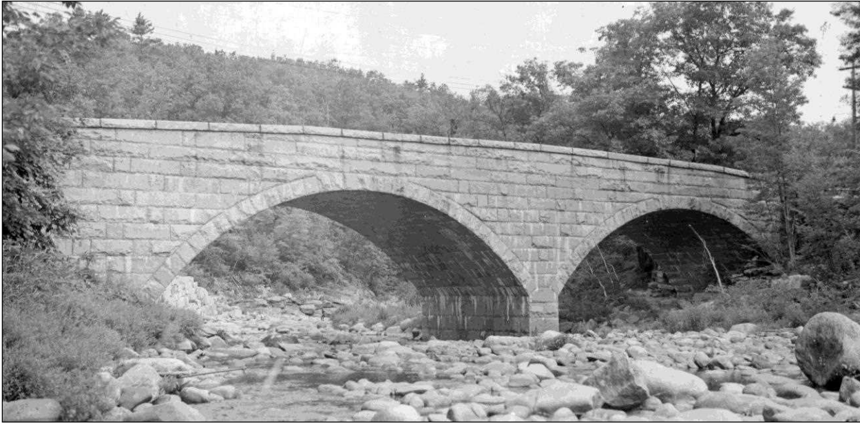
FIGURE 67: Milford 052/135, "County Bridge" (1917). Each arch has a clear span of 60 feet. Note the remarkable similarity to the arch bridge designed three years later for Barre, Vermont shown in Figure 68. Photo July 29, 1940 (NHHD Bridge Inventory Card). Bridge remains in service.
