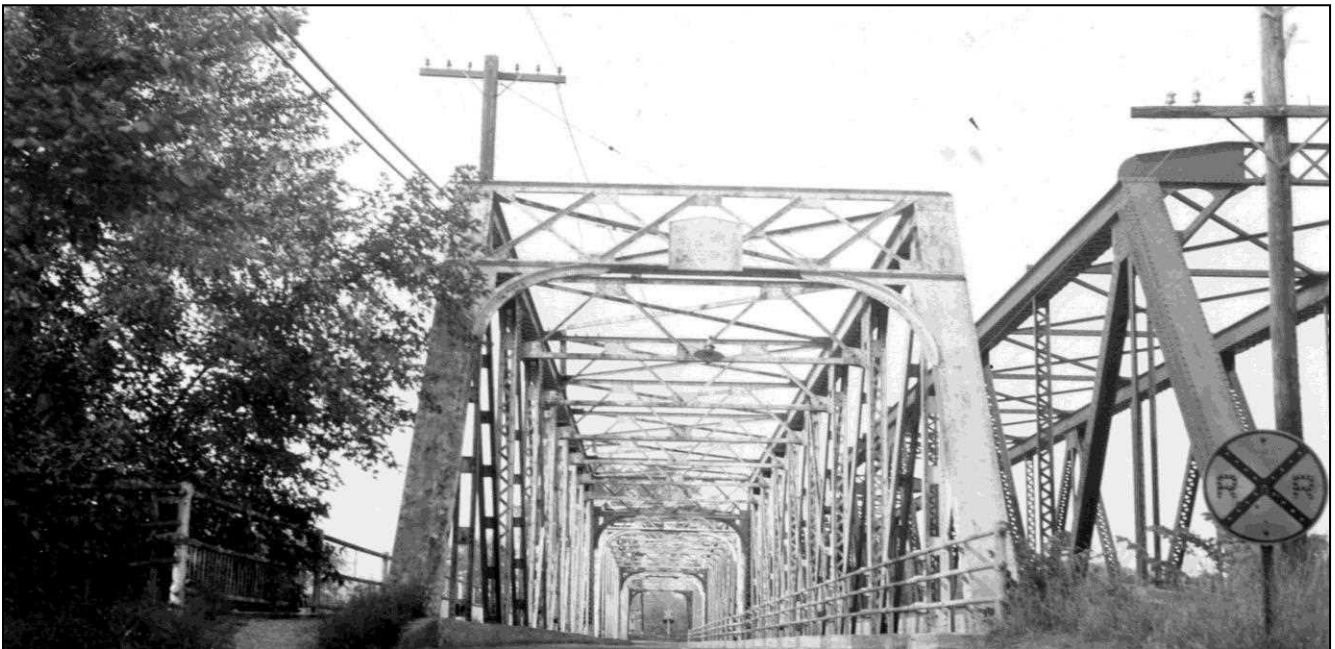
FIGURE 40: Concord 136/115, Federal Bridge (1915). Photo c. 1940 showing south approach and portal with Boston & Maine Railroad Bridge at right (NHHD Bridge Inventory Card, no date, c. 1940).
