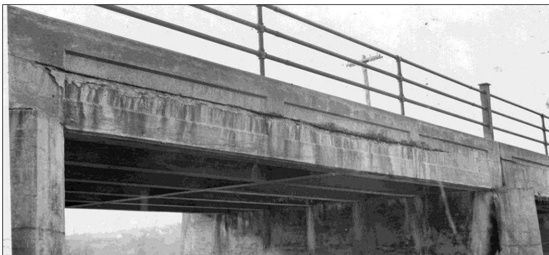
FIGURE 61: Elm Street Bridge, Newport (1916). Section sketch showing concrete encased I-beams, an inefficient and short lived bridge type that was incorrectly identified in bridge records as a concrete T-beam bridge (NHHD Bridge Inventory Card).
