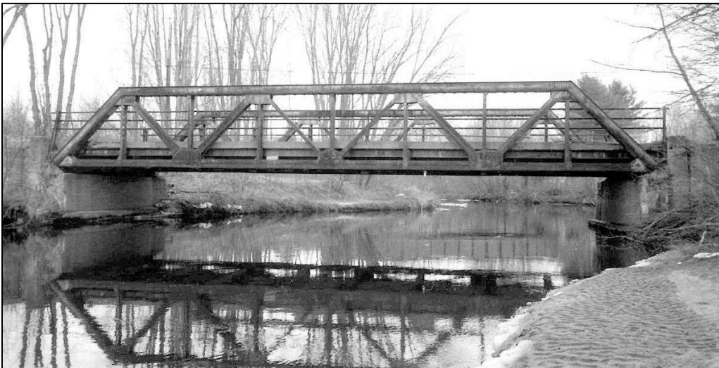
FIGURE 70: Canaan 091/030, Blackwater Road over Mascoma River. Designed by Storrs and built by United Construction Co. in 1921. This bridge was documented in 1992 prior to demolition and included large-format photographs, Storrs' original plans and fabrication shop drawings. Documentation photo dated April 2, 1992 (NHDHR HPD NH-519).
