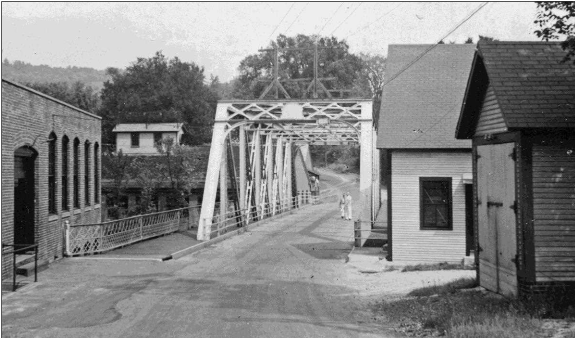
FIGURE 1: Claremont 091/118, Plains Road over Sugar River. This single 131' span high Pratt truss was designed by John Storrs and built by United Construction Co. in 1906. Replaced in 1974. Photo August 26, 1942 (NHHD Bridge Inventory Card).
