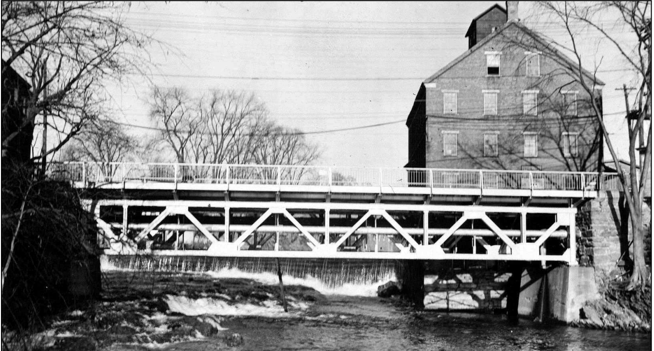
FIGURE 48: Claremont 122/098, "Lower Village Bridge" carrying Main Street over Sugar River. Storrs designed this 100' Warren deck truss for the City in 1915, as well as the Broad Street Bridge (Figures 51-52). Built by Boston Bridge Works at a cost of $7,990. Storrs was paid $399.50 for engineering services. The bridge was documented to HAER standards in 1995 prior to its replacement the next year (see HAER NH-23). Photo November 19, 1940 (NHHD Bridge Inventory Card).
