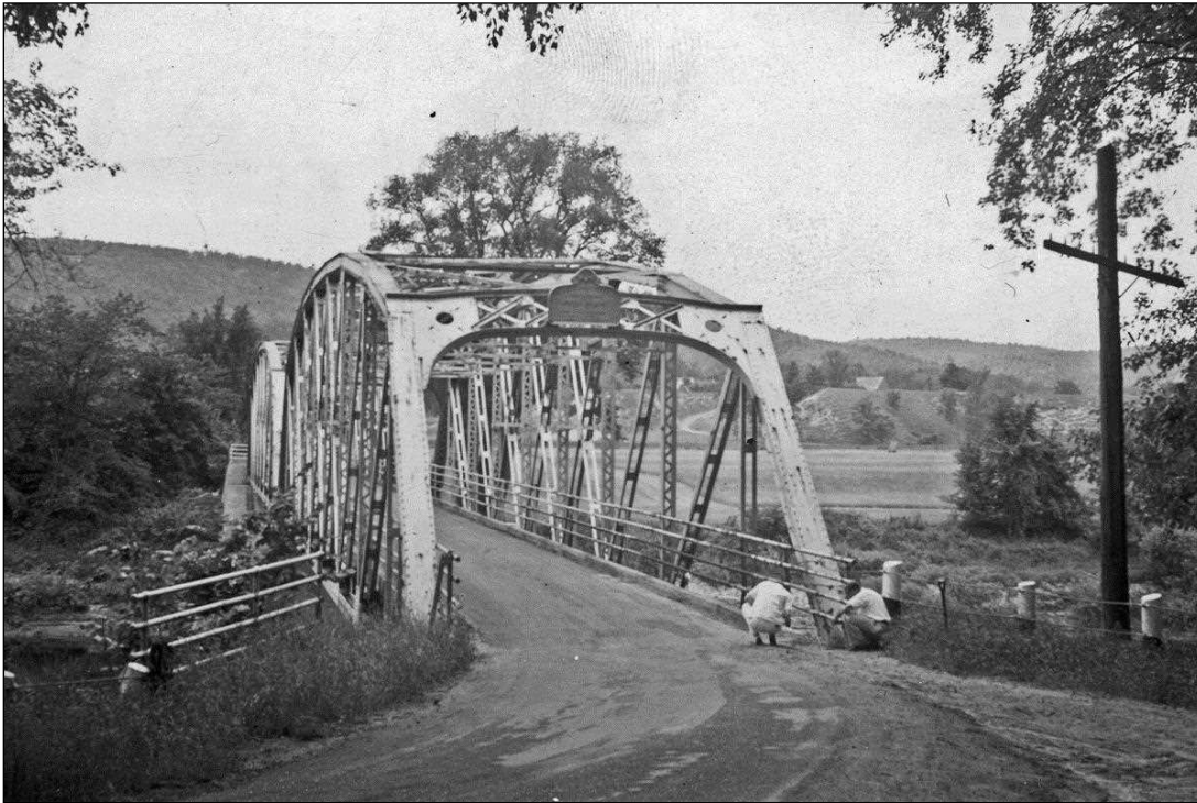
FIGURE 32: Haverhill 099/149, Newbury Road Bridge over Connecticut River between Haverhill NH and Newbury VT, built 1913, replaced in 1968. John W. Storrs designed repairs for the rare two-lane, three truss covered bridge built 1834 that predated this structure. A flood in 1913 damaged the bridge and it was taken down and replaced with the two-span Pratt truss steel bridge shown above in 1942. United Construction Company built the bridge on new concrete abutments and center pier; Storrs served the towns as consulting engineer. Photo July 22, 1942 (NHHD Bridge Inventory Card).
