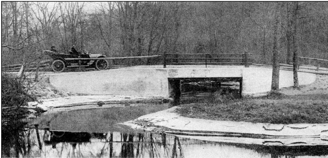
FIGURE 25: Bow 135/160 Turkey River Bridge, an 18' span jack arch built 1911 by Boston Bridge Works. Upstream side, pictured in Storrs & Storrs bridge construction handbook (Storrs & Storrs, 1918, p. 11). Demolished and replaced in 1959 with I-89 Ramp.
