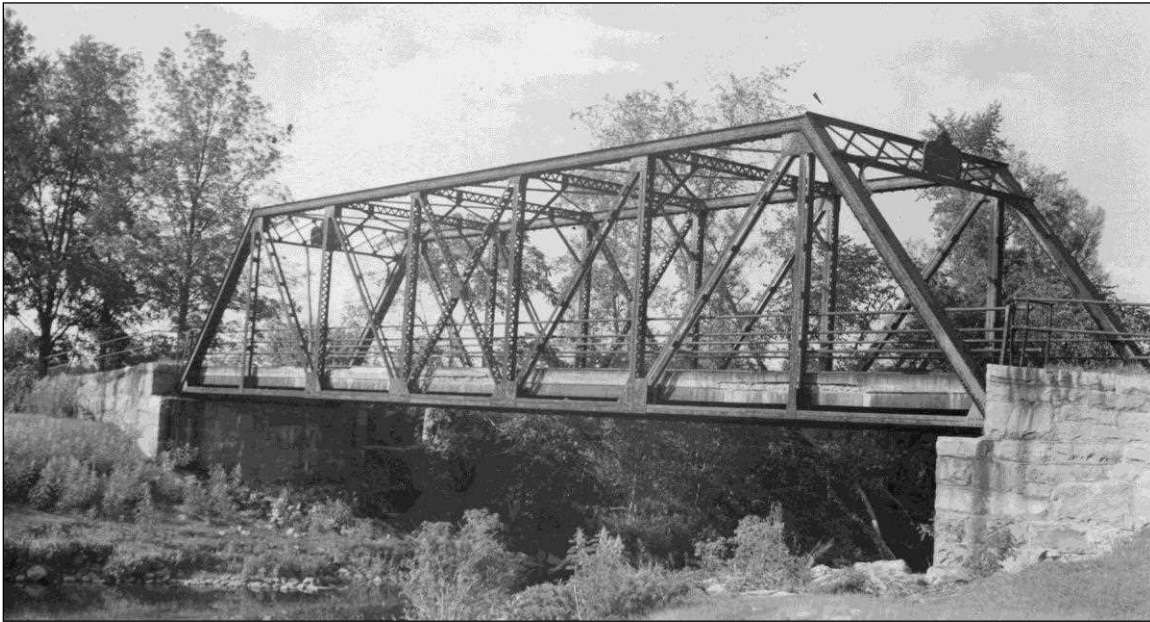
FIGURE 28: Amherst 186/107, "Cricket Corner Bridge" carrying NH 122 over Souhegan River. This single-span riveted high Pratt truss was built in 1912 by United Construction Co. Replaced in 1956. Storrs designed at least five high Pratt truss bridges in 1912. This one had seven panels, 14'-10" long, for a total length between the bearing pins of 103'-10". Photo August 9, 1940 (NHHD Bridge Inventory Card).
