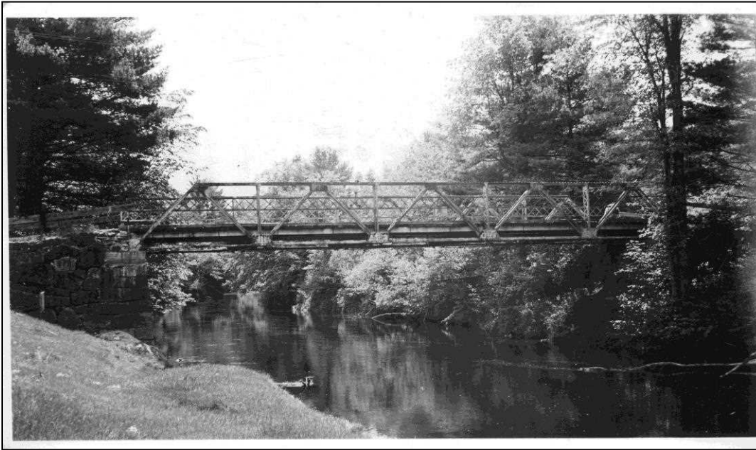
FIGURE 9: Hopkinton 134/166, East Penacook Road over Blackwater River. A single 70' span Warren pony truss, designed by John Storrs and built by United Construction Company, 1907. Replaced in 1967. This bridge replaced a covered bridge that Storrs inspected for Hopkinton Selectmen in April 1907. He reported that "To properly and effectively repair your bridge and put it into safe condition would cost from $500 to $600; this includes shingling the roof. The bridge would then probably be alright for several years. An estimate for a steel bridge to take the place of the present structure, would be from $1200 to $1500." The new bridge was chosen and set on reinforced concrete bridge seats cast atop the existing stone abutments. Photo May 27, 1942 (NHHD Bridge Inventory Card).
