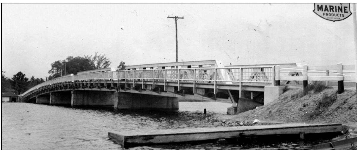
FIGURE 57: Belmont-Tilton 072/148, Winnisquam Bridge. Downstream side. Field inspection photo made June 13, 1940 (NHHD Bridge Inventory Card)
