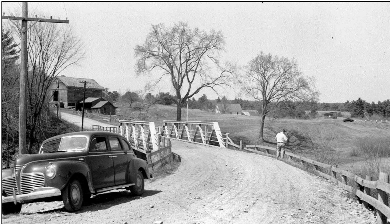
FIGURE 35: Concord 163/185 over Soucook River. Known as "Richardson Mill Bridge." This 81-foot Warren pony truss was designed by Storrs for the City of Concord and built by Berlin Construction Co. in 1914. Demolished 1988. Photo April 24, 1942 (NHHD Bridge Inventory Card).
