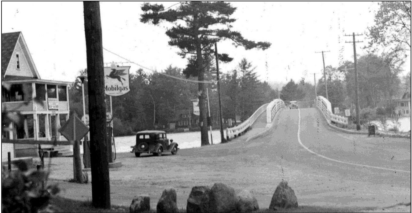
FIGURE 58: Belmont-Tilton 072/148, Winnisquam Bridge (1916). North approach. Field inspection photo made June 13, 1940 (NHHD Bridge Inventory Card)
