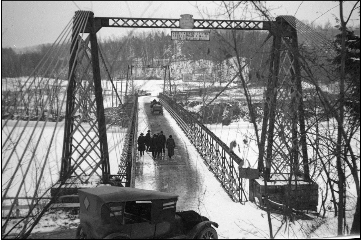
FIGURE 19: In the winter of 1921 John Storrs inspected ice damage to the abutments of the Chesterfield-Brattleboro Suspension Bridge along with town officials. The famous bridge was built in 1889 by the Berlin Iron Bridge Company with a clear span of 320 feet. The roadway was carried on a through-truss suspended from fourteen individual cables strung over iron towers. Repairs were made and the bridge continued to serve until November 6, 1935 when the truss was found severely buckled and broken in several places. The damaged had been done by an overweight ten wheel truck and trailer that snuck over the bridge the night before. The bridge was again repaired to carry light traffic but the following March it was inundated and ripped from its anchorages by the Great Flood of 1936. The cables were salvaged to support a temporary pedestrian suspension bridge over the Merrimack River at the site of Manchester's MacGregor Bridge (aka the Notre Dame Bridge), which had also been destroyed by the flood (Storrs Photograph Collection).
