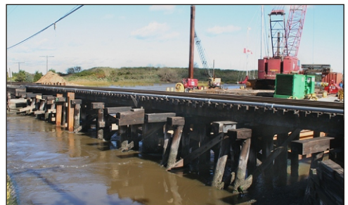
NJ Transit Railroad Trestle over Manasquan River Brielle, NJ
