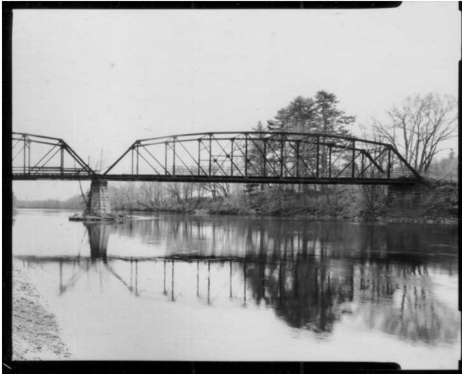
NH-669-8 Upstream elevation of west span. Looking southeast.
