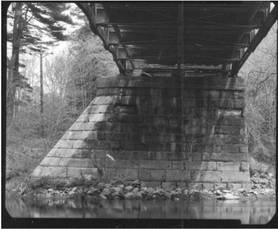
NH-669-16 Pier, west elevation. Looking northeast.
