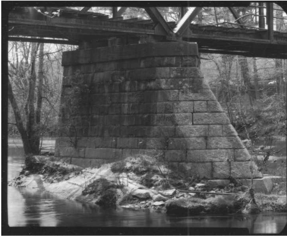
NH-669-17 Pier, east elevation. Looking south.
