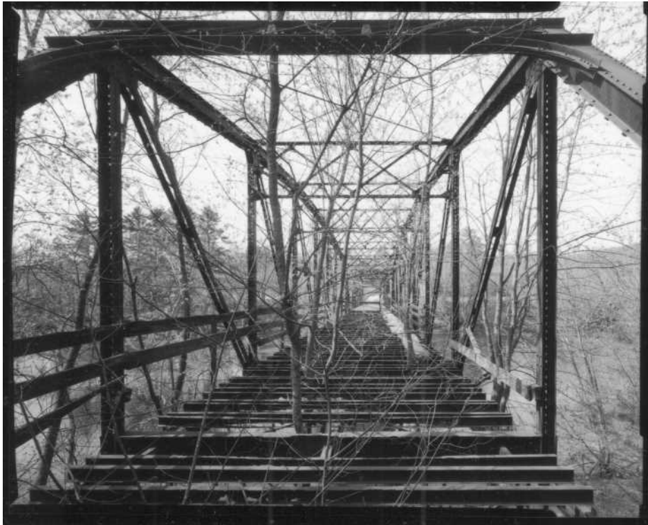
NH-669-10 East (Canterbury) portal and barrel view through trusses. Looking southwest.
