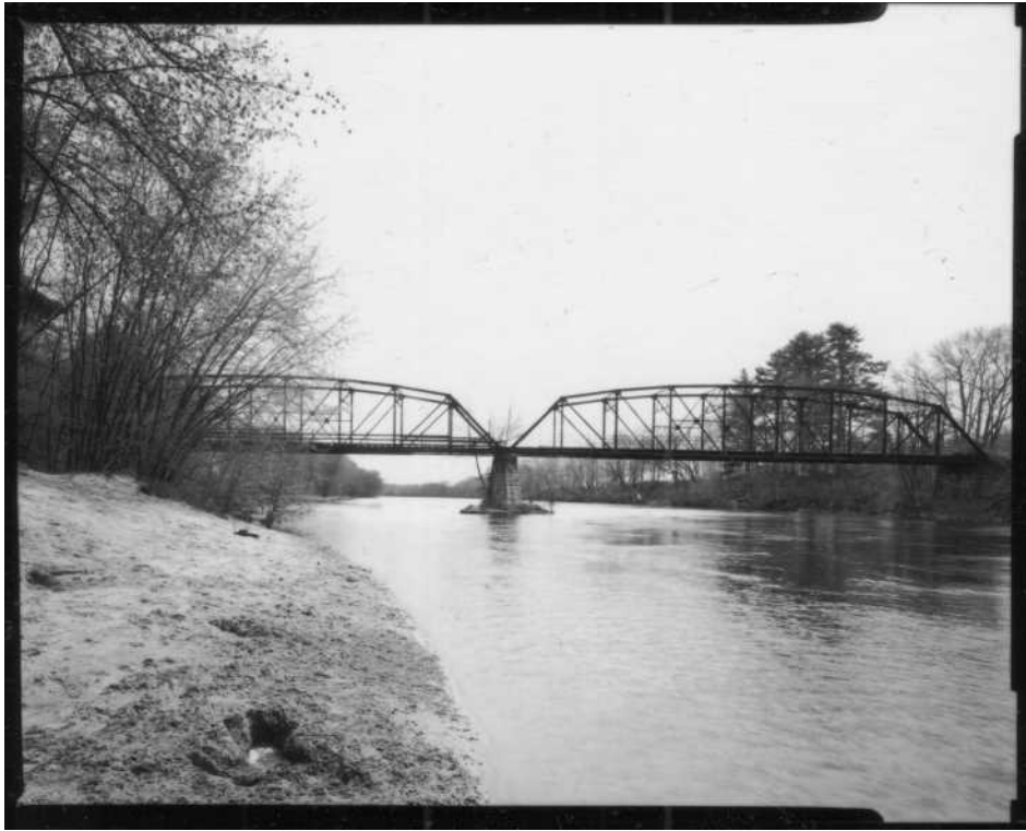
NH-669-7 Upstream elevation of bridge spans. Looking southeast.
