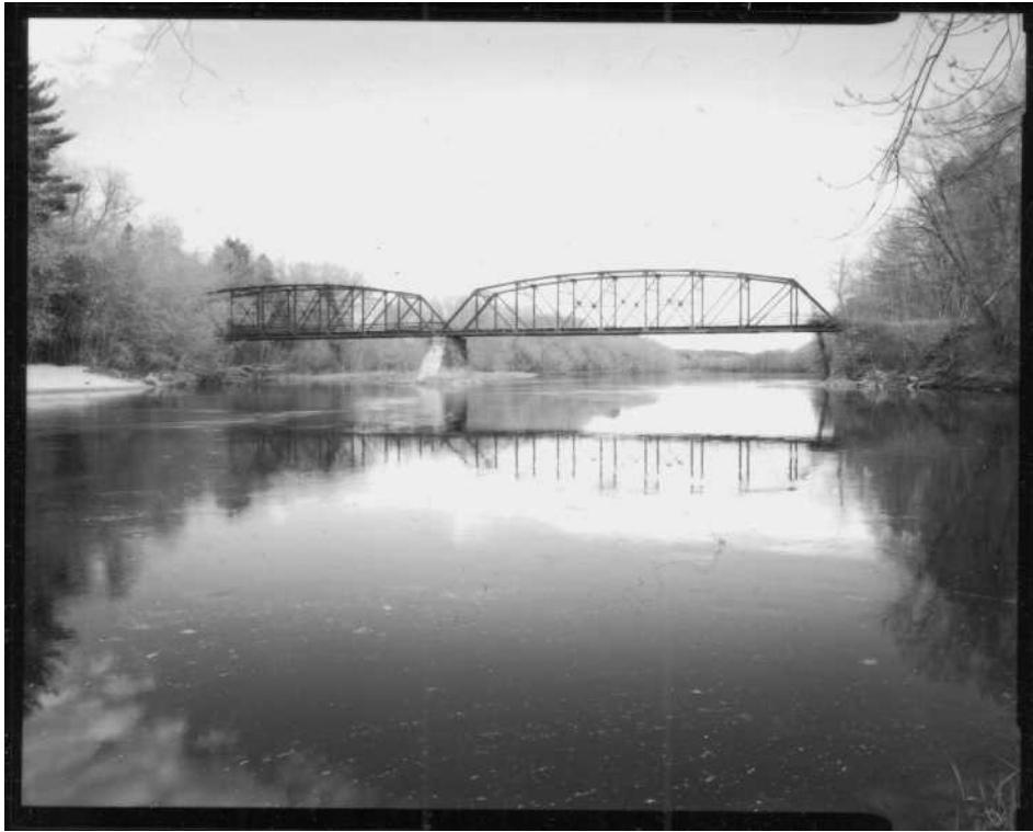
NH-669-5 View of bridge in context from upstream. Looking east.
