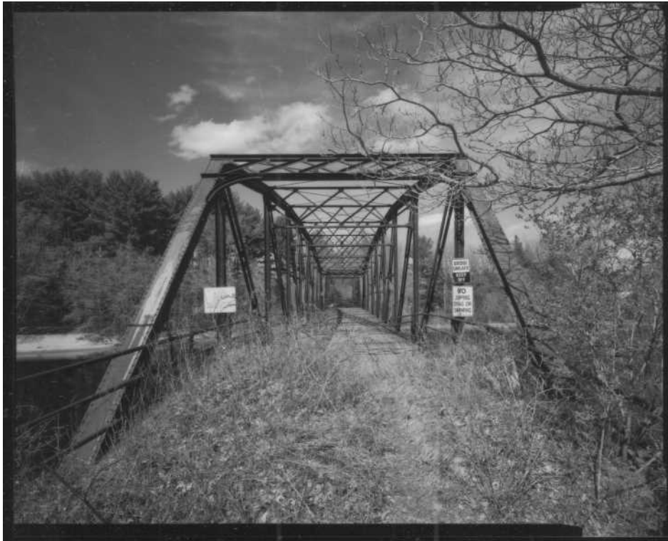
NH-669-9 West (Boscawen) portal and barrel view through trusses. Looking northeast.
