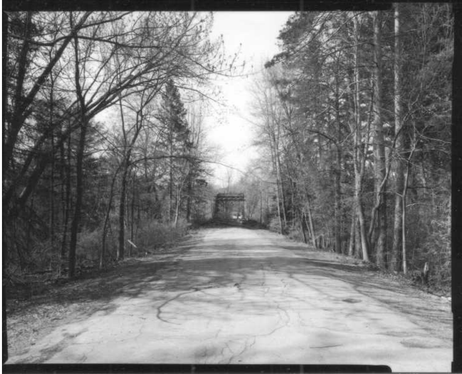
NH-669-1 East approach to bridge (Canterbury end). Looking southwest.
