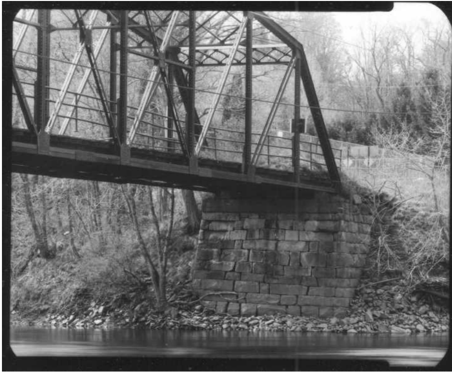
NH-669-13 West (Boscawen) abutment. Looking south.
