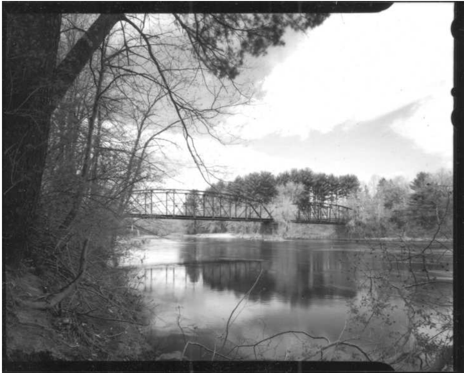
NH-669-4 View of bridge in context from downstream. Looking northwest.
