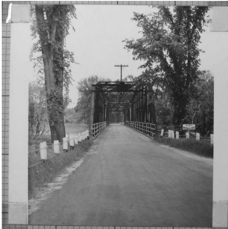
FIGURE 7: 1940 Photo of Boscawen approach, looking northeast (NHHD Bridge Inventory Card).
