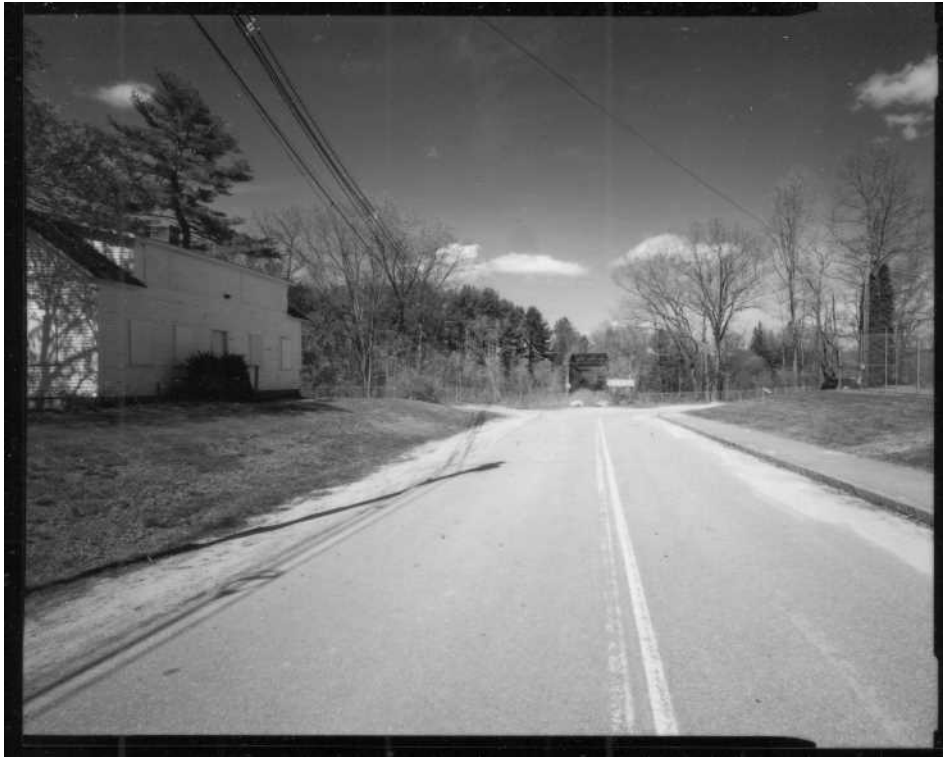
NH-669-2 West approach to bridge (Boscawen end). Looking northeast.
