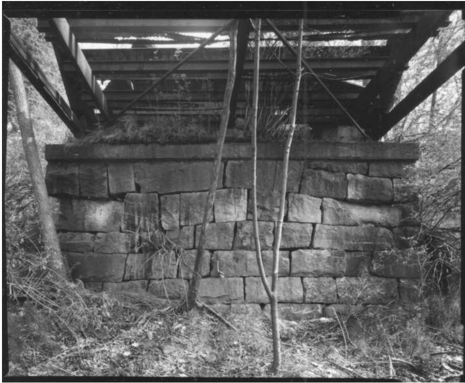
NH-669-14 East (Canterbury) abutment. Looking northeast.
