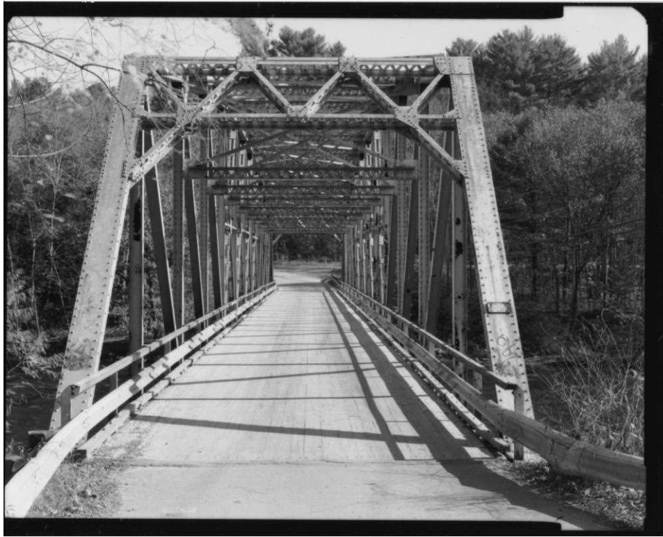
NH-599-5 West portal and deck, view east.
