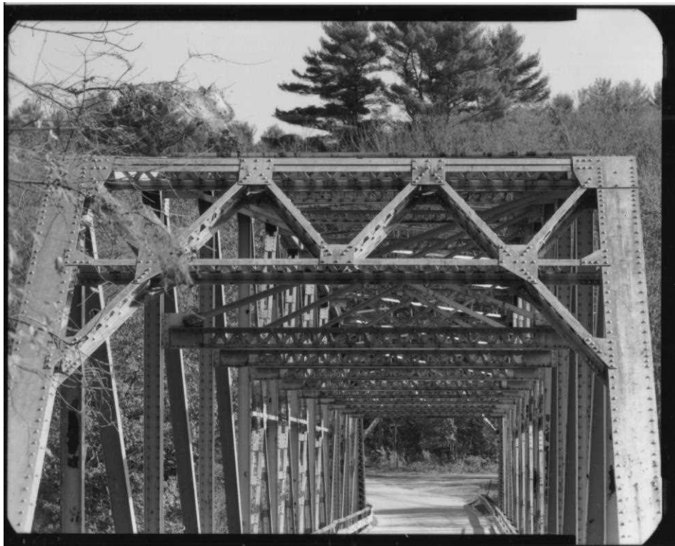
NH-599-18 Detail of portal bracing, view west.
