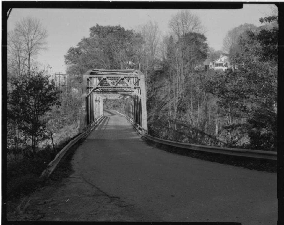
NH-599-4 East approach, showing full portal, view west.
