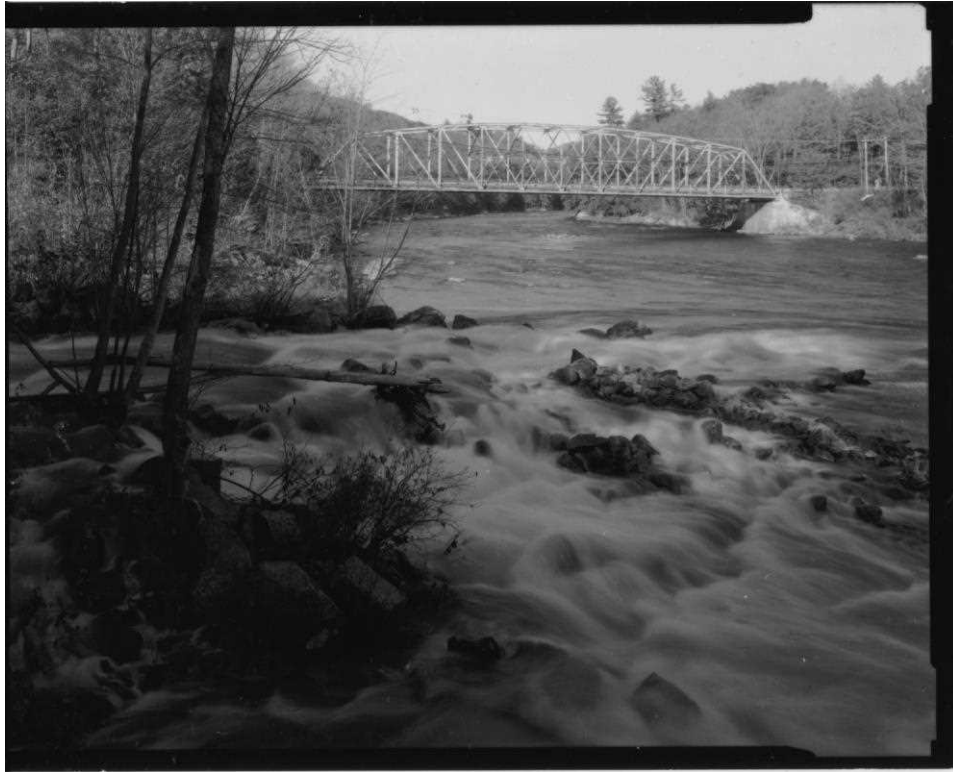
NH-599-1 Overall view of bridge in context, view north.
