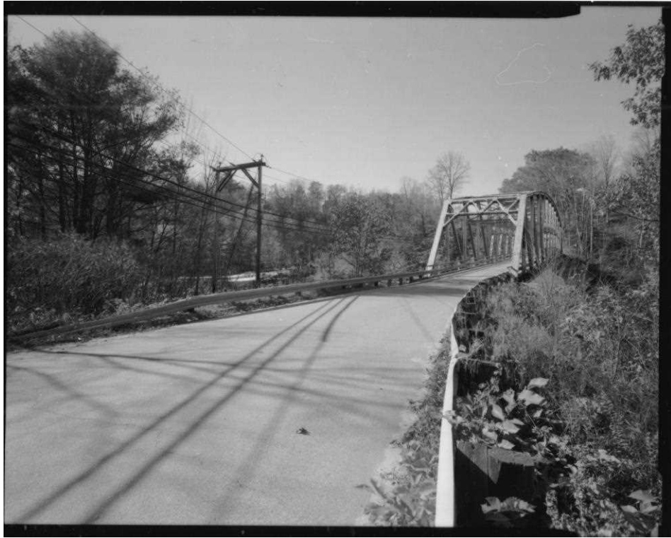
NH-599-3 West approach, view northeast.
