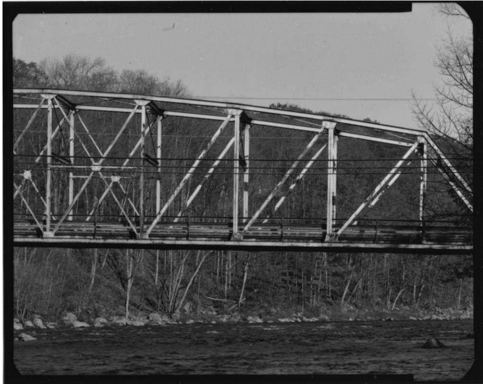
NH-599-7 Elevation of four individual panels along south elevation, view north.
