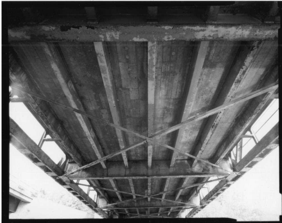
NH-599-12 Close-up underside detail of floor system, view east.
