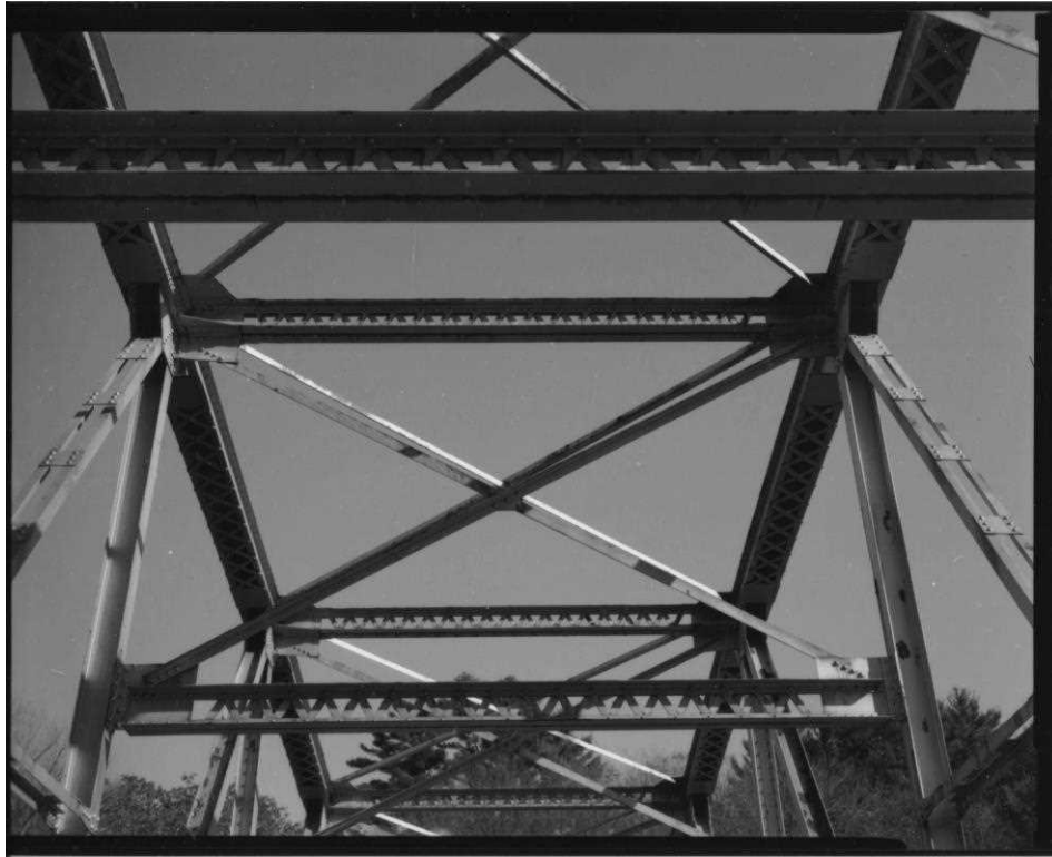
NH-599-17 View of upper struts, laterals, sway-brace, view east.
