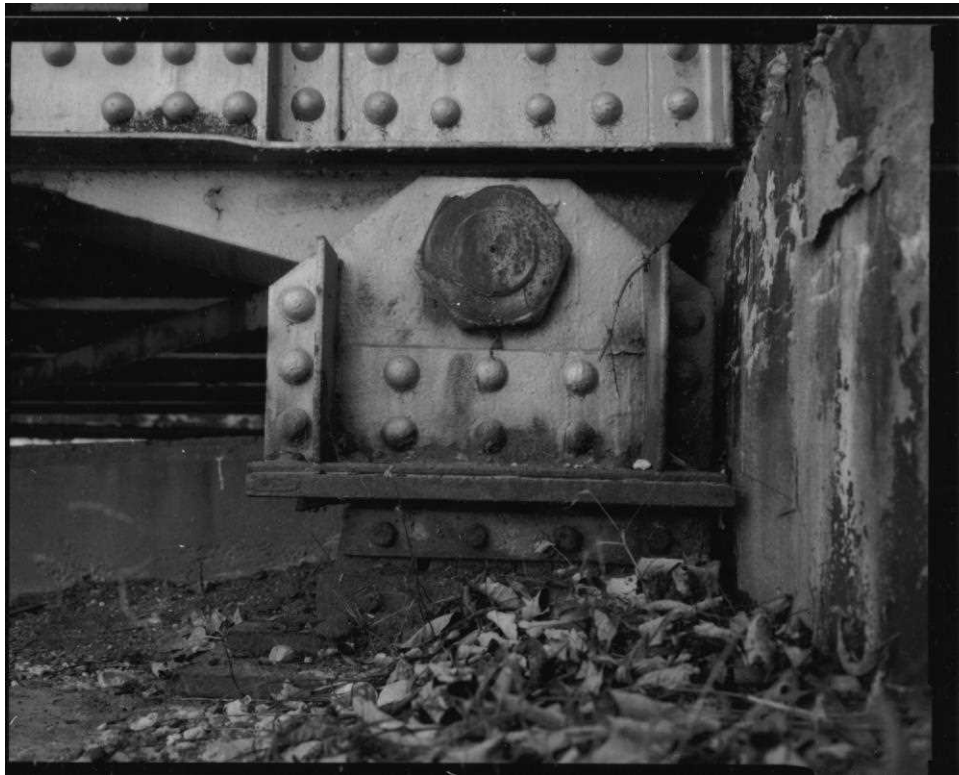
NH-599-14 Detail of northwest expansion bearing, view south.
