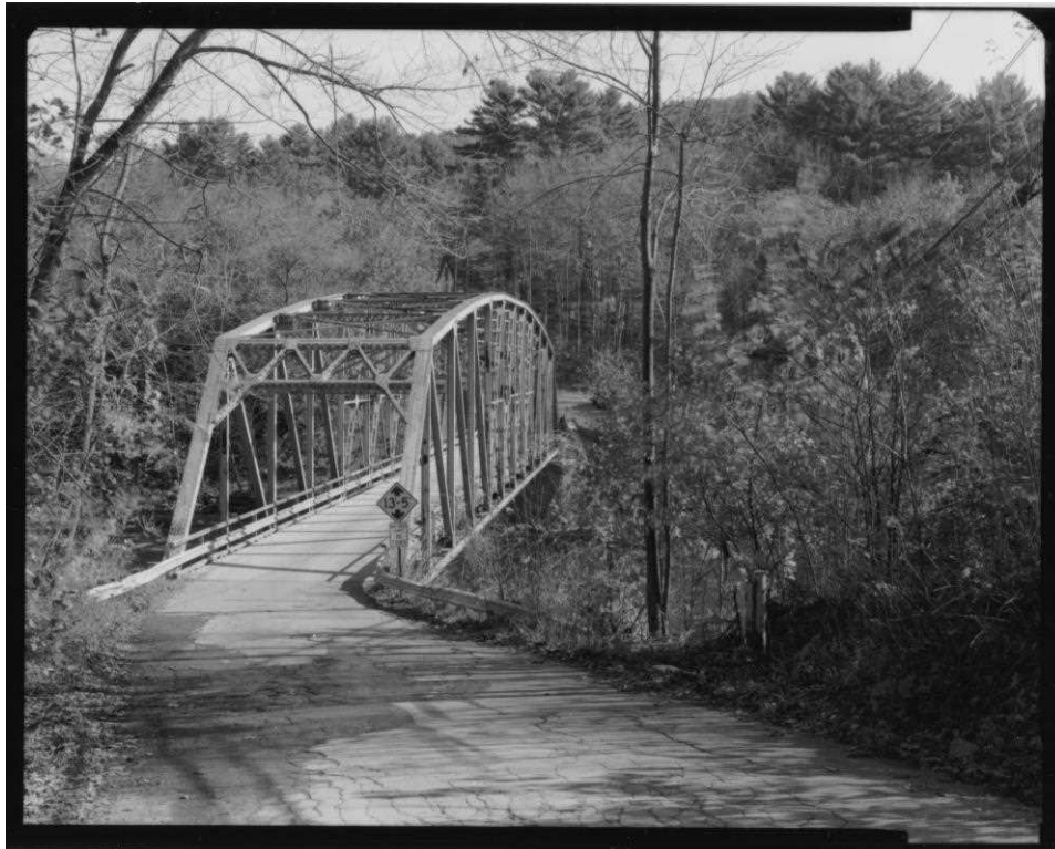
NH-599-2 Overall view of bridge in context, view west.
