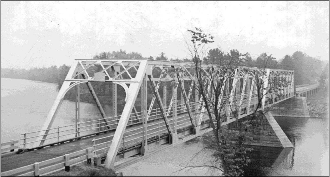
FIGURE 31: John Storrs co-designed bridge. Concord 070/117, Sewells Falls Bridge, two span Pratt thru truss carrying Sewells Falls Road over Merrimack River, built 1915, replaced 2016. W. B. Howe, city engineer, also named on plans. Berlin Construction Company, Berlin, CT, contractors. Two 165' spans. Photo May 15, 1942 (NHHD Bridge Inventory Card).
