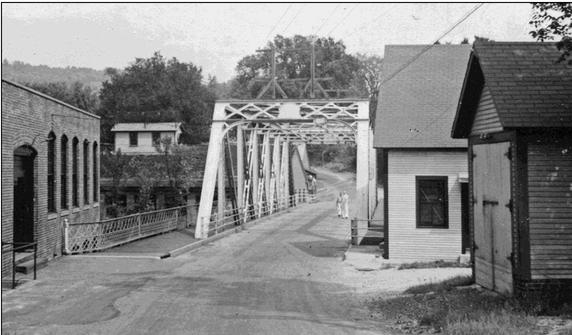
FIGURE 24: John Storrs designed bridge. Claremont 091/118, single span Pratt thru truss carrying Plains Road over Sugar River, built 1906, replaced 1974. United Construction Co., contractor. 131'-0" span between bearings. Photo August 26, 1942 (NHHD Bridge Inventory Card).
