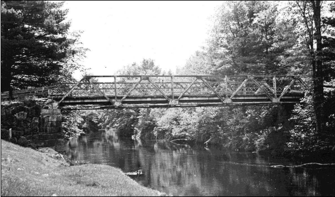
FIGURE 25: John Storrs designed bridge. Hopkinton 134/166, single span Warren pony truss carrying East Penacook Road over Blackwater River, built 1907, replaced 1967. United Construction Co., contractor. 70'-0" span between bearings. Photo June 27, 1942 (NHHD Bridge Inventory Card).
