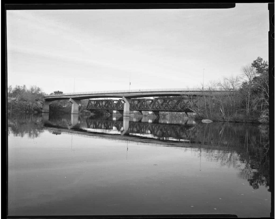
NH-737-03 Bridge in context from downstream, just visible behind Memorial Bridge and B&MRR Bridge. Looking northeast.
