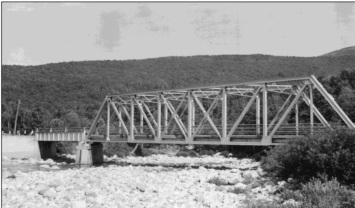
FIGURE 30: John Storrs designed bridge. Gorham 092/058, one Pratt thru truss span, one thru plate-girder span, carrying NH 16 over Peabody River, built 1912, replaced 1950. United Construction Co., contractor. 128'-0" span between bearings. Photo August 29, 1940 (NHHD Bridge Inventory Card).
