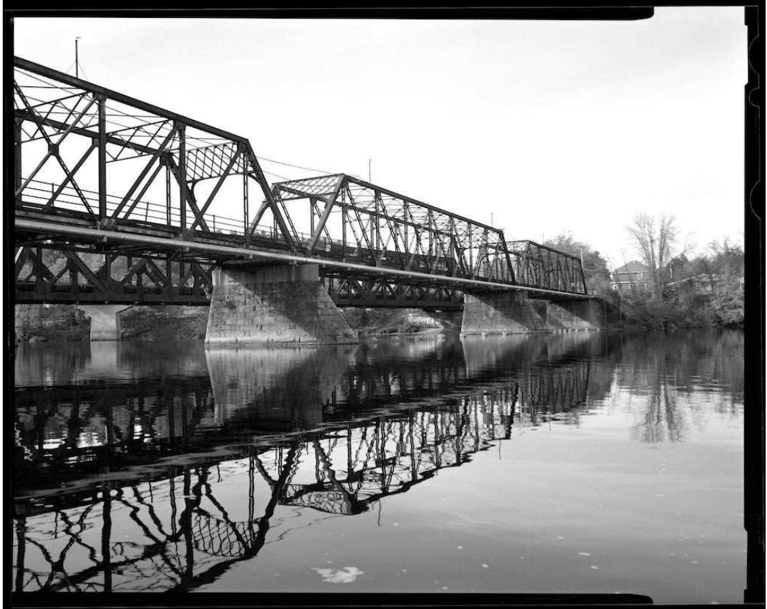
NH-737-06 Oblique view of upstream side of bridge. Looking northwest.
