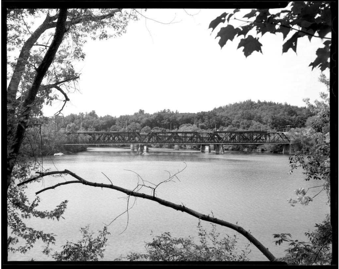
NH-737-01 Bridge in context from upstream. Looking southwest.
