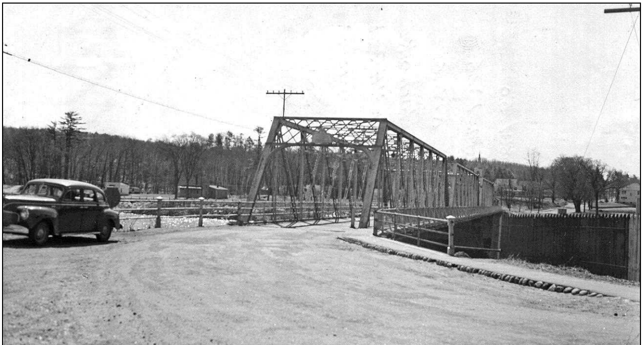
FIGURE 20: Hooksett Village Bridge, April 13, 1942, NHHD Bridge Inventory Card. Notation reads "north approach looking toward junction US 3" (NHDOT Bridge Files).
