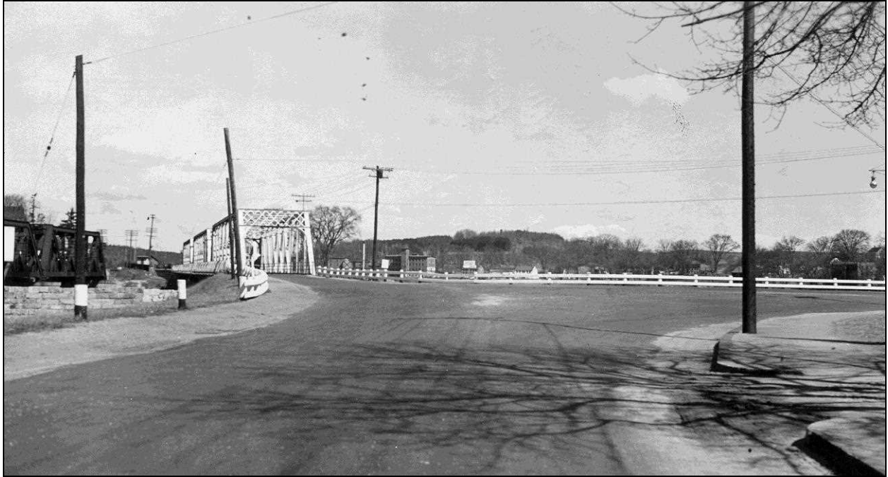
FIGURE 19: Hooksett Village Bridge, April 13, 1942, New Hampshire Highway Department (NHHD) Bridge Inventory Card. Notation reads "south approach, looking toward junction NH 3 A" (NHDOT Bridge Files).
