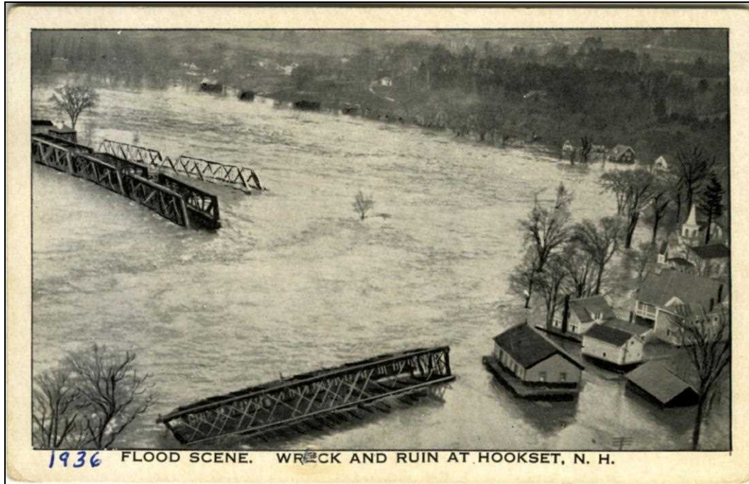
FIGURE 15: "Flood Scene. Wreck & Ruin at Hooksett, NH." Postcard 1936, Tichnor Bros. Boston, MA, publisher. The south span of the Village Bridge was carried away with the impact of a span of the B&MRR Hooksett Falls Bridge that was torn free by the flood from its location just upstream. The two remaining spans of the Village Bridge are seen at upper left; a section of the lattice truss railroad bridge is seen at bottom center, grounded or continuing downstream (Historic Documentation Co.).
