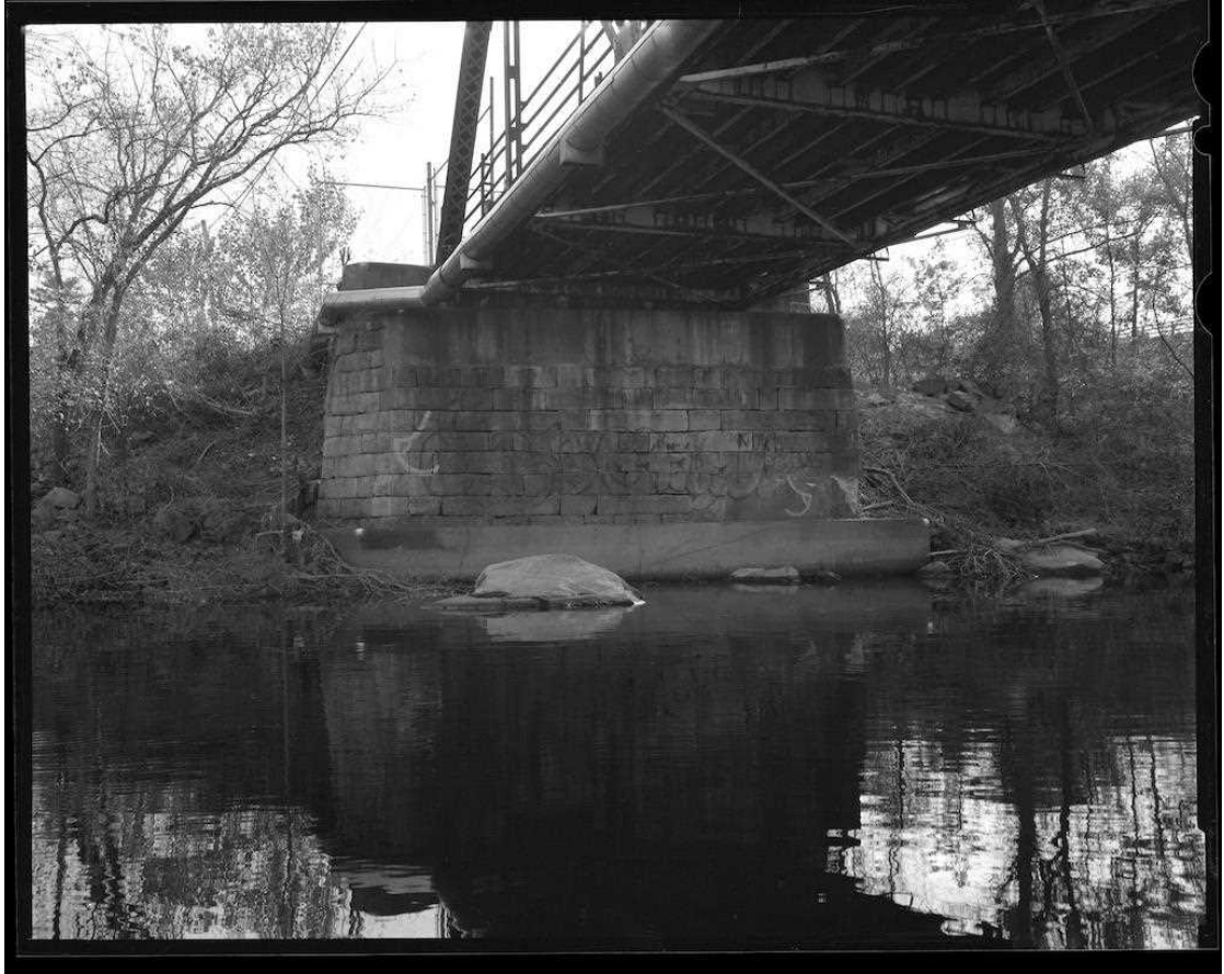
NH-737-11 South abutment. Looking south.
