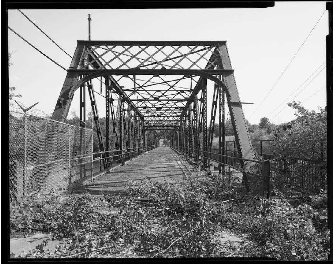
NH-737-14 North portal and barrel view through trusses. Looking south.
