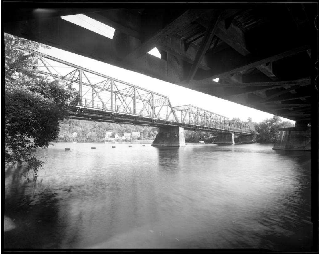
NH-737-05 Bridge in context, showing oblique elevation of downstream side, from under B&MRR Bridge. Looking southeast.
