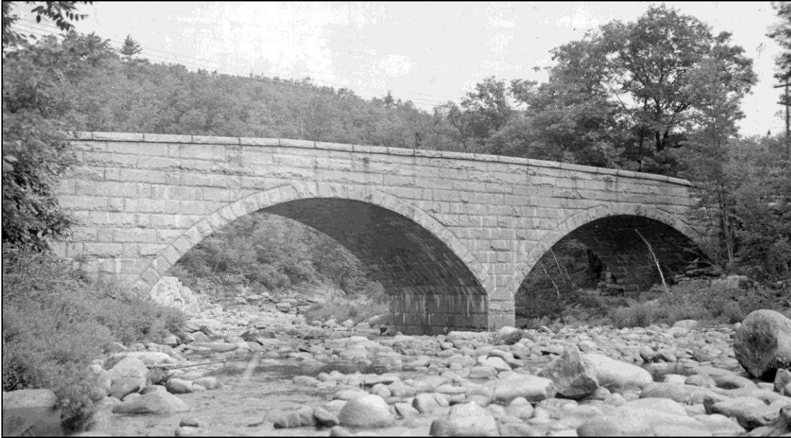
FIGURE 33: John Storrs designed bridge. Milford 052/135, "County Bridge," two span stone arch carrying Wilton Road over Souhegan River, built 1917, repaired 1950, in service. Lovejoy Granite Co, Milford, contractor. 60'-0" clear span each. Photo July 29, 1940 (NHHD Bridge Inventory Card).
