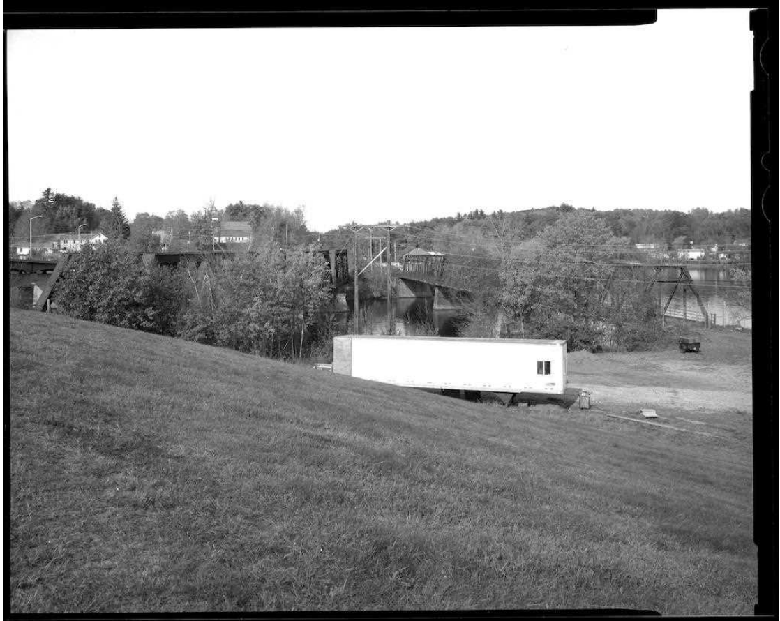
NH-737-02 Bridge in context from Memorial (Main Street) Bridge. Looking northeast.
