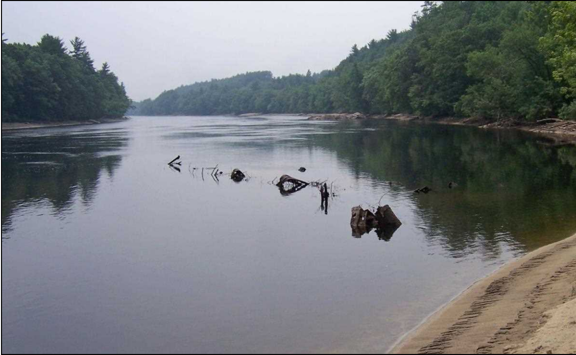
FIGURE 23: Wreckage of south truss span of Village Bridge, in river below Riverside Street about 300 feet south of Memorial Bridge. The remains are exposed during periods of low river levels when maintenance is performed on the Amoskeag Dam in Manchester (Hooksett Heritage Commission).
