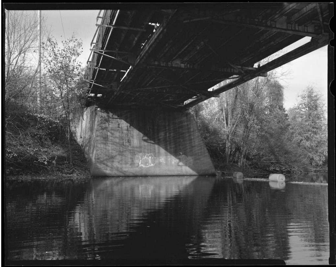
NH-737-12 North abutment. Looking north.
