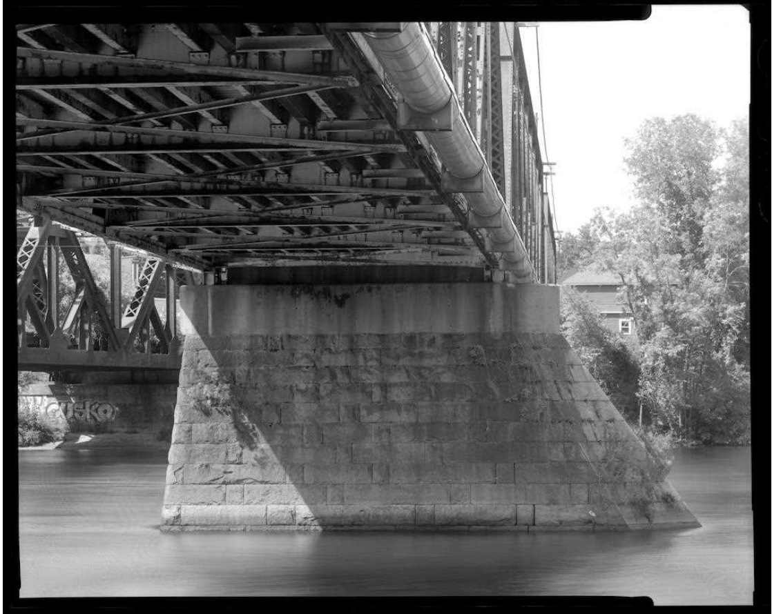
NH-737-13 Detail of South Pier, south face. Looking north.
