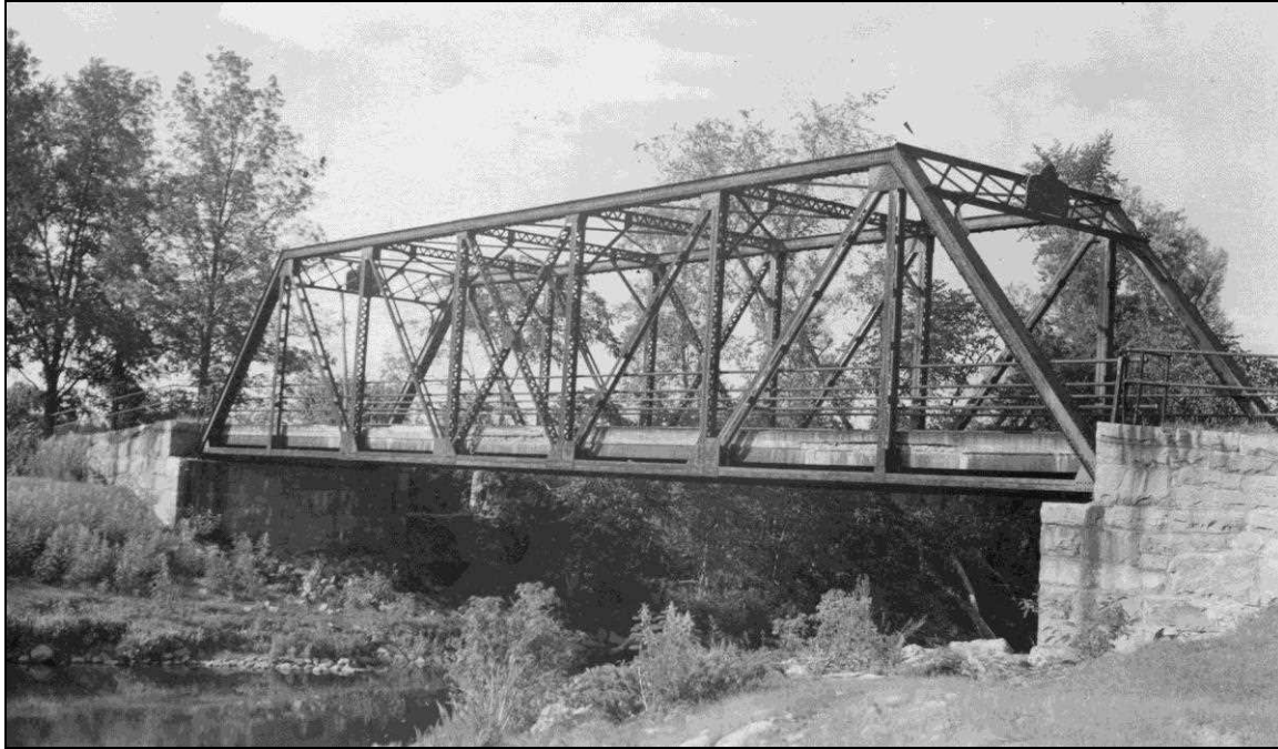
FIGURE 29: John Storrs designed bridge. Amherst 186/107, "Cricket Corner Bridge," single-span riveted Pratt truss carrying NH 122 over Souhegan River. Built 1912, replaced 1956. United Construction Co., contractor. 99'-9" clear span. Photo August 9, 1940 (NHHD Bridge Inventory Card).
