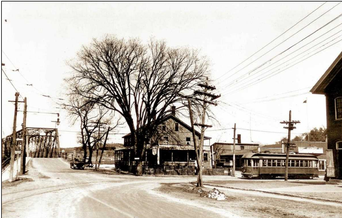
FIGURE 14: Photograph taken before 1933 of south approach to Village Bridge, left, showing trolley line and buildings on Common Avenue before alteration of area by 1936 flood (Hooksett Heritage Commission).
