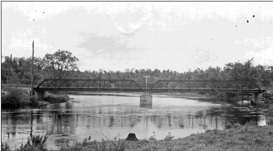
FIGURE 28: John Storrs designed bridge. Tilton-Northfield 128/158 (now 109/062), two span Warren pony truss carrying NH 140 over Winnepesaukee River. Built 1910, replaced 1968. Canton Bridge Co., contractor. 67'-7" span (each) between bearings. Photo June 17, 1942 (NHHD Bridge Inventory Card).
