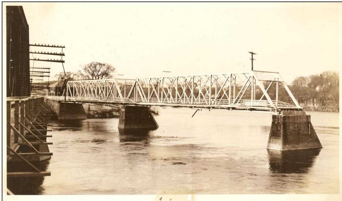
FIGURE 16: Village Bridge, photograph, 1936, after Flood of 1936, showing south span missing, right, and temporary sidewalk erected on B&MRR Bridge, left. Note original iron-lattice sidewalk railing on Village Bridge with sections missing and bent over. The railing was completely replaced with a more modern steel balustrade railing as part of the contract that replaced the lost span (Hooksett Heritage Commission).
