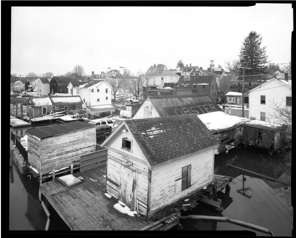
NH-566-3: View, showing north and east side of property taken from Peirce Island Bridge. Looking southwest.
