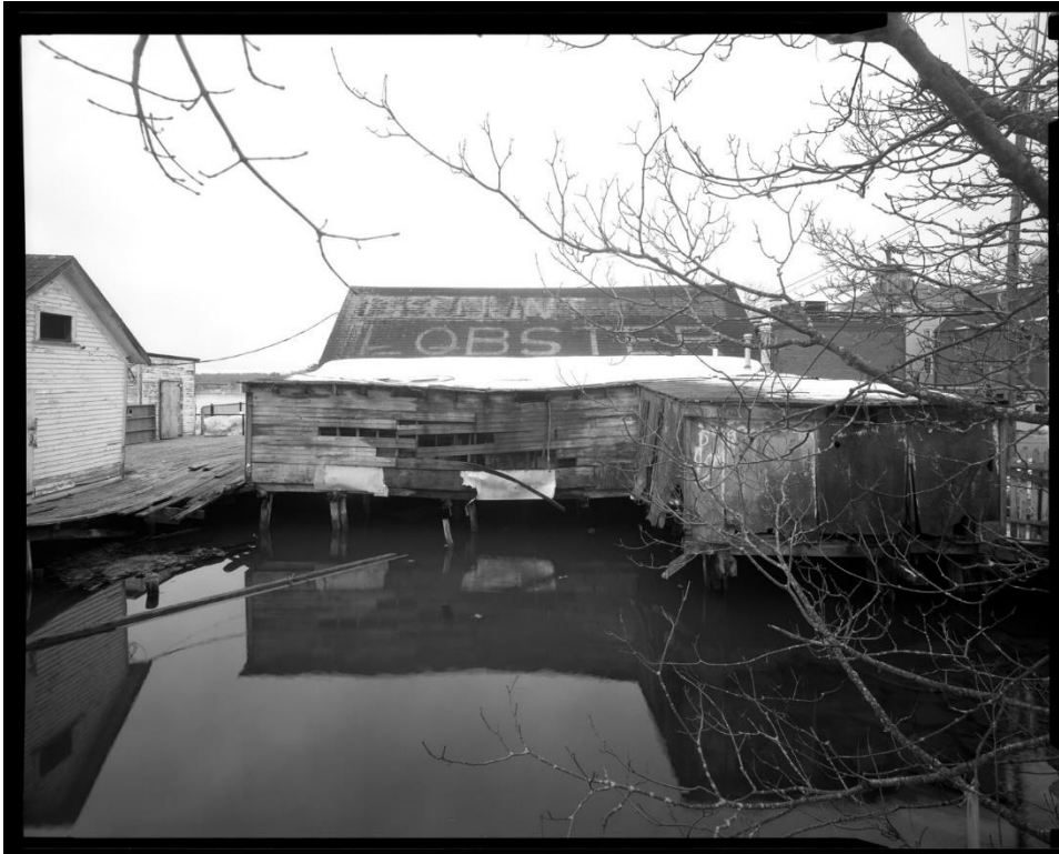
NH-566-5: North elevation of Market, Office & Shop (A), showing shed-roof additions, Lobster Pound (A-1) and Storeroom (A-2). Looking south.
