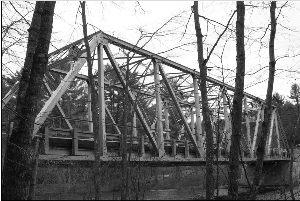
Effingham NH – Freedom ME, High Pratt Truss Bridge (176/185)
