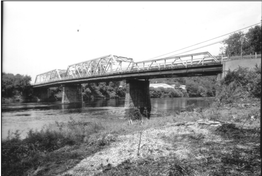
NH-665-36 Overall south elevation of bridge after removal of trees. Looking northwest.
