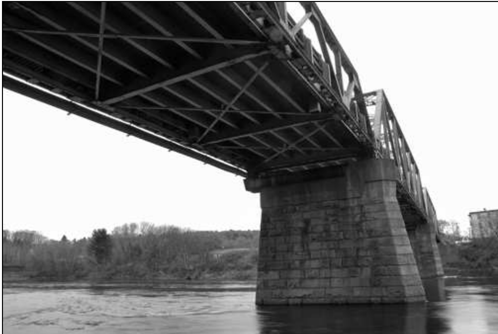
NH-665-26 East pier showing nosing profile on upstream face. Looking southwest.
