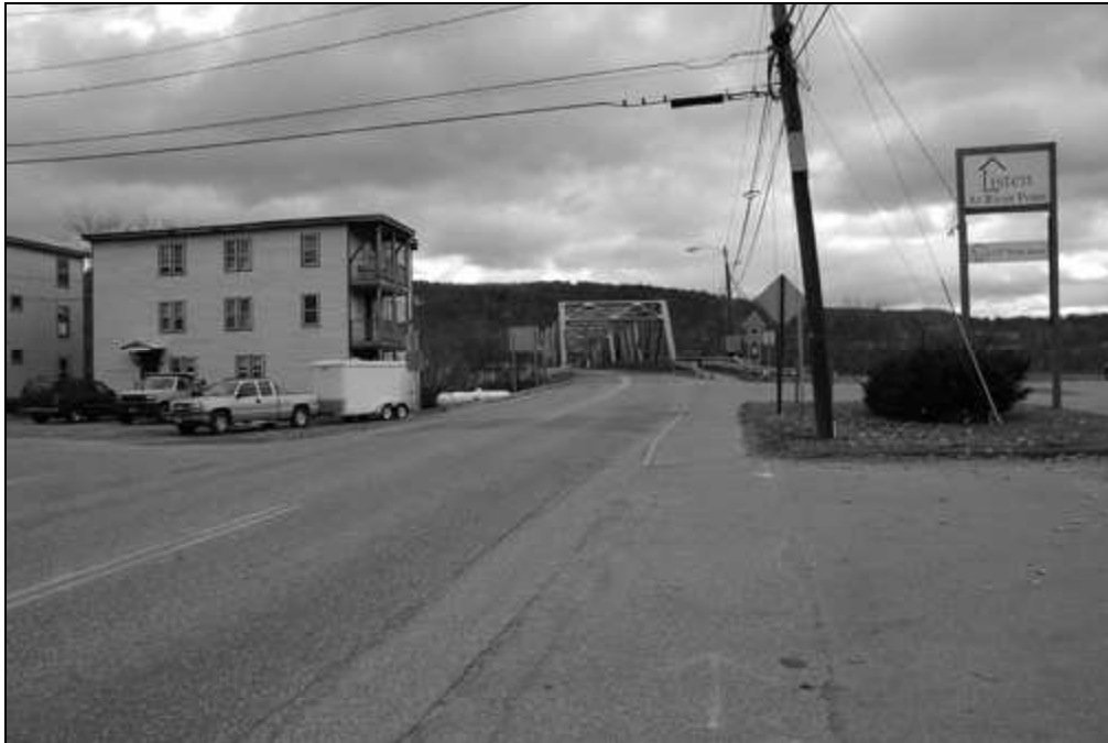
NH-665-1 West approach to bridge (Vermont end) showing portal of High Pratt Truss. Looking east southeast.
