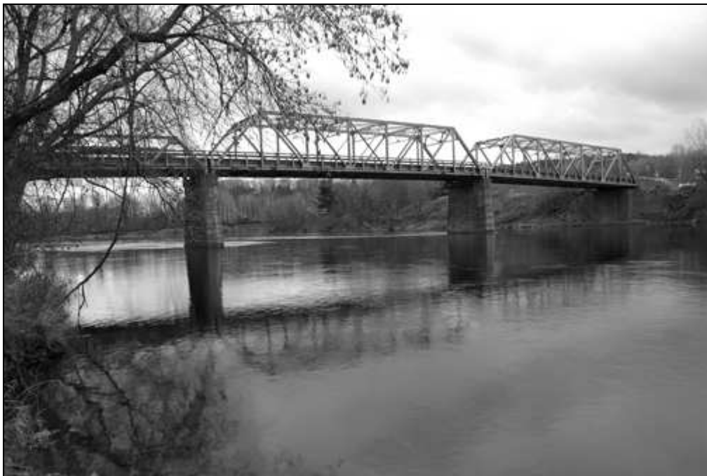
NH-665-27 Overall view of the upstream (north) side of the bridge. Looking southwest.
