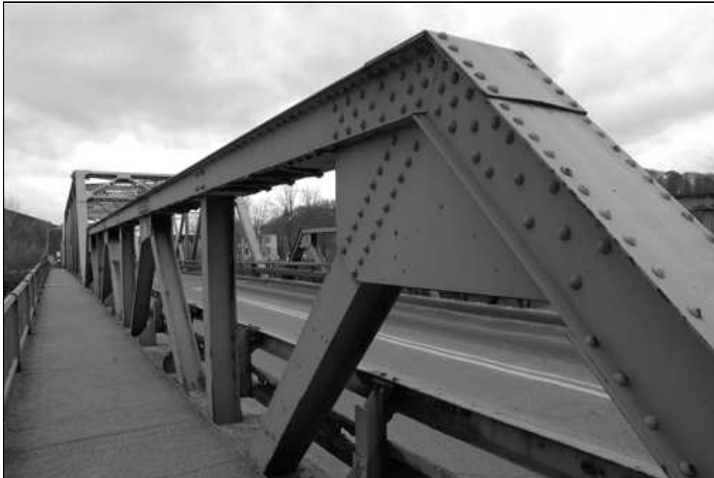
NH-665-16 Warren truss, south elevation and sidewalk. Looking west-northwest.
