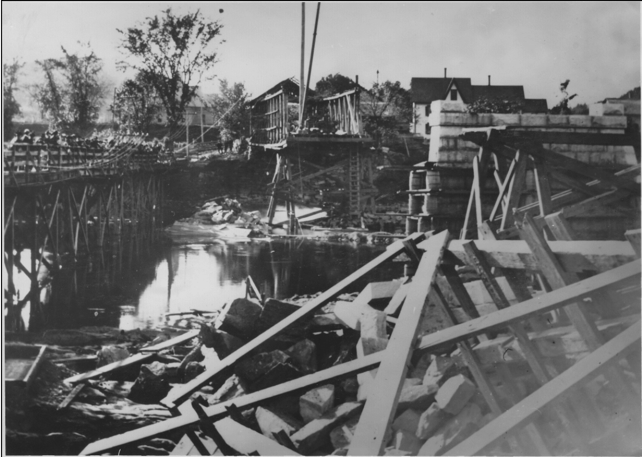
Piers for the Third Lyman's Bridge under construction in 1896, using part of the covered bridge as support for a derrick, with the temporary bridge downstream. Courtesy of Hartford [VT] Historical Society
