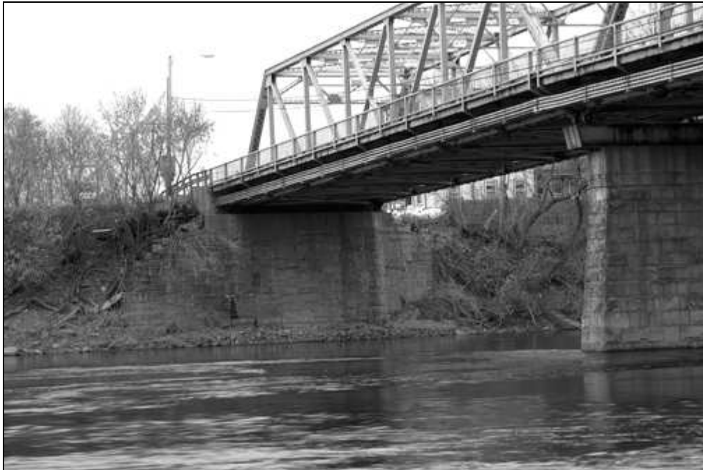
NH-665-20 West (Vermont) abutment. Looking northwest.
