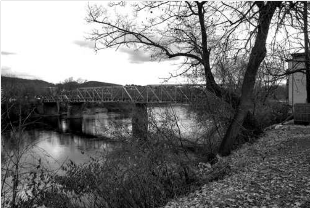
NH-665-3 View of bridge in context from upstream on Vermont side. Looking southeast.
