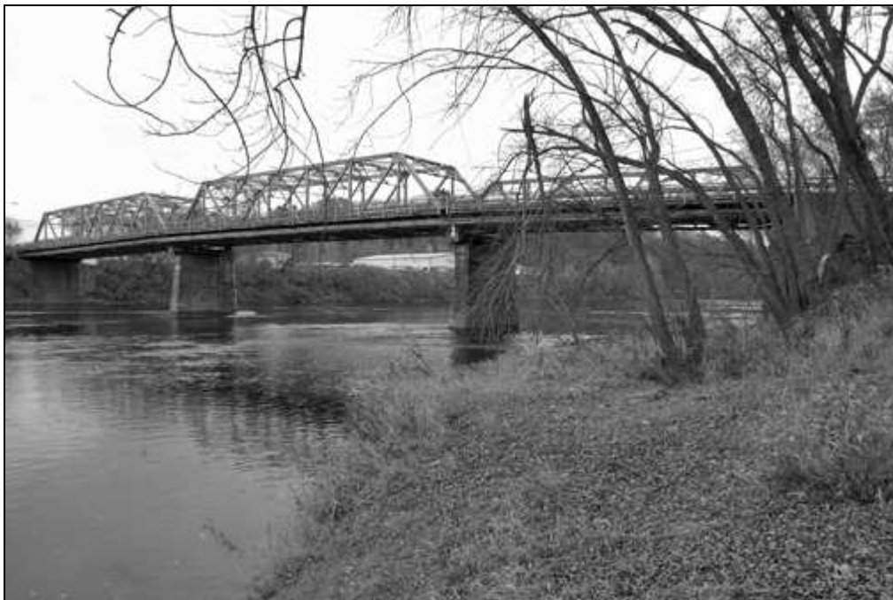
NH-665-19 Overall view of downstream (south) side of the bridge from New Hampshire side. Looking northwest.
