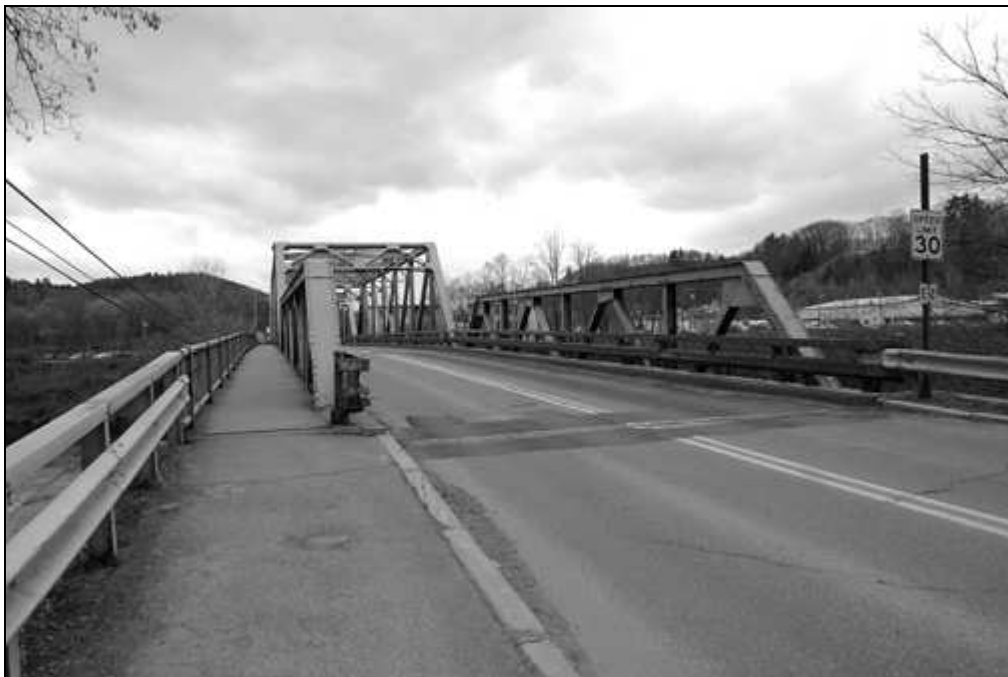
NH-665-15 East approach and Low Warren Truss span. Looking northwest.
