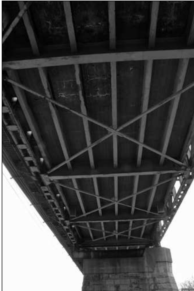
NH-665-25 Detail of floor system under the Warren Truss. Looking west.
