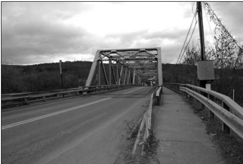
NH-665-2 West portal of High Pratt Truss (Vermont end). Looking east northeast.
