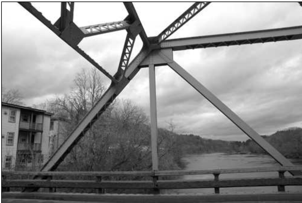
NH-665-13 View of the west portal and end post connection. Looking north.
