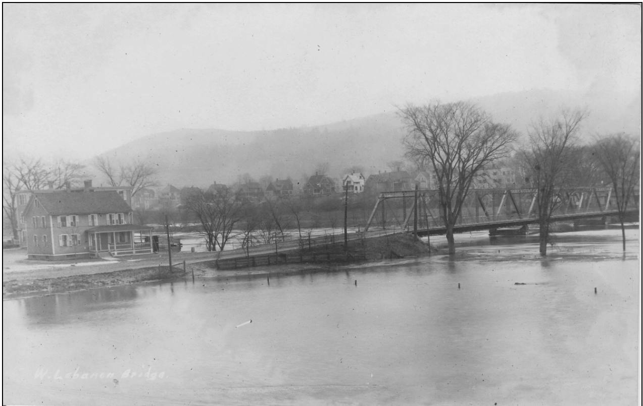
Post card view of the Third Lyman's Bridge during the flood of November 3-4, 1927.
