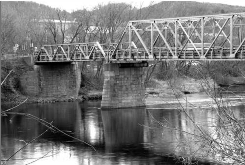
NH-665-4 View of Warren Truss (NH end), east abutment and pier. Looking southeast.
