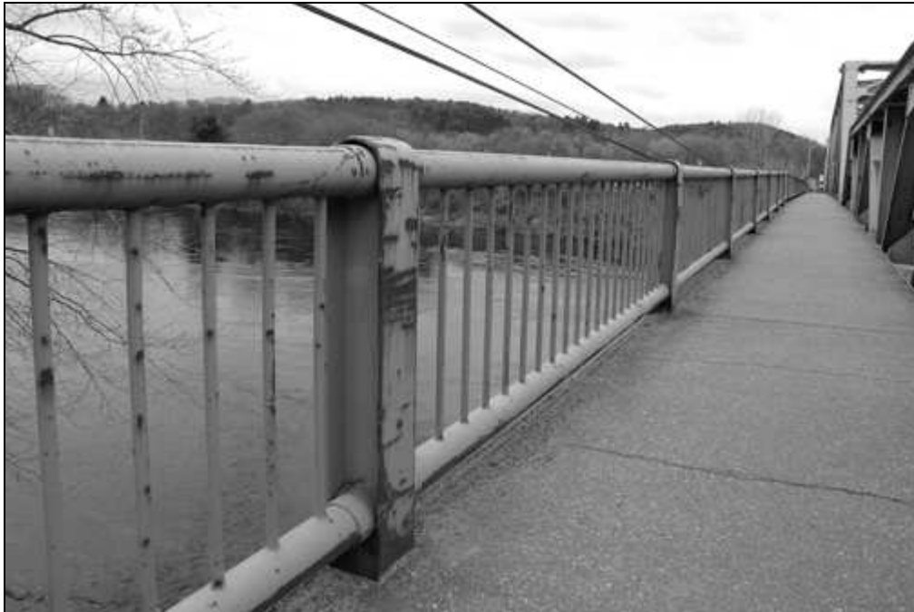
NH-665-18 Sidewalk and railing detail on downstream side. Looking west southwest.
