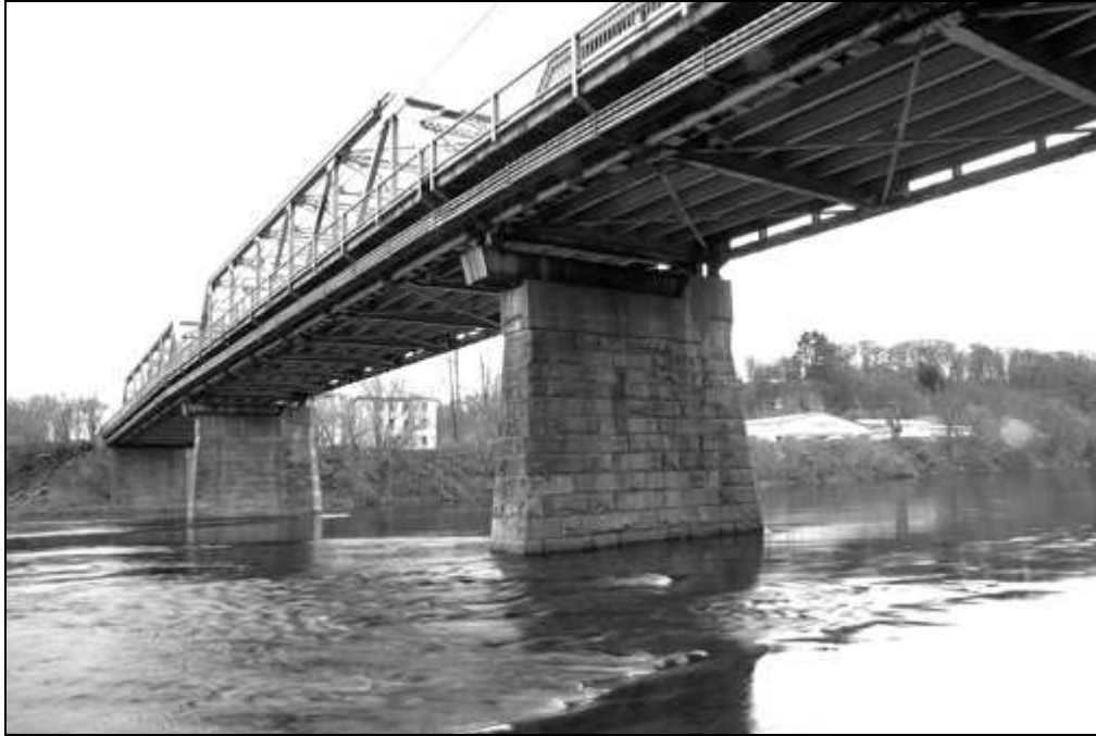
NH-665-22 Overall view of underside and floor system. Looking northwest.
