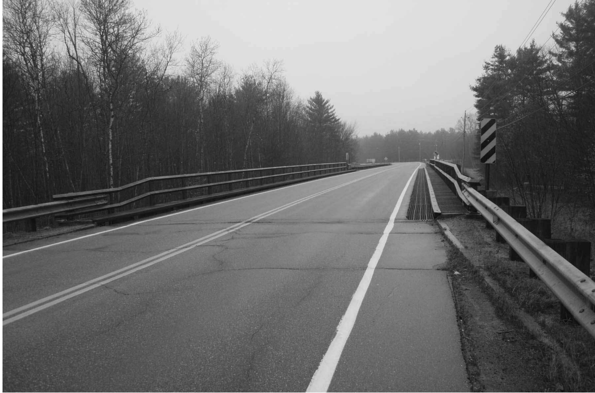
Photo # 2 description: Overall view at road level from south approach.
