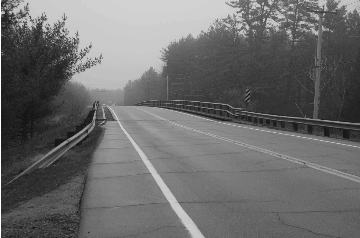
Photo # 2 description: Roadway view showing deck beam camber.
