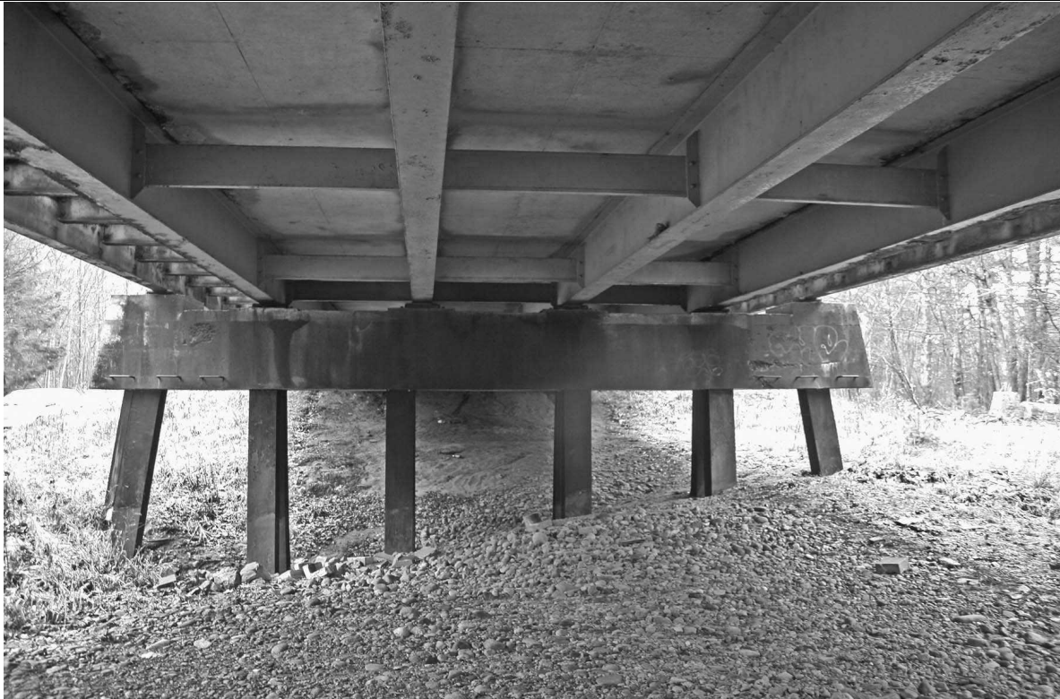
Photo # 5 description: Underside view of deck, stringers, diaphragms, H-pile bent .
