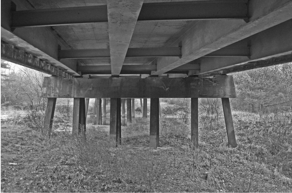
Photo # 6 description: Underside and H-pile bent.
