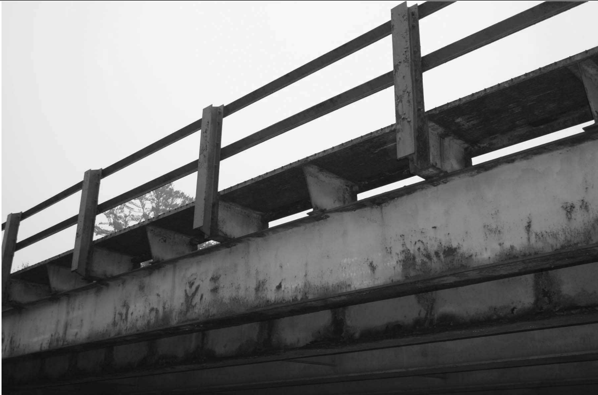
Photo # 7 description: Railing and grid sidewalk assembly.
