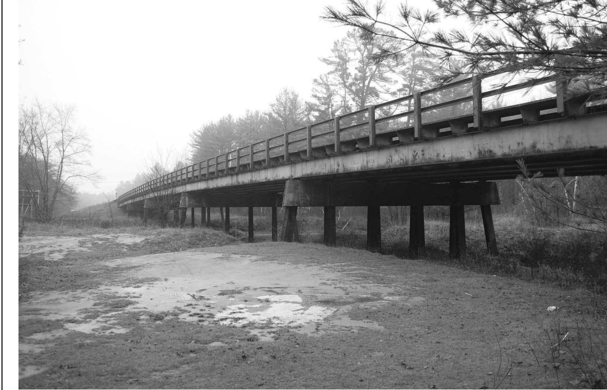
Photo # 4 description: Overall view of downstream side.
