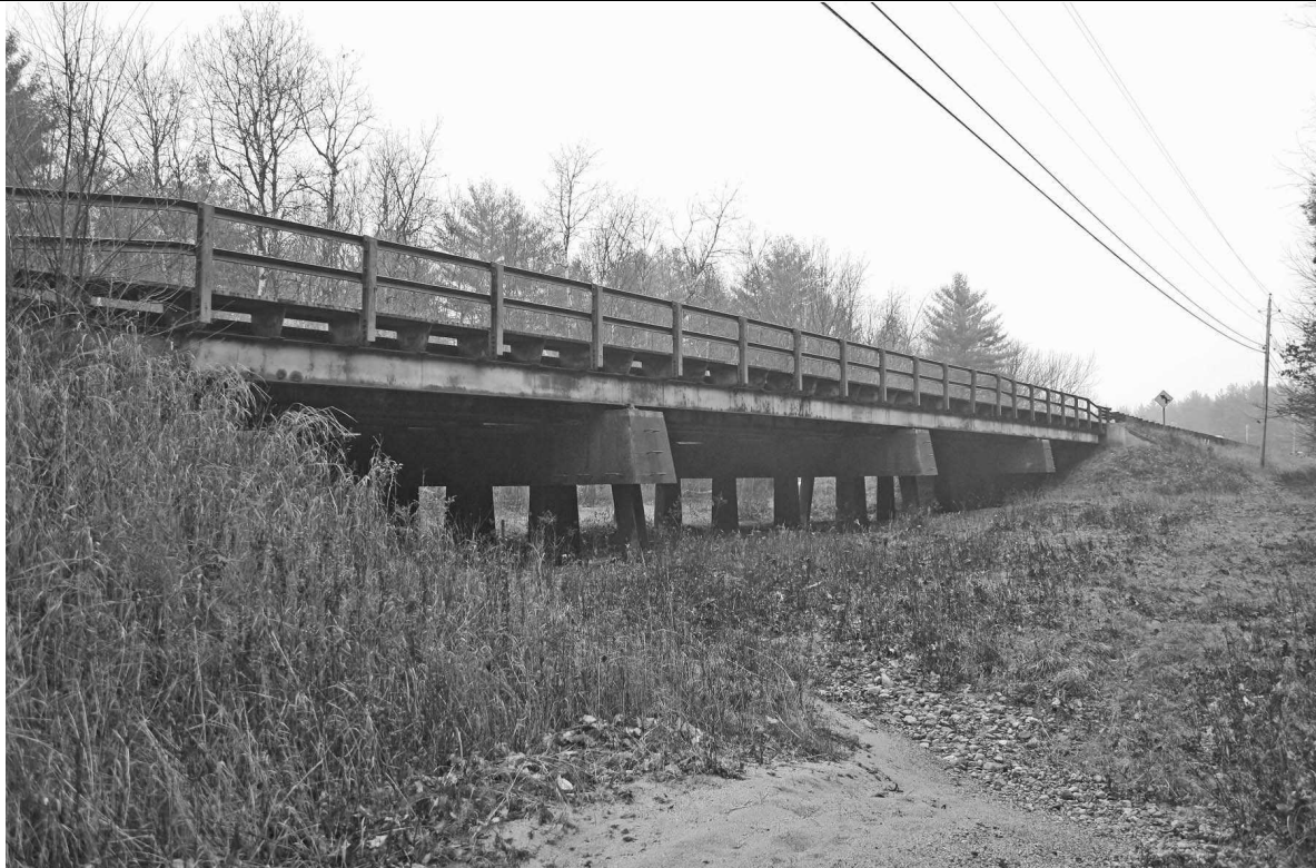
Photo # 3 description: Downstream (East) elevation.
