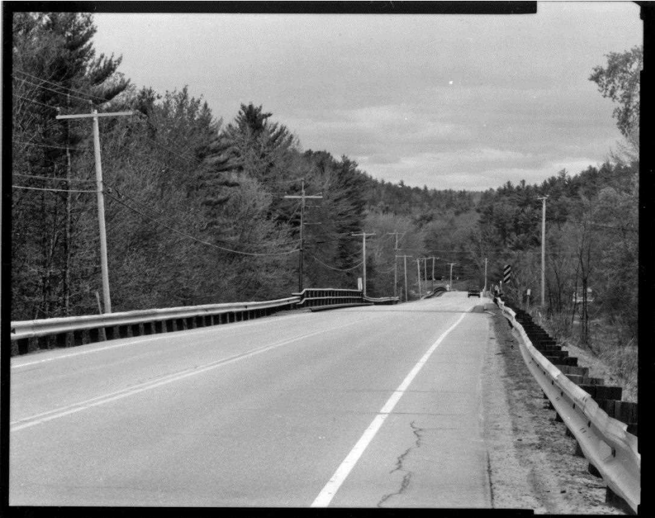
NH-744-12: Bearcamp River Relief Bridge, north approach with Bearcamp River Bridge visible in distance. Looking southwest.
