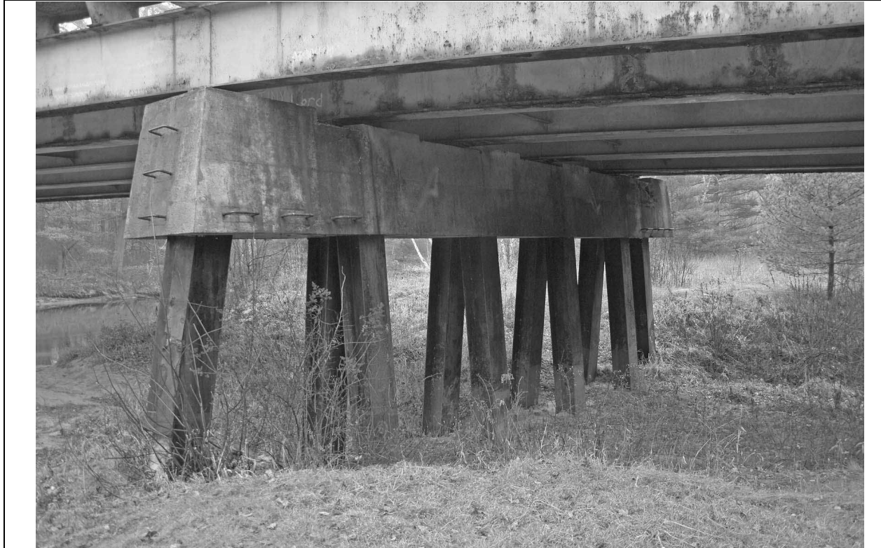
Photo # 9 description: H-pile bent showing double battered A-frame type piles.
