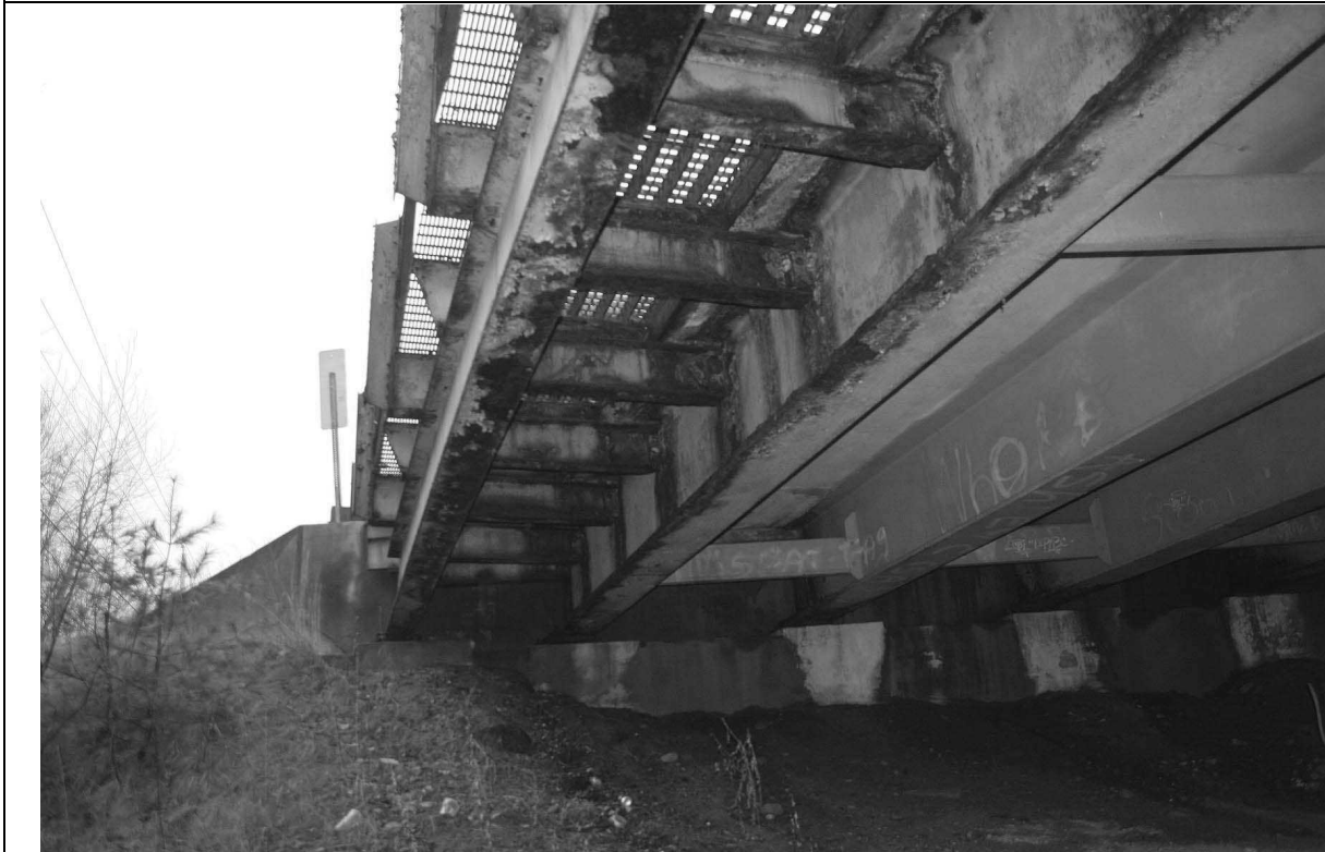
Photo # 5 description: Concrete abutment and underside of steel grid shoulders.
