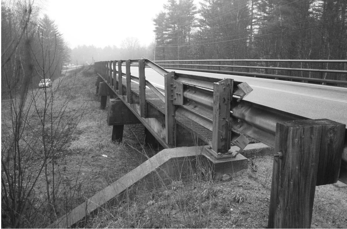
Photo # 4 description: Top of abutment, railing and bents.
