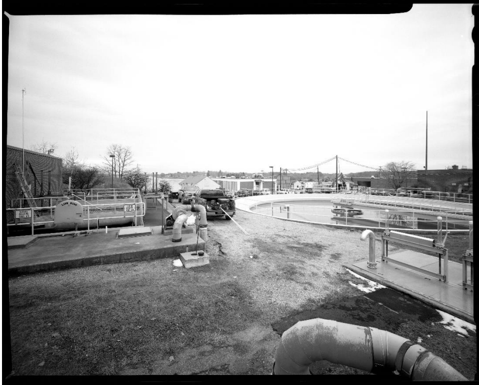
NH-743-1: Context view, looking past Grit Chambers (left) and Clarifier No. 2 (right), showing front of Sludge Processing Building in distance (center). Looking southeast.
