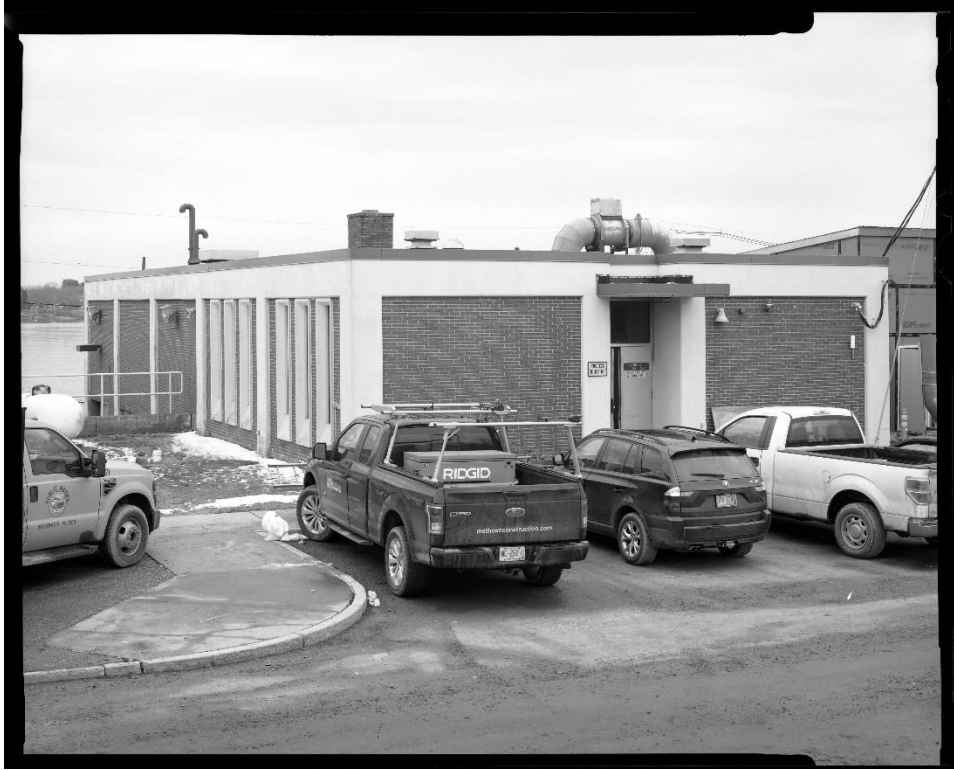
NH-743-2: Oblique view of front and north side of Sludge Processing Building. Looking southeast.
