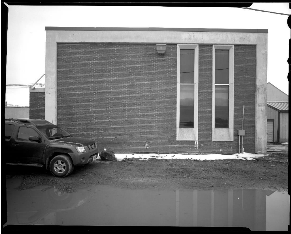
NH-743-5: Rear elevation of Sludge Processing Building. Looking west.
