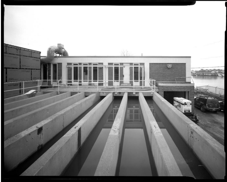
NH-743-4: South side of Sludge Processing Building, rear section, showing Chlorine Contact Tanks in foreground. Looking north.
