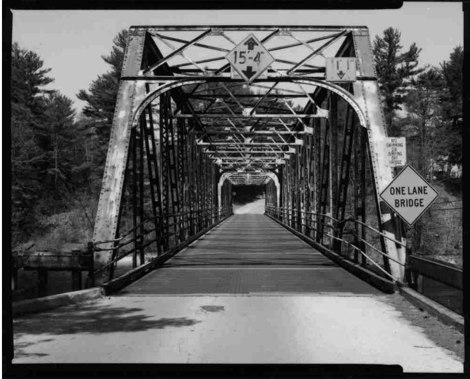
NH-727-13 South portal. Looking north.
