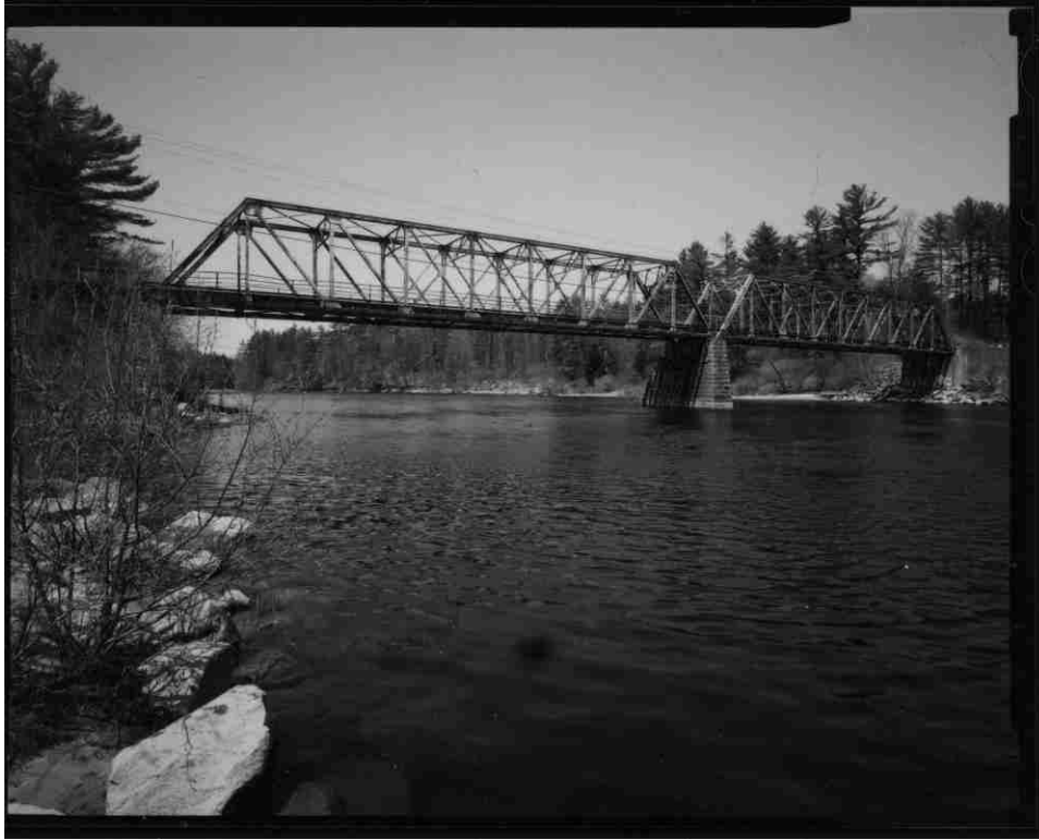
NH-727-3 Downstream (east elevation), oblique view. Looking northwest.
