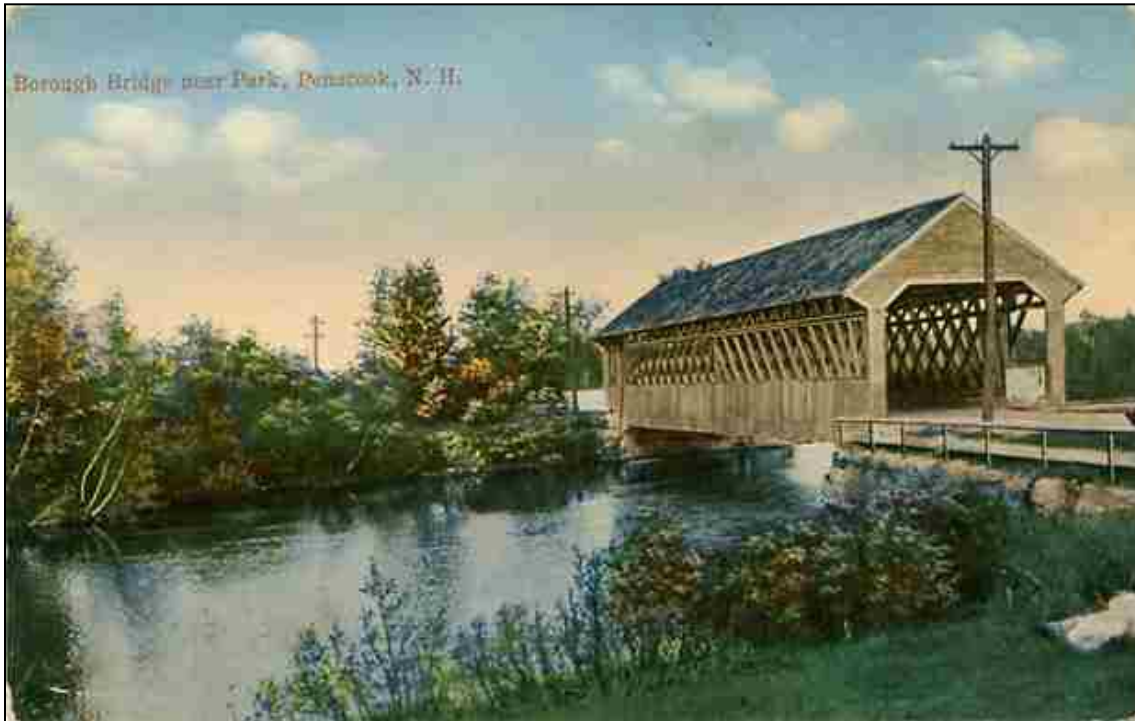
FIGURE 34: Borough Bridge over Contoocook River canal near Holden's Mill, Penacook. Date of original bridge unknown; substantially rebuilt in 1892 as shown in postcard, circa 1910. Replaced by steel truss bridge in 1915 (Penacook Village Association).
