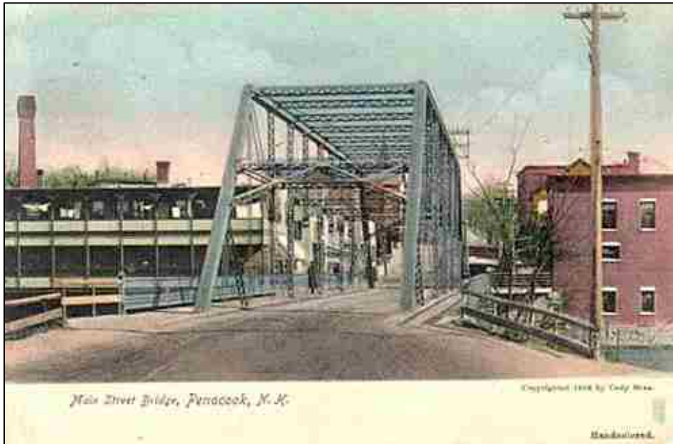
FIGURE 41: Main Street Bridge Penacook, north approach, looking south. Pratt truss built 1898 by Wrought Iron Bridge Company, Canton, Ohio, replaced 1915. Postcard dated 1906 (Penacook Village Association).
