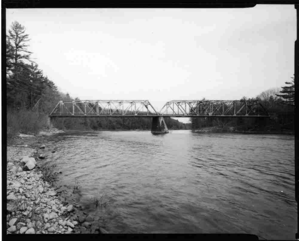
NH-727-2 Upstream side (west elevation) of north span. Looking east.
