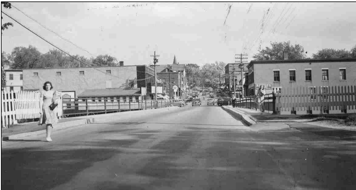
FIGURE 47: Main Street Bridge Penacook, built 1915. North approach, photo dated June 12, 1940 (NHDOT bridge card Concord 040/090).
