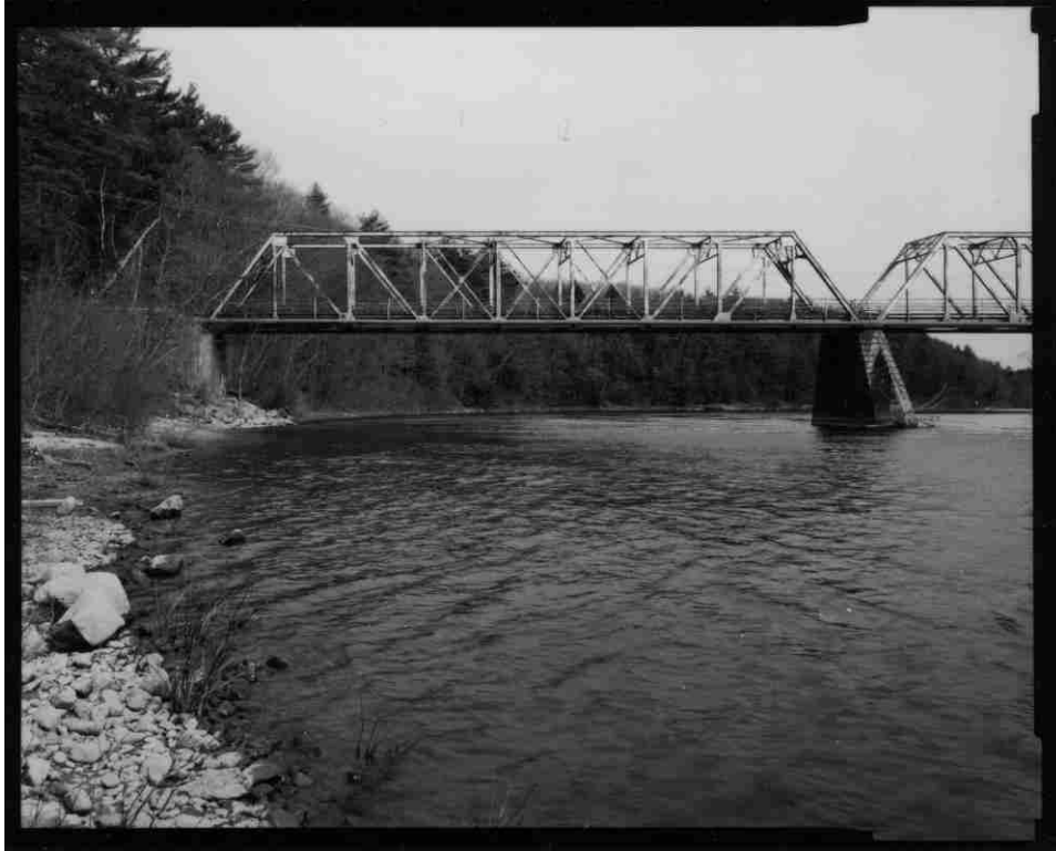
NH-727-4 West elevation of north span. Looking east.
