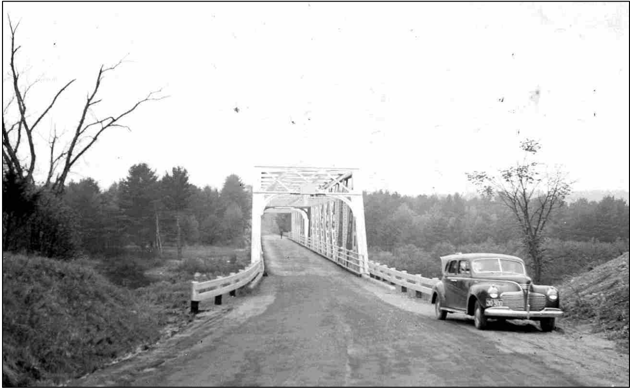
FIGURE 10: Sewall's Falls Bridge, north approach. Field inspection photo made by NHHD engineer Wendell H. Piper, May 15, 1942 (NHHD Bridge Inventory Card, Concord 070/117).
