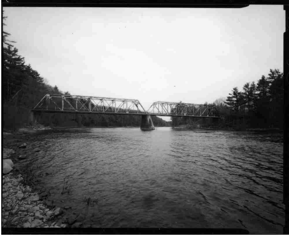
NH-727-1 Context view from upstream of bridge. Looking southeast.
