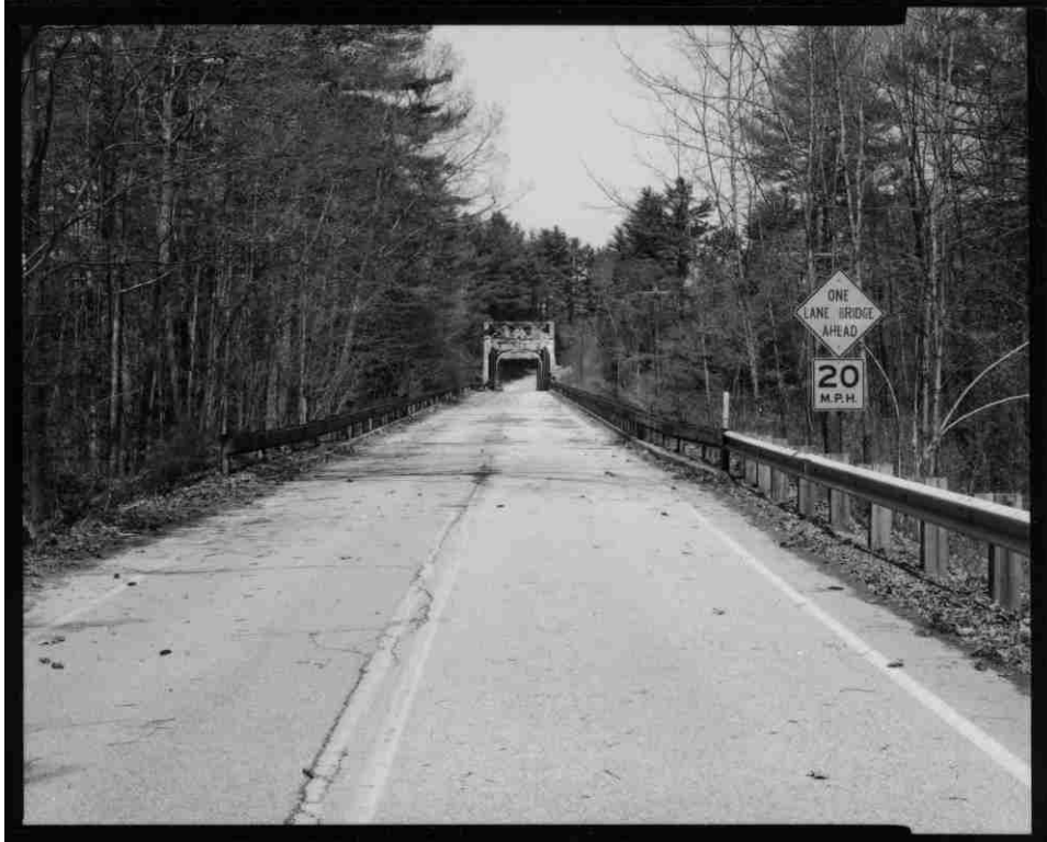
NH-727-5 South approach roadway, deck spans and context. Looking north.
