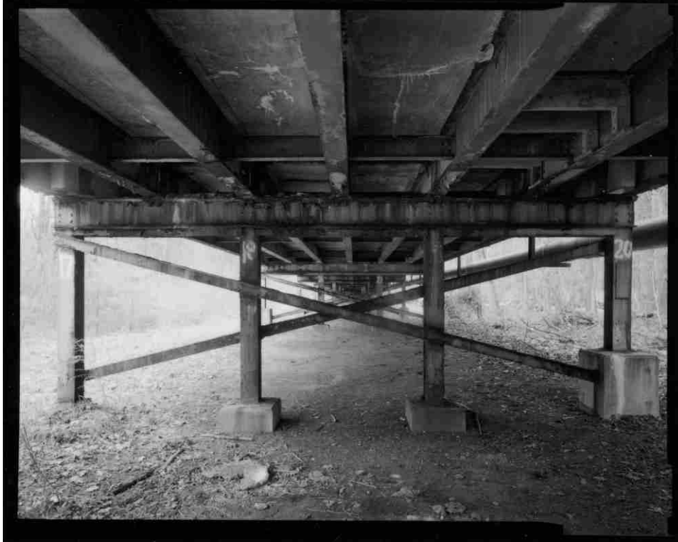
NH-727-20 Underside of approach spans and detail of bent. Looking south.
