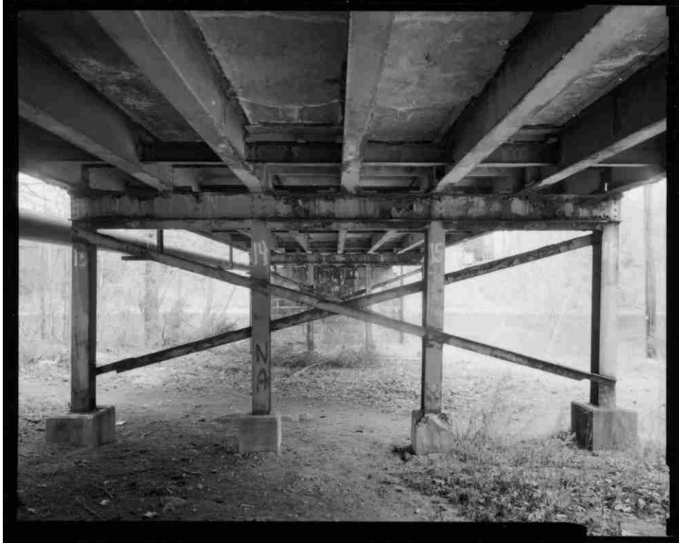
NH-727-21 Underside of approach spans and detail of bent. Looking north.
