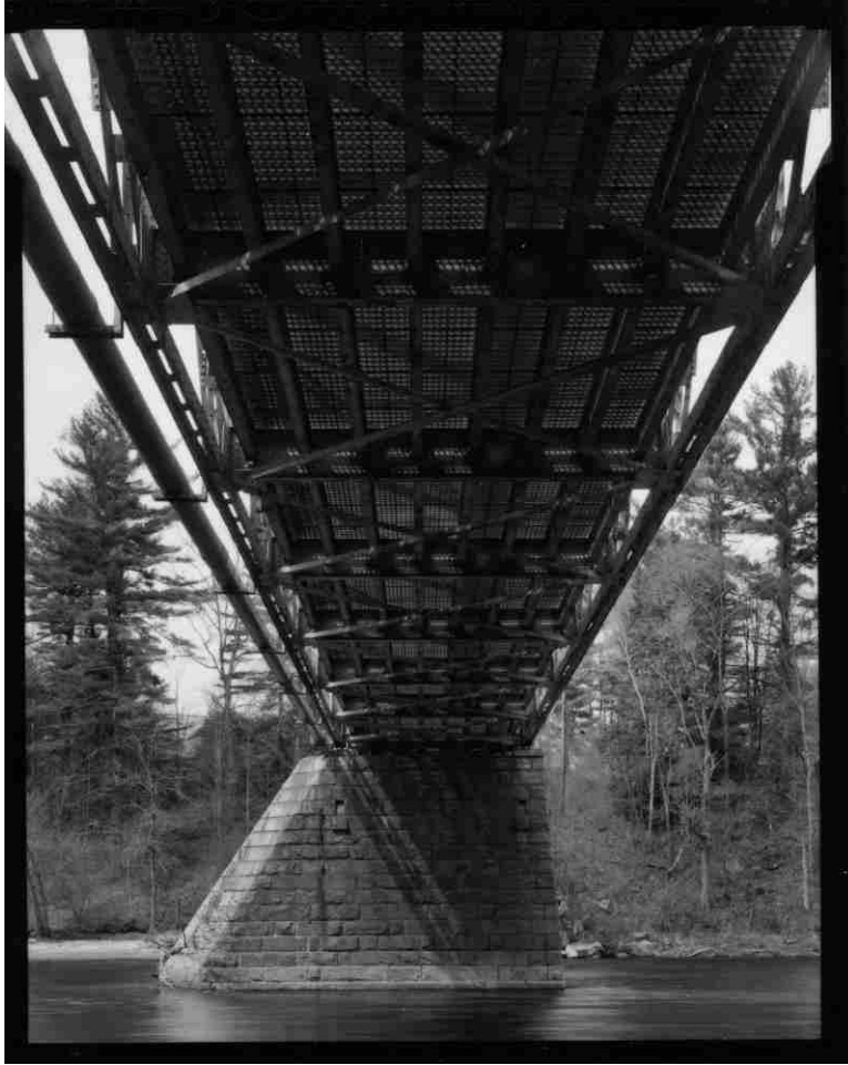
NH-727-17 Underside of south truss, showing floor system. Looking north.
