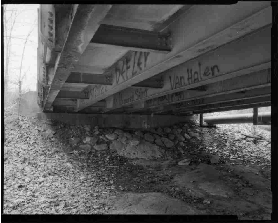
NH-727-10 South abutment carrying first deck approach span. Looking southwest.
