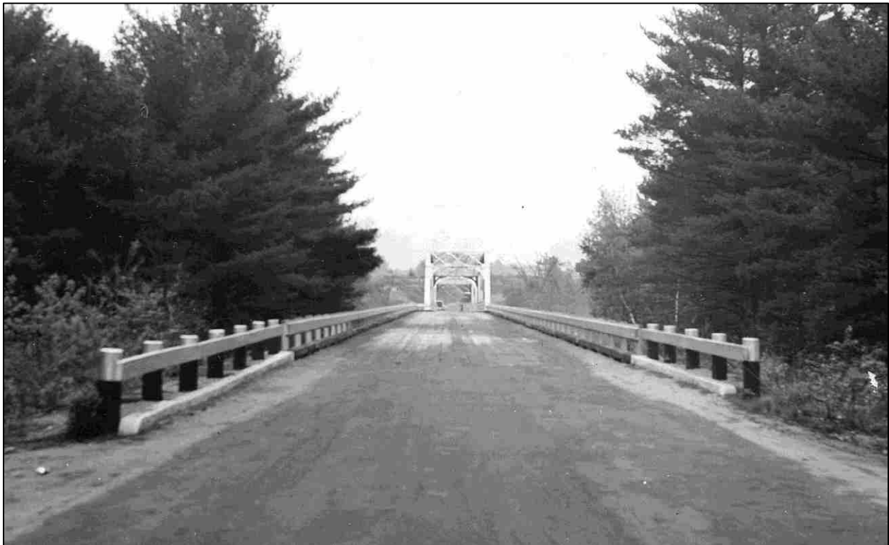
FIGURE 11: Sewall's Falls Bridge, south approach. Field inspection photo made by NHHD engineer Wendell H. Piper, May 15, 1942 (NHHD Bridge Inventory Card, Concord 070/117).
