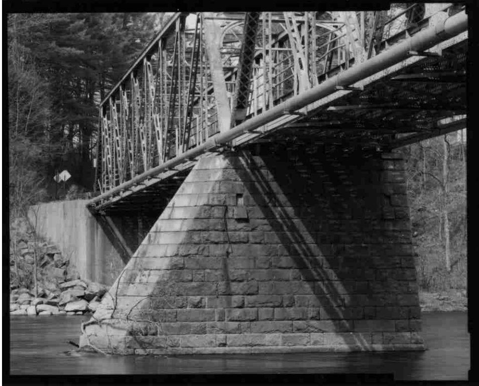
NH-727-11 Center pier detail, south side. Looking northeast.
