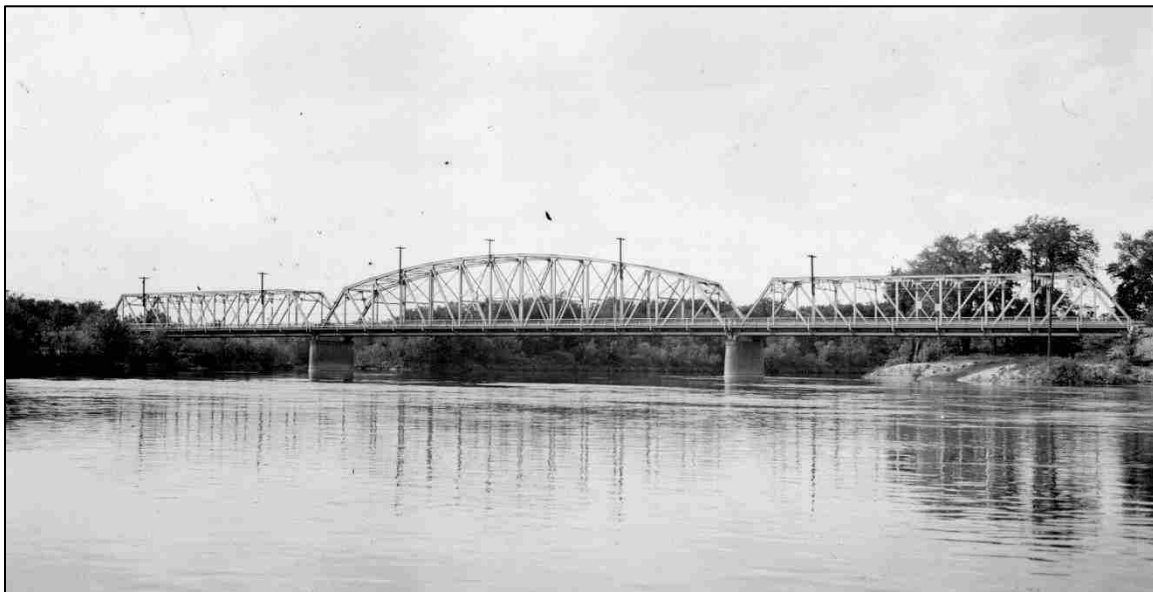
FIGURE 33: South End Bridge built 1933; photo dated 1940 replaced 1915 Pembroke Bridge. The South End Bridge (Concord 186/103) was replaced in 1998 with the present 5-span I-beam stringer bridge Concord 185/104, since named the Korean Veterans Memorial Bridge (NHDOT bridge card Concord 186/103).
