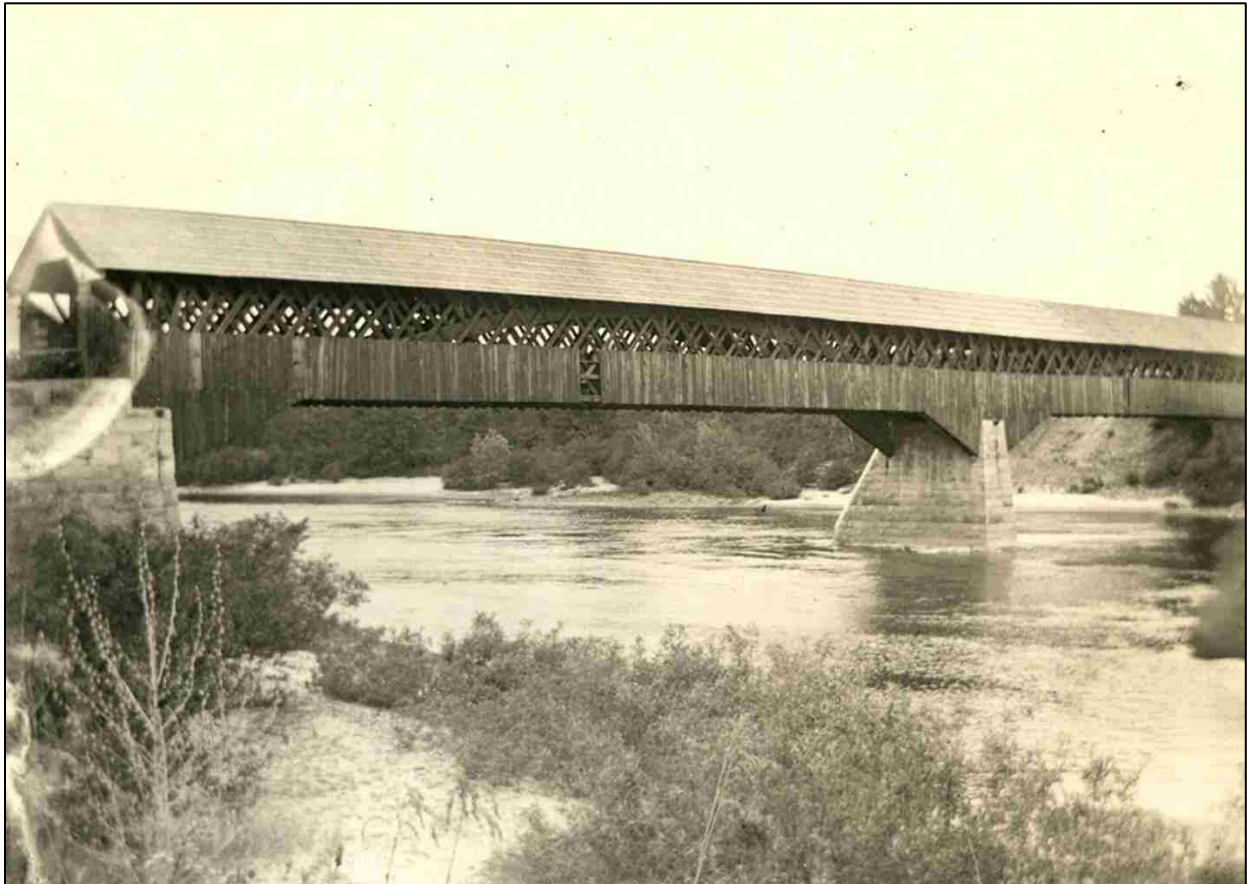
FIGURE 27: Sewall's Falls Bridge, built 1873. Substructure by Lyman R. Fellows; Superstructure by Dutton Woods (Courtesy of National Society for the Preservation of Covered Bridges).
