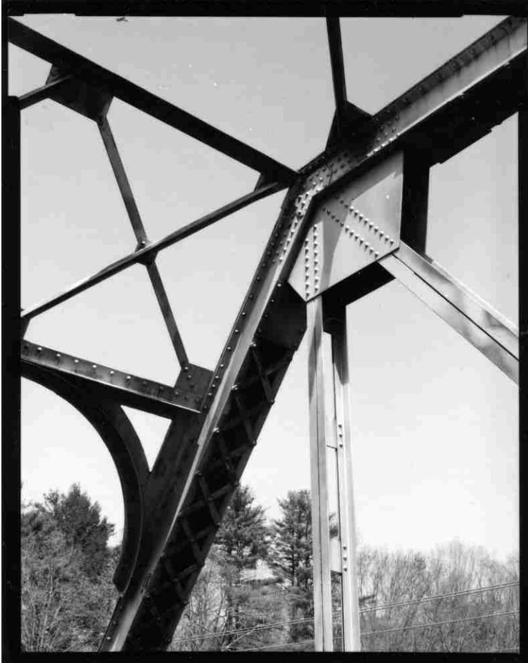
NH-727-22 Detail of upper chord and endpost connection. Looking northeast.
