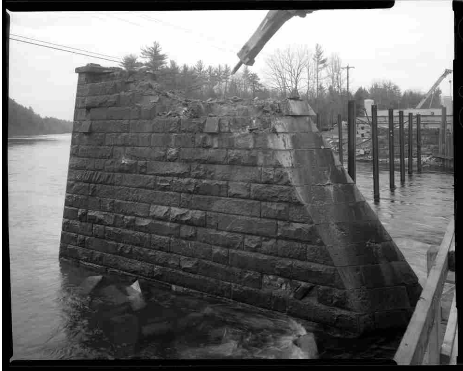
NH-727-30 Center pier, north elevation, showing demolition, 23 March 2016. Looking northeast.
