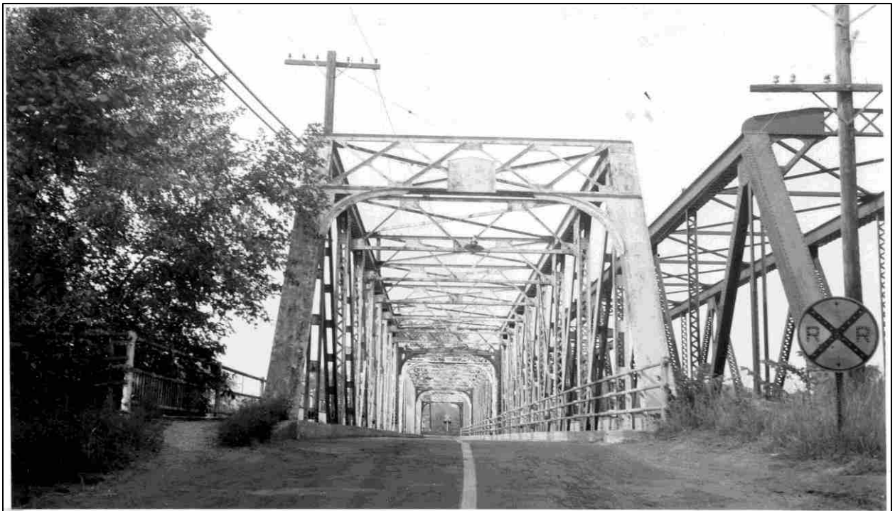
FIGURE 38: Federal Bridge, built 1915, showing south approach and portal. Photo c. 1940. Boston & Maine Railroad Railroad Bridge at right (NHDOT bridge card Concord 136/115, no date, c. 1940).
