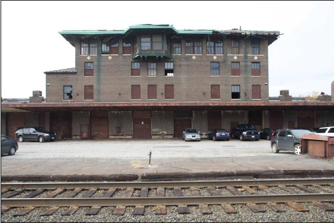
-019 Signal Tower, south elevation. Looking northwest.
