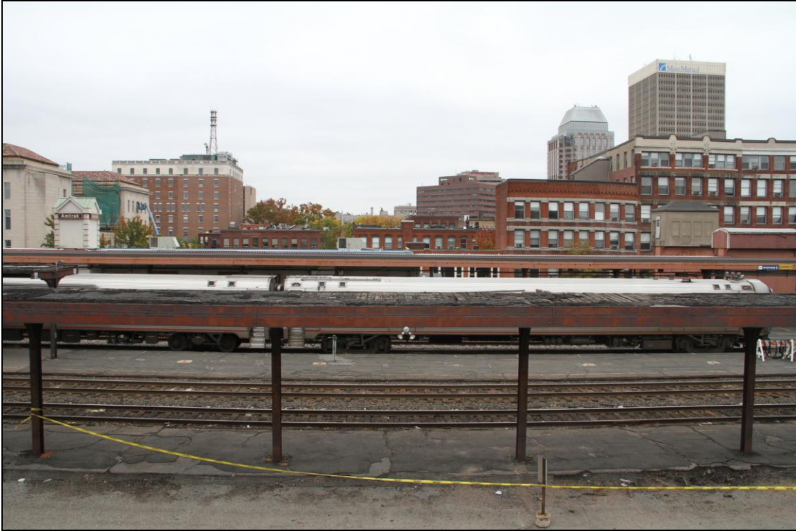
-035 Context, from roof, across tracks and platforms. Looking southeast.
