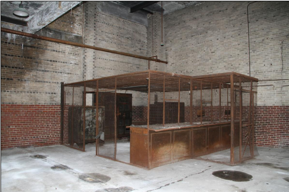
-058 Interior, second floor, Railway Express office showing wire-enclosed safe room. Looking west.
