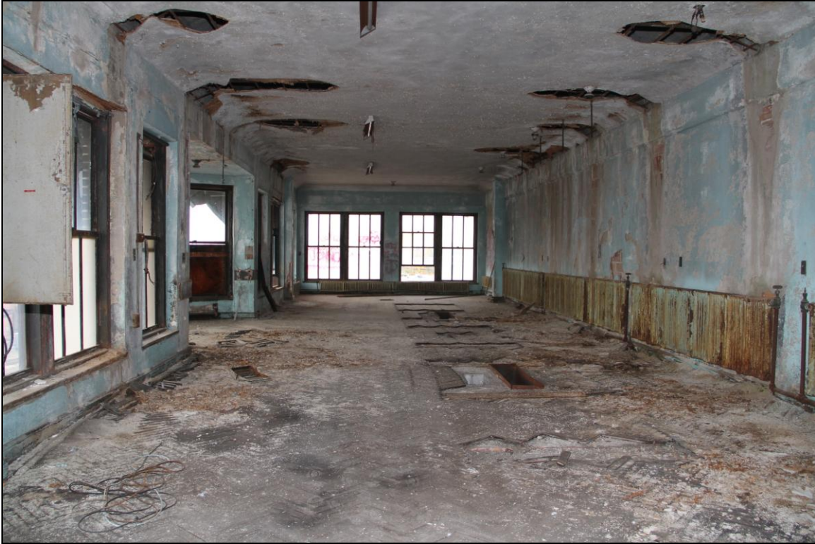
-080 Interior, Signal Tower, level 3, main control room, overall view. Looking southwest.
