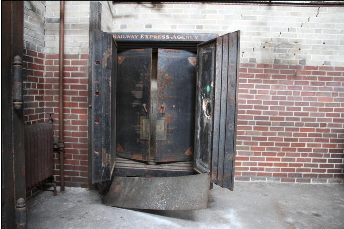
-061 Interior, second floor, Railway Express office, detail of safe. Looking northwest.
