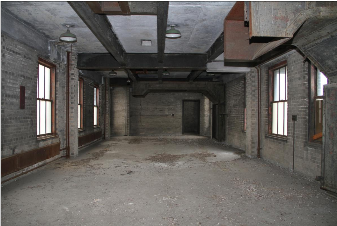
-073 Interior, Signal Tower, level 1, room. Looking southwest.
