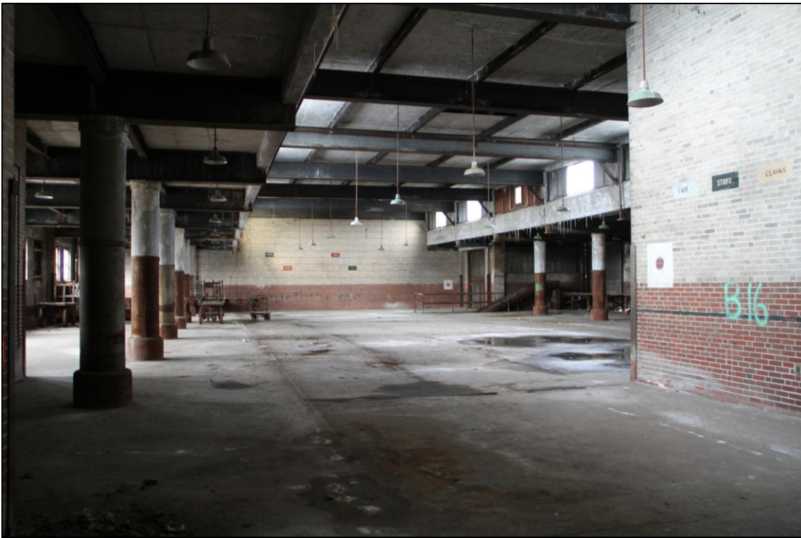
-052 Interior, second floor, west baggage room, overall view. Looking northeast.
