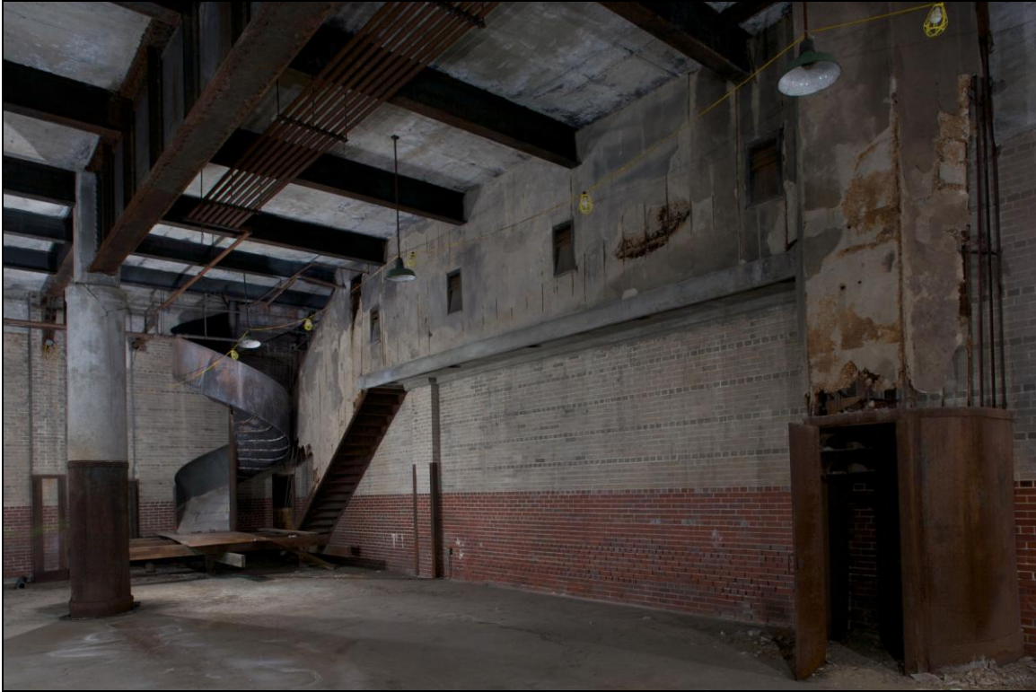
-047 Interior, first floor, east freight room, showing spiral chute and overhead observation tunnel. Looking south.
