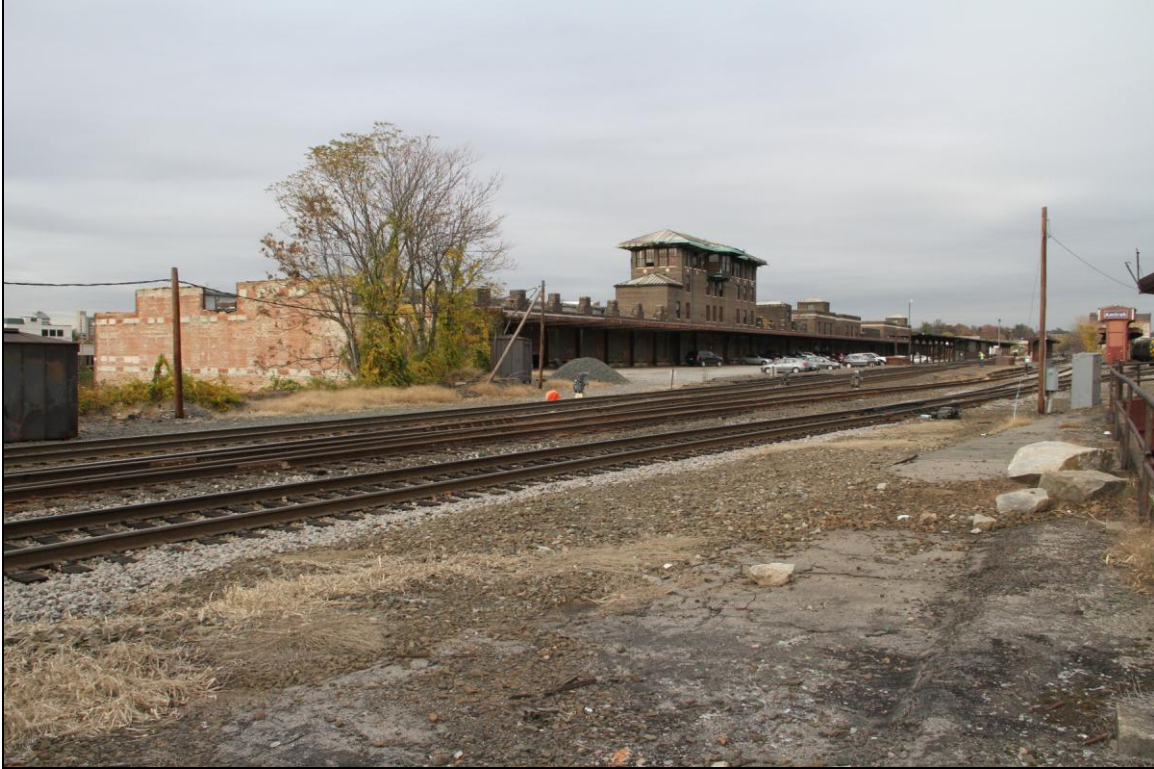
-017 Context from track level, west end of station yard, showing overall view of trackside (south) elevation of Baggage Building and Passenger Station. Looking north.
