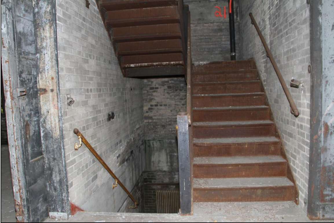
-072 Interior, Signal Tower, level 1, stairway. Looking northwest.
