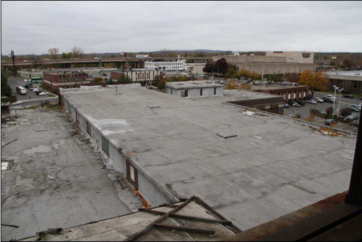
-039 Context, from roof, to Main Street, showing existing bus station. Looking west.
