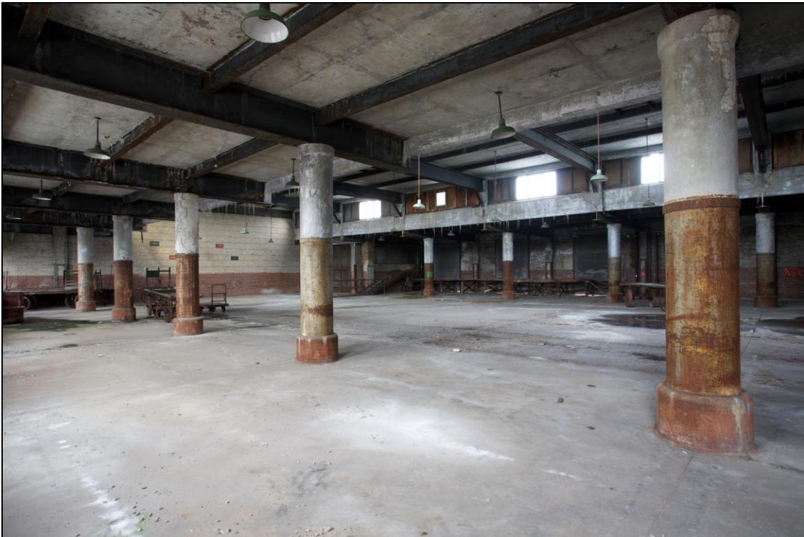
-054 Interior, second floor, west baggage room, overall view. Looking east.
