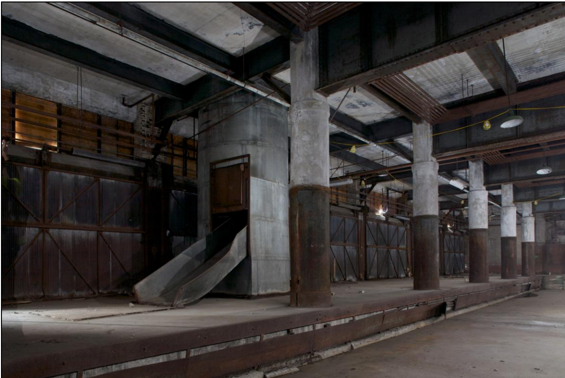
-046 Interior, first floor, east freight room, showing loading dock, doors and luggage/parcel chute. Looking northeast.
