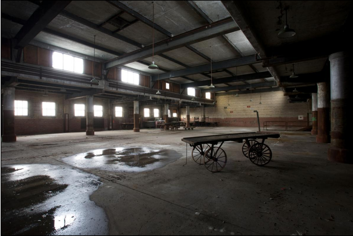
-057 Interior, second floor, west baggage room, overview, showing baggage cart. Looking north.
