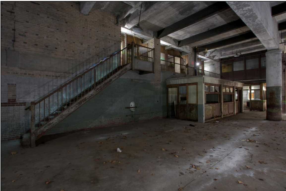
-044 Interior, first floor, west freight room, showing office areas. Looking west.
