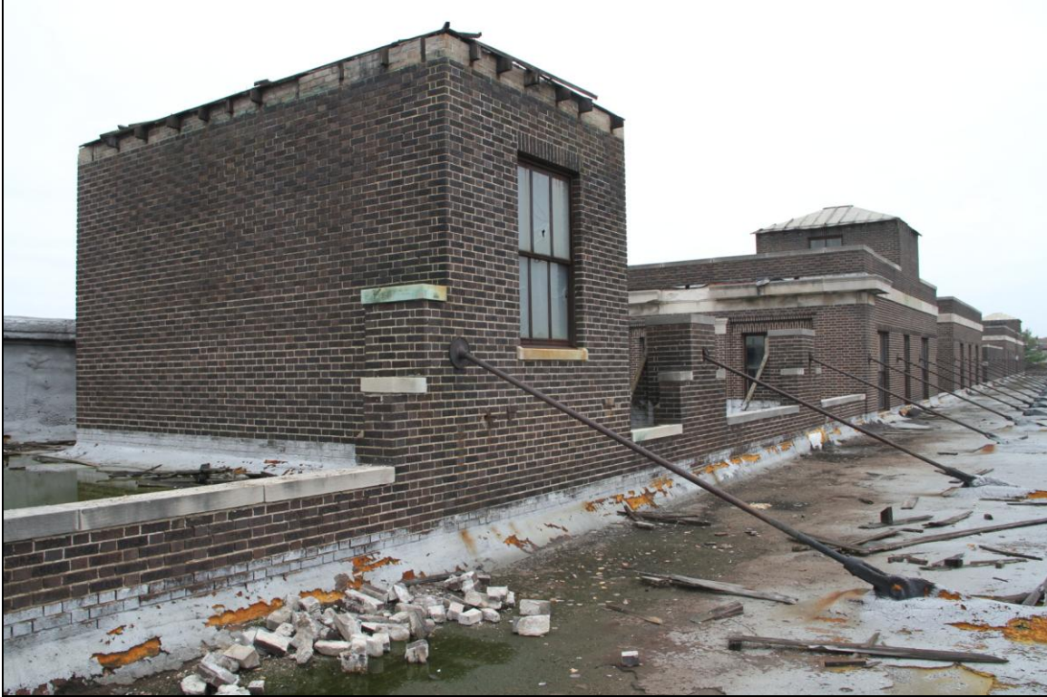
-029 Detail of canopy tie-rods and elevator tower. Looking northeast.
