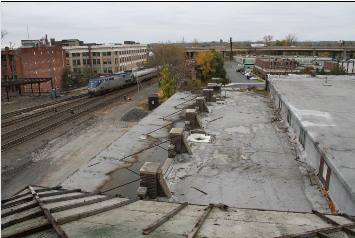
-038 Context, from roof, showing Route 91 in distance. Looking southwest.
