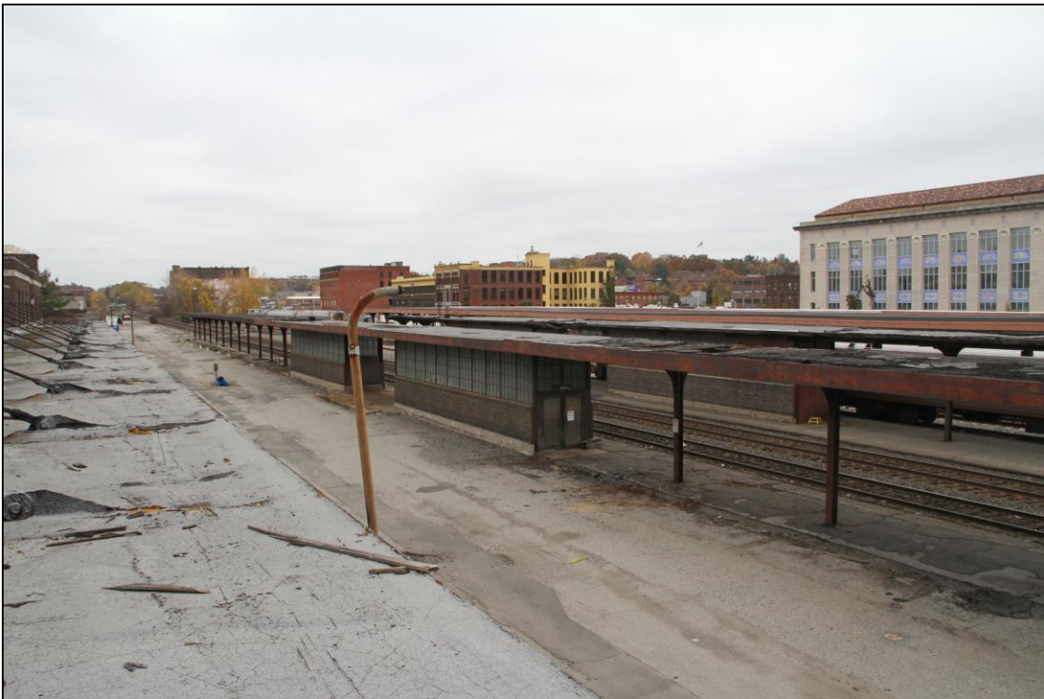
-034 Context, from roof, across tracks and platforms. Looking east.
