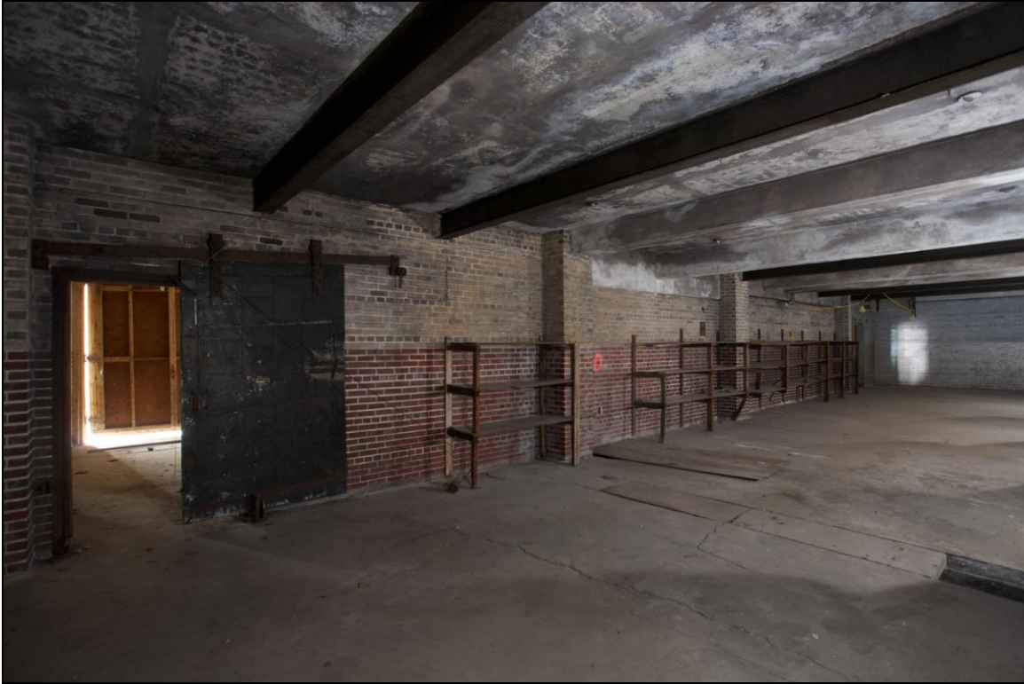
-043 Interior, first floor, storeroom. Looking east.
