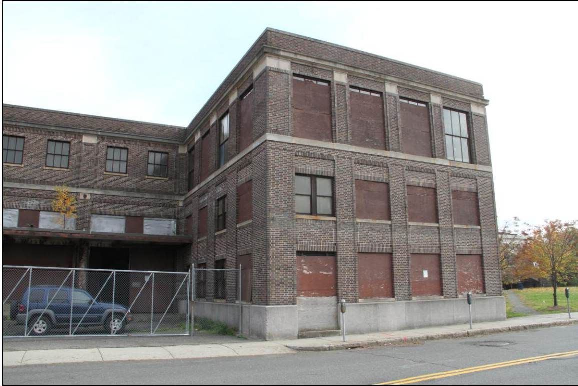
-013 Front of office wing. Looking south.
