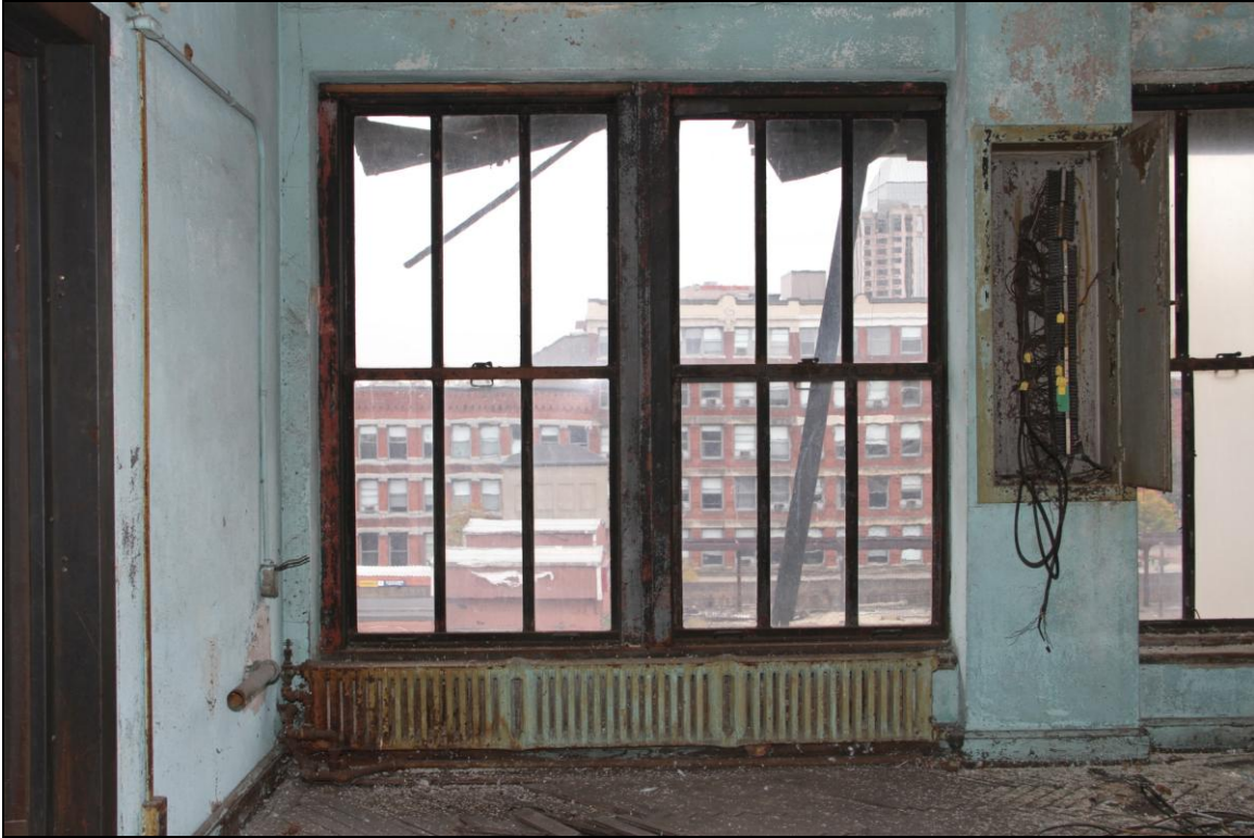
-082 Interior, Signal Tower, level 3, main control room, window detail. Looking southwest.
