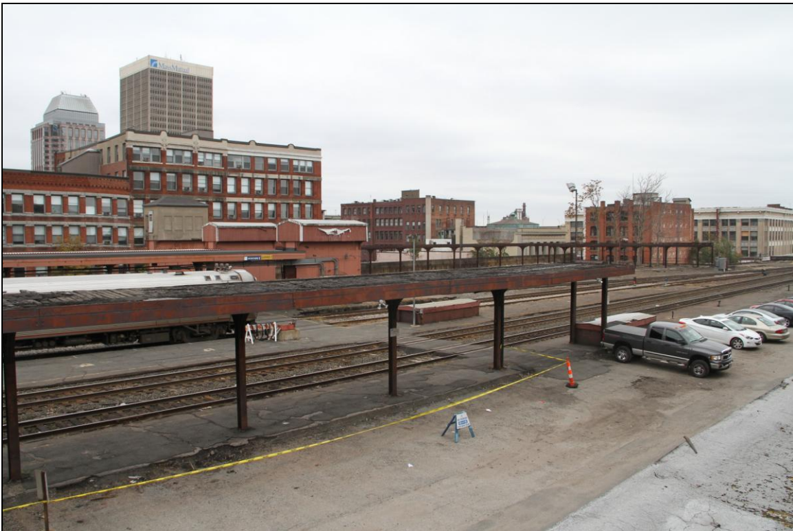
-036 Context, from roof, across tracks and platforms. Looking south.
