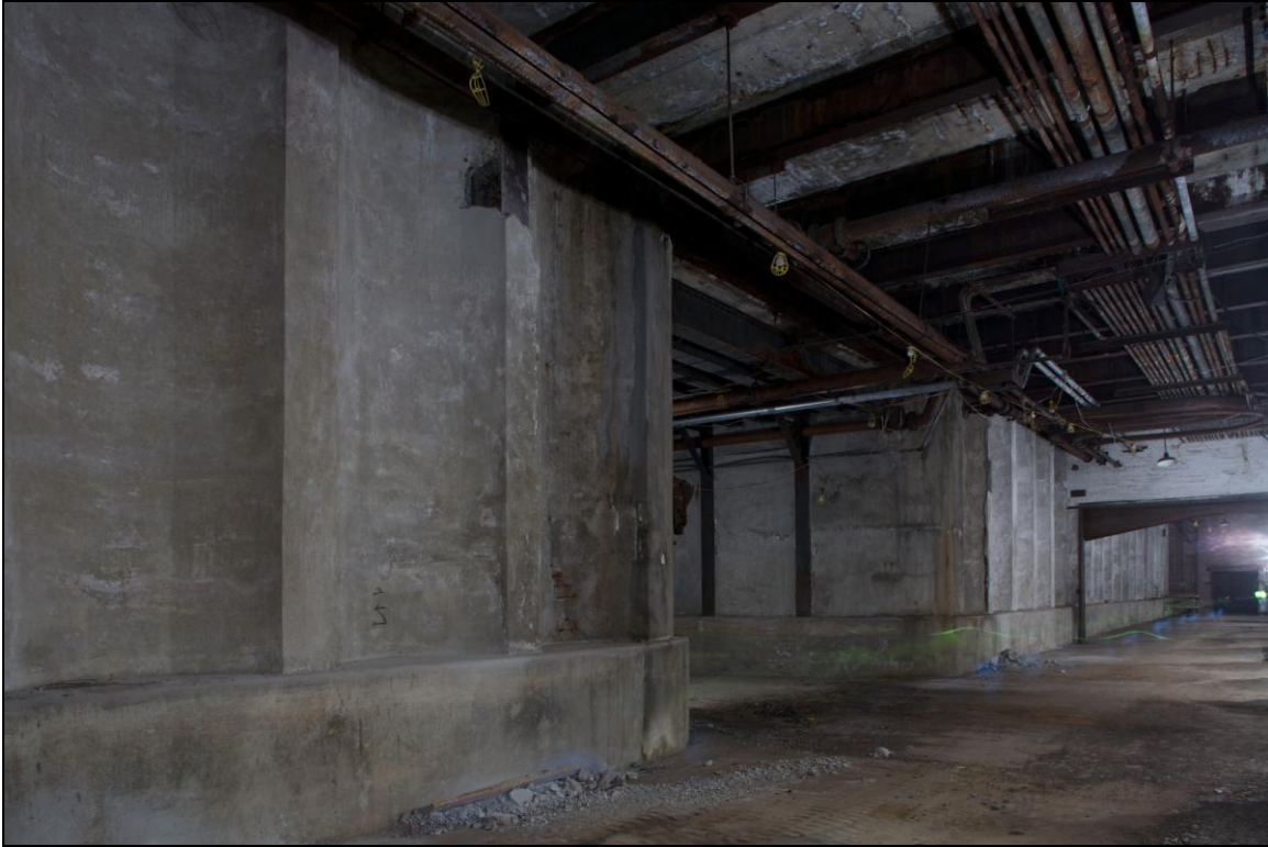
-051 Interior, first floor, back hallway. Looking southwest.
