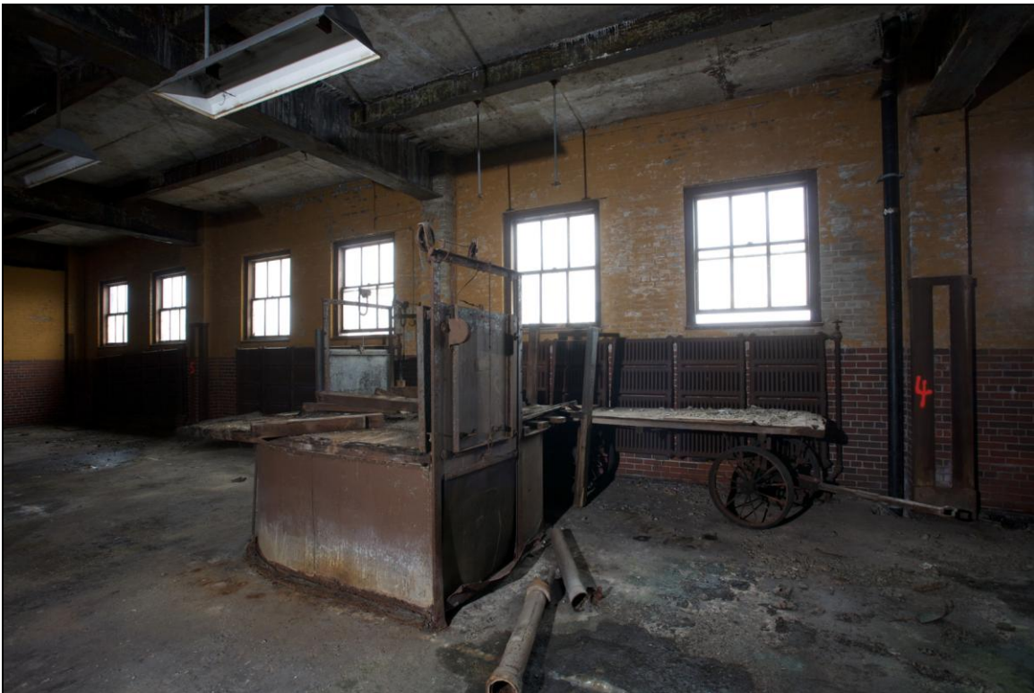
-070 Interior, second floor, east baggage room, showing spiral baggage chute, windows and heating radiators. Looking northwest.
