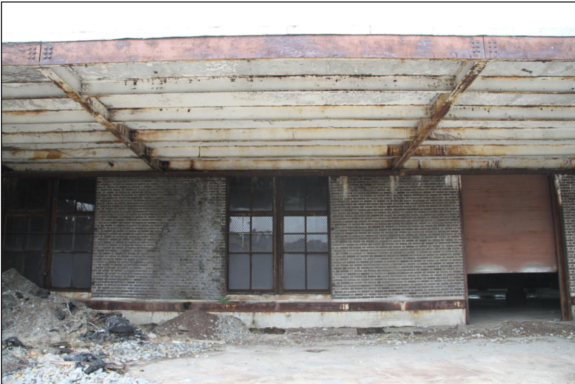
-022 Detail of window and canopy, south elevation, track level. Looking northwest.
