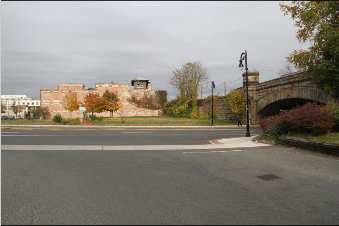
-015 Context from bus station, showing west elevation of Baggage Building and stone arch railroad bridge over Main Street. Looking northeast.
