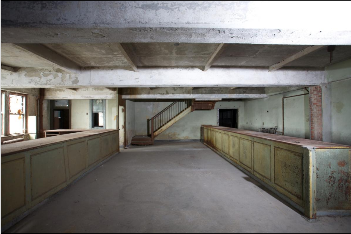
-041 Interior, first floor, office wing, showing customer counters. Looking southeast.
