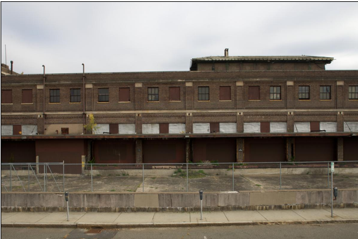
-008 Front elevation, mid-section. Looking southeast.
