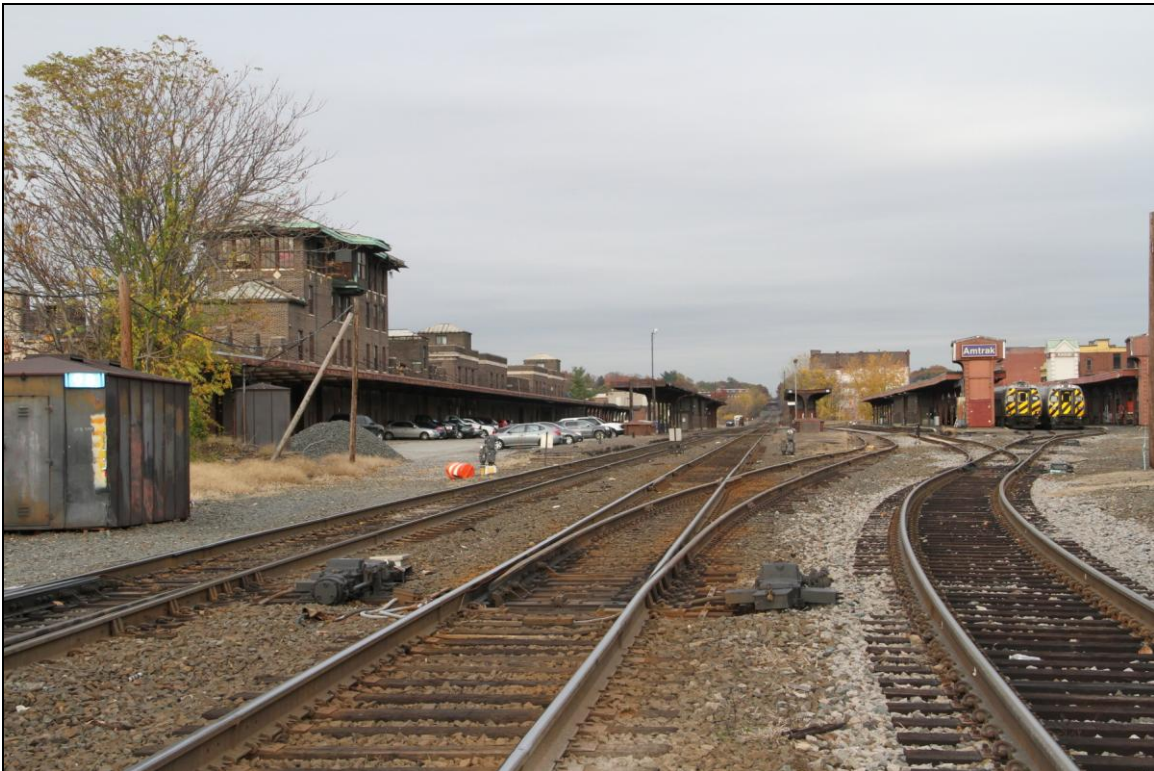
-018 Context from track level, west end of station yard, showing overall view of tracks and platforms. Looking northeast.
