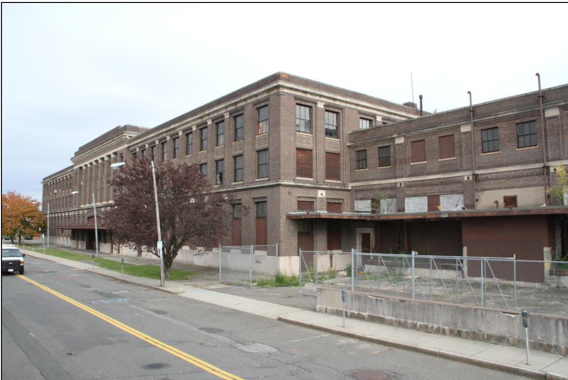
-004 Context, showing connection of Baggage Building, right, with Passenger Station, left. Looking east.
