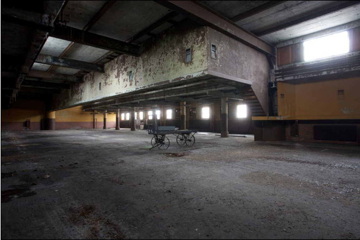
-069 Interior, second floor, east baggage room, overall view. Looking west.
