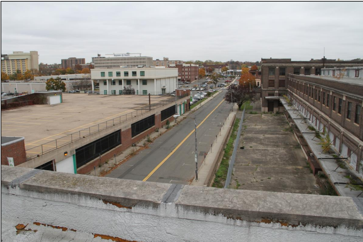
-012 Context, from roof, along Frank B. Murray Street. Looking northeast.
