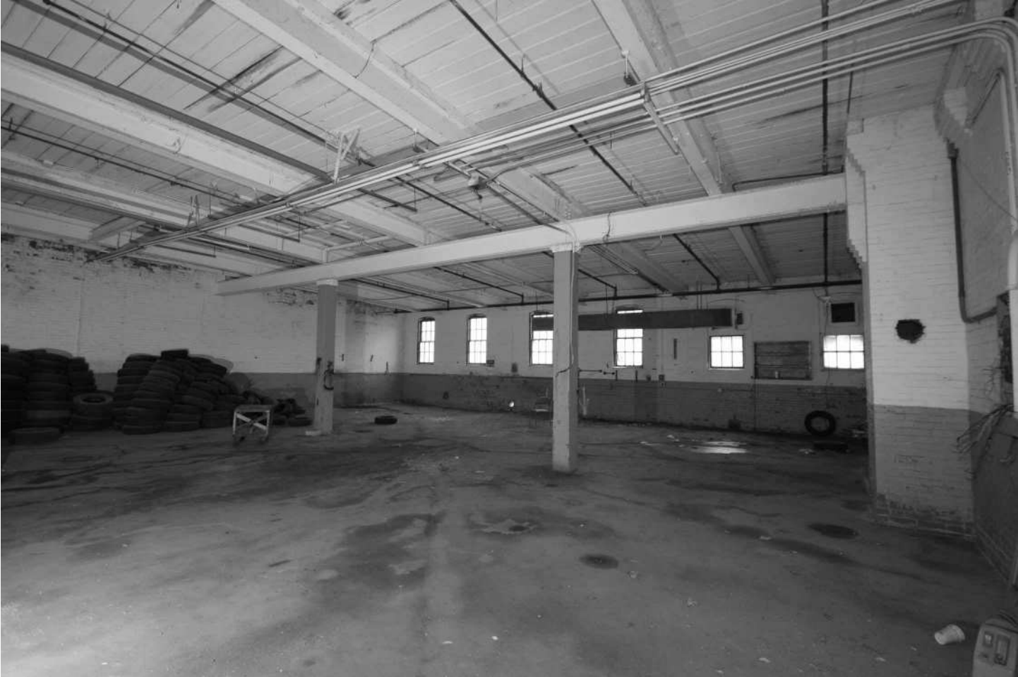
-38 Interior view, Building 1, overall view of garage bays. Looking northeast.
