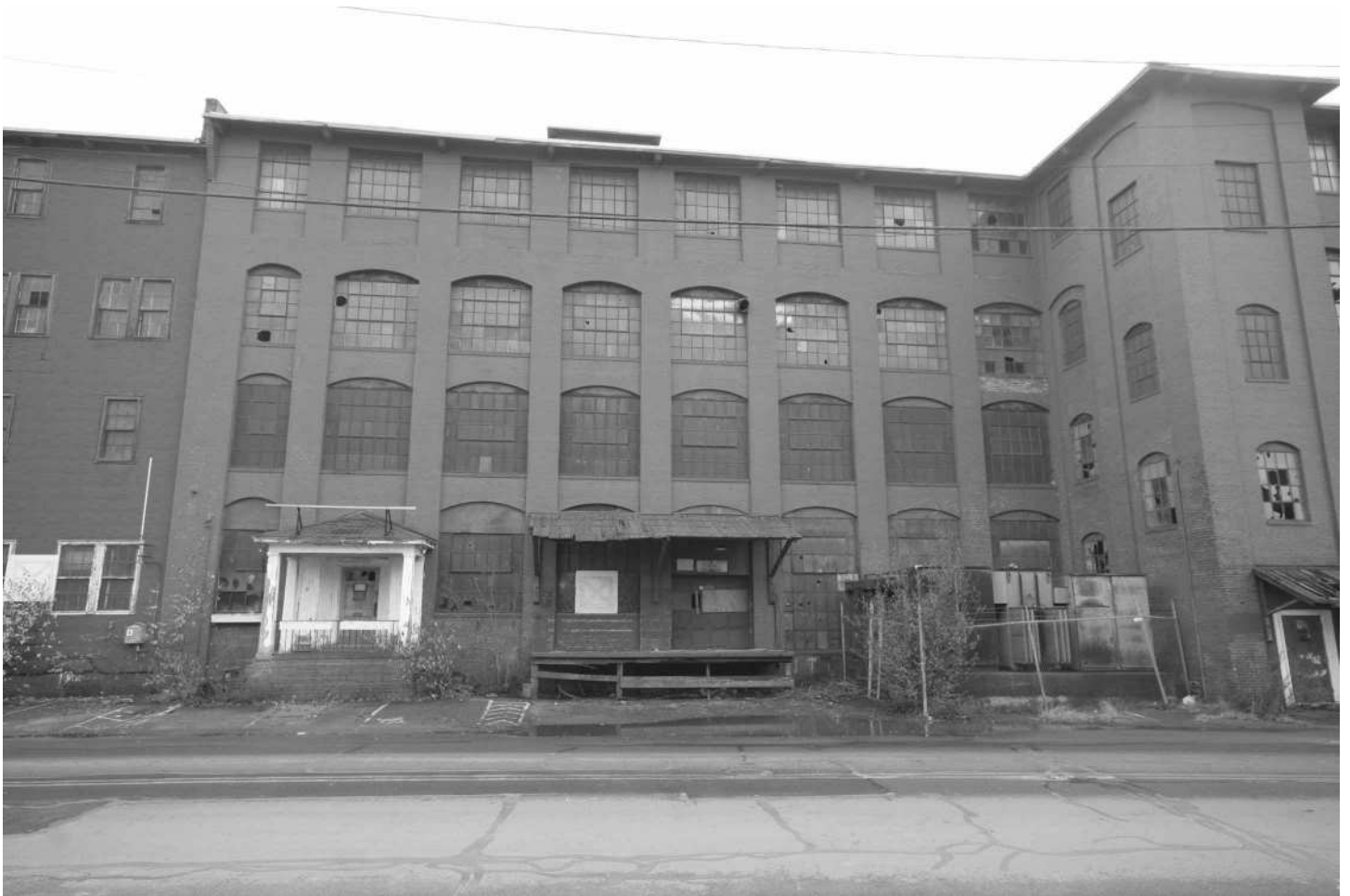
-13 Building 4, west elevation continued. Looking east.
