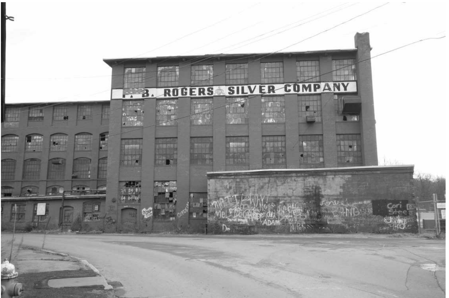
-08 Building 5, west elevation. Looking east.
