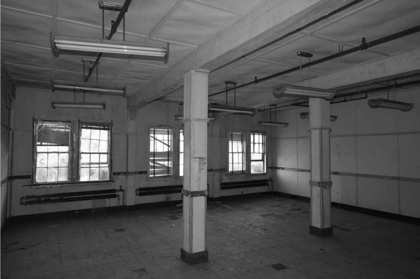
-56 Interior view, Building 3S, first floor, office area. Looking east.
