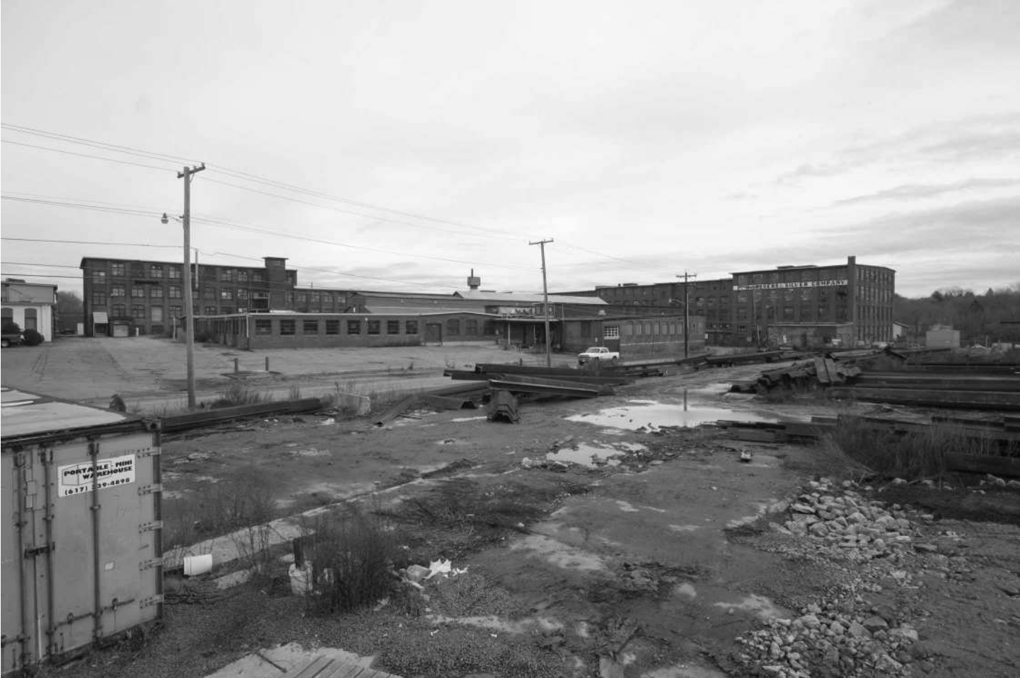
-05 Context, from southwest, view along Fifth Street. Looking east.
