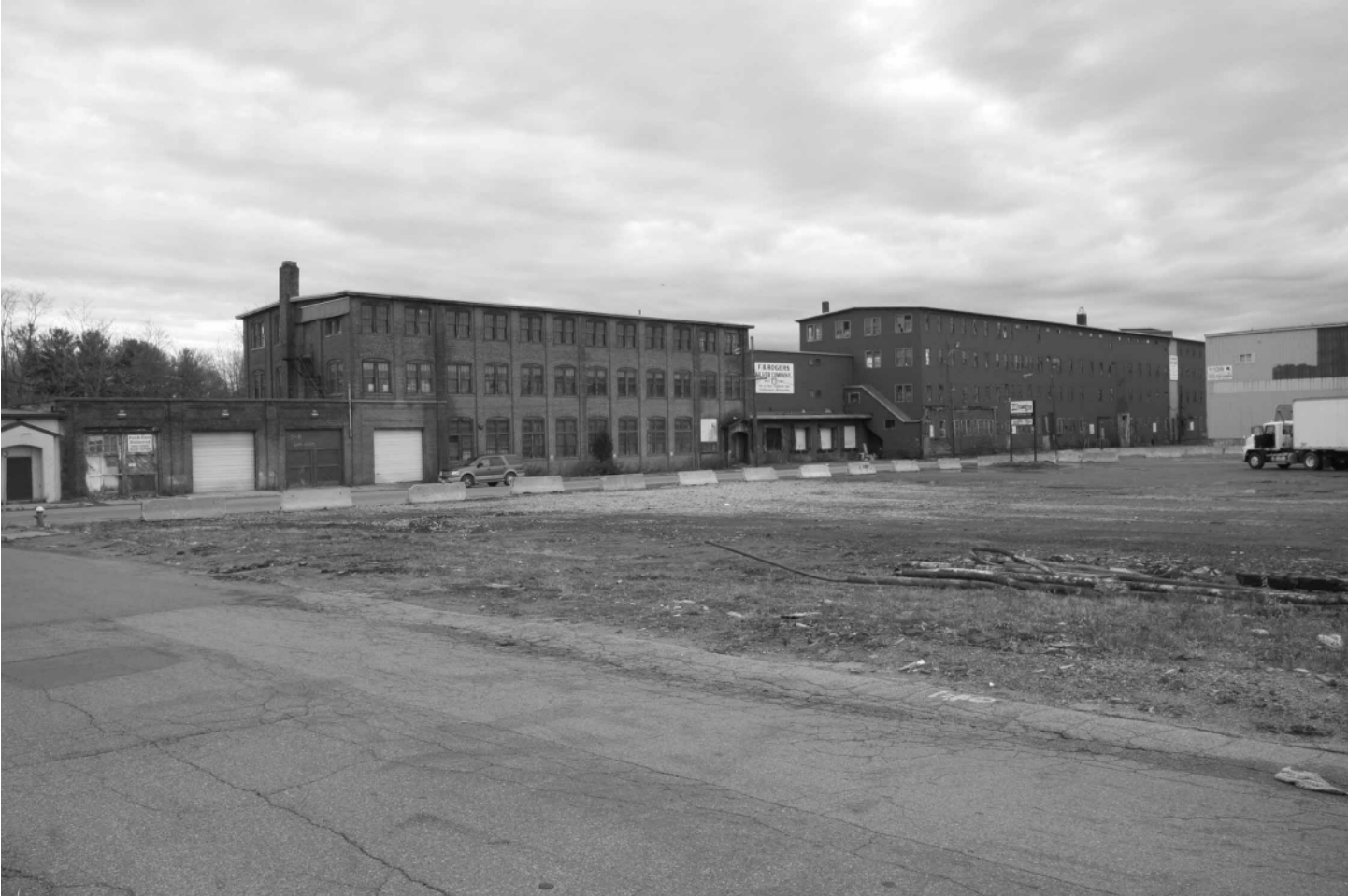
-04 Overall view of buildings at north end of complex. Looking southeast.
