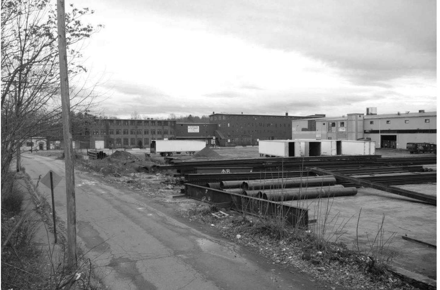
-03 Context, from west, view along Third Street and across steel storage yard. Looking southeast.
