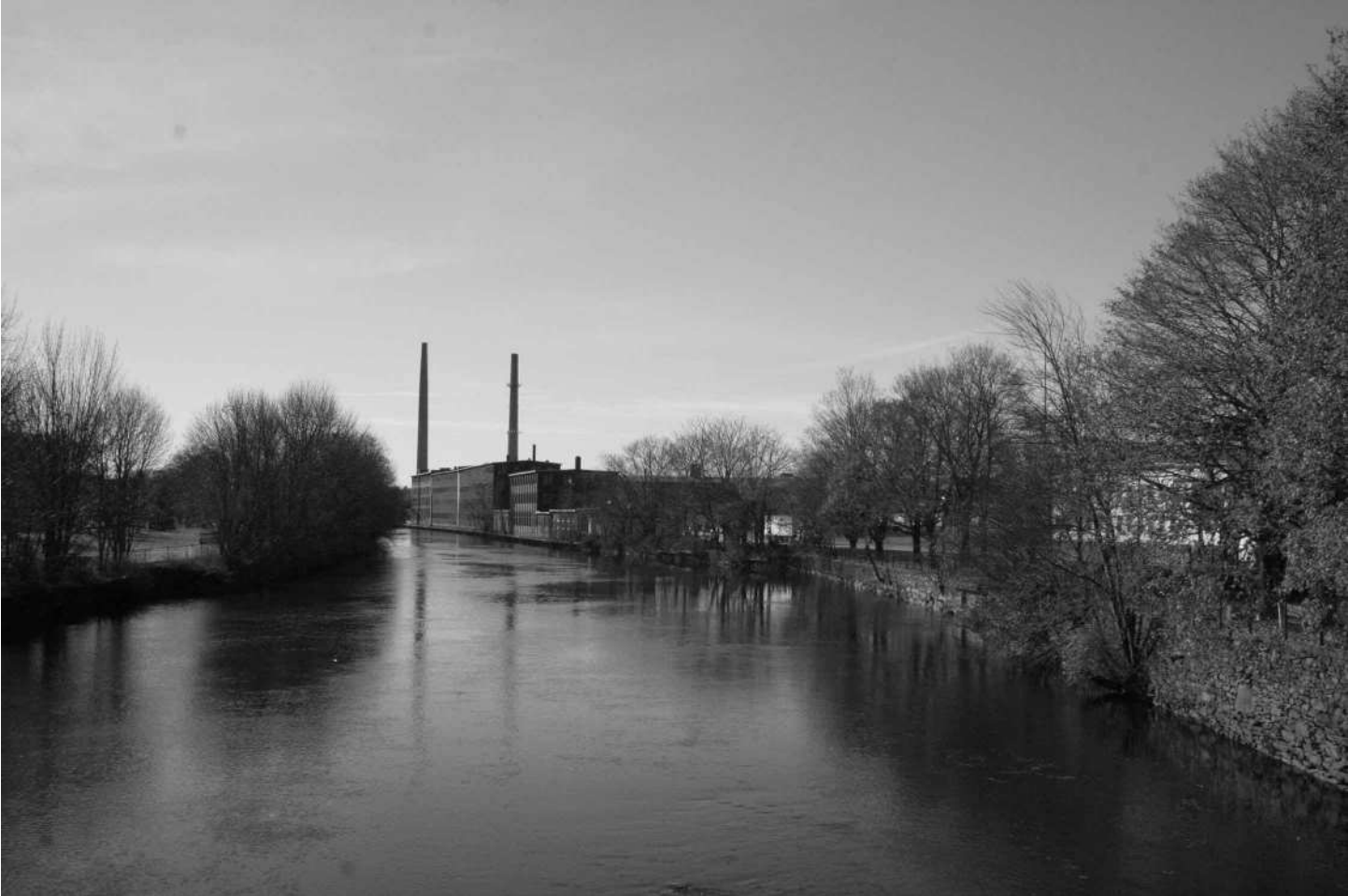
-01 Context, from Plain Street Bridge over Taunton River. Looking south.
