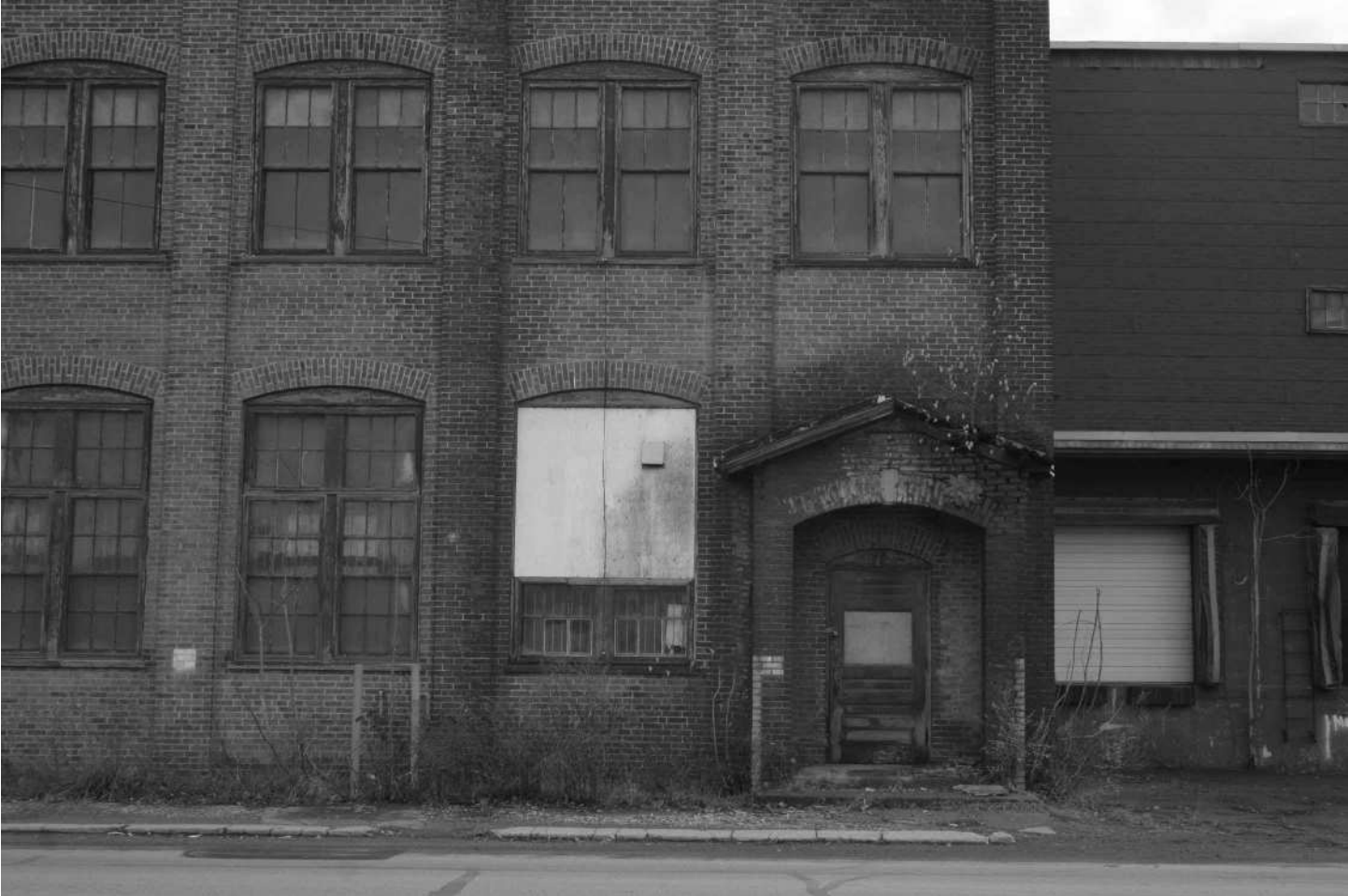
-25 Detail of Building 2, (refer to Photo 24), showing entrance portico, window types and brick work. Looking east.
