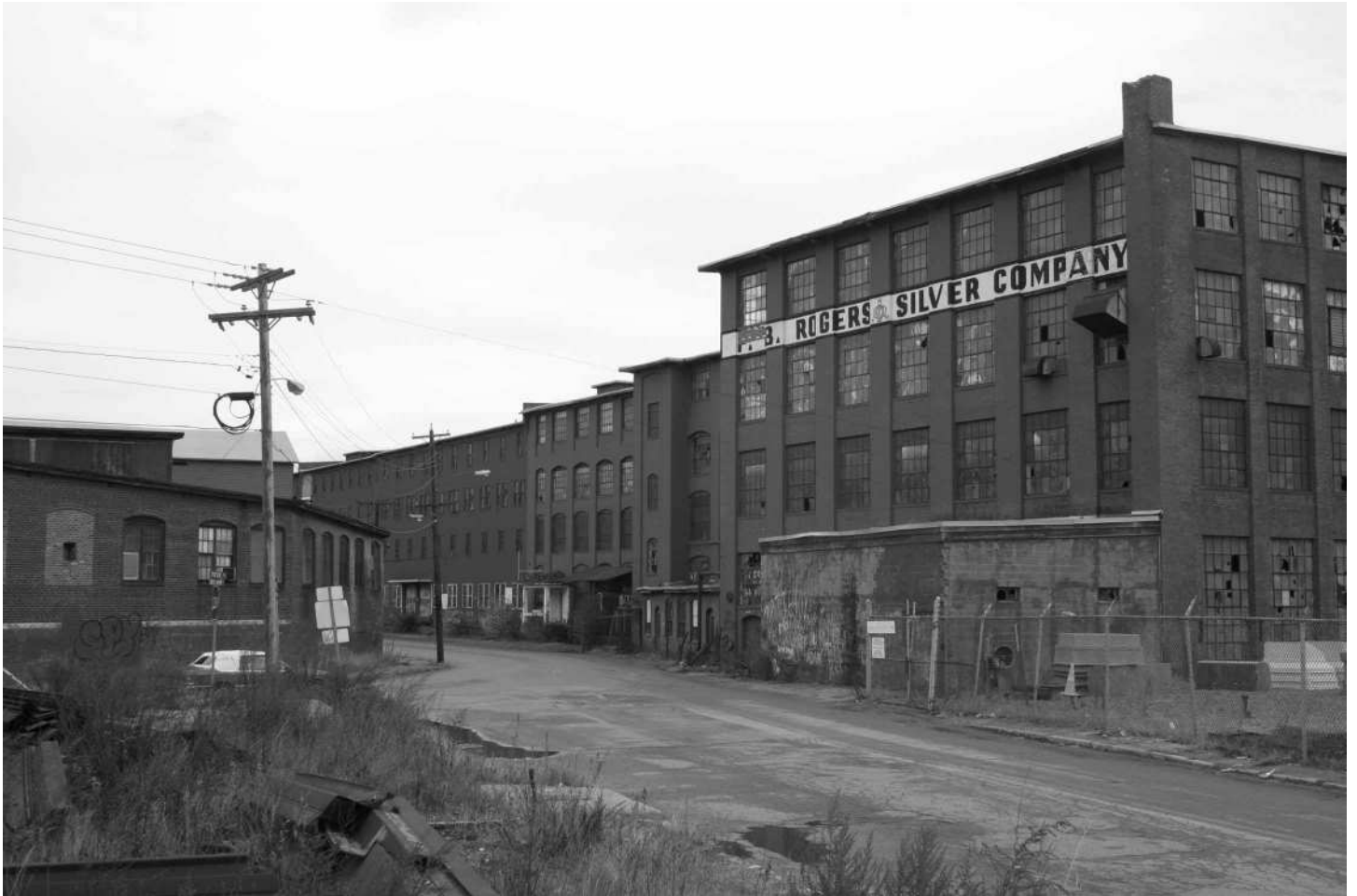
-06 Overall view of buildings at south end of complex. Looking northeast.
