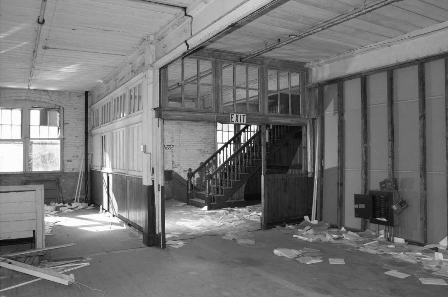
-40 Interior view, Building 2, second floor, stair hall enclosure. Looking southwest.
