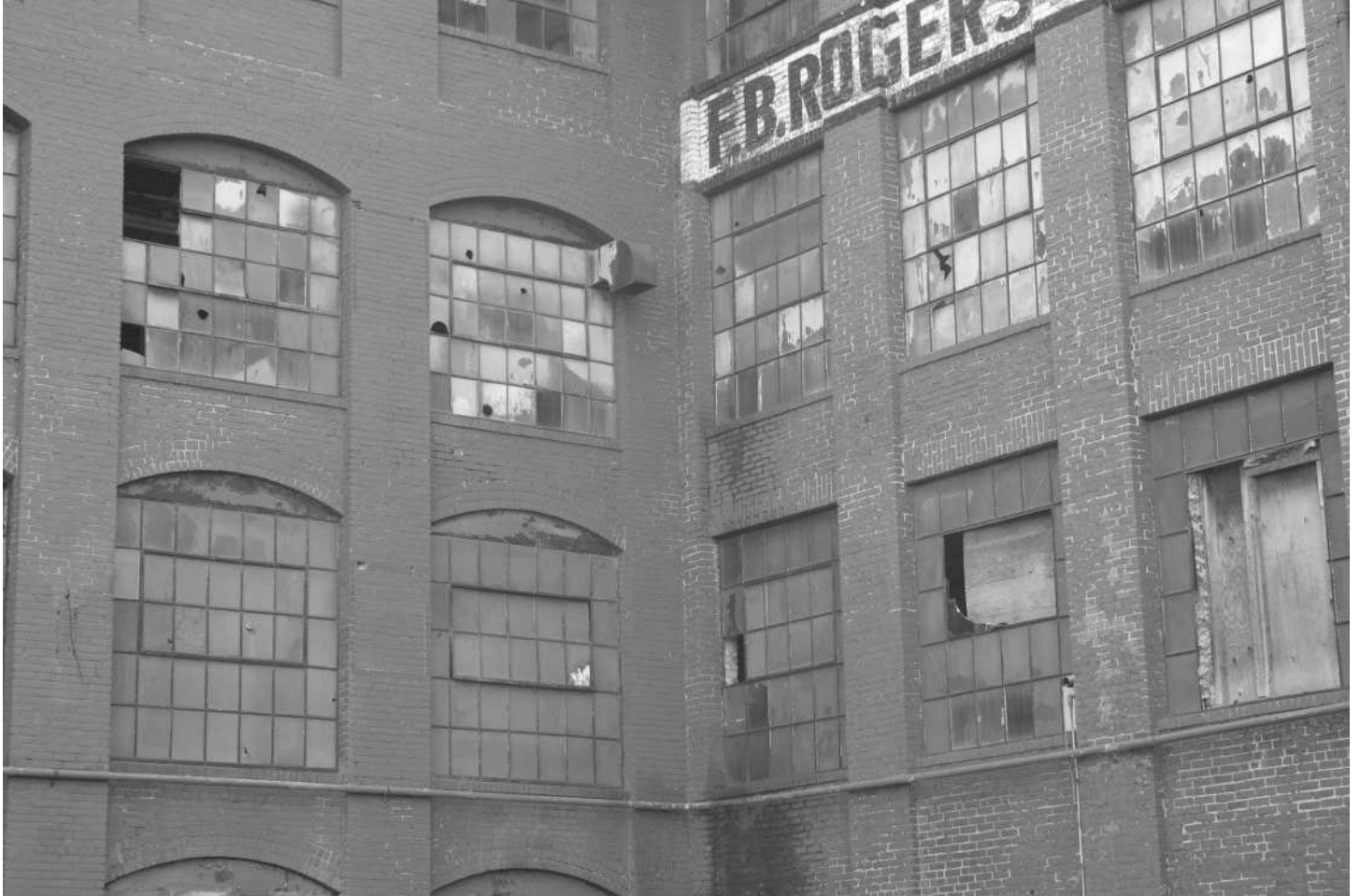
-12 Detail of windows in Buildings 4 and 5 (refer to Photo 9). Looking southeast.
