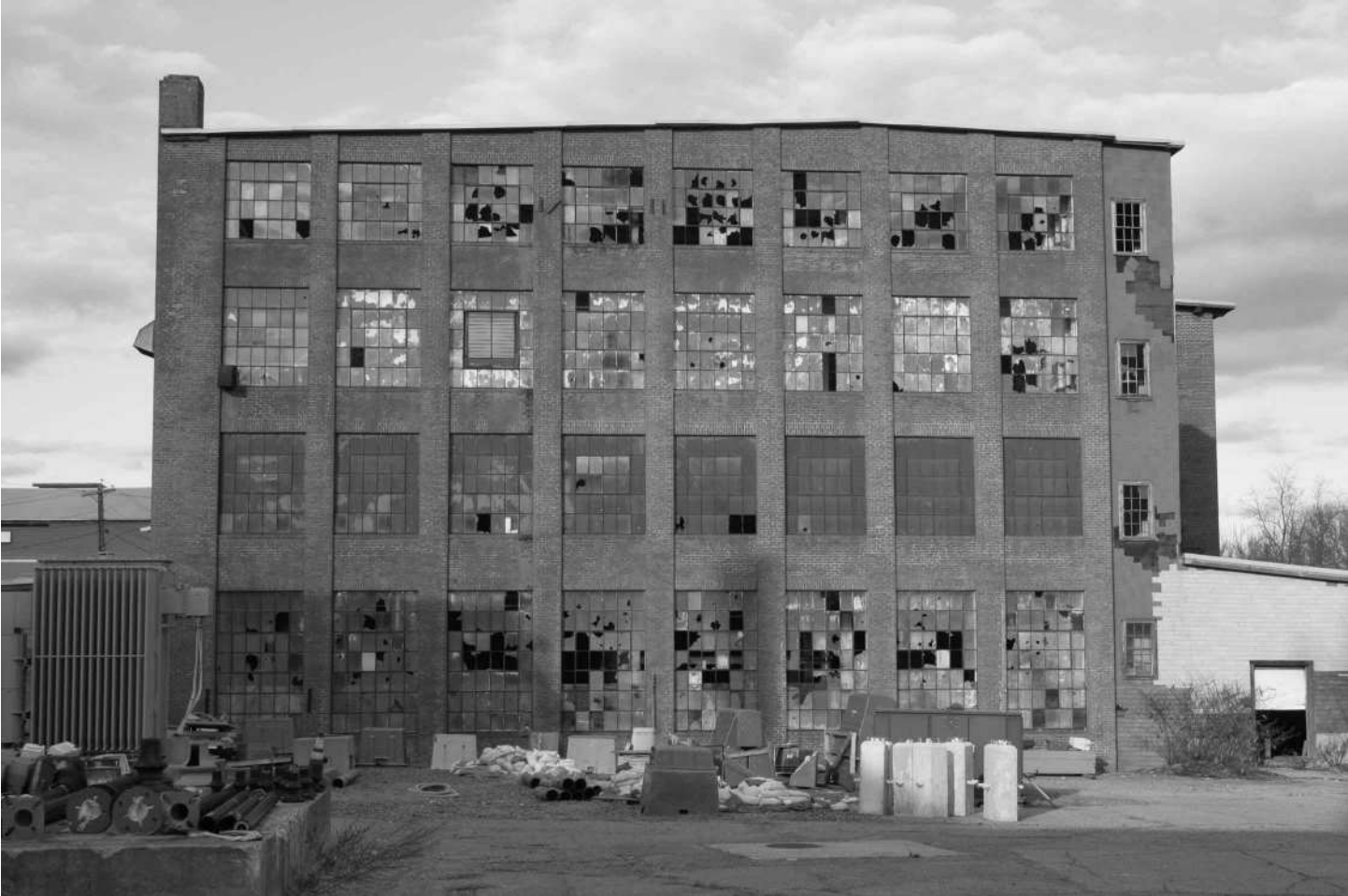
-07 Building 5, south elevation. Looking north.
