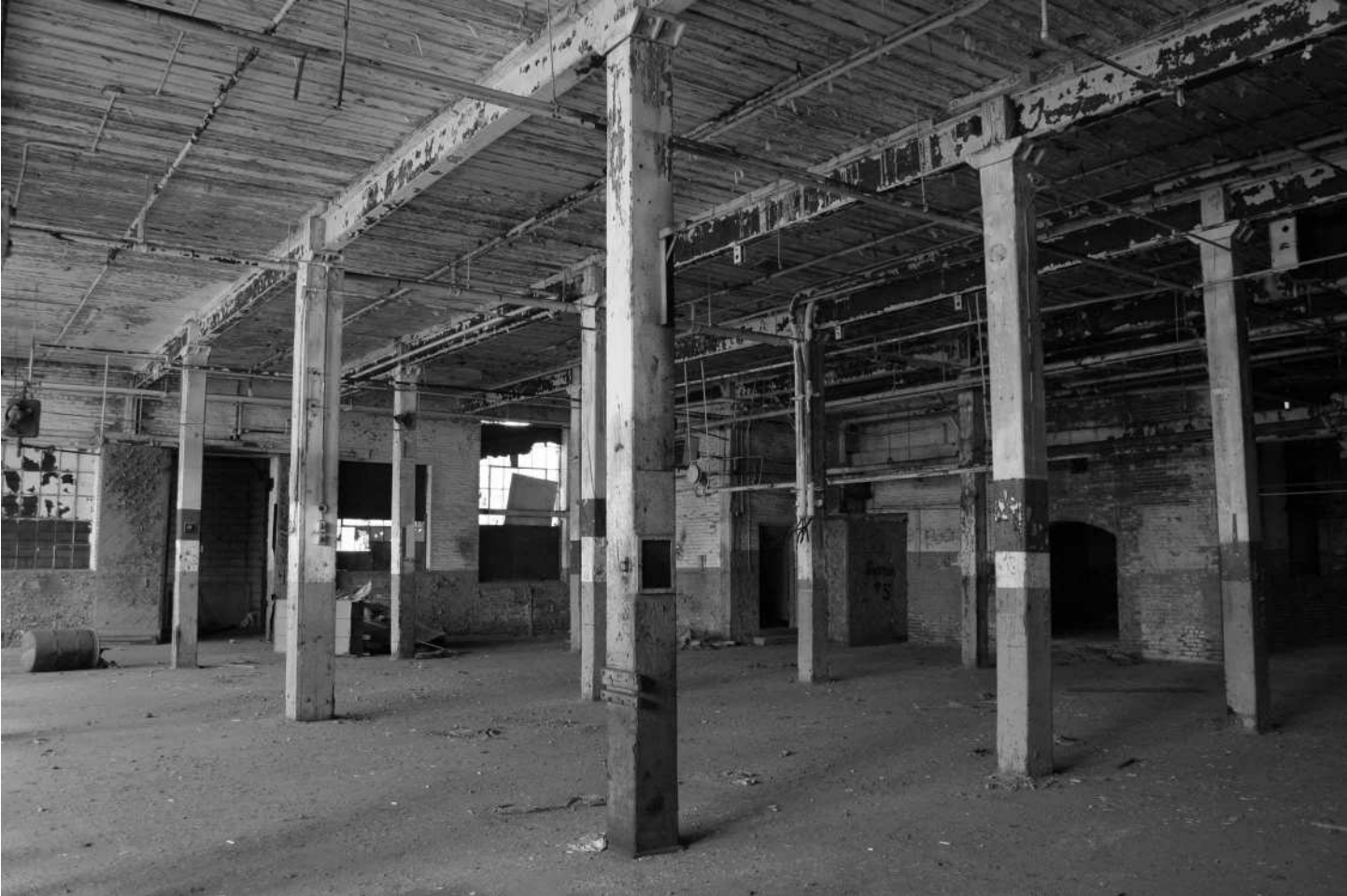
-60 Interior view, Building 5, first floor. Looking northwest.
