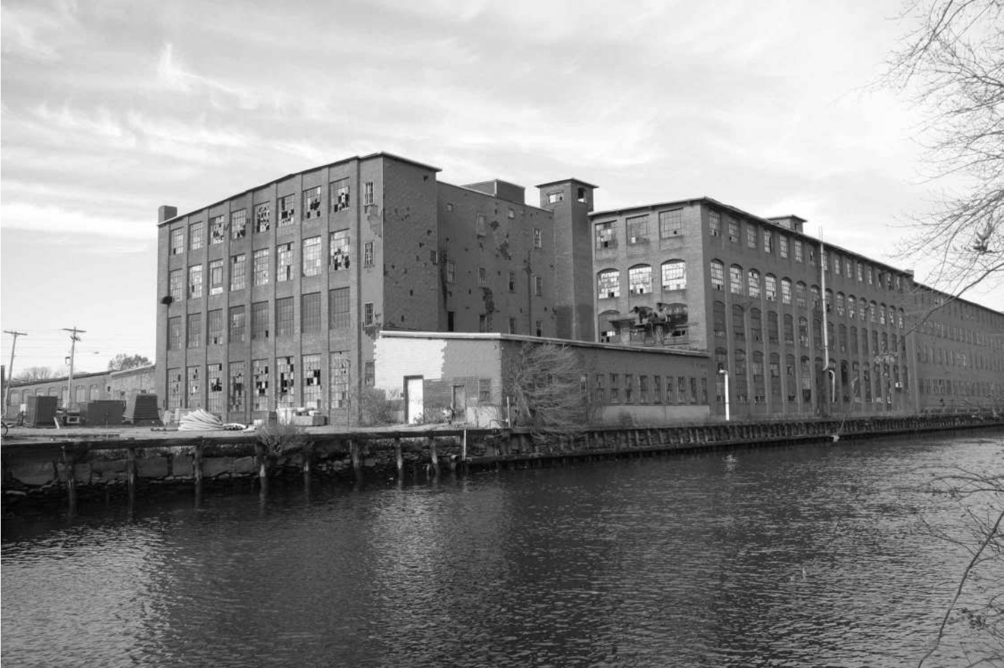
-30 Overall view of south and east elevations of Buildings 4 and 5 at south end of complex. Looking northwest.
