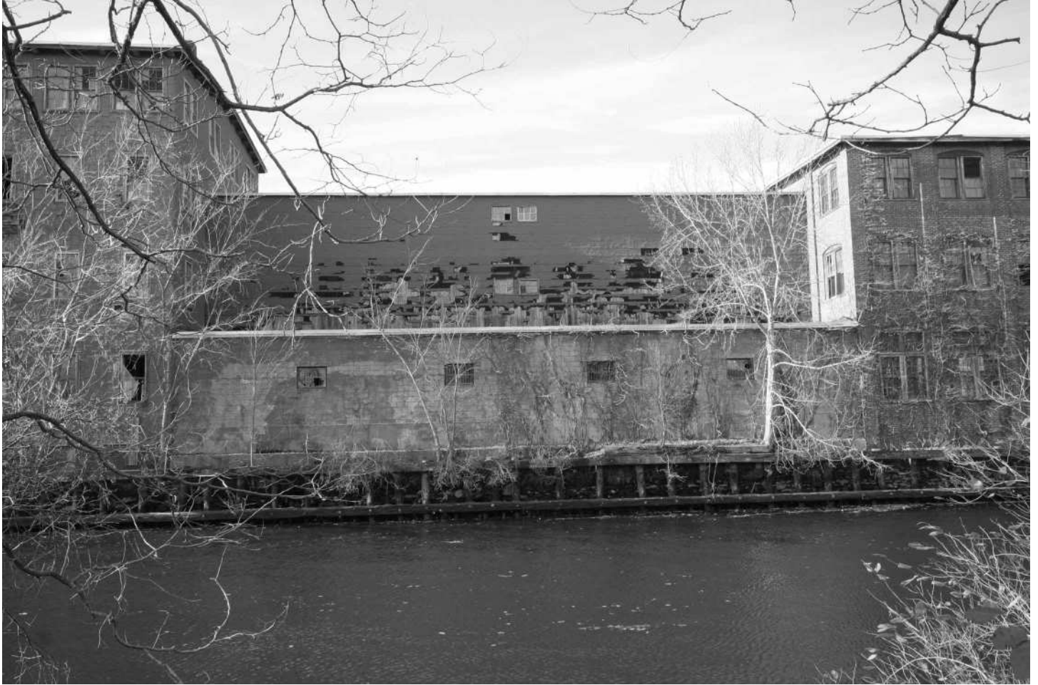
-35 Loading dock building with enclosed walkways above, east elevation. Looking west.
