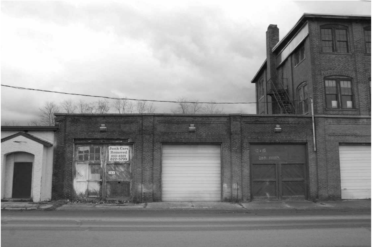
-26 Building 1, west elevation. Looking east.
