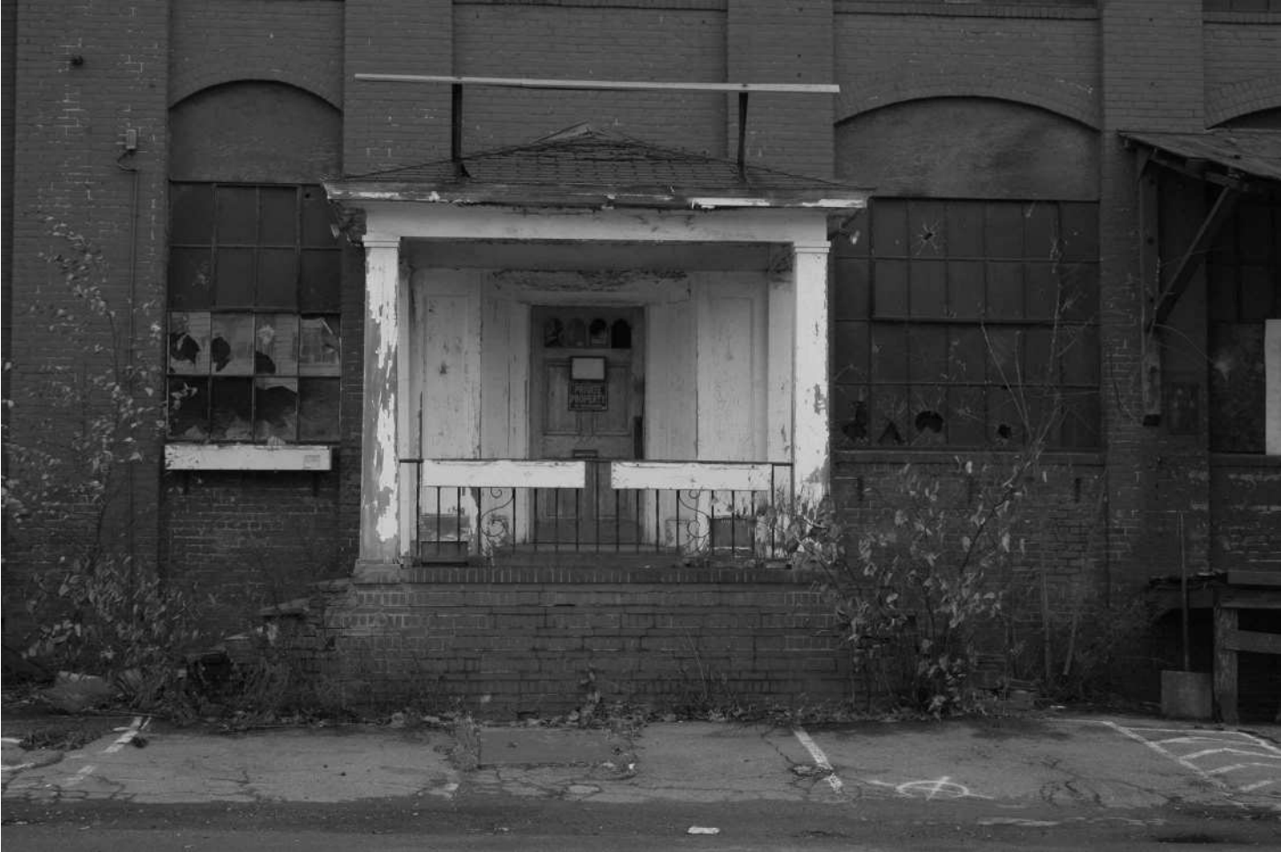
-15 Detail of main entrance, Building 4, (refer to Photo 13). Looking east.
