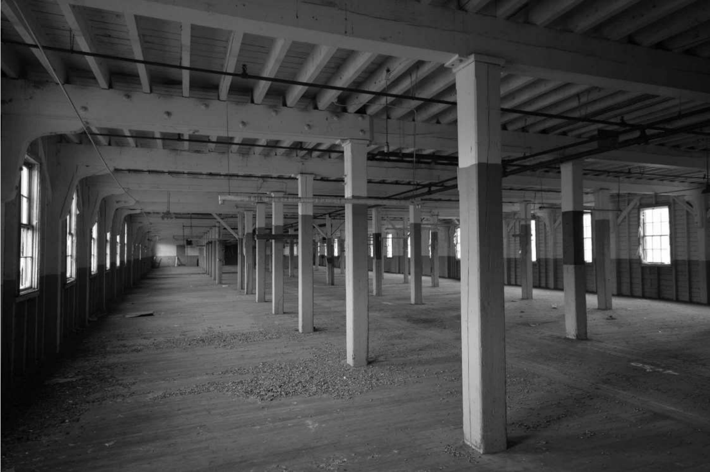
-54 Interior view, Building 3S, third floor, overall view of warehousing floor. Looking south.
