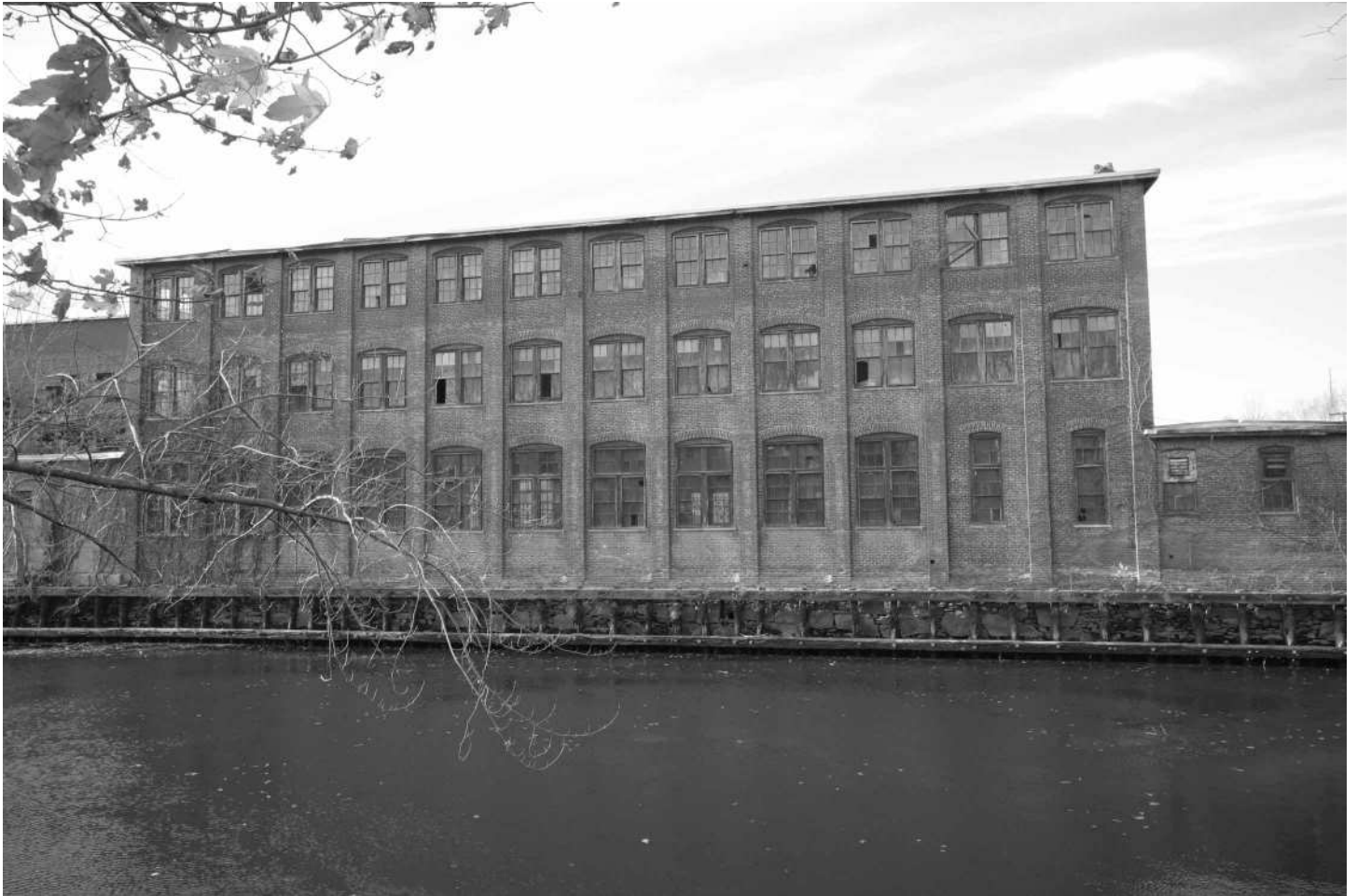
-36 Building 2, east elevation. Looking west.
