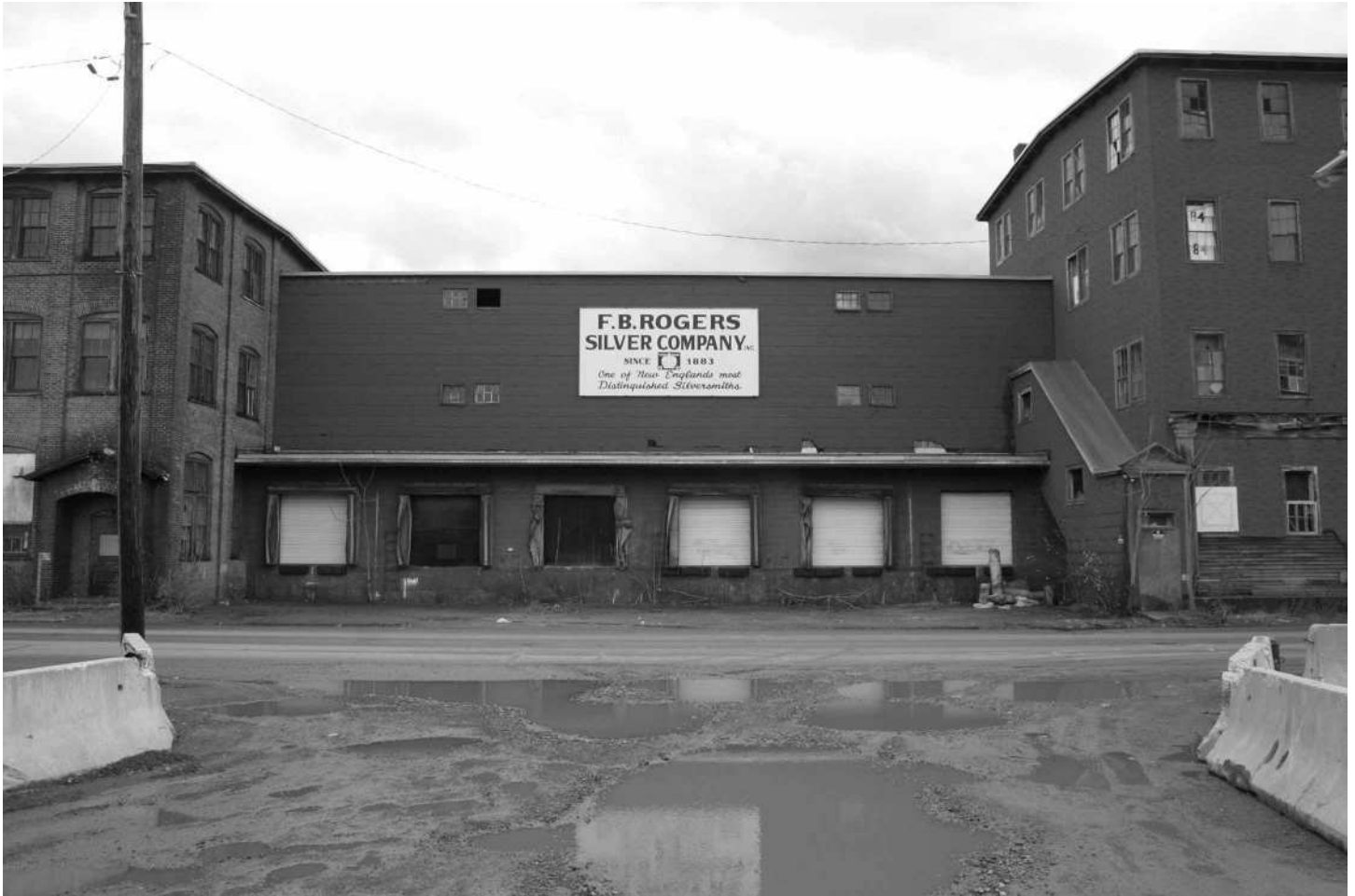
-23 Loading dock building with enclosed walkways above connecting Building 3N to Building 2, west elevation. Looking east.
