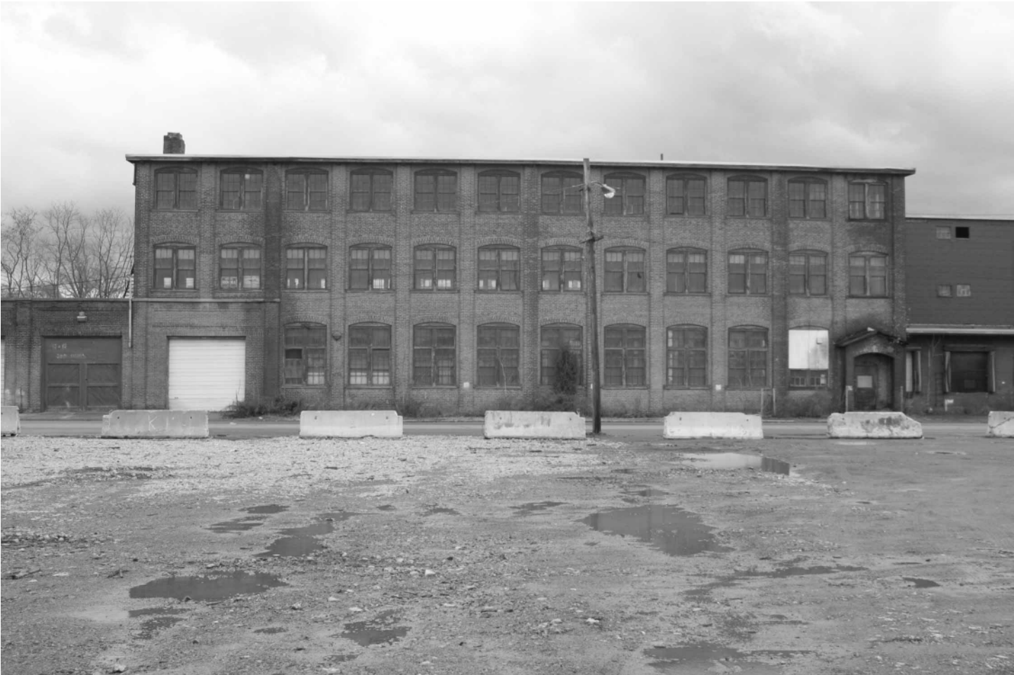
-24 Building 2, west elevation, view east.
