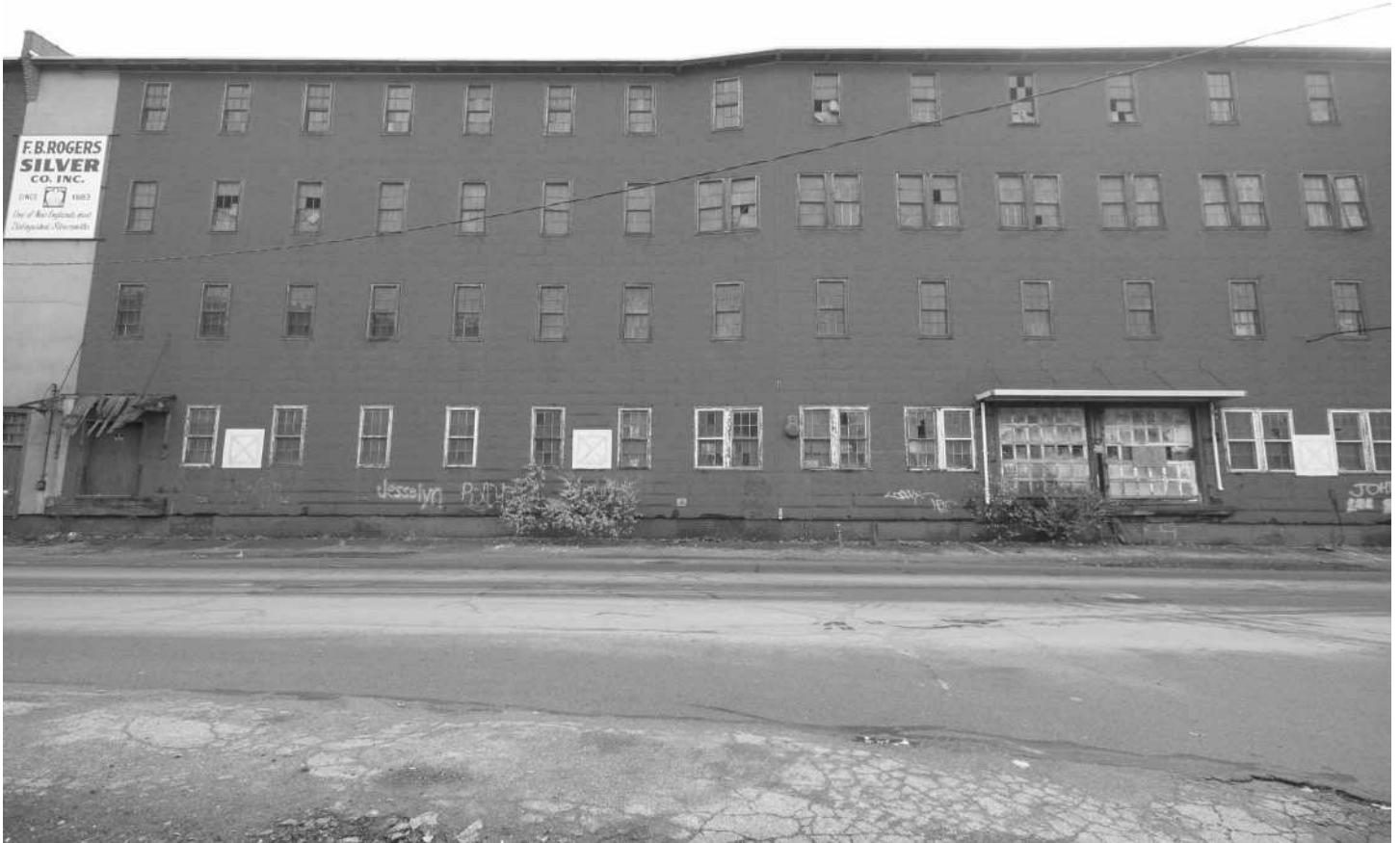
-17 Building 3S, west elevation continued. Looking east.
