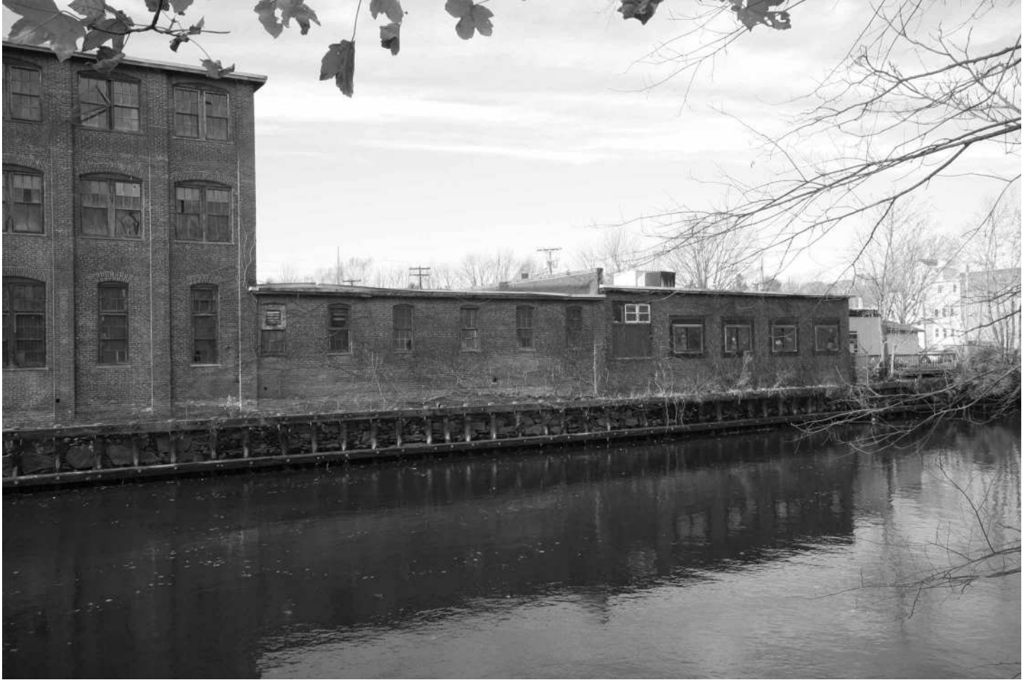
-37 Building 1, east elevation. Looking west.
