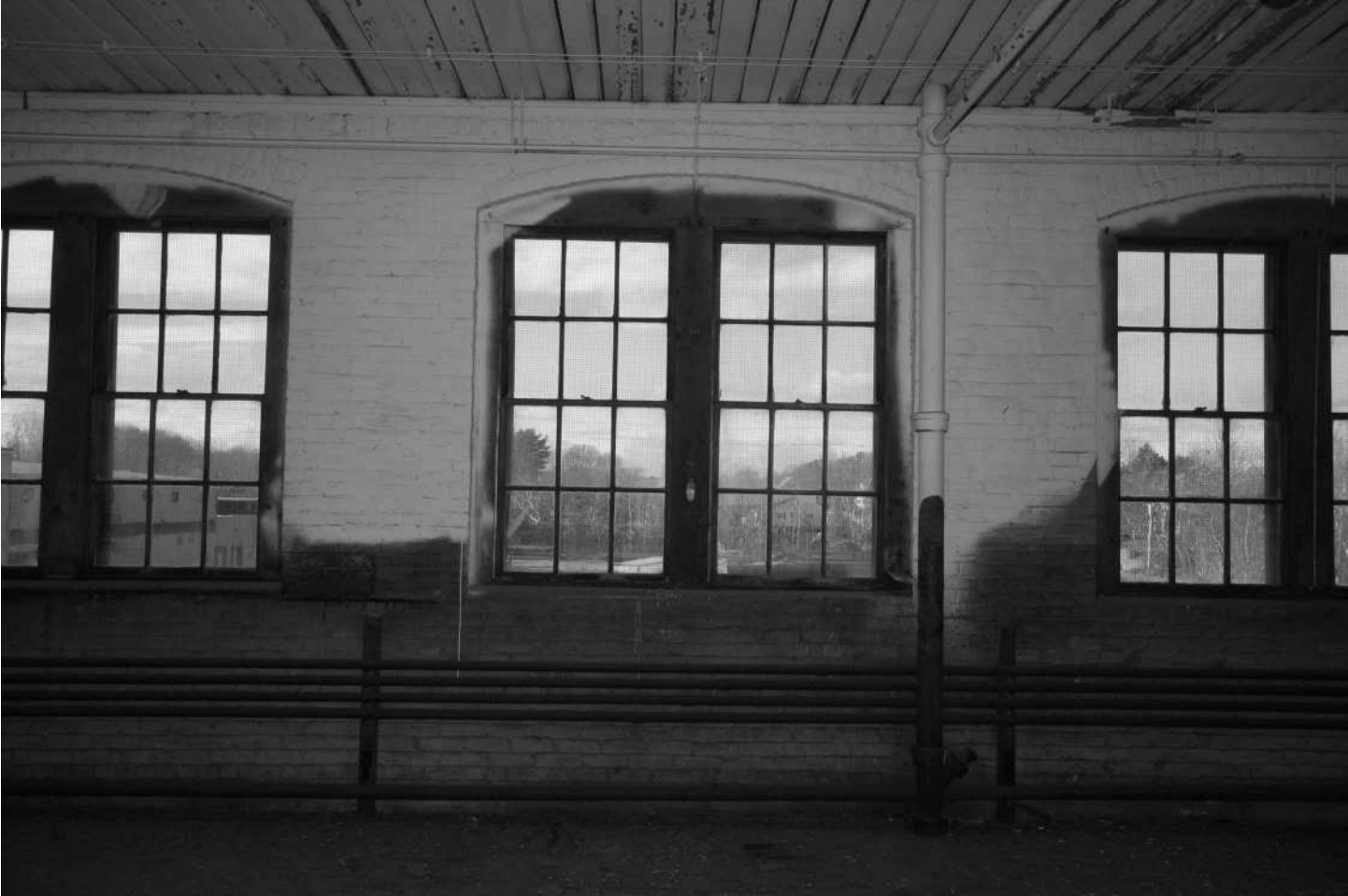
-43 Interior detail, Building 2, third floor, west wall window detail. Looking west.
