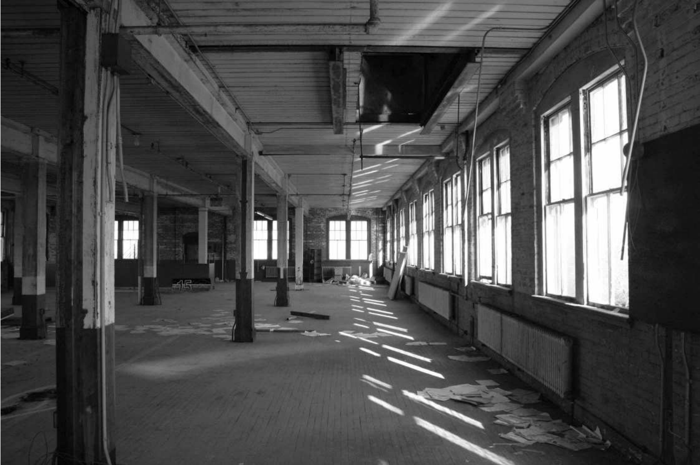
-41 Interior view, Building 2, second floor, factory floor along east wall. Looking north.
