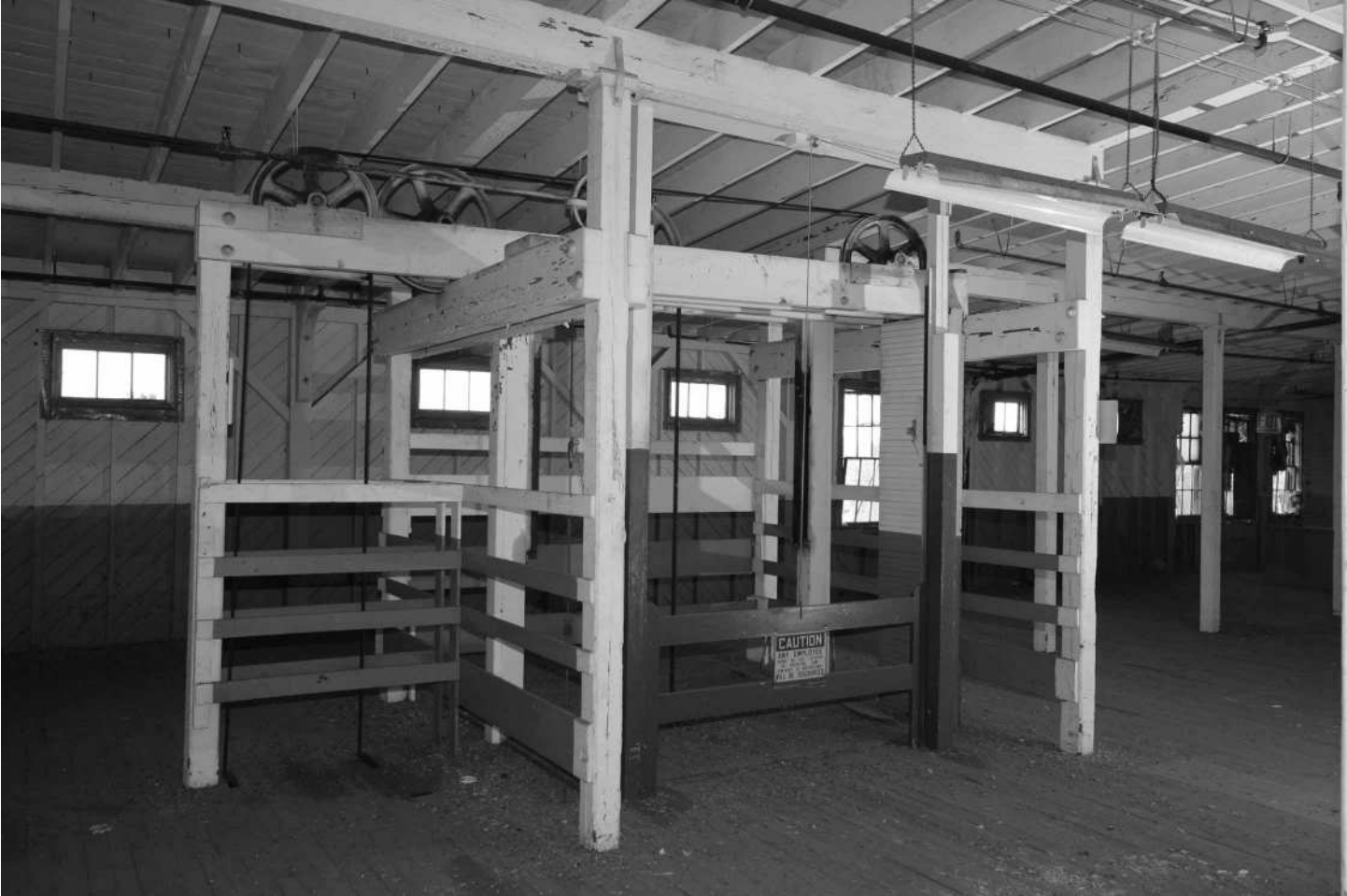
-48 Interior detail, Building 3N, fourth floor, freight elevator. Looking west.
