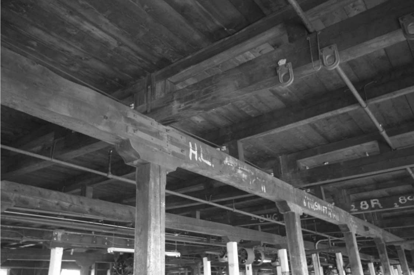
-52 Interior detail, Building 3N, fourth floor, roof structural framing. Looking north.
