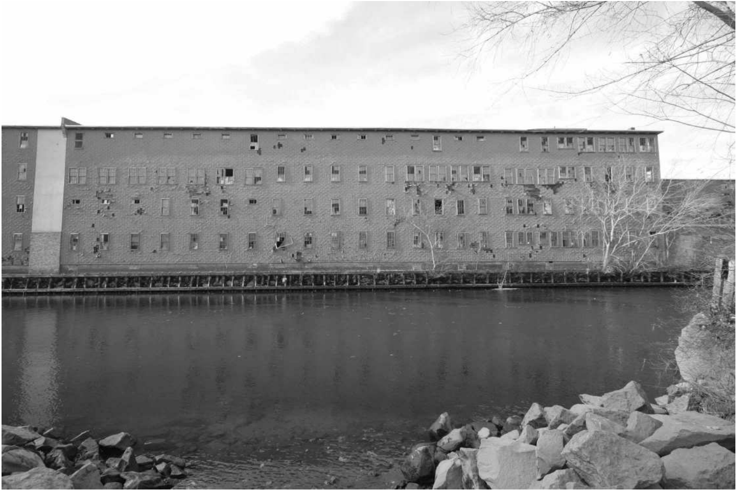
-34 Building 3N, east elevation. Looking west.
