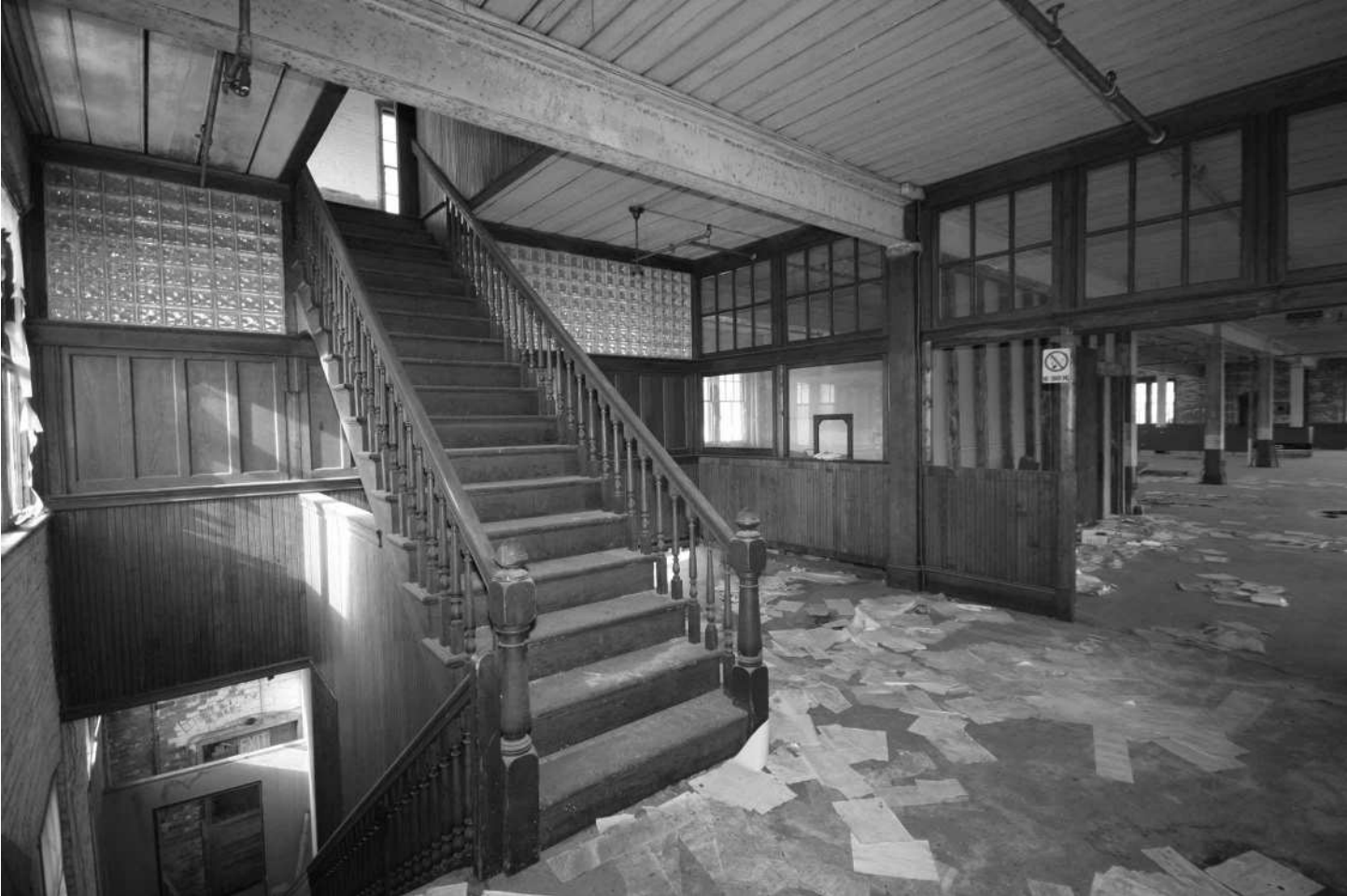
-39 Interior detail, Building 2, second floor, staircase and stair hall. Looking northwest.
