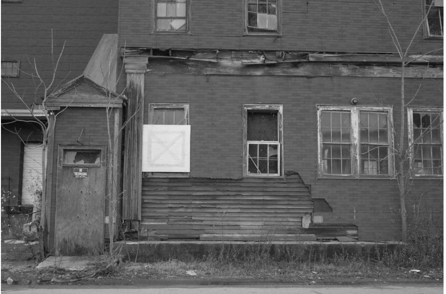
-21 Detail of Building 3N (refer to Photo 20), showing siding types, windows, door and remains of decorative wood pilaster and entablature. Looking east.
