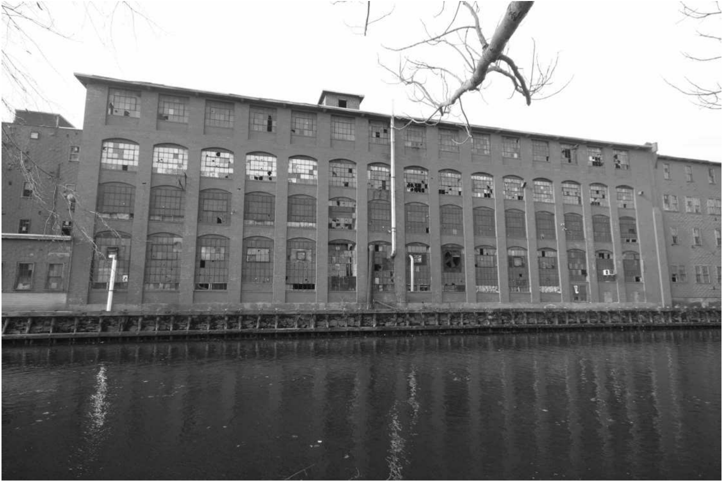
-32 Building 4, east elevation. Looking west.
