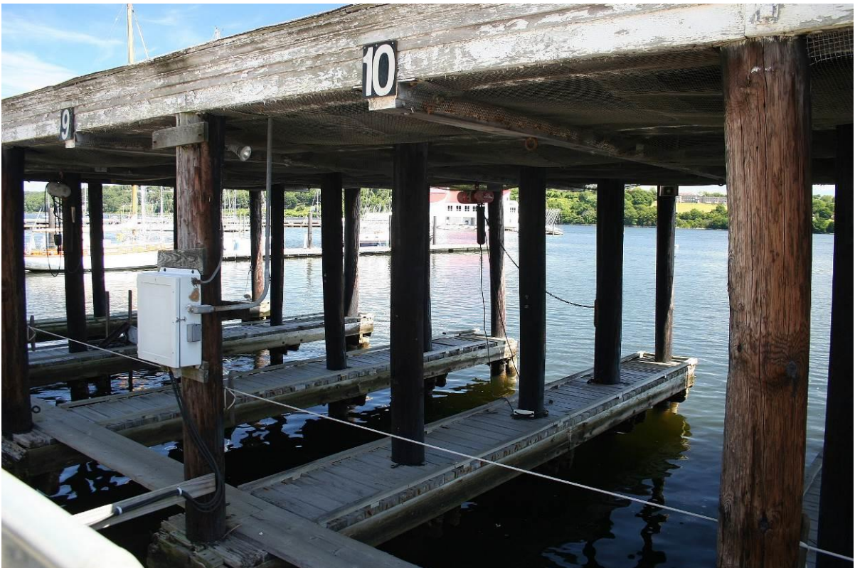
Photo # 24 North Boat House, interior, looking northeast.
