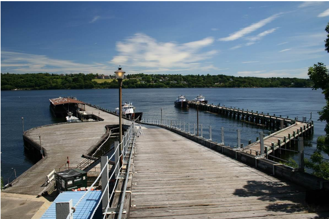
Photo # 02 Ramp to Main Pier, looking east, showing Pier Addition on left connecting to shore, T-Boat Pier on right and South Boat House attached to north side of Main Pier.
