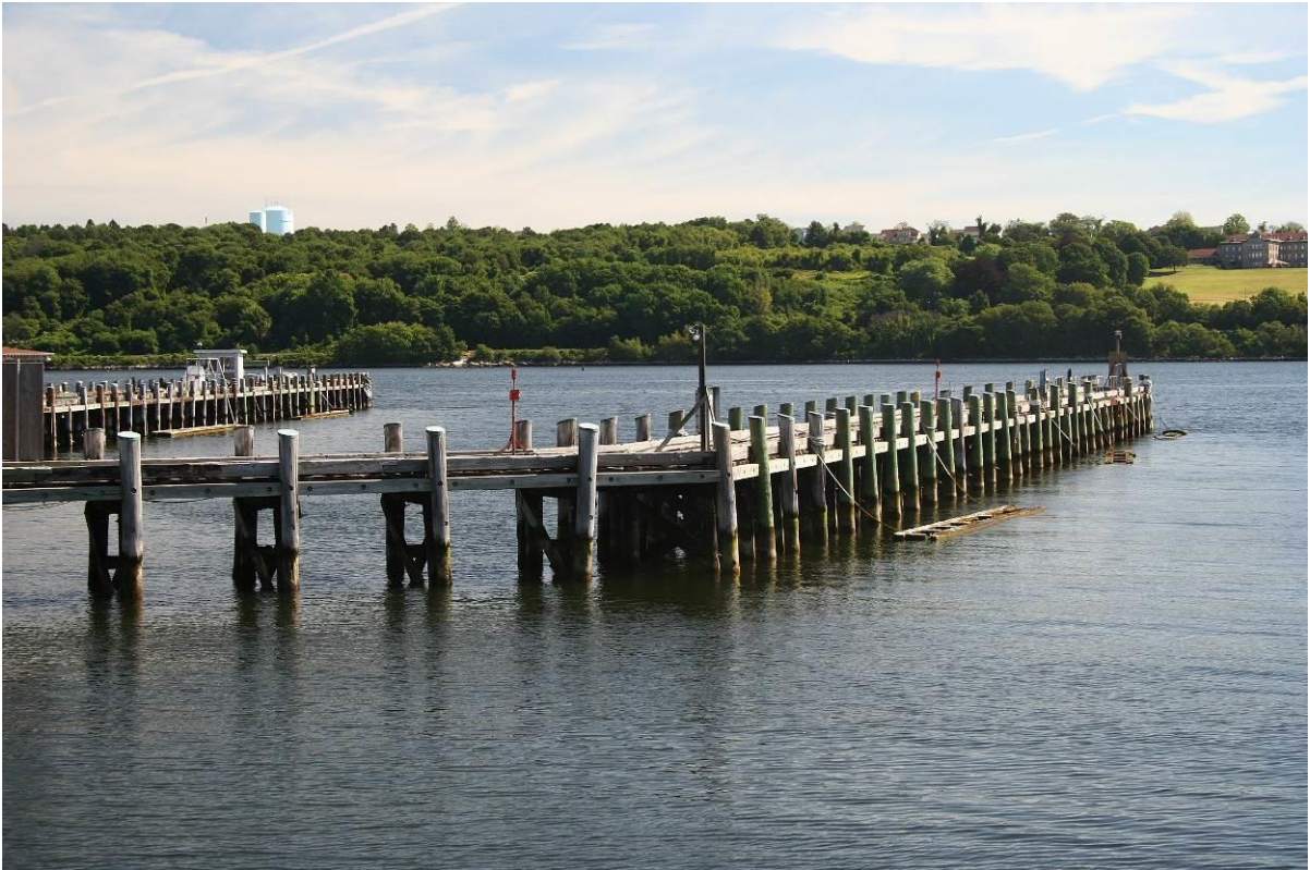
Photo # 25 T-Boat Pier, south elevation, looking northeast.
