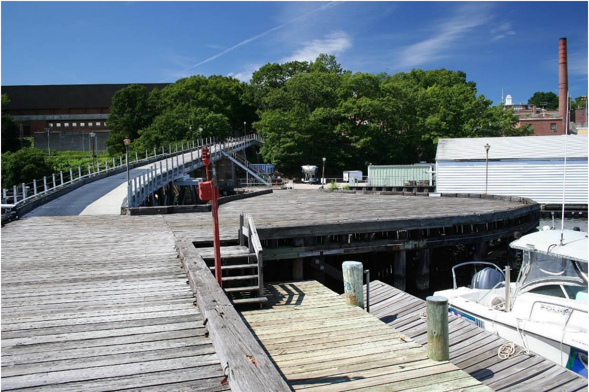
Photo # 03 Ramp and Pier Addition, looking west to shore, showing stairs to Low-Tide Dock on north side of Main Pier.
