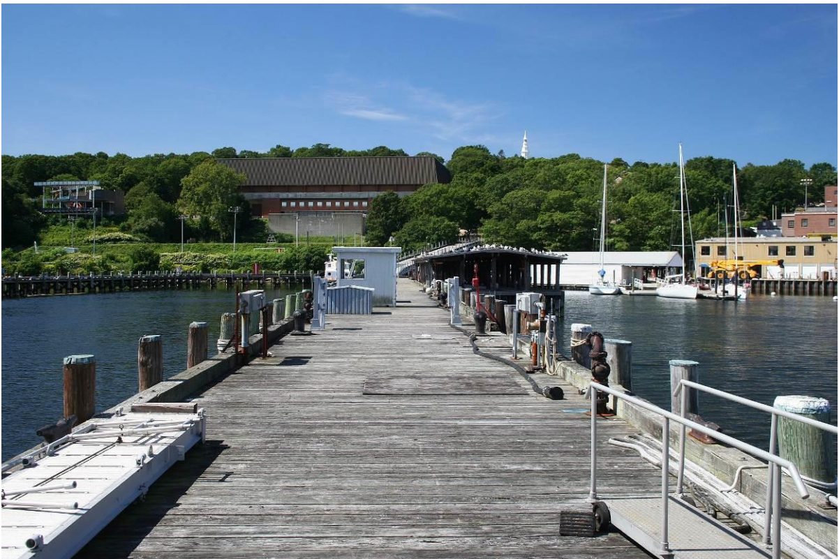
Photo # 12 Main Pier, view from end looking southwest to shore.
