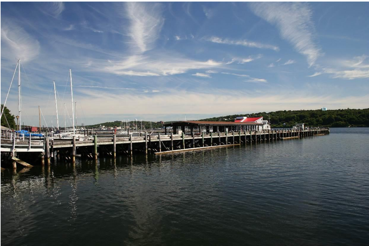
Photo # 10 Overview of Main Pier, looking northeast, showing connection to Ramp on left and South Boat House on opposite side of pier.
