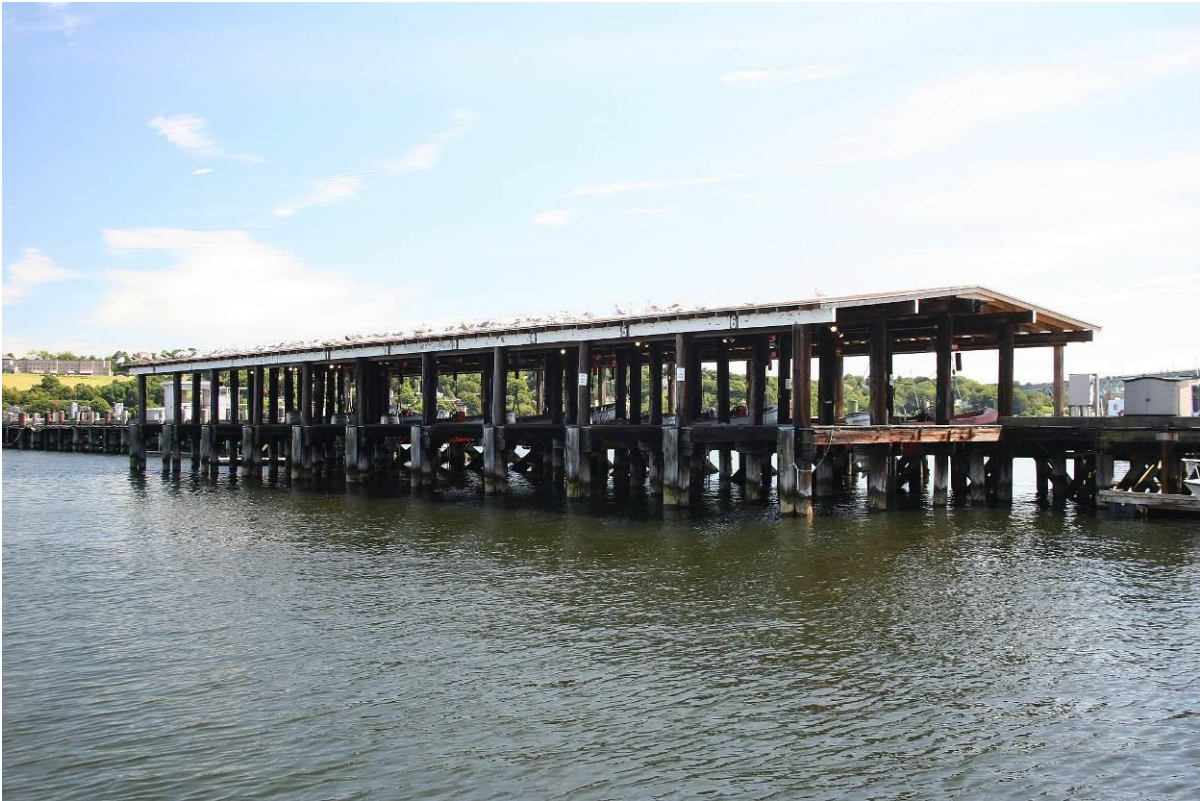
Photo # 19 South Boat House, north and west elevations, looking southeast.
