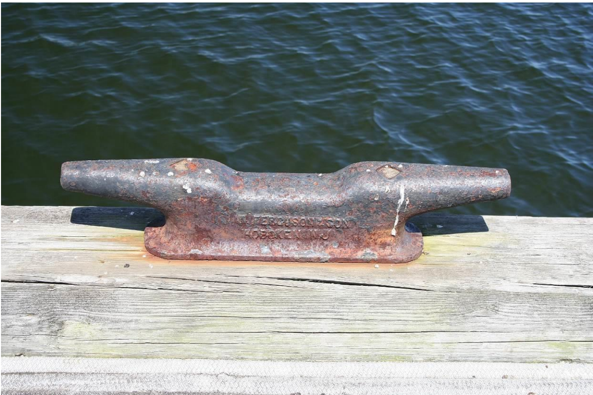
Photo # 14 Detail of iron Cleat on Main Pier for securing lines, looking northwest. Cleat embossed "F. Ferguson & Son, Hoboken, NJ."
