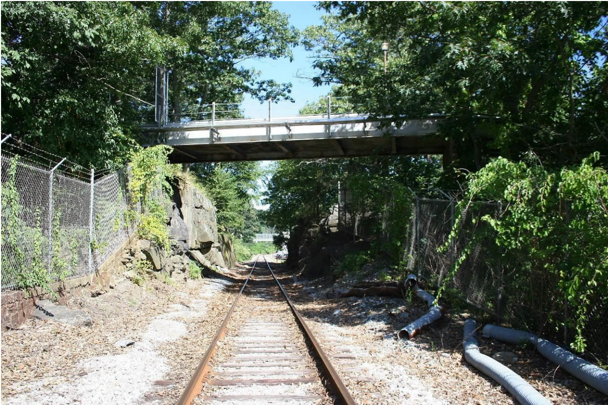
Photo # 07 Bridge to Pier, spanning railroad tracks, looking northwest.
