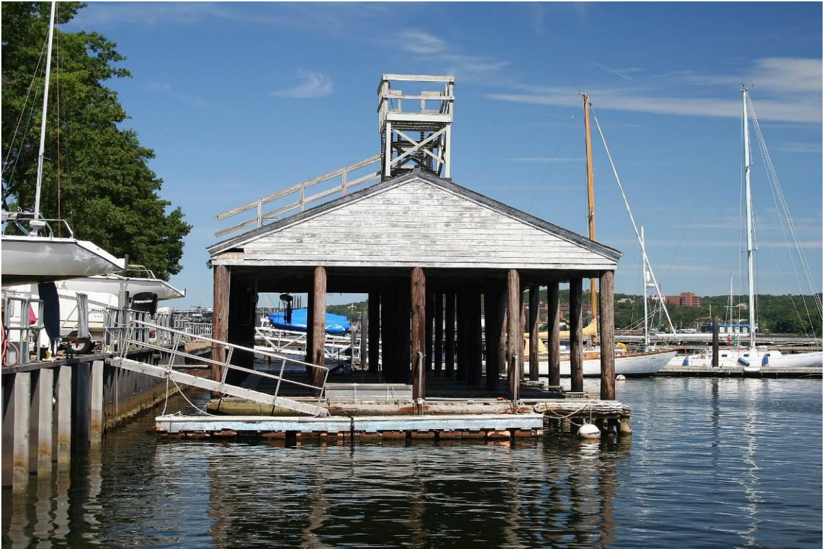
Photo # 21 North Boat House, south elevation, looking north, showing steel shoreline bulkhead on left and observation (reviewing) platform on roof.
