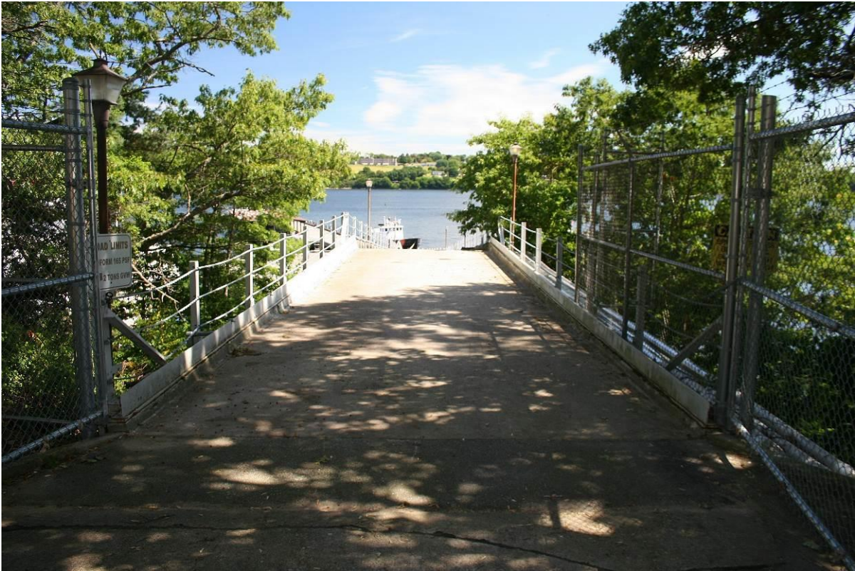
Photo # 09 Bridge to Pier spanning railroad tracks, looking east.
