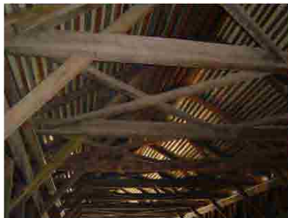
Upper Lateral Bracing
