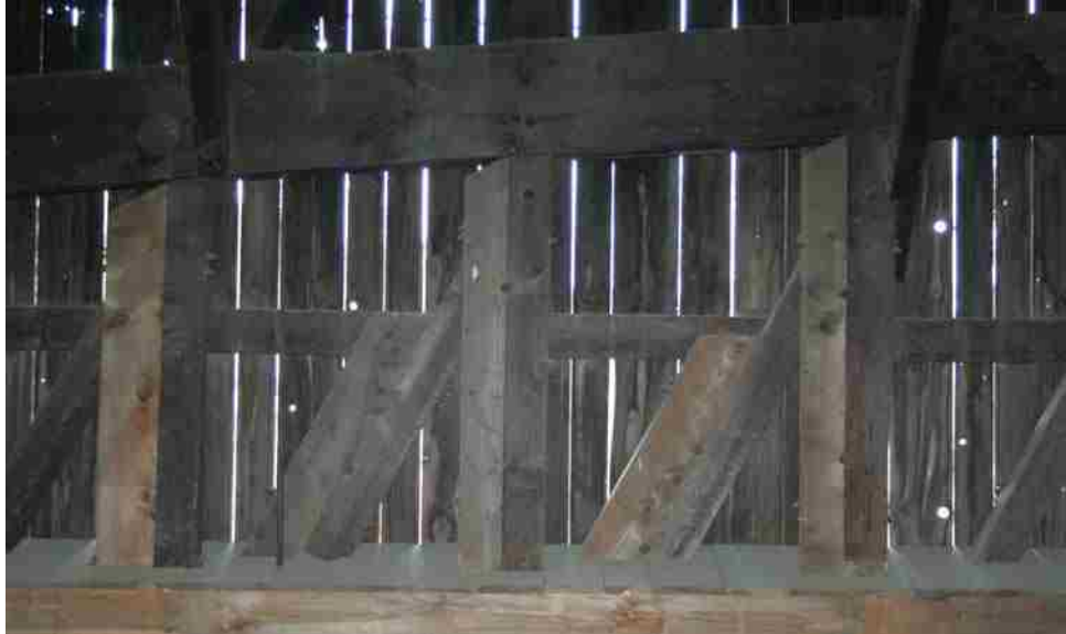
Photo No. 4-11 Diagonal N17L -N18U, Spliced Member
