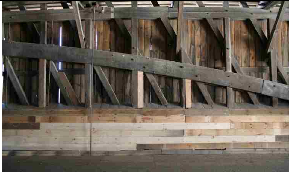
Photo No. 5-7 Built In Arch S14 – S10
