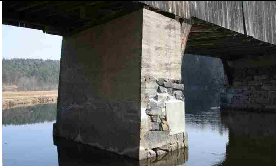
Photo No. 23-2 Pier 1 South (repaired 2007)
