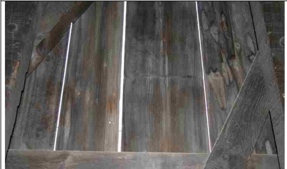
Photo No. 17-5: 15-1/2" & 10-3/4" boards @ Post N10-N11 w/ vertical saw marks
