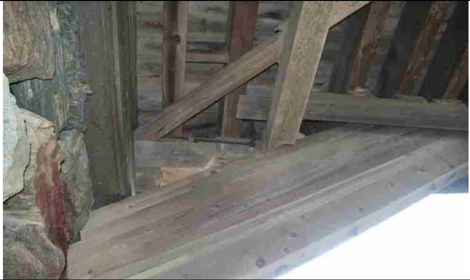
Photo No. 24-5 Abutment, East
