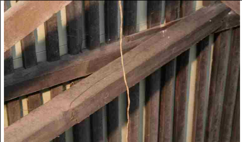
Photo No. 8-4 Knee Brace N5, Split
