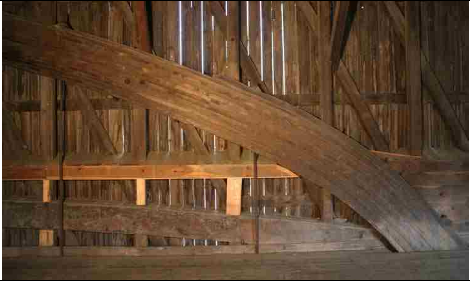
Photo No. 5-10 Built In Arch N56 – N61
