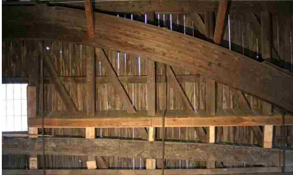
Photo No. 19-6 Added Arch N58 – N54 above Built-in arch below
