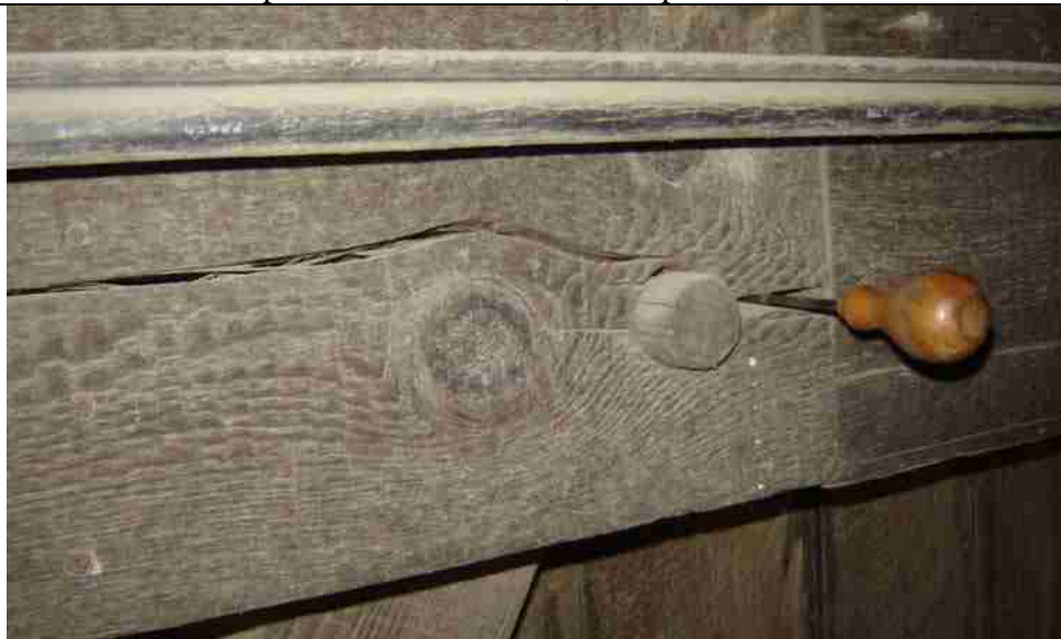
Photo No. 1-6 Top Chord S92 – S96 C, 24” Split at S92
