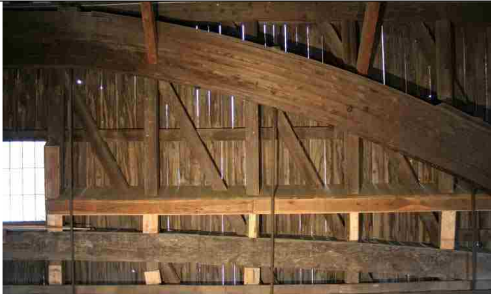
Photo No. 5-9 Built In Arch N58 – N54
