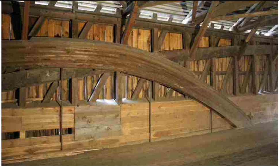
Photo No. 5-5 Built In Arch S31 Oblique
