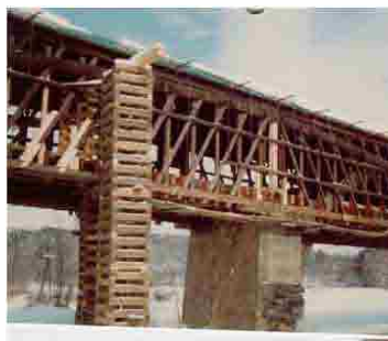
Pier 1 During Repairs made in the 1980's
