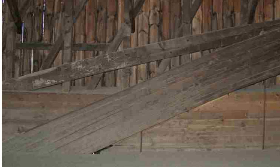
Photo No. 19-2 Added Arch S90 – S86 with flatter Built-in arch behind
