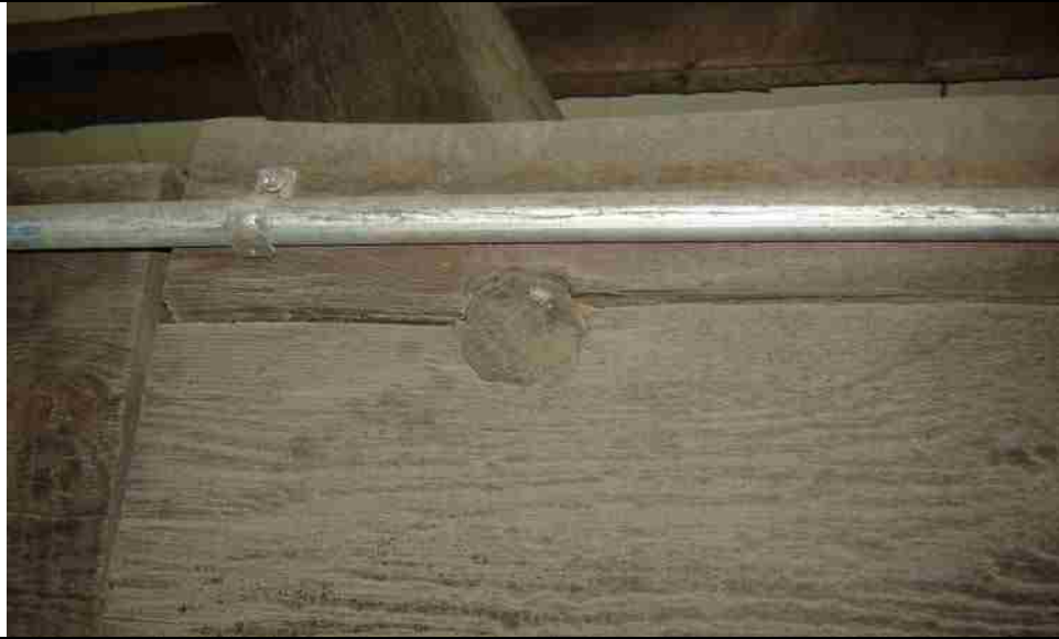
Photo No. 1-6 Top Chord S92 – S96 C, 24” Split at S92
