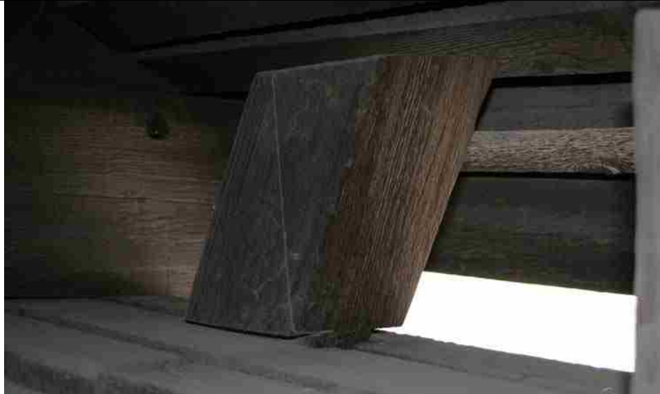
Photo No. 4-15 Diagonal N66L – N67U, Splits in Upper Tail
