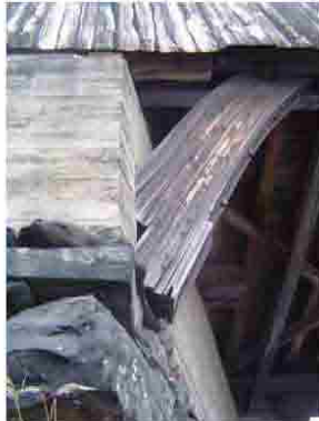
Southwest Arch Bearing at Pier One
