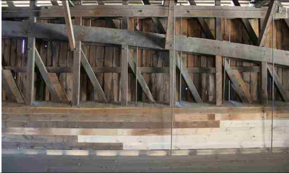
Photo No. 5-2 Built In Arch S18 – S14
