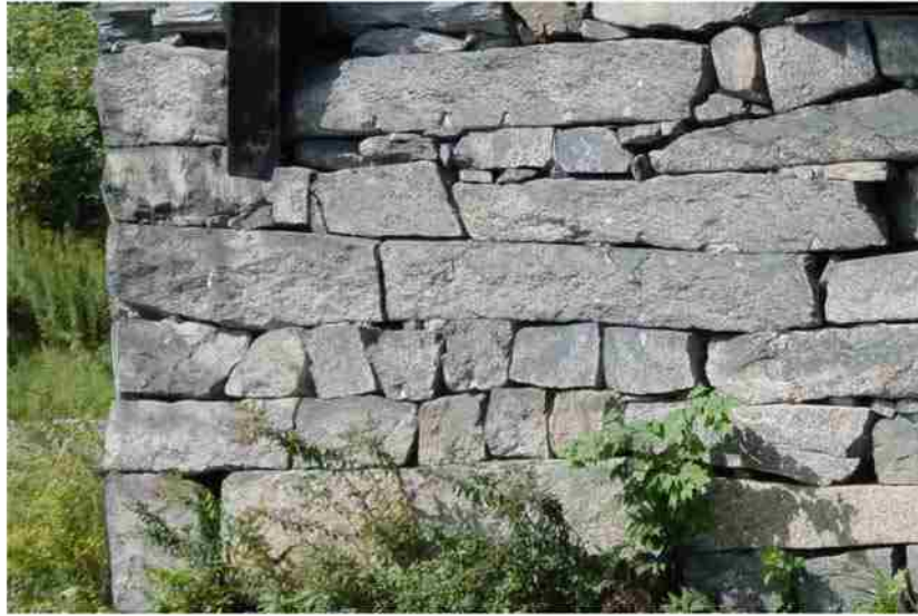
Detail of east face of Pier 2, Bath Village Bridge
