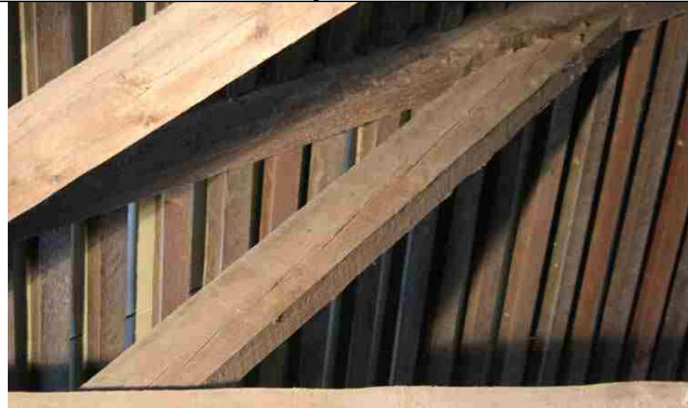
Photo No. 8-7 Knee Brace S49, Split
