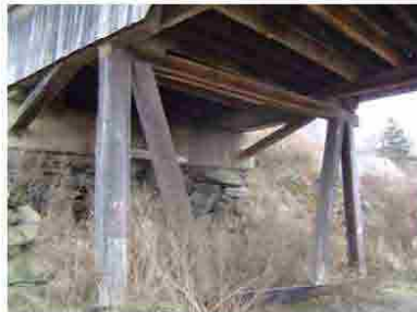
Timber Bents at West Span
