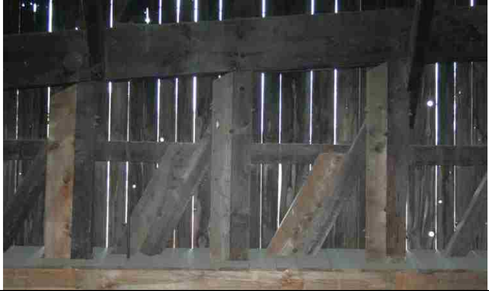
Photo No. 3-4 Vertical Truss Member N16, Spliced Members
