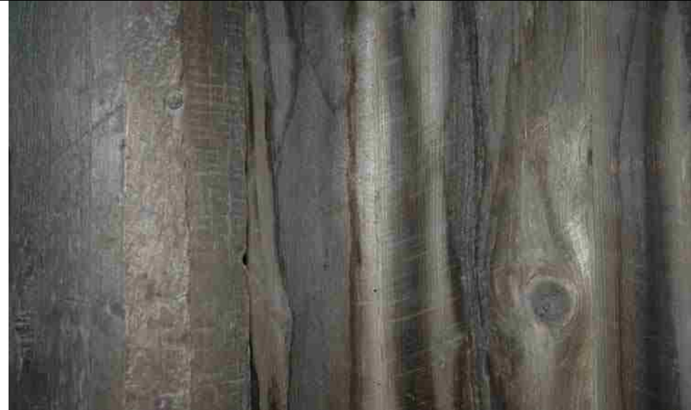
Photo No. 17-7: Post with vertical saw marks; siding board with circular saw marks
