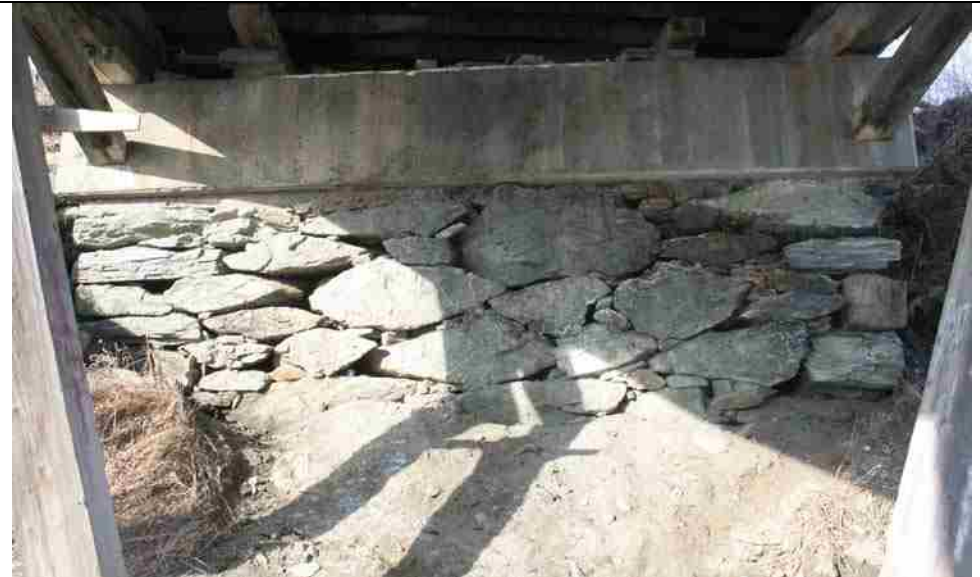
Photo No. 24-3 Abutment, West
