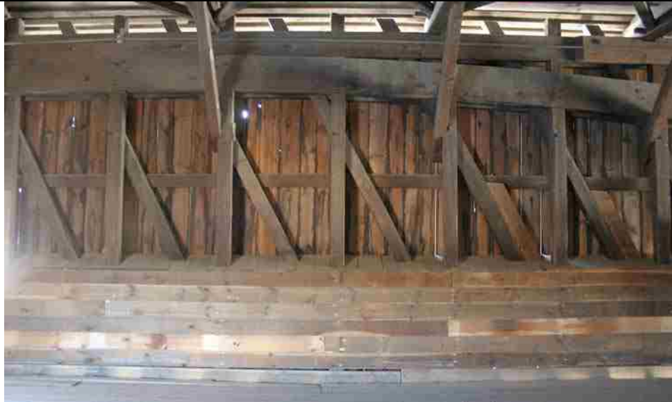
Photo No. 5-6 Built In Arch S22 – S18
