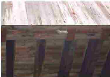
Span 5, North Lower Chord
