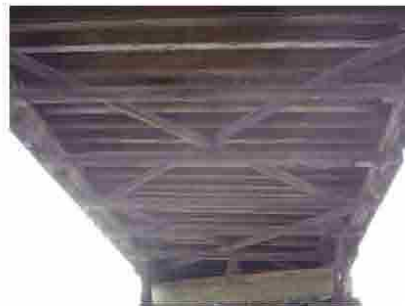
Typical Floor Framing
