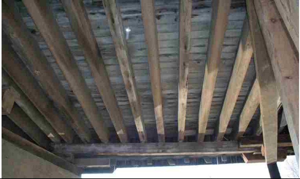
Photo No. 13-6 Floor Beams, Bent 3 – Pier 1
