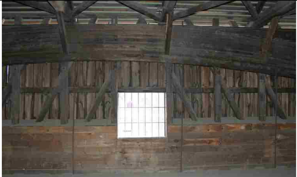
Photo No. 19-4 Added Arch S79 – S75
