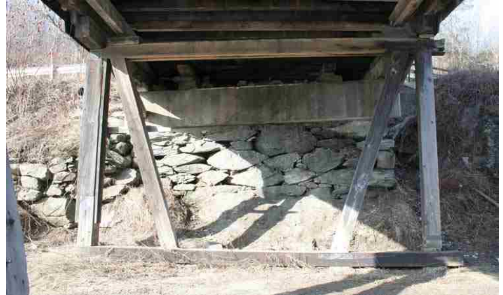
Photo No. 25-2 Bent 1
