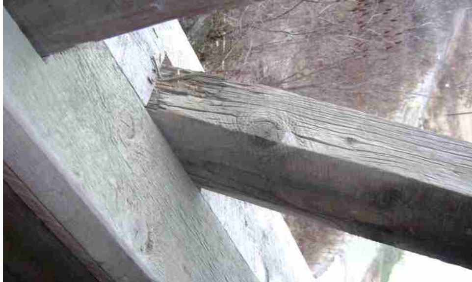
Photo No. 4-8 Diagonal N3L – N4U, Rot
