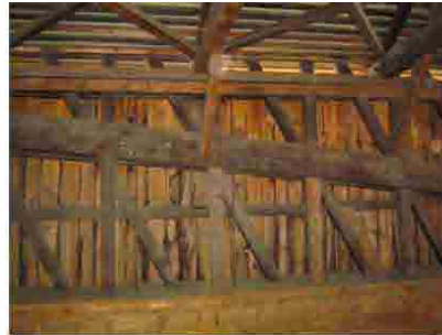
Typical Truss Section
