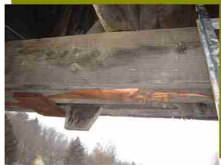
North Truss Near Node 17
