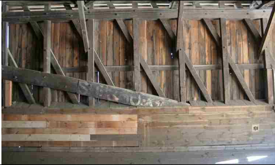
Photo No. 5-8 Built In Arch S10 – S6
