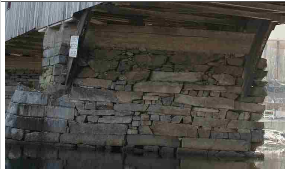
Photo No. 23-3 Pier 2 North
