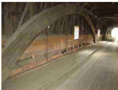
Added Arch and Original Arch (Behind Siding)
