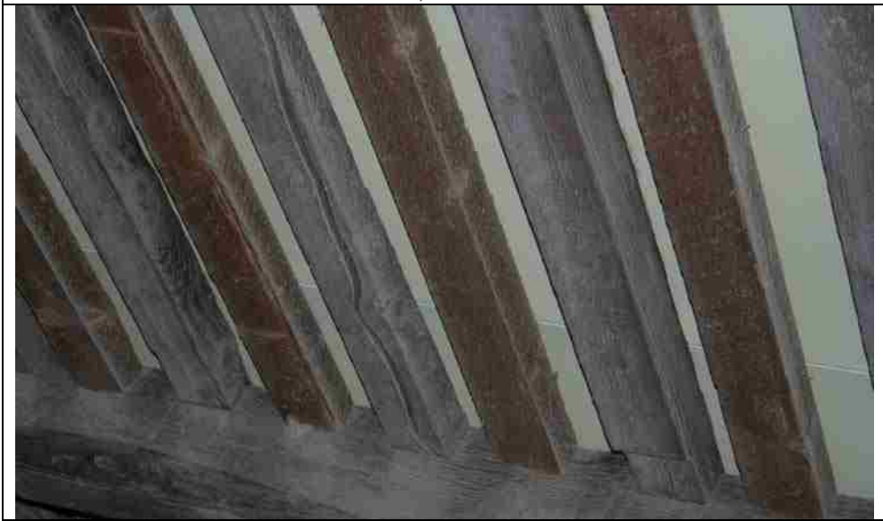
Photo No. 11-3 Purlin at node S85, Crack
