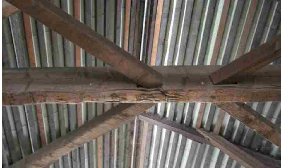
Photo No. 7-3 Upper Lateral S27– S29, Laterals joined to cross beam
