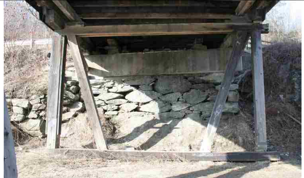
Photo No. 24-2 Abutment, West
