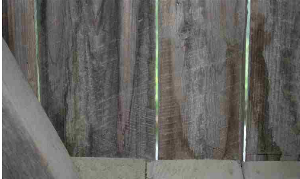
Photo No. 17-9: Double circular saw marks (cross-hatch) on 9-.5" & 7.5" boards
