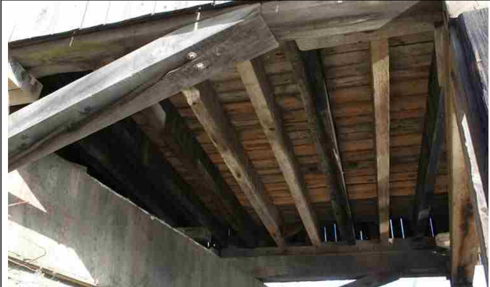
Photo No. 13-3 Floor Beams, West – Bent 1
