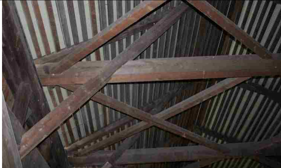
Photo No.8-2 Knee Brace S29, Split
