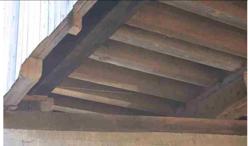
Photo No. 13-7 Floor Beams, N24 – N26
