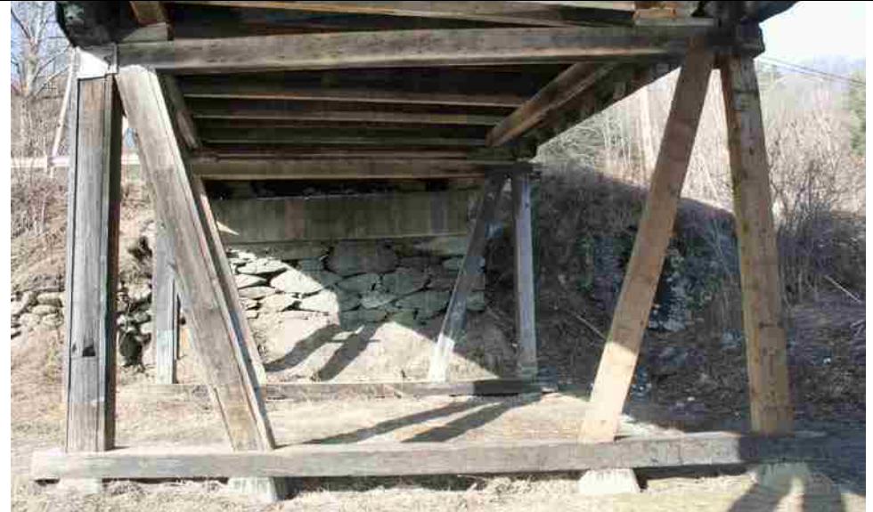
Photo No. 25-3 Bent 2
