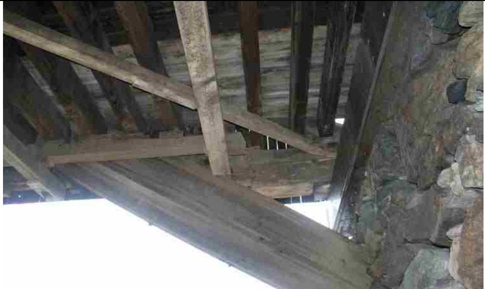
Photo No. 24-4 Abutment, East
