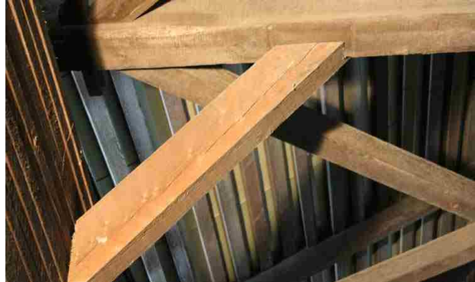
Photo No. 8-6 Knee Brace S49, Split
