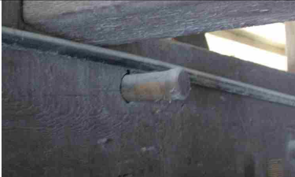
Photo No. 12-2 Trunnel S75, Popped out
