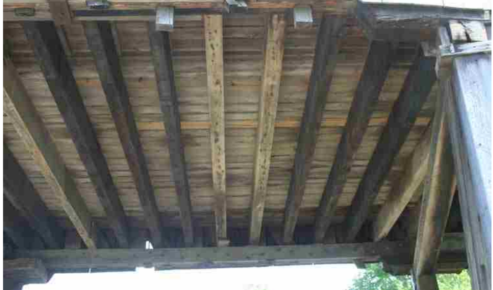
Photo No. 13-2 (6.17.09) Floor beams, dark new 1988; lighter are older
