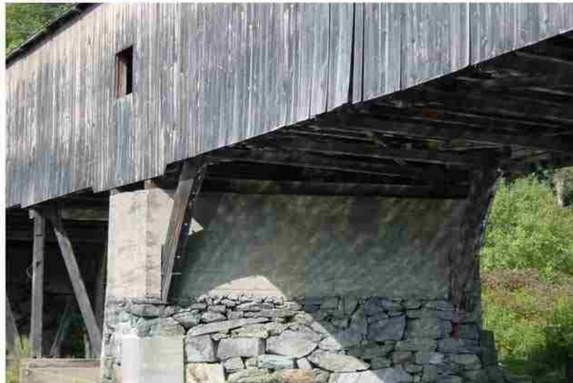
East face of Pier 3, Bath Village Bridge
