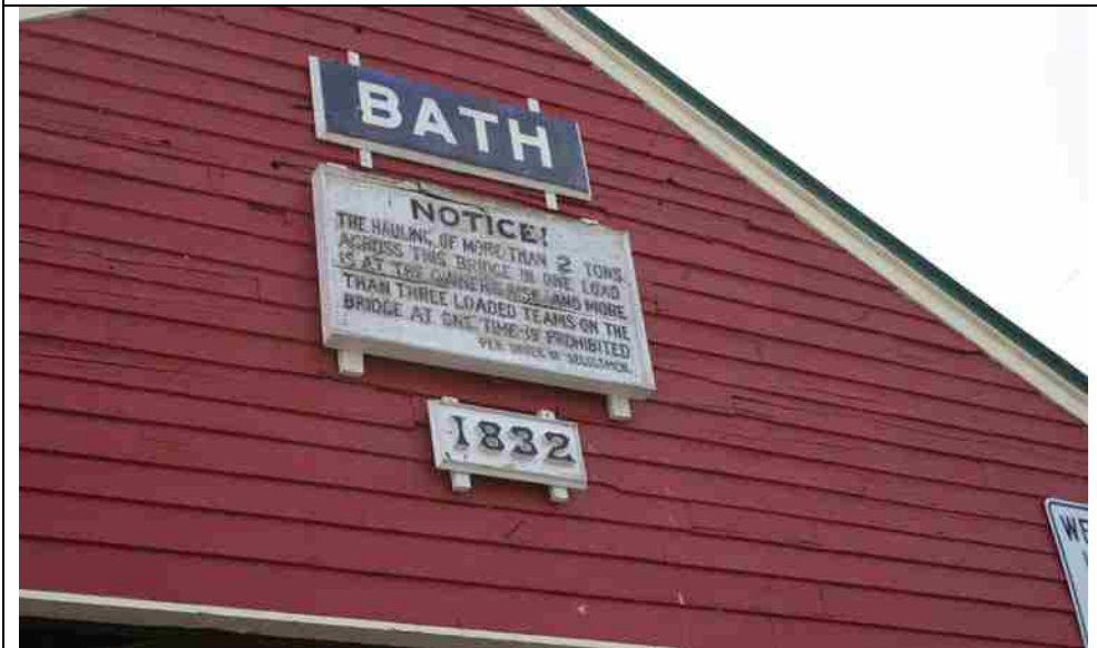
Photo No. 16-4 East Portal detail.
