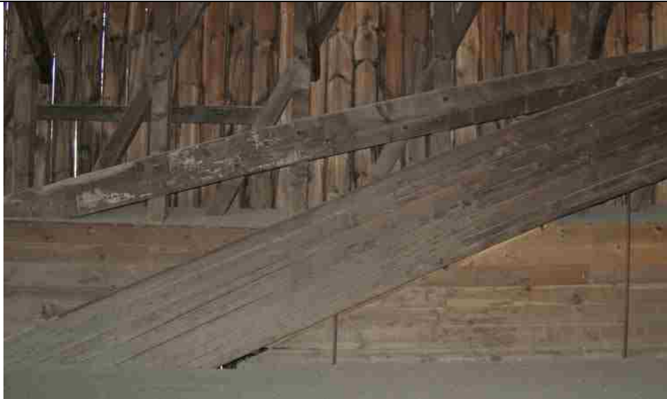
Photo No. 5-3 Built In Arch S90 – S86
