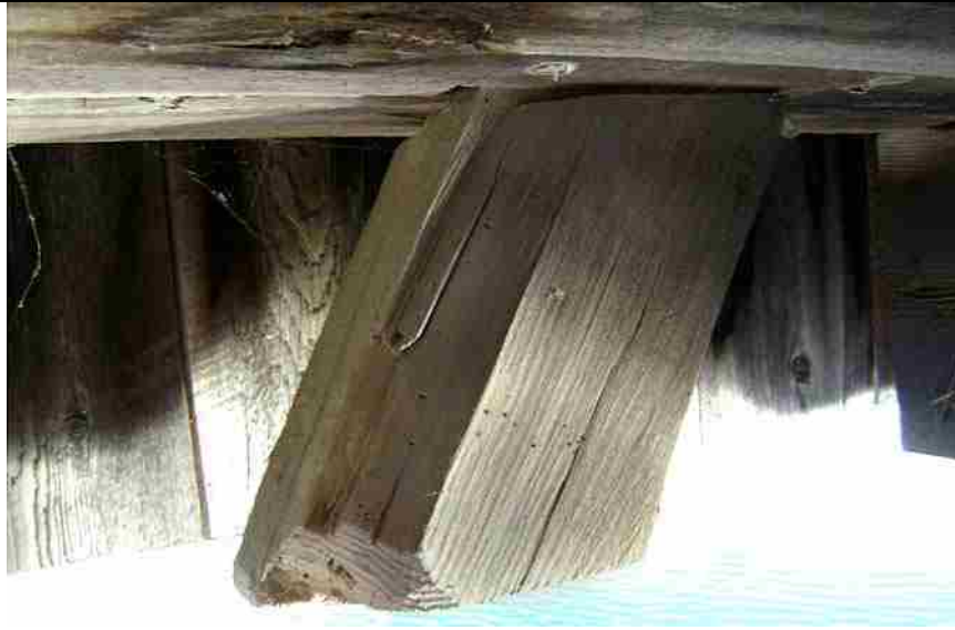
Photo No. 4-16 N73L-N74U, Split at Base, Waning
