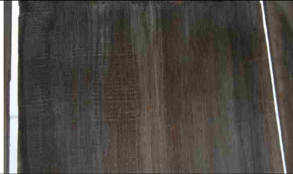
Photo No. 17-6: Detail of 15-1/2" board @ Post N10-N11 showing vertical saw marks
