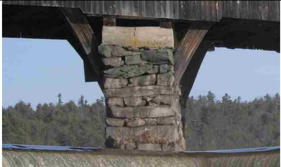
Photo No. 23-4 Pier 2 South
