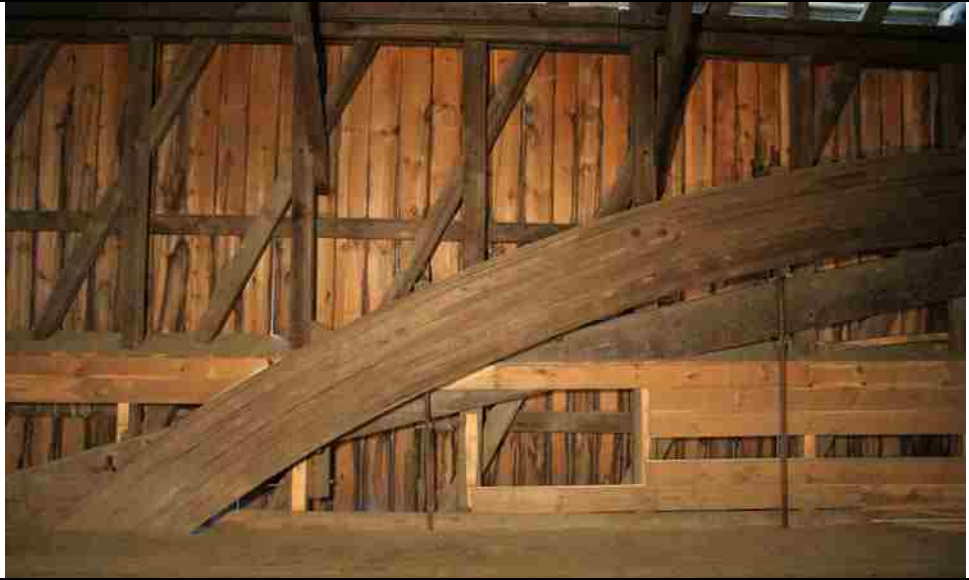
Photo No. 5-4 Built In Arch S40 – S34
