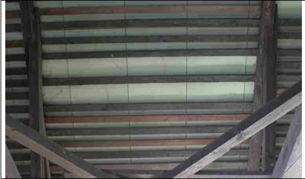
Photo No. 11-3 Purlin at node S85, Crack
