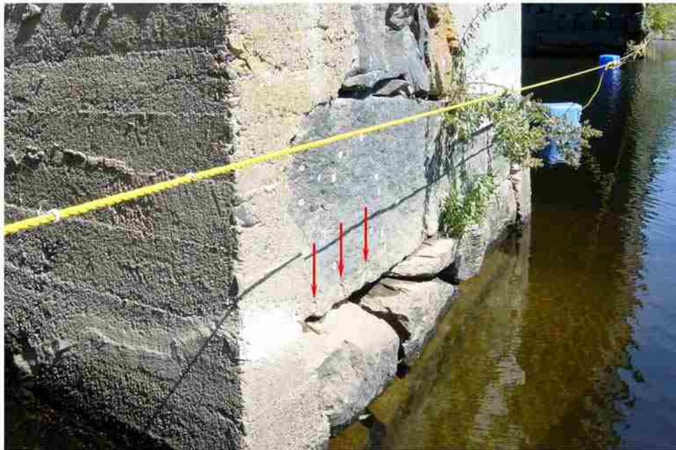
South face of Pier 3, Bath Village Bridge
