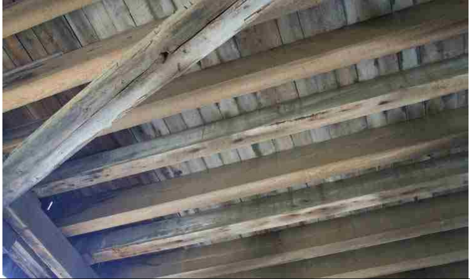
Photo No. 13-5 Floor Beams,
