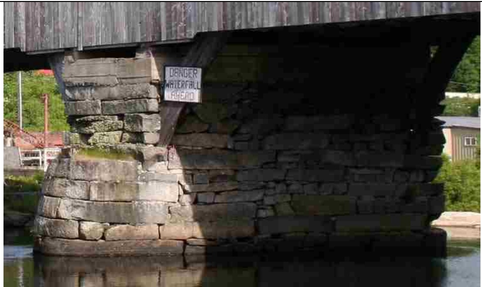
Photo No. 23-5 Pier 2 North
