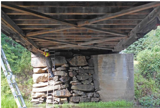
Floor beams span between lower chords.
