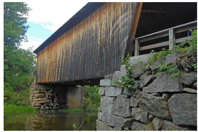
South abutment, downstream side at left; north abutment visible across river.
