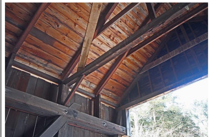
North Portal inside
