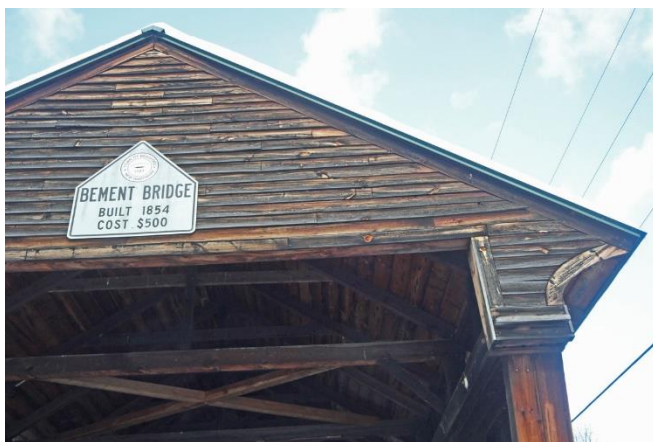
South Portal detail
