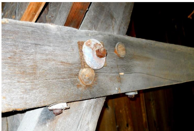
Crack in upper chord at Node 3. Note added vertical thru bolt reinforcement.
