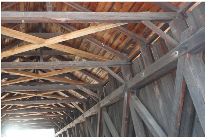
Oblique view of west truss showing braces and counter braces in X between posts.
