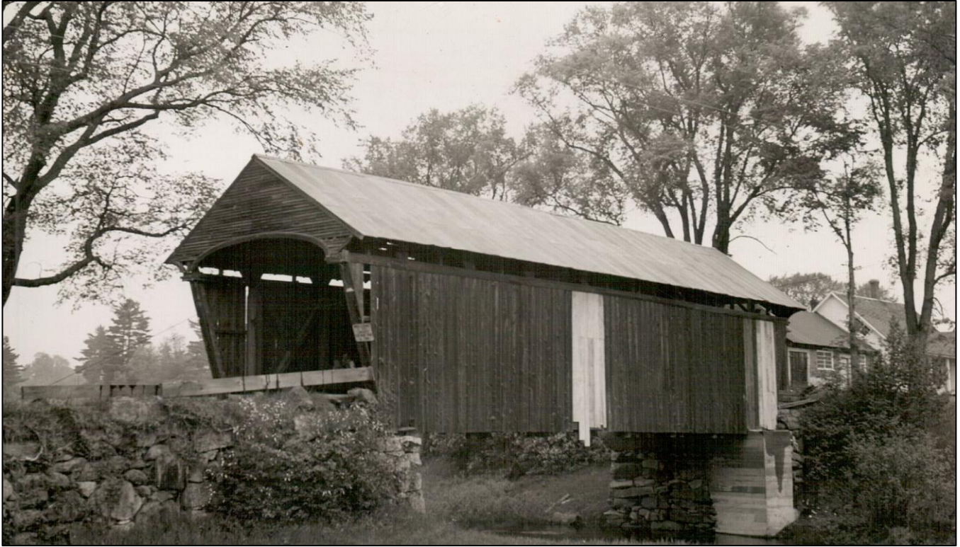
FIGURE 10: Bement Bridge, south portal and downstream (east) side, 1942, showing north abutment repaired with cast-in-place concrete, repairs to wood siding and to corrugated sheet metal roof (NHHD Bridge Inventory Card 5/20/1942).
