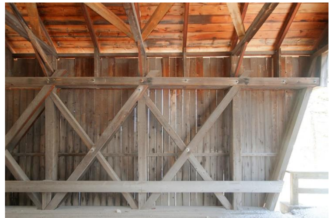
Rectified view of posts of west truss, north end
