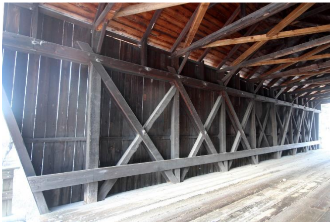
Oblique view of west truss with eight posts
