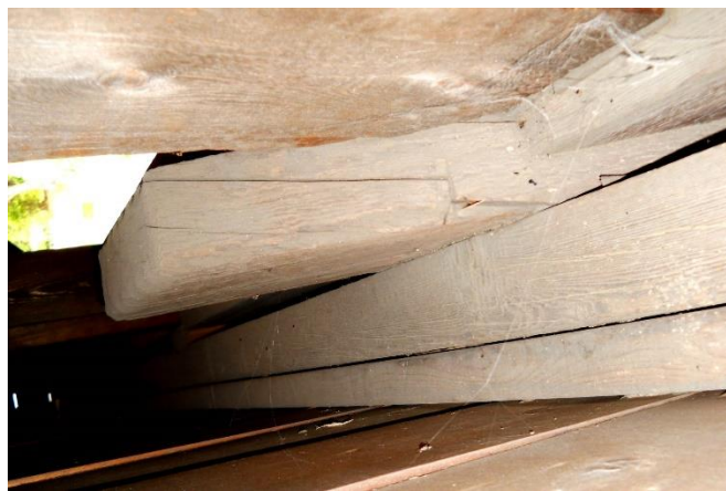
Counter brace with w/ structural split at Node 1 to be replaced.
