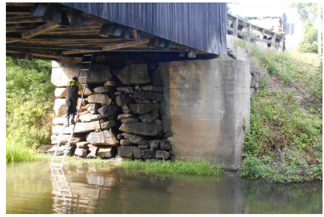
North Abutment, showing concrete repair and upstream side.
