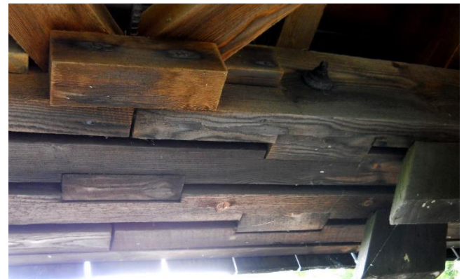
Critical lower chord splice joints adjacent to Node 6 post.
