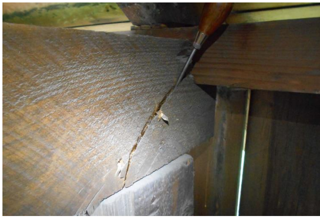
Cracked cross beam end at Node 1, west truss.
