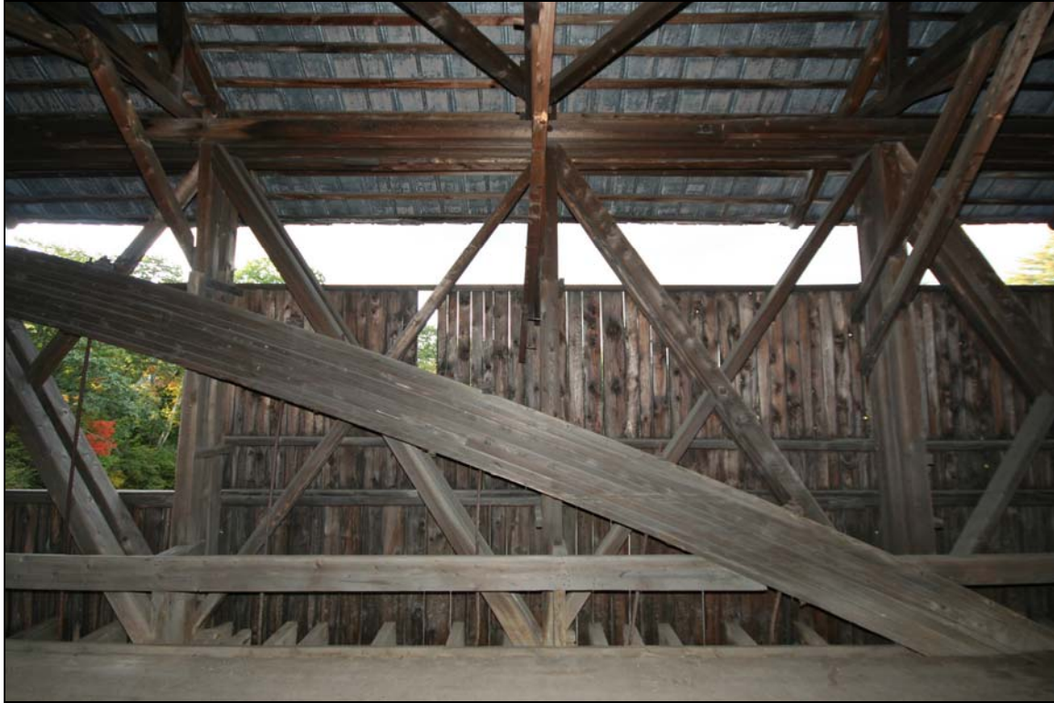
Photo No. 7: South truss and arch of west span. View south.
