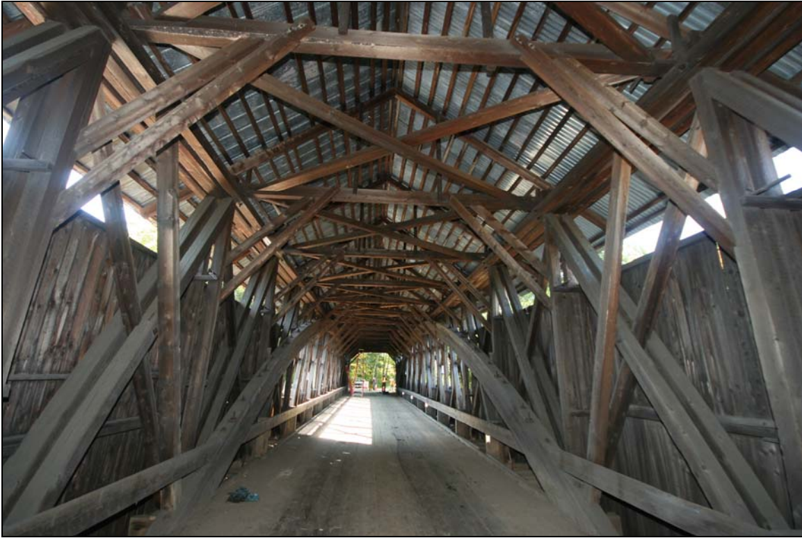
Photo No. 1: Interior view of bridge. View W.
