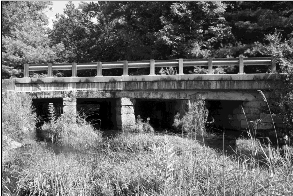
Photo No. 3: This four-span stone slab structure (Amherst Bridge 159/105) once carried Boston Post Road over Beaver Brook in Amherst, NH. It provides an example of the variability in assigning the term culvert or bridge to certain structures. On the basis of the length of the individual spans, which do not exceed 8 feet, it can be labeled a four-barrel stone box culvert. But with a primary function to convey traffic, the absence of an overlying filled embankment, and most importantly, the need to regularly inspect the structure due to its greater susceptibility to catastrophic collapse than a single channel culvert, it was designated a bridge by NHDOT. This large and very rare example of a stone culvert with more than two spans is now bypassed by a modern bridge.
