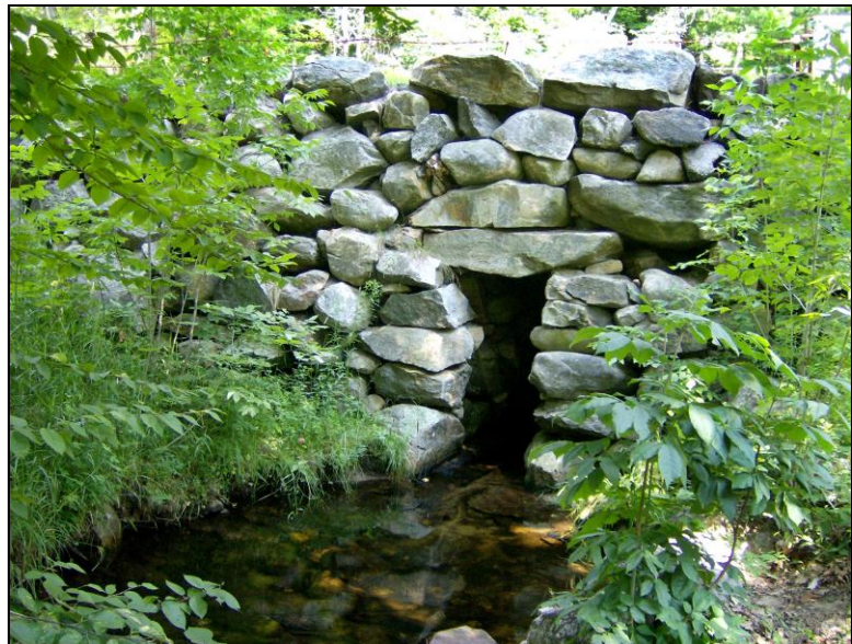
Photo No. 22: Box culvert of dry-laid fieldstone very randomly laid.
