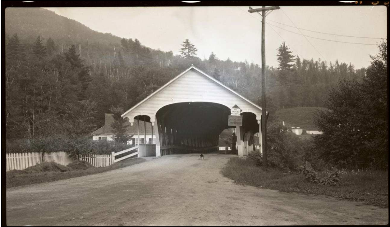
Figure 12: Photo dated August 28, 1948, prior to construction of pier. Note sag in bridge seen in the roadway guardrail. (Source: Collection of the National Society for the Preservation of Covered Bridges).
