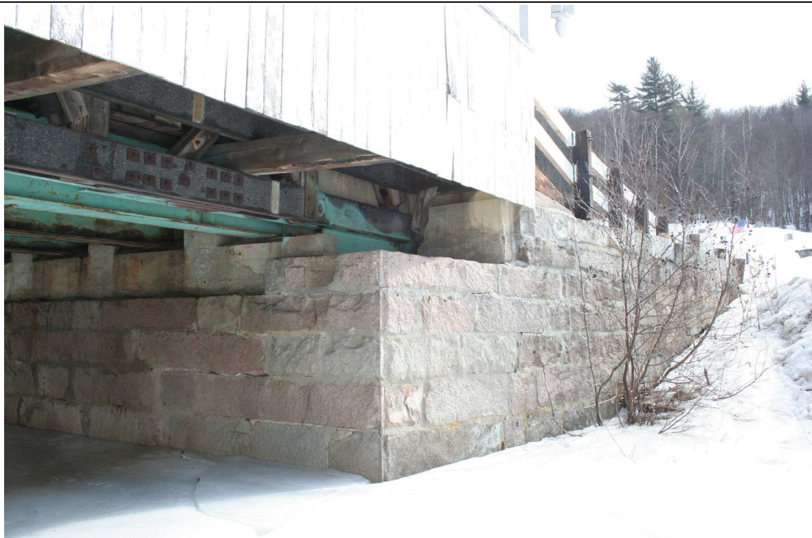
FIGURE: 4.2.1-6: South abutment, face and downstream corner
