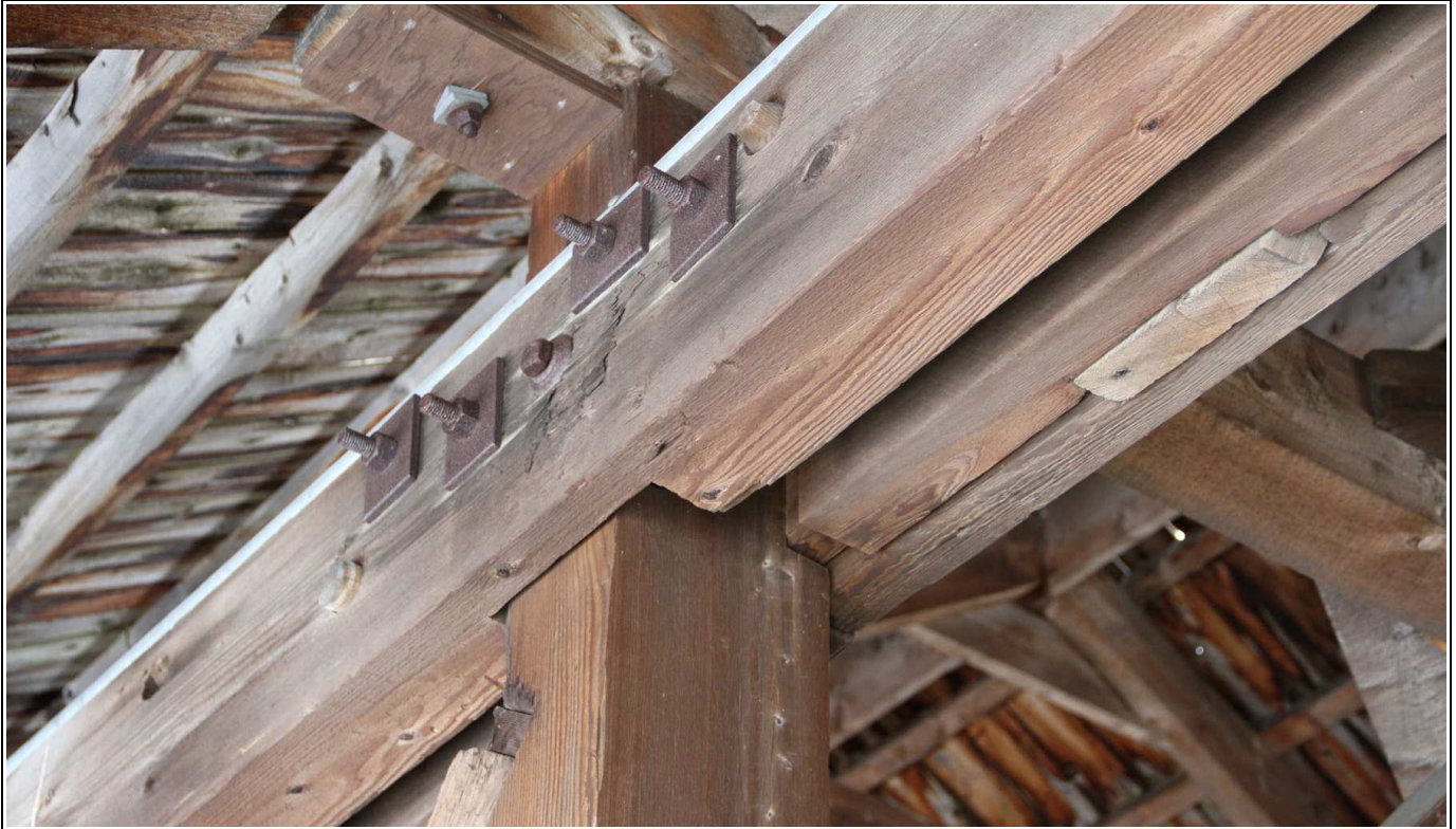
FIGURE: 4.2-3: Upper chord connection to posts showing wood trunions and thru-bolts.
