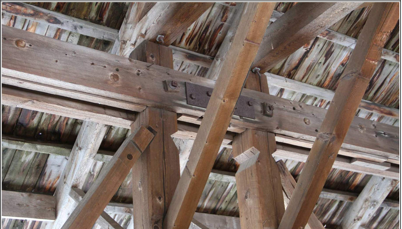
FIGURE: 4.2-6: Upper chord at mid-span showing bolted steel plate splice connection.
