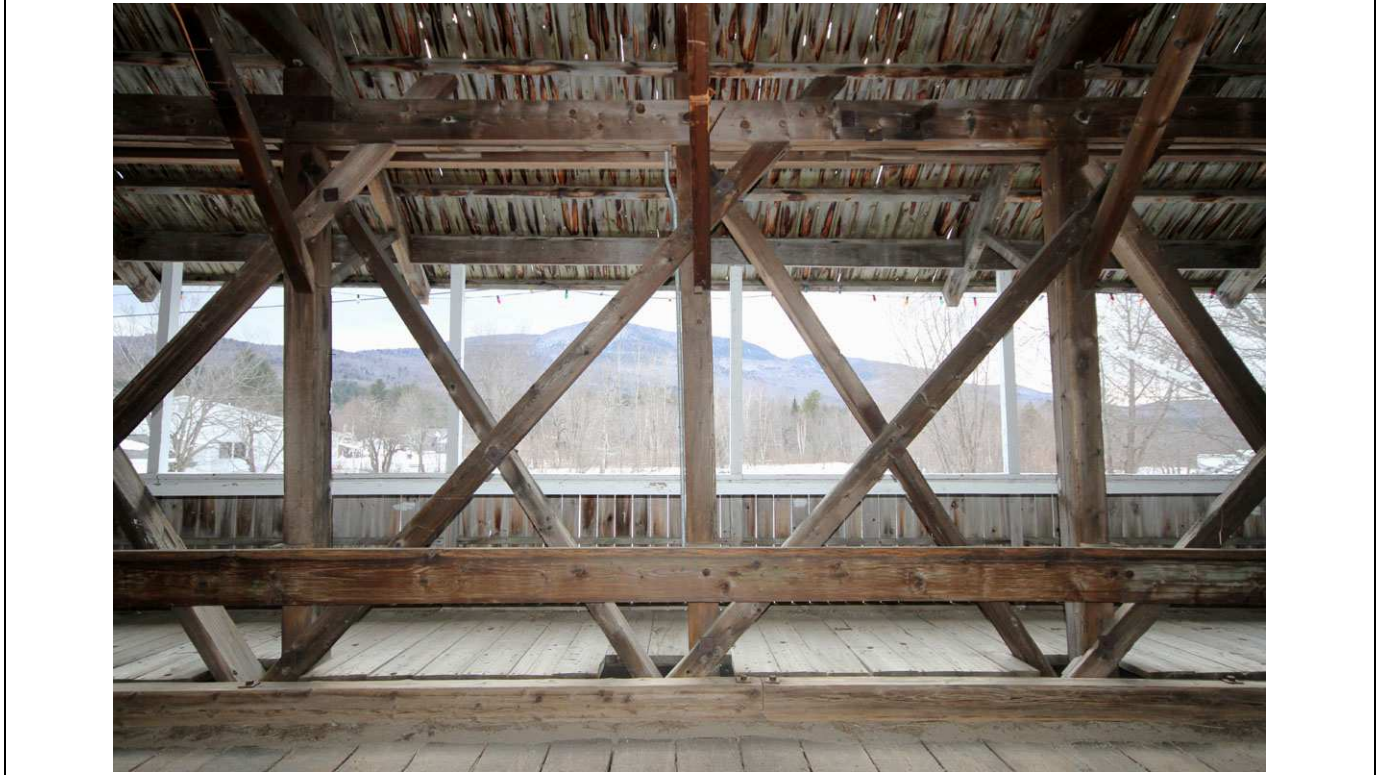
FIGURE: 4.4-4: Overall view of verticals (posts).
