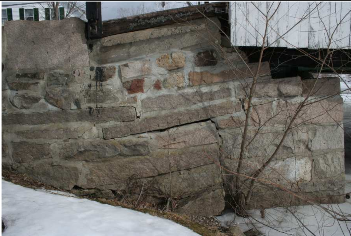
FIGURE: 4.10-6: Detail of north abutment, downstream wingwall.
