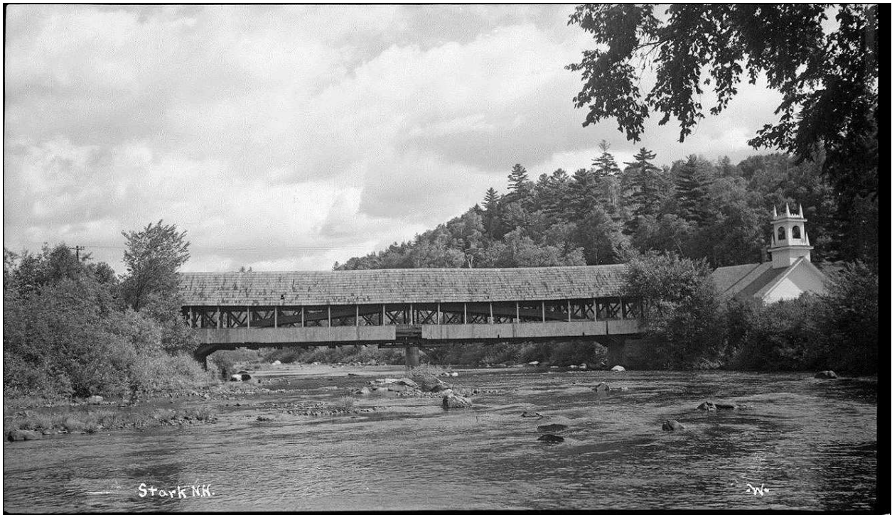
Figure 15: Photo of downstream side of bridge, circa 1950. New pier supporting bridge visible under removed siding. (Source: Collection of the National Society for the Preservation of Covered Bridges).
