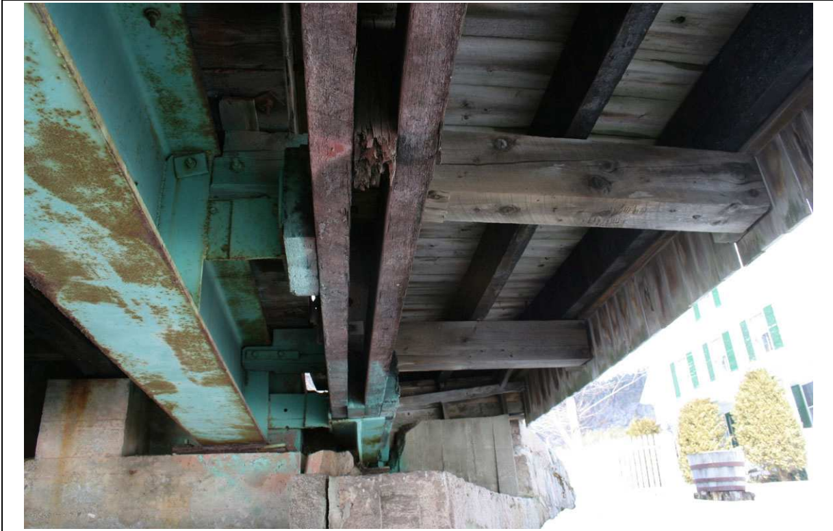
FIGURE: 4.9-3: Underside of sidewalk showing cantilevered floor beams and stringers.
