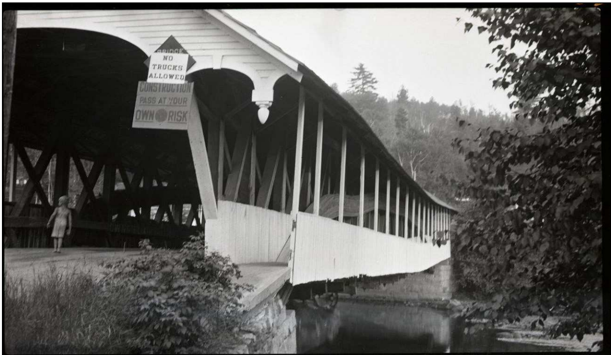
Figure 13: Photo dated August 28, 1948, prior to construction of pier. Note deformed arch. (Source: Collection of the National Society for the Preservation of Covered Bridges).
