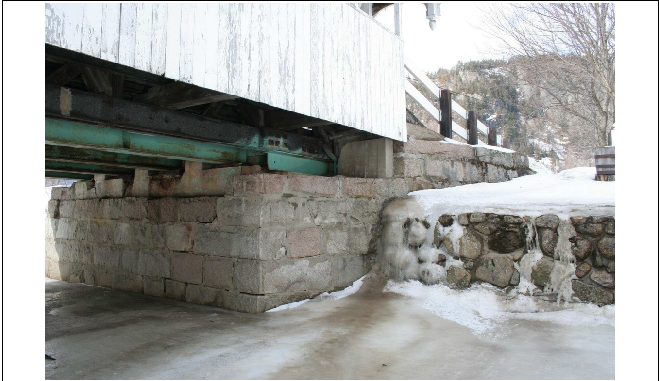
FIGURE: 4.10-2: North abutment, upstream corner.
