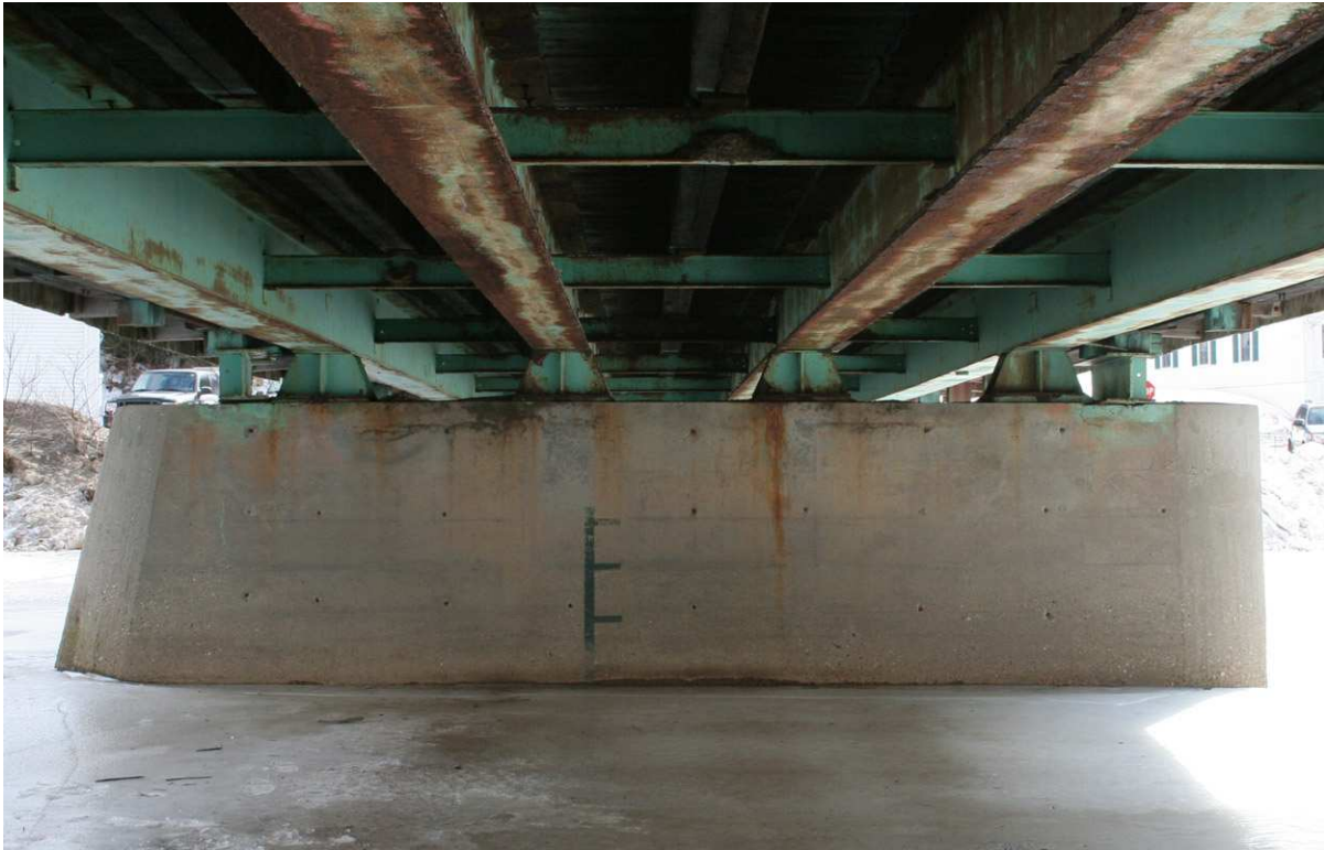
FIGURE: 4.11-5: Elevation view of pier and bearings.
