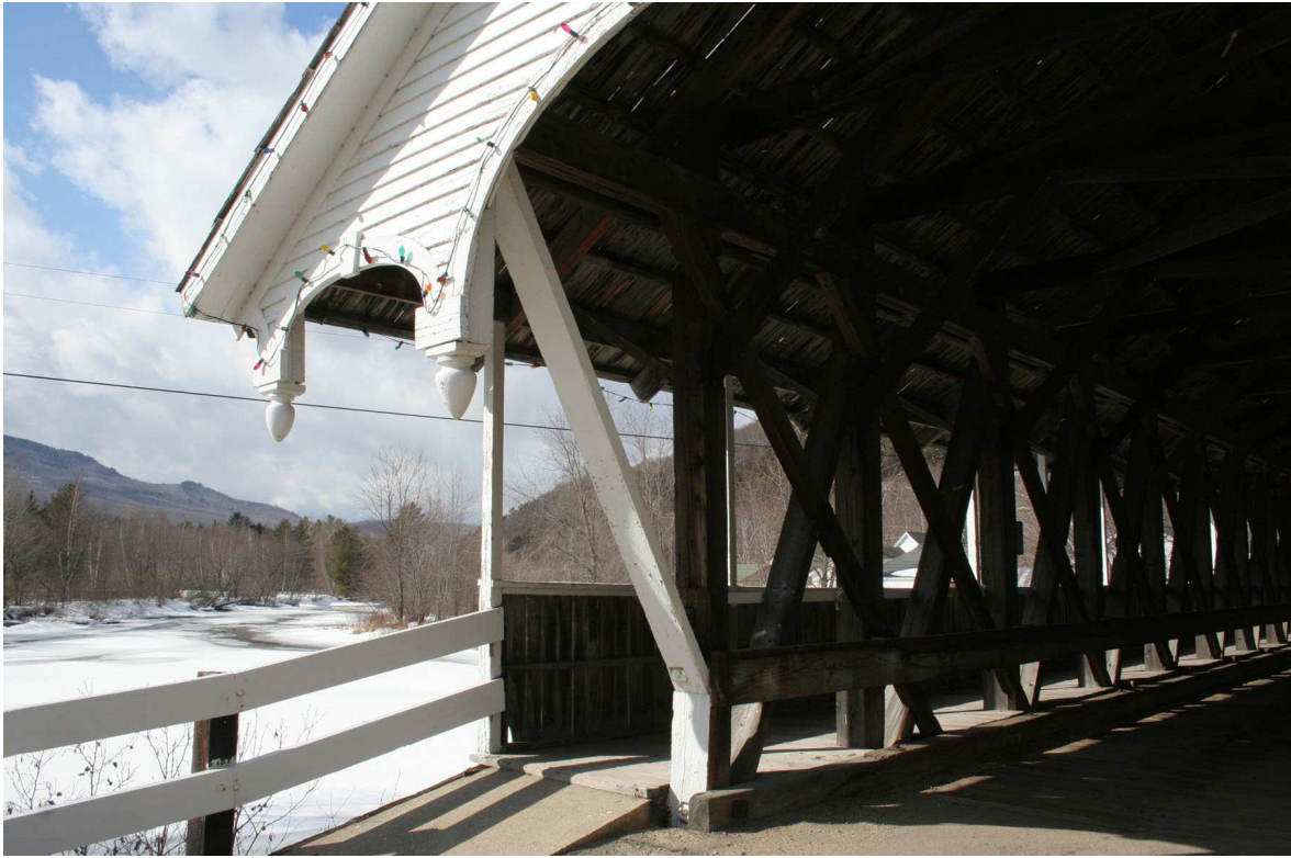
FIGURE: 4.12-3: Detail of projected portal wall.
