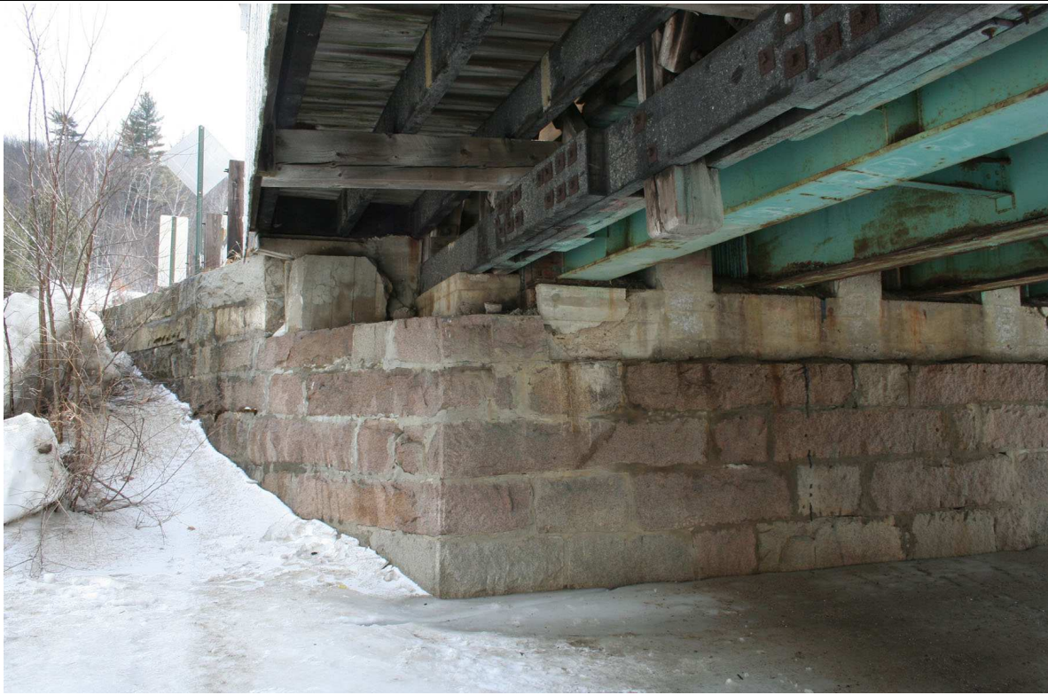
FIGURE: 4.2.1-5: South abutment, face and upstream corner
