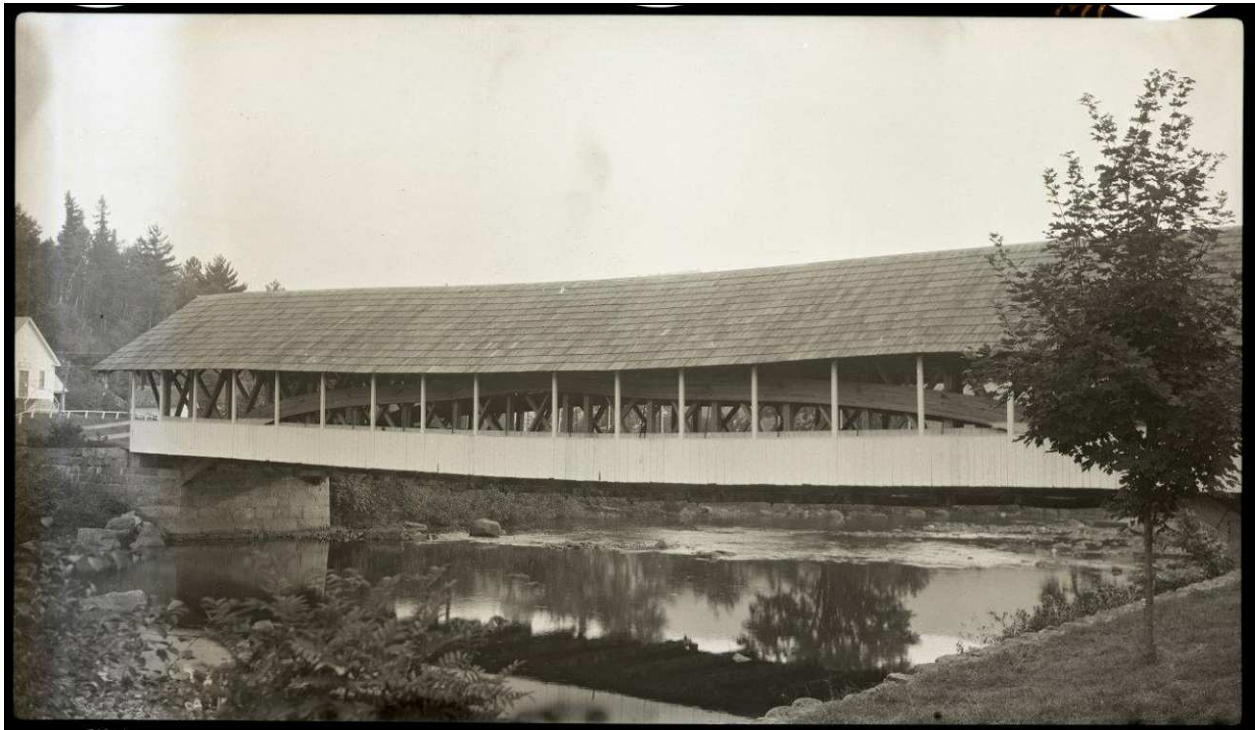
Figure 11: Photo dated August 28, 1948, just prior to construction of the center concrete pier (Source: Collection of the National Society for the Preservation of Covered Bridges).
