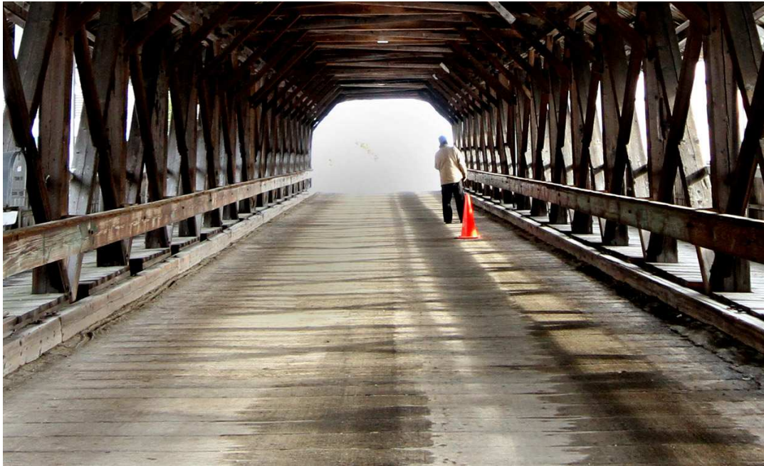
FIGURE: 4.8-1: Bridge floor.
