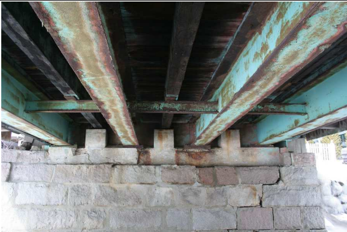
FIGURE: 4.11-5: Elevation view of pier and bearings.
