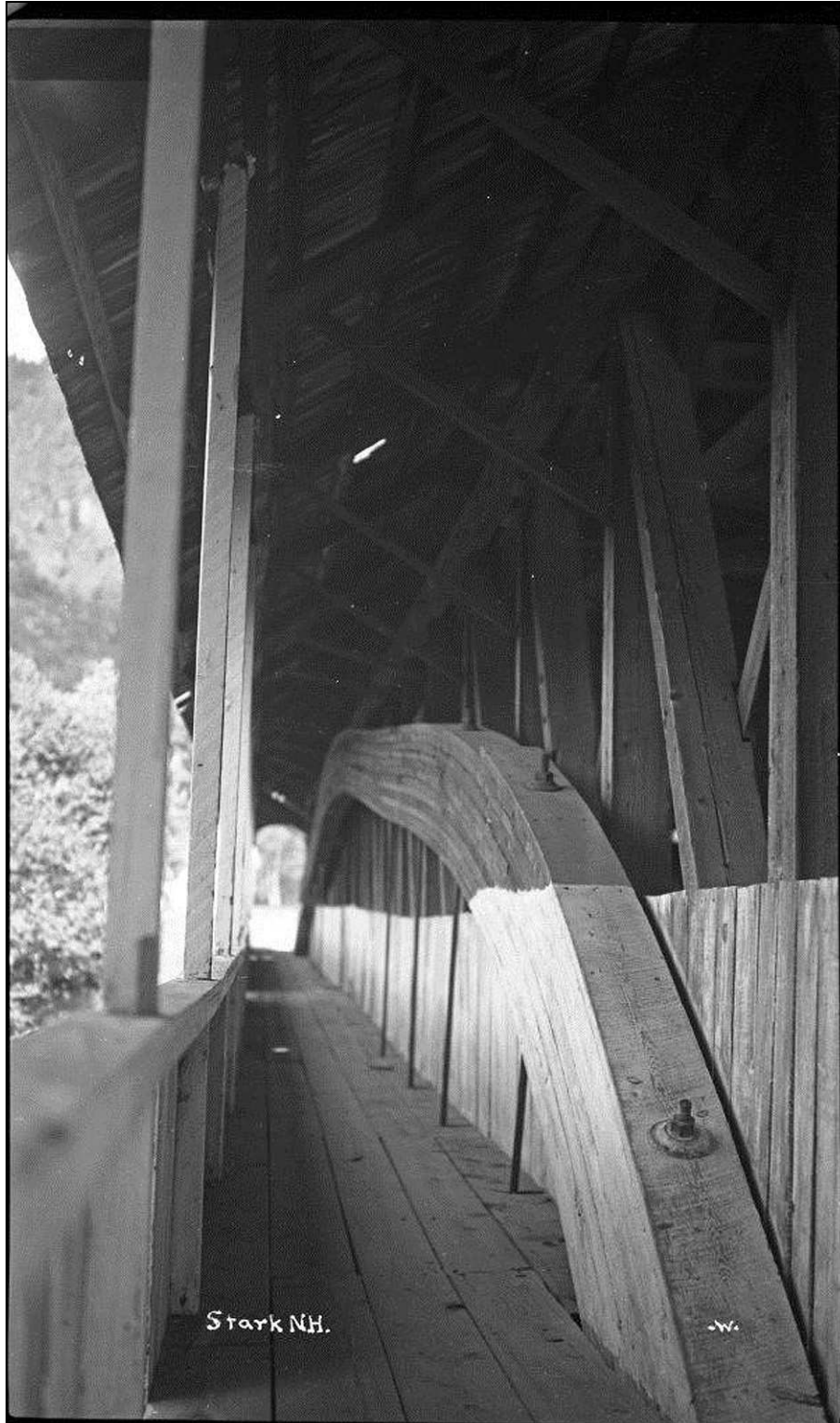
Figure 18: Photo of arch and sidewalk, circa 1950. (Source: Collection of the National Society for the Preservation of Covered Bridges).
