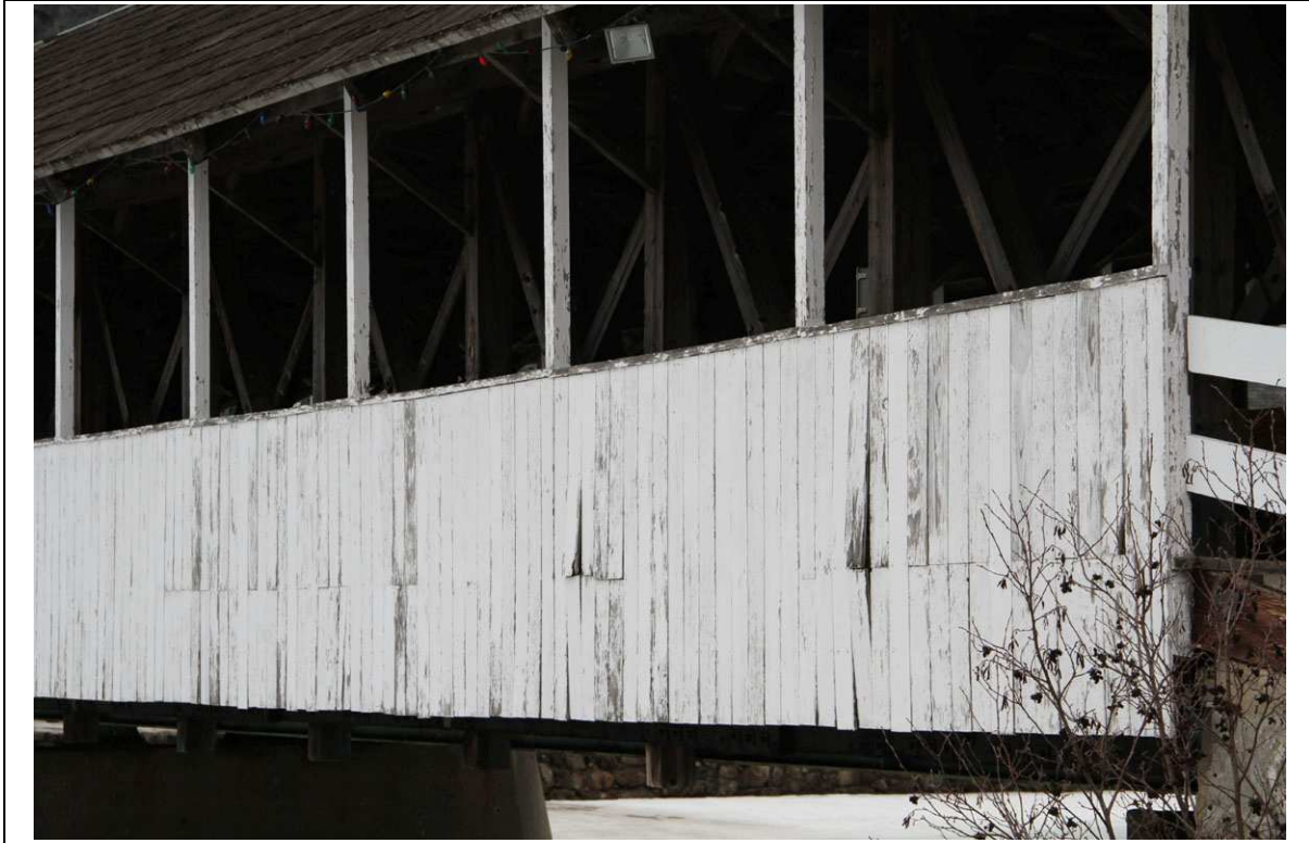
FIGURE: 4.9-5: Vertical wood siding railing on sidewalk.
