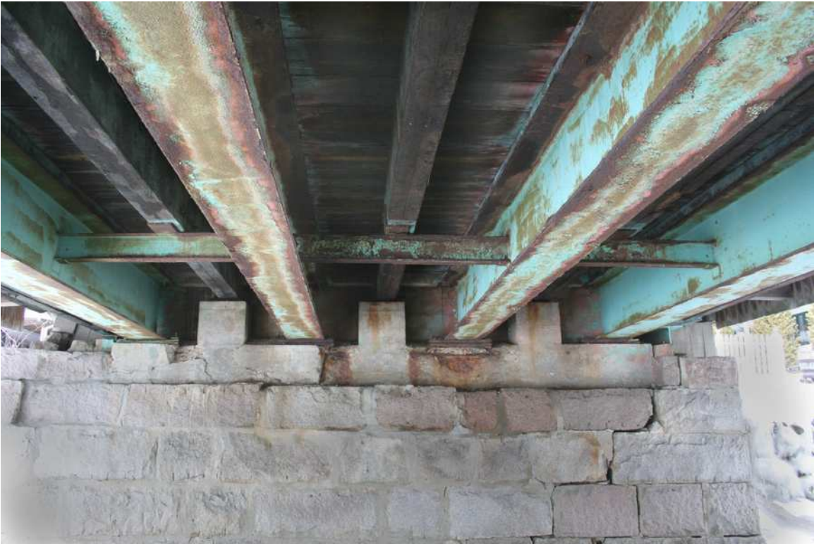
FIGURE: 4.1-3: I-beam stringers, diaphragms and intermediate stringers.
