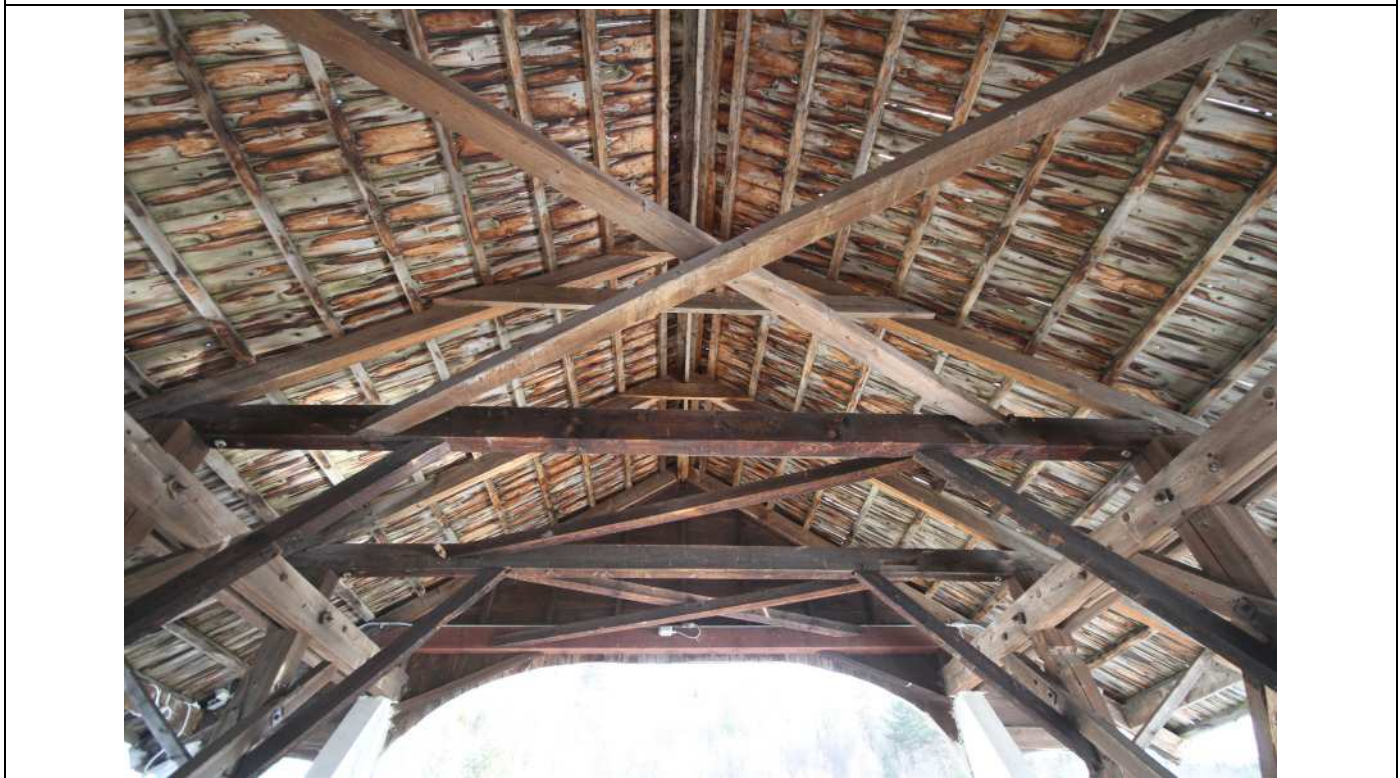
FIGURE: 4.7-3: Overall view of roof system.
