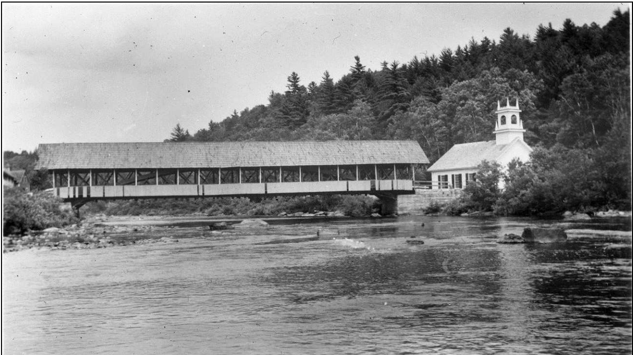
Figure 4: Early 20th century view (ca. 1925) of west elevation of Stark Bridge before bridge began sagging in the 1930s. Note missing siding boards. (Source: Collection of the National Society for the Preservation of Covered Bridges).
