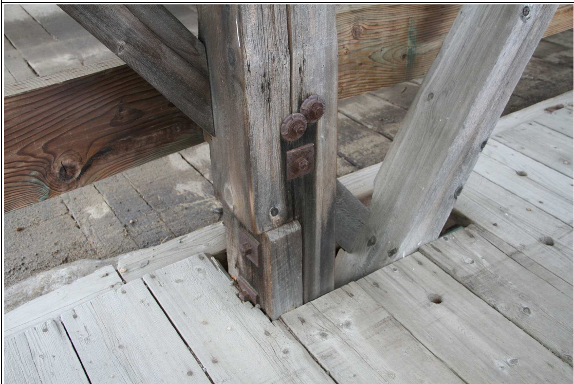
FIGURE: 4.4-8: Vertical with splice at bottom
