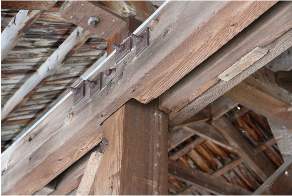
FIGURE: 4.4-5: Vertical connection to upper chord showing multiple thru-bolts.
