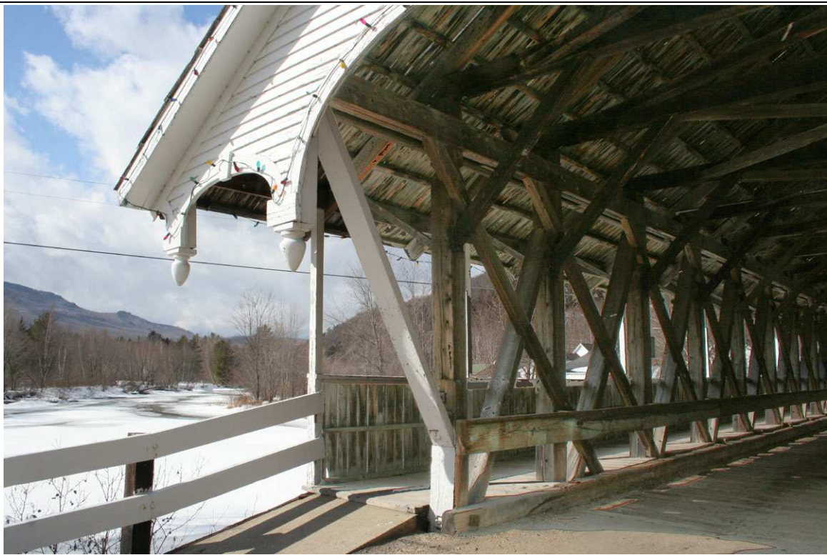
FIGURE: 4.9-4: Interior view of sidewalk.
