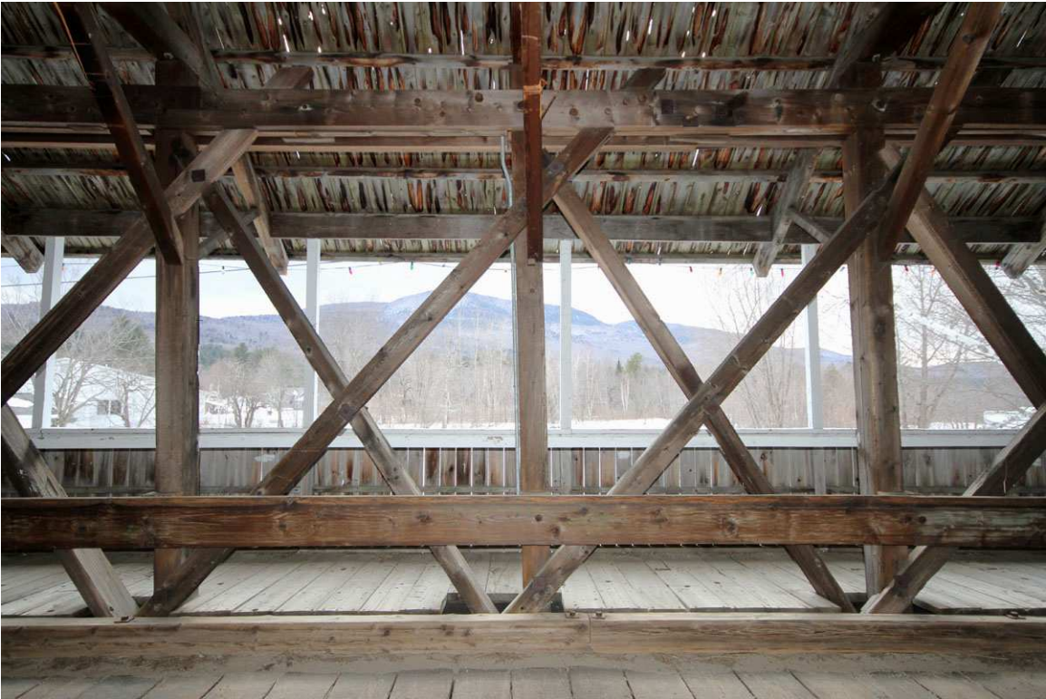
FIGURE: 4.5-3: Overall view of diagonals
