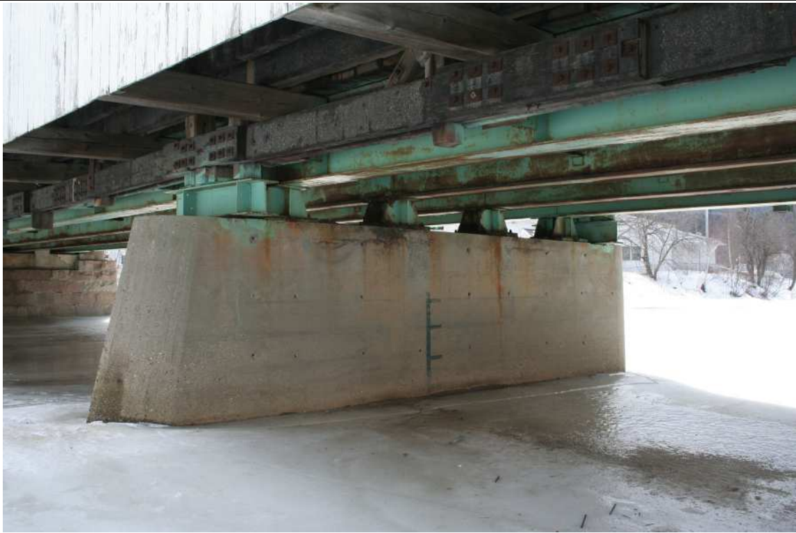
FIGURE: 4.11-4: View of pier and pedestal bearings.
